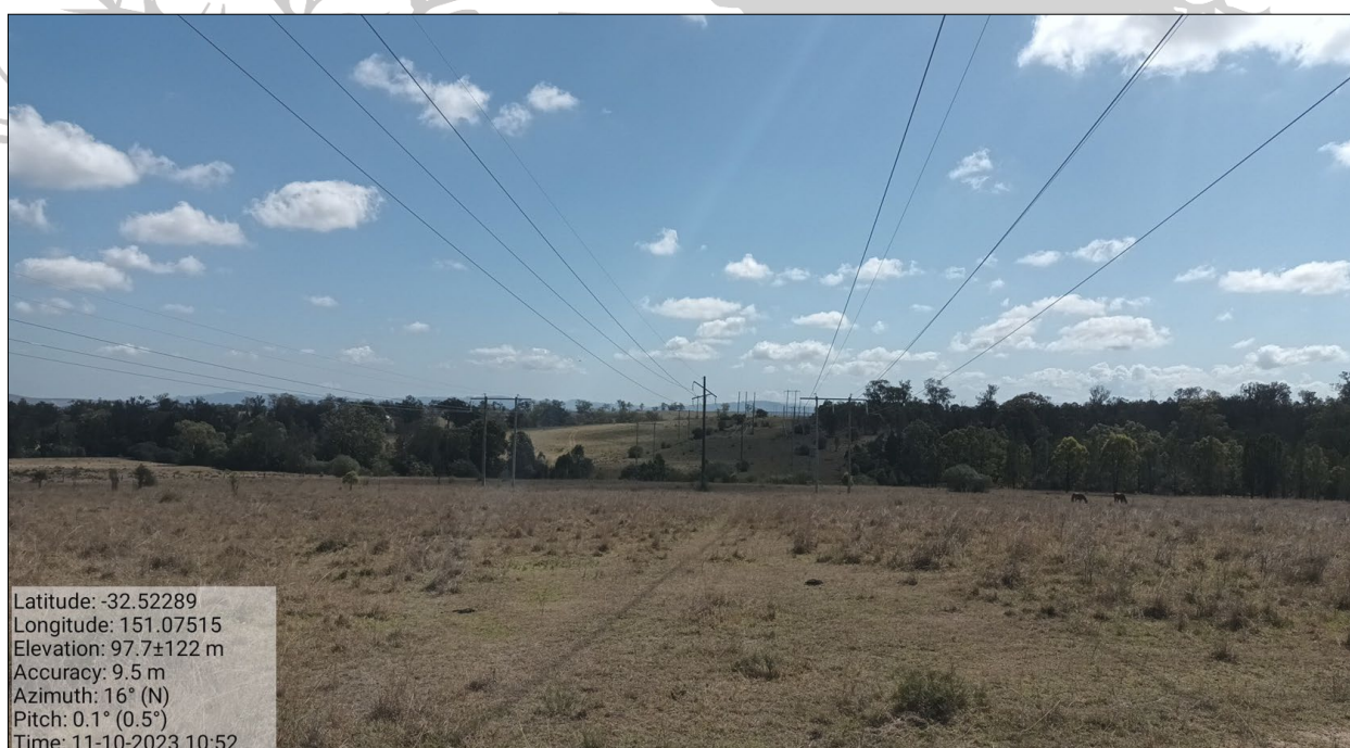
Plate 8: Existing transmission line easement running through the middle of the subject site (Photo Point 29)
