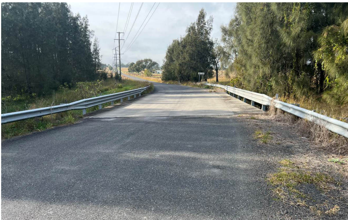
Plate 8 - Maison Dieu Road near Rix's Creek (culvert)
