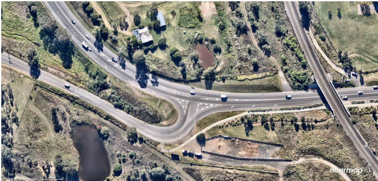
Plate 12 - New England Highway / Maison Dieu Road intersection.
