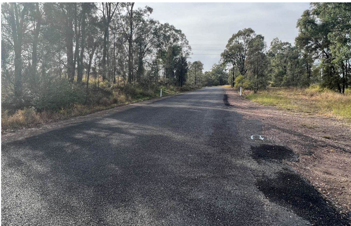
Plate 7 - Maison Dieu Road near site.
