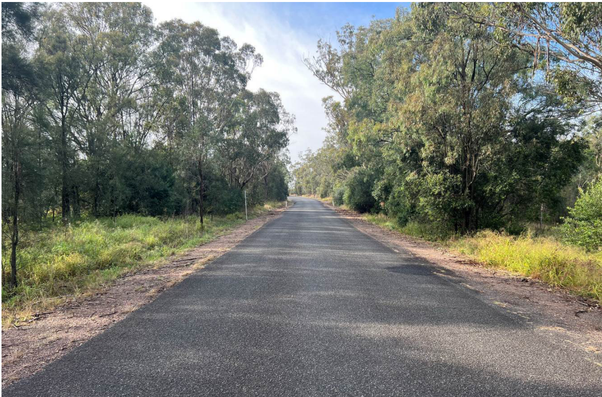
Plate 2 - Maison Dieu Road near proposed main site access A
