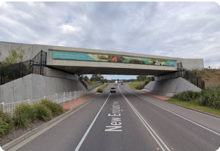
Below: Rail overpass at Gowrie Gates north west of Singleton - 5.6m height restriction
