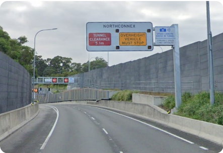
Above: M11 NorthConnex tunnel entrance at Pennant Hills - 5.1m height restriction
