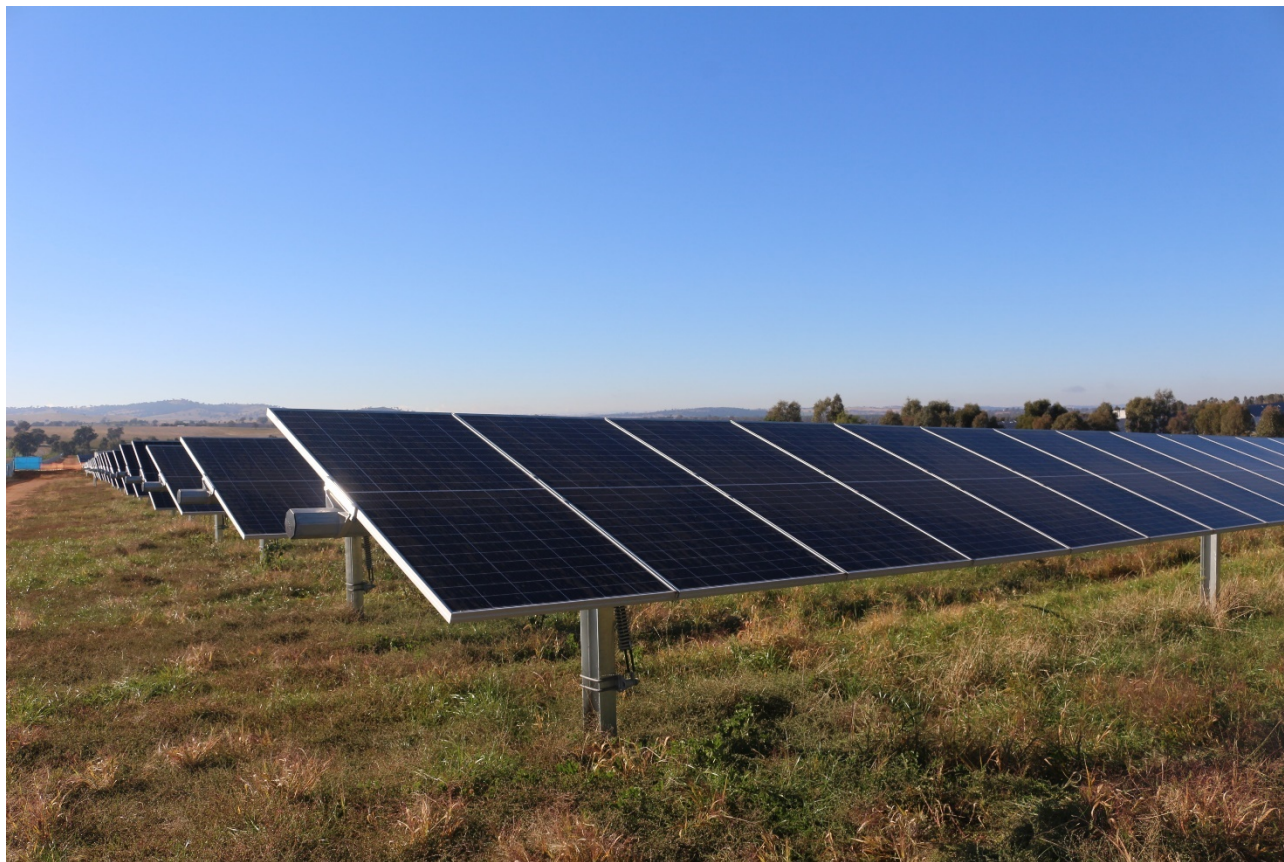
Photograph 3.1 Example of solar PV modules mounted to single axis tracking structures
