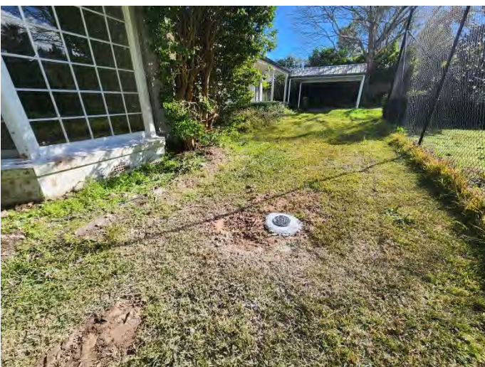
Plate 11 – View of the groundwater bore well MW1.
