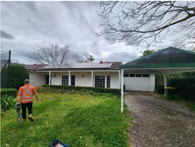
Plate 3 – View of 293 Mona Vale Road from the north.
