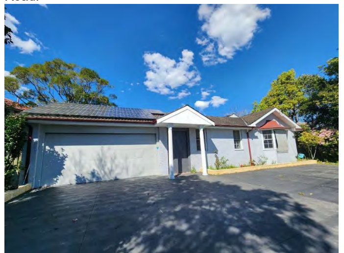
Plate 12 – View of the residence 295 Mona Vale Road
