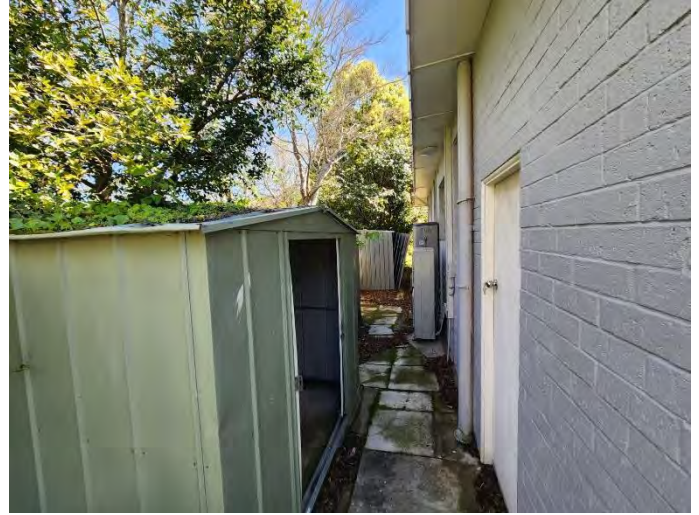
Plate 14 – View of shed adjacent to house (295 Mona Vale Road).
