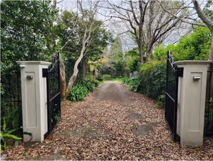
Plate 1 – Remote operated gate to enter 293 Mona Vale Road. The view is towards the east.
