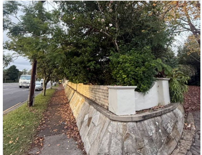
13. Existing boundary wall and vegetation along Mona Vale Road.
