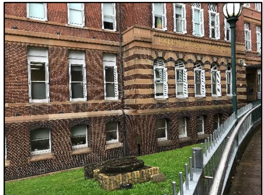
Figure 41. External view to details on the primary façade of the Albert Pavilion – note the banded brick and sandstone masonry.
