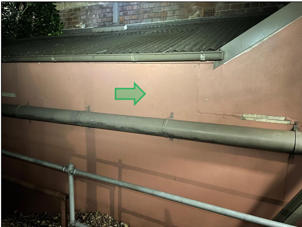
Photograph 6 Exterior non-asbestos fibre cement wall lining. Location of sample 'B94-EXT-WALL-A05'. No asbestos detected.
