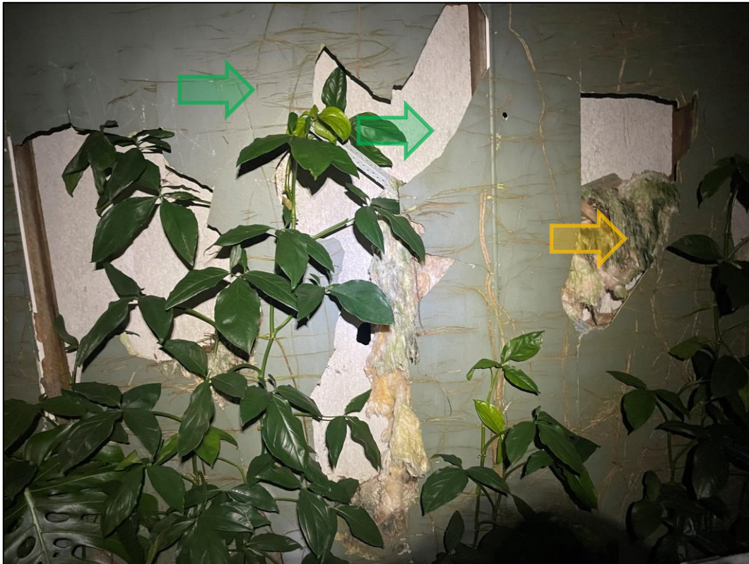
Photograph 7 External and internal non-asbestos fibre cement wall linings identified on the external shed. Location of samples 'B94-SHED-EXT-WALL-A03' and 'B94-SHED-EXT-WALL-A04'. No asbestos detected. Presumed SMF insulation observed.
