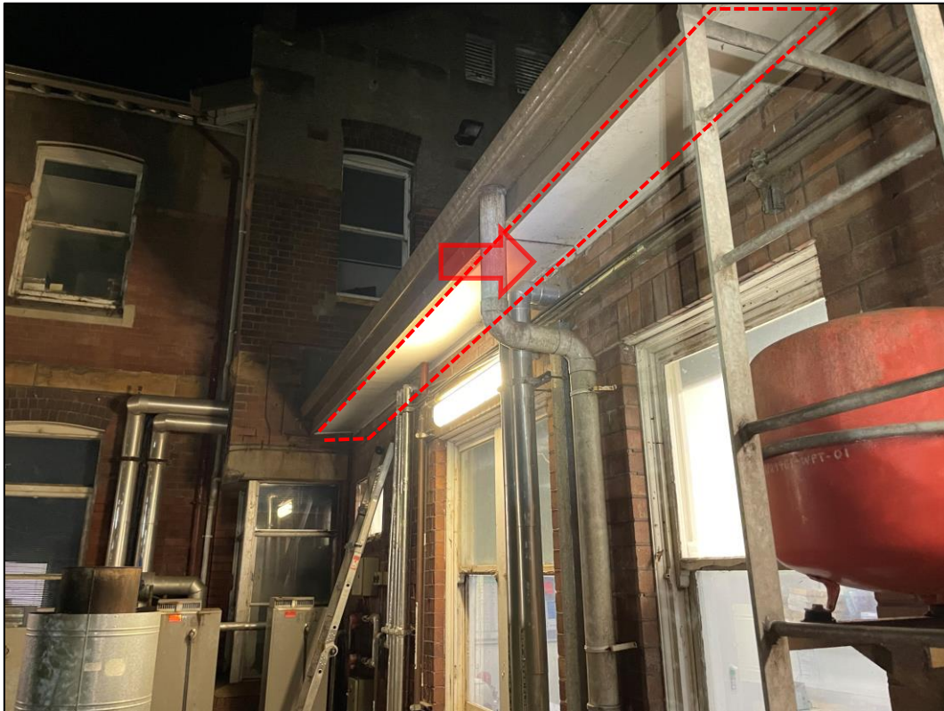
Photograph 5 Asbestos fibre cement eaves identified on the exterior of the building. Location of sample 'B94-LG-EAVES-A02'.
