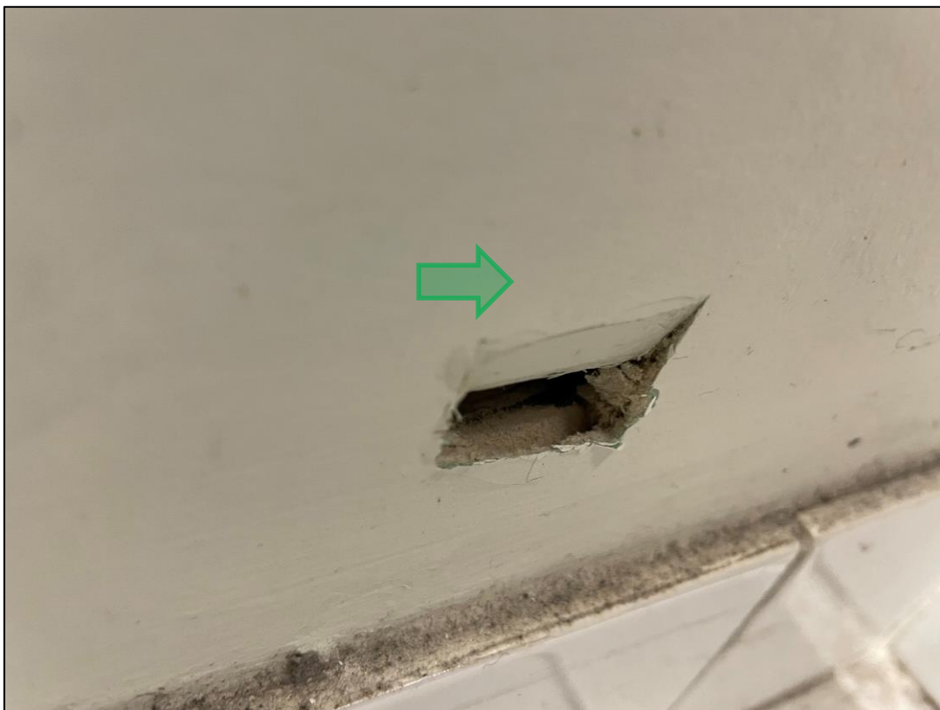
Photograph 4 Non-asbestos fibre cement observed within the bathrooms. Location of sample 'B94-LG_BATH-A01'.
