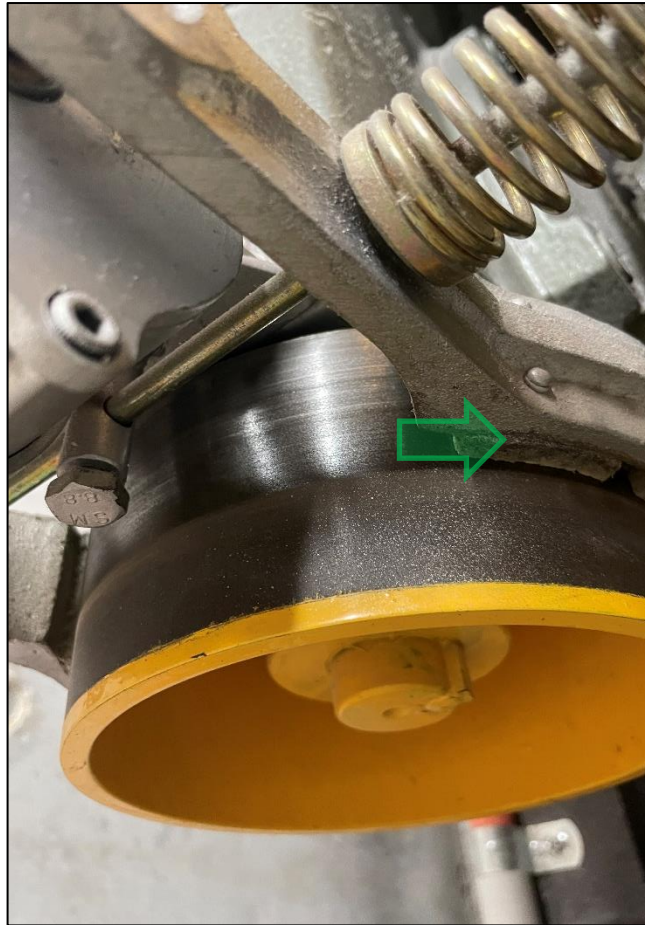
Photograph 5 Example of brake pad identified in lift motor room 9. Location of sample 'B75-L4-PLANT-LMR-BRAKE-ASB05' No asbestos detected.
