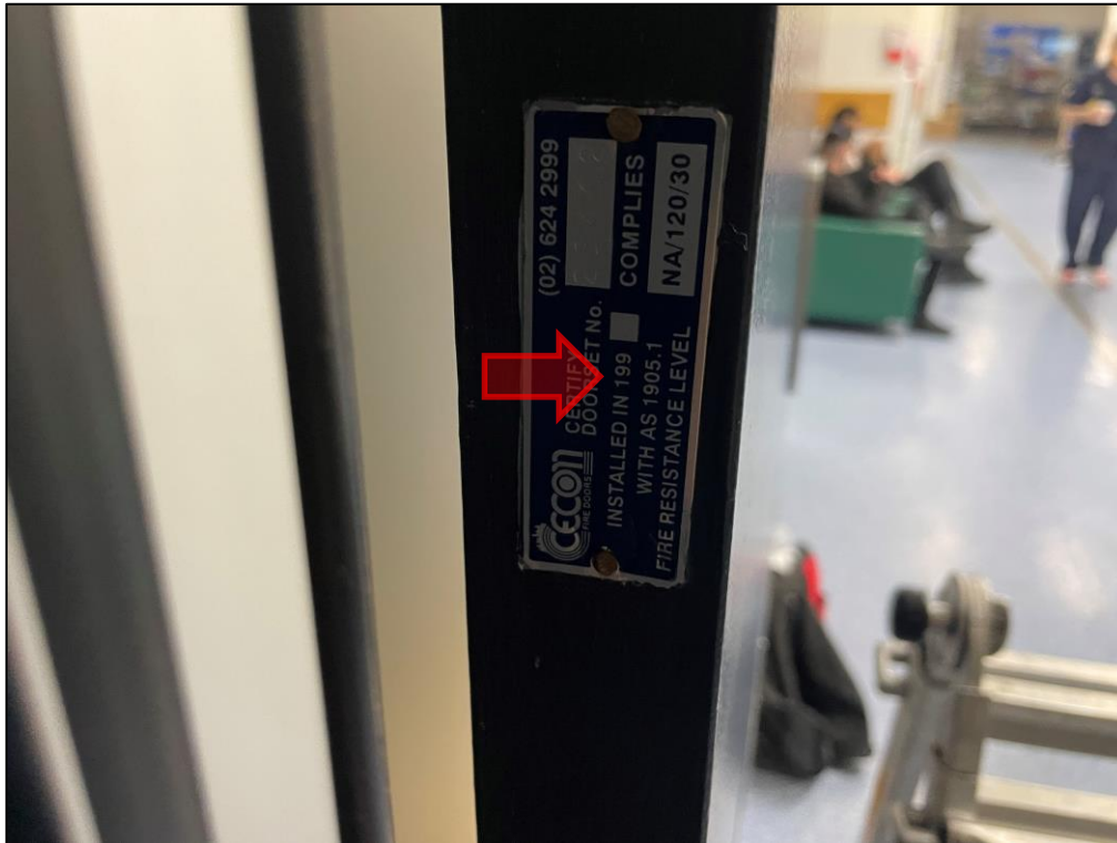
Photograph 15 Example of fire door compliance plate observed on level 4. Year of manufacture 199? indicates that there may be asbestos within the door.
