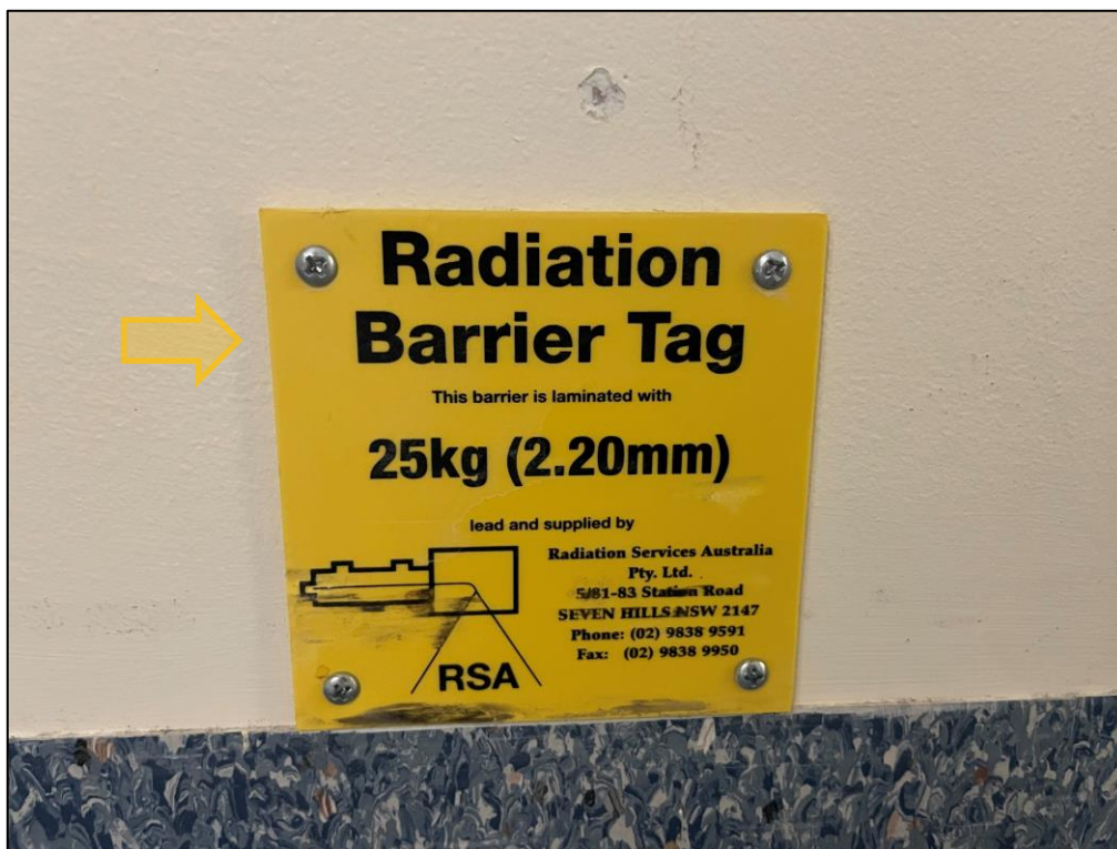
Photograph 12 Example of tag applied to walls / doors / windows with lead lining.
