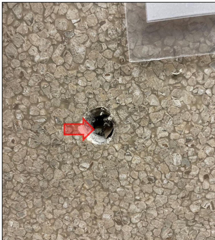
Photograph 2 Close up photograph of utility room floor lining where asbestos fibre cement was identified.
