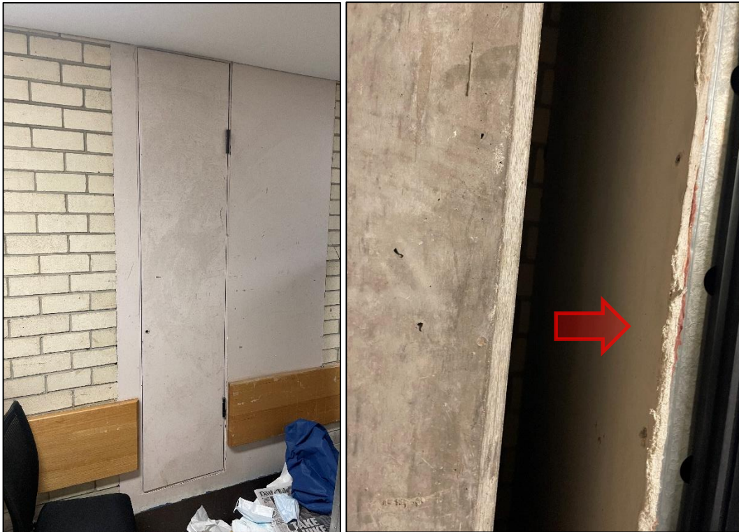
Photograph 3 Services cupboard located on various levels (left), containing internal asbestos fibre cement wall lining (right). Location of sample 'B89-23-HALL-CUPBOARD-ASB01'. Asbestos detected.
