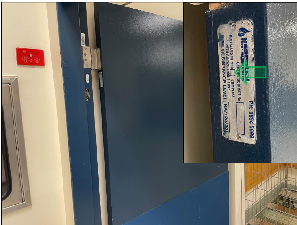
Photograph 16 Example of fire door located on level 3 with black 'PADDE' compliance plate on door frame, but with new door with 2000 + compliance plate. Not suspected of containing asbestos.
