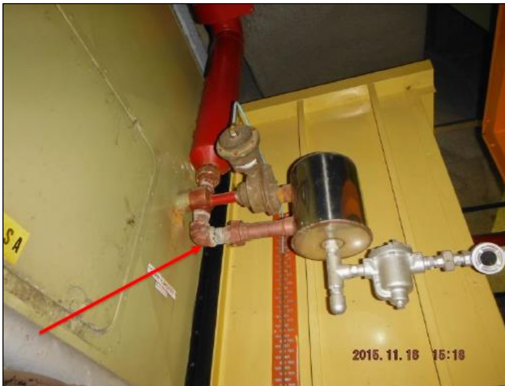
Photograph 10 Example of red asbestos gasket identified in old pipework. Photograph courtesy of Environmental Monitoring Services 'Building 75 – E Block, RPA Hospital, Camperdown NSW' Asbestos Register. Asbestos detected during sampling.
