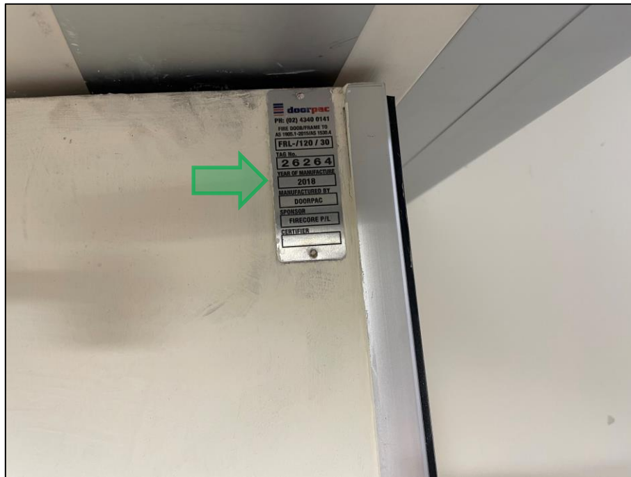
Photograph 13 Example of fire door compliance plate observed on level 6. Year of manufacture 2018 indicates that there is no asbestos within the door.
