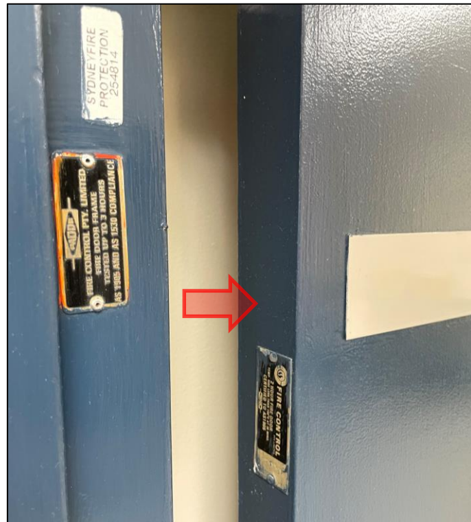
Photograph 17 Example of fire door located on level 3 with black 'PADDE' compliance plate on both door and door frame. Presumed to contain asbestos.
