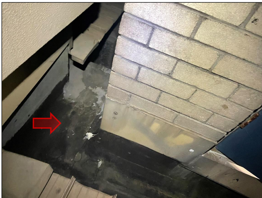
Photograph 8 Example of asbestos bituminous membrane identified on the roof of building 75 and 89. Location of sample 'B89-L12-ROOF-MASTIC-ASB04'. Asbestos detected.
