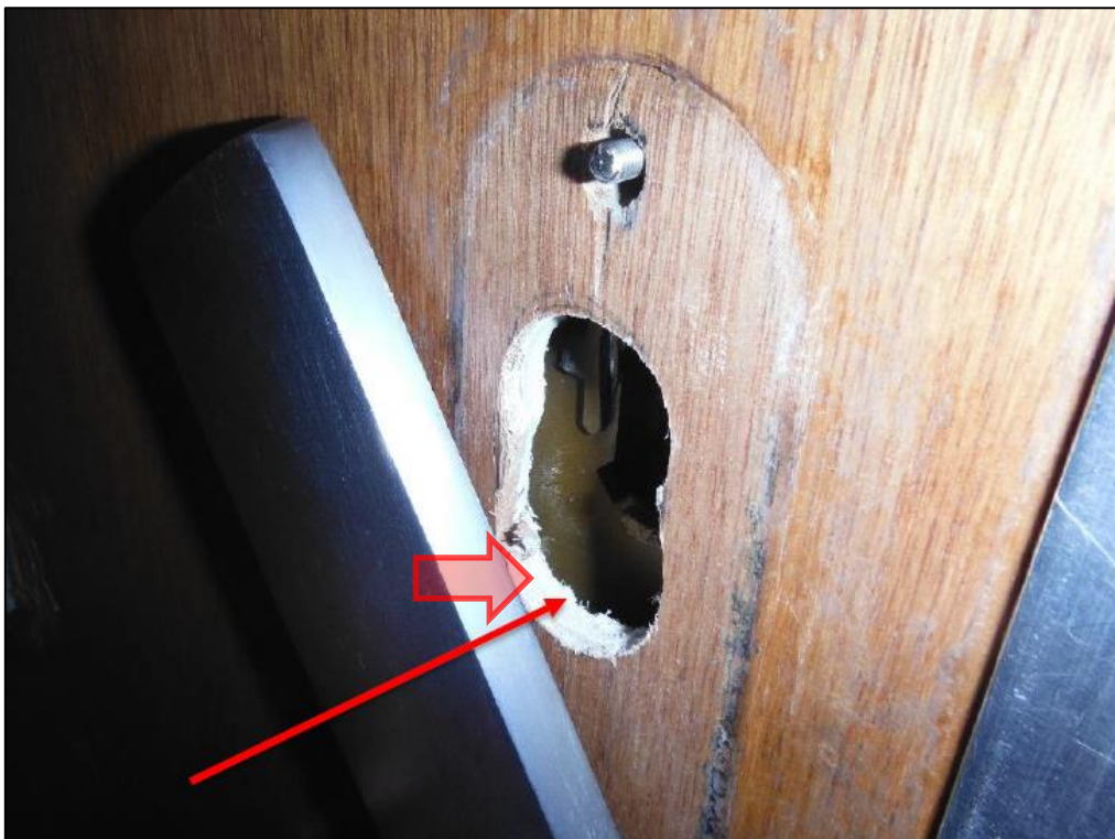
Photograph 6 Example of timber veneered door with internal asbestos insulation. Photograph courtesy of Environmental Monitoring Services 'Building 75 – E Block, RPA Hospital, Camperdown NSW' Asbestos Register. Asbestos detected during sampling.
