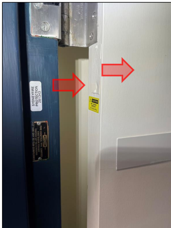
Photograph 11 Compliance plate without date (note black 'PADDE Fire Control Pty Ltd' compliance plates are taken to be indicative of asbestos containing fire doors). Additionally, a "presumed to contain" asbestos sticker had been previously applied to the door to indicate that it may contain asbestos.
