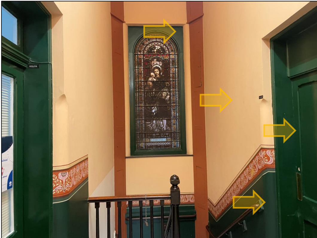
Photograph 3 Example of green and cream lead paint systems identified on the L5 entrance hallway walls.
