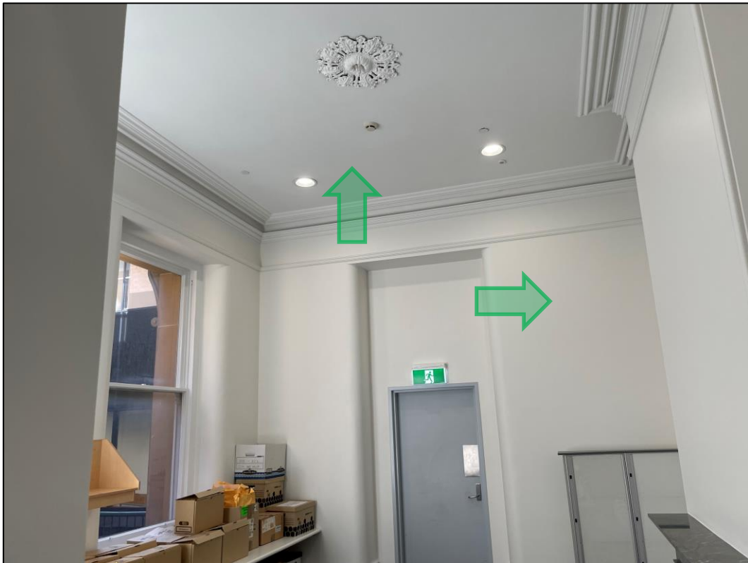
Photograph 6 Example of most rooms encountered throughout L6 and L7 of B64. Rendered brick wall, non-lead containing paint, and plasterboard ceiling lining.
