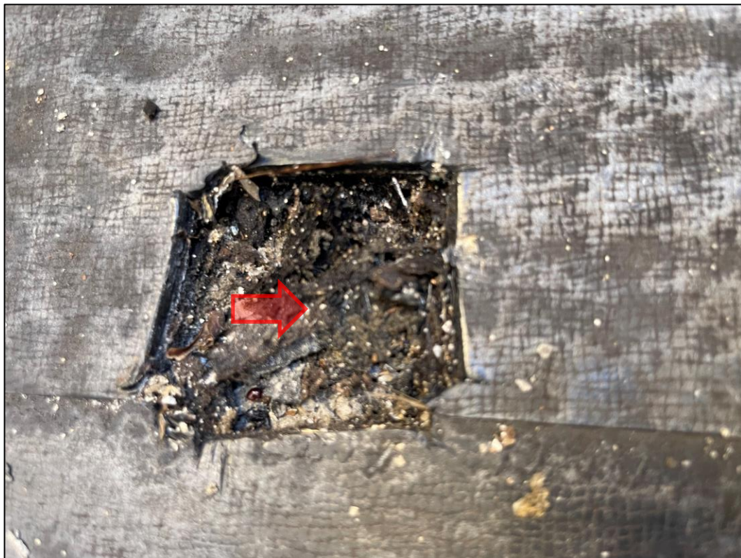
Photograph 2 Example of asbestos containing bituminous layer, underlying black vinyl covering on the L6 flat roof. Location of sample 'B64-L6-ROOF-ASB01'. Chrysotile asbestos detected.
