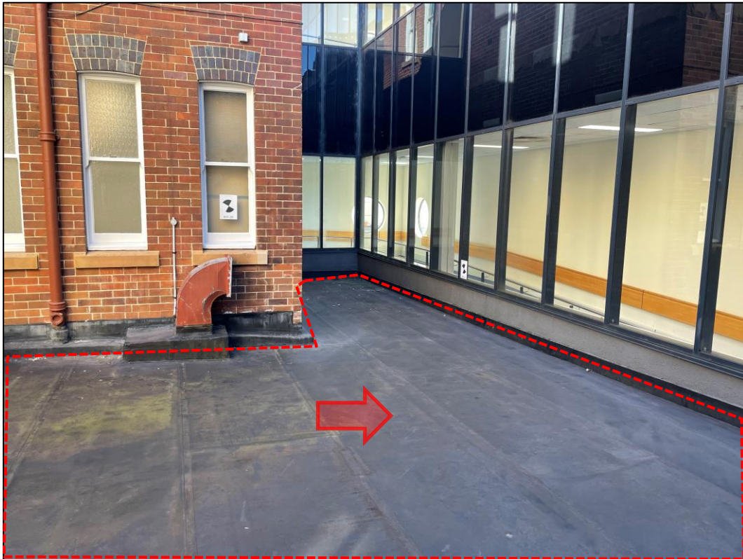
Photograph 1 Asbestos bituminous layer (underlying observable black vinyl covering), observed on L6 flat roof. Chrysotile Asbestos detected.
