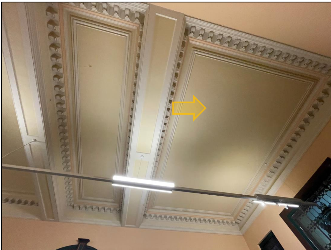
Photograph 4 Example of cream presumed lead paint systems identified on the L5 entrance hallway ceiling.
