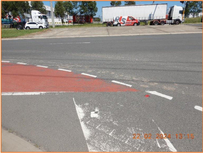
Figure 426: Reasonable - General condition of flexible pavement.
