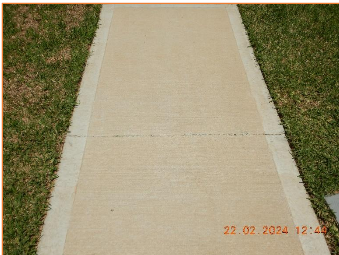
Figure 92: Reasonable - General condition of footpath. Minor hairline cracking observed.
