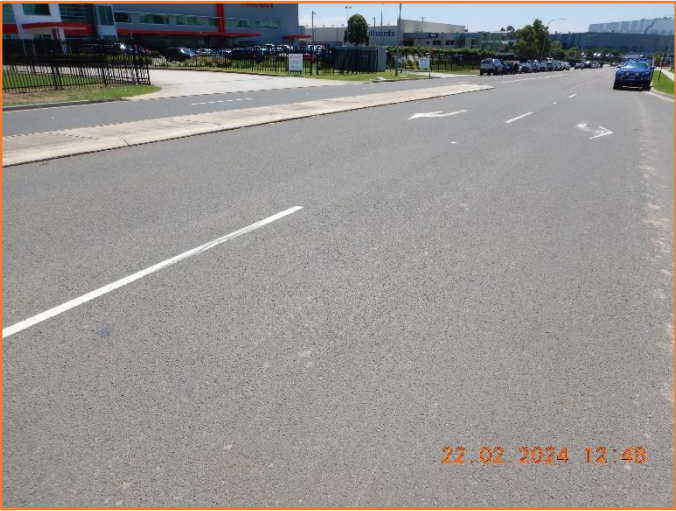
Figure 143: Reasonable - General condition of flexible pavement.
