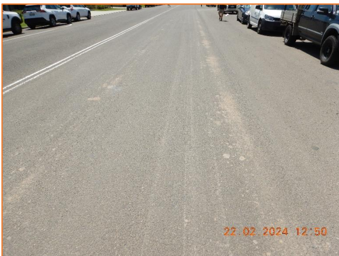
Figure 167: Reasonable - General condition of flexible pavement.
