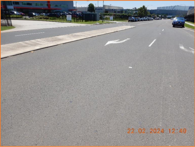
Figure 145: Reasonable - General condition of flexible pavement.
