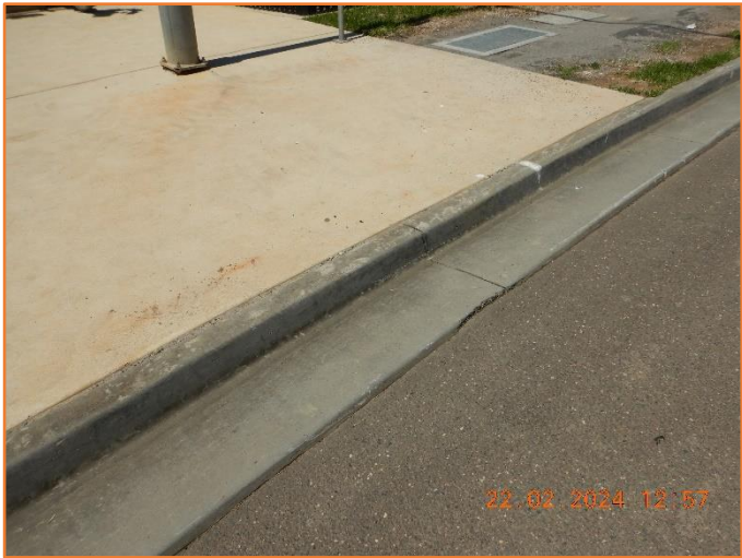
Figure 233: Reasonable - General condition of kerb and gutter.
