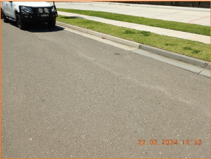
Figure 195: Reasonable - General condition of flexible pavement.
