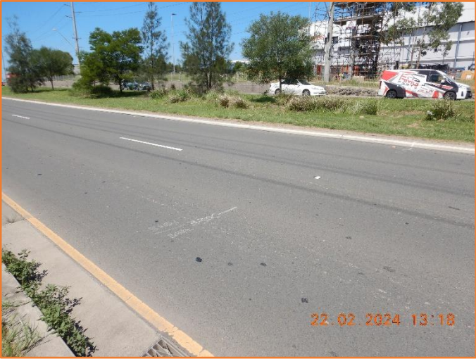
Figure 446: Reasonable - General condition of flexible pavement.
