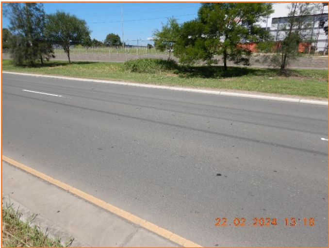
Figure 450: Reasonable - General condition of flexible pavement.
