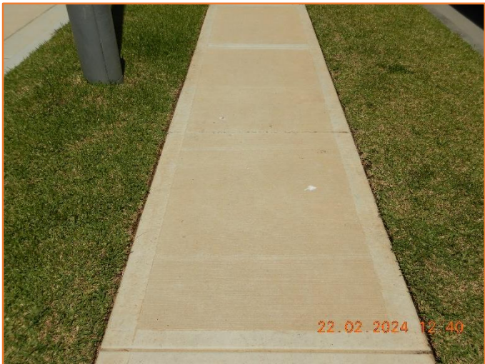
Figure 42: Good - General condition of footpath.
