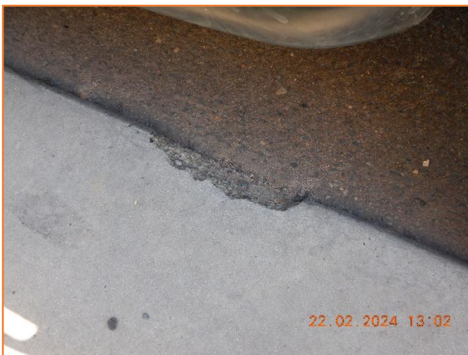
Figure 290: Reasonable - General condition of kerb and gutter. Minor spalling observed.
