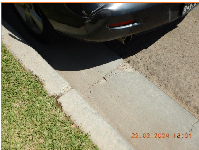
Figure 284: Reasonable - General condition of kerb and gutter. Minor spalling observed.
