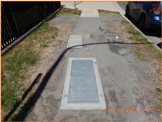
Figure 23: Reasonable - General condition of service pits.
