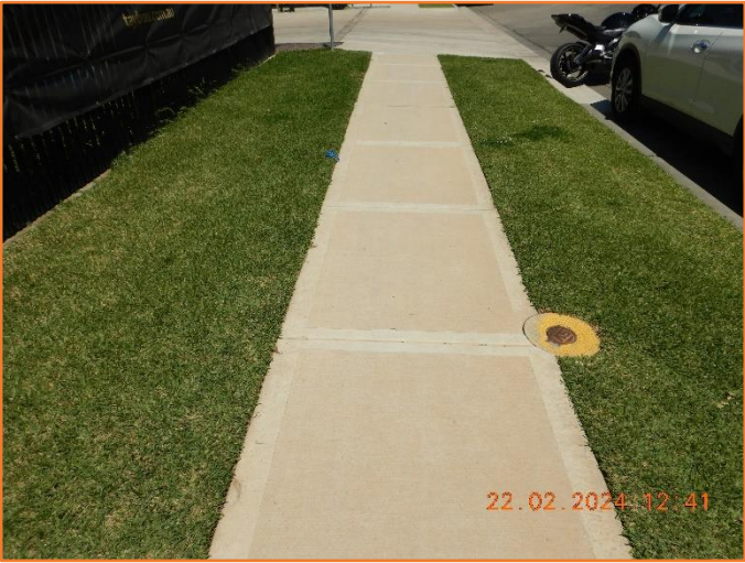
Figure 56: Good - General condition of footpath.
