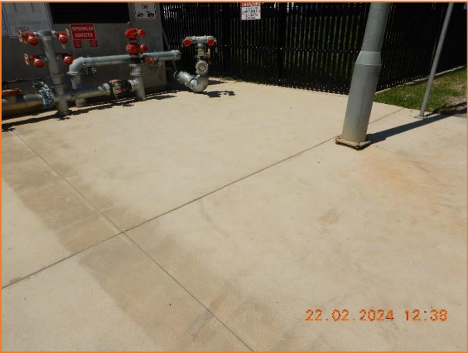
Figure 20: Reasonable - General condition of footpath.
