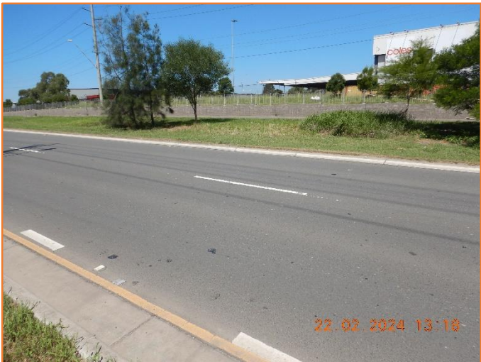
Figure 451: Reasonable - General condition of flexible pavement.
