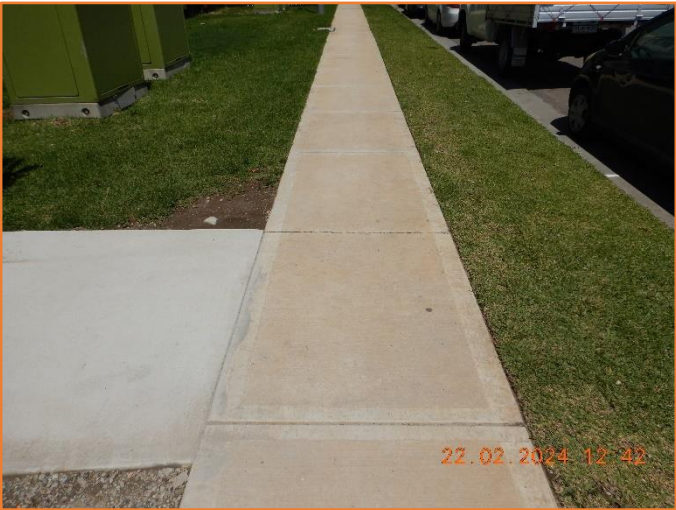
Figure 69: Good - General condition of footpath.
