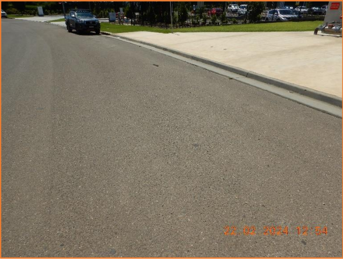
Figure 205: Reasonable - General condition of flexible pavement.
