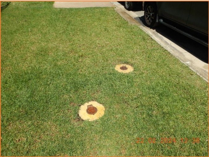
Figure 9: Reasonable - General condition of service pits.
