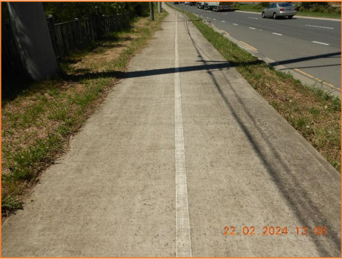
Figure 342: Reasonable - General condition of footpath.
