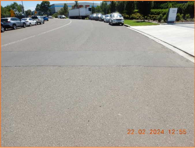
Figure 215: Reasonable - General condition of flexible pavement.
