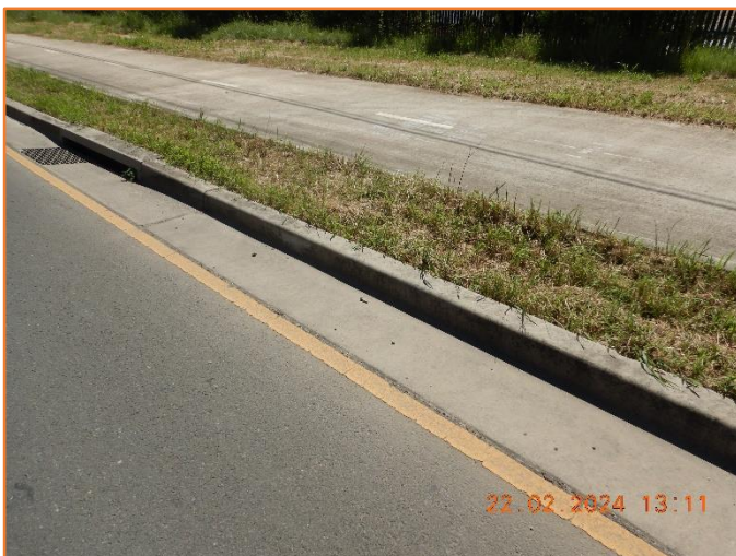
Figure 385: Reasonable - General condition of kerb and gutter.
