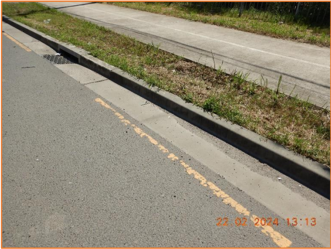
Figure 406: Reasonable - General condition of kerb and gutter.
