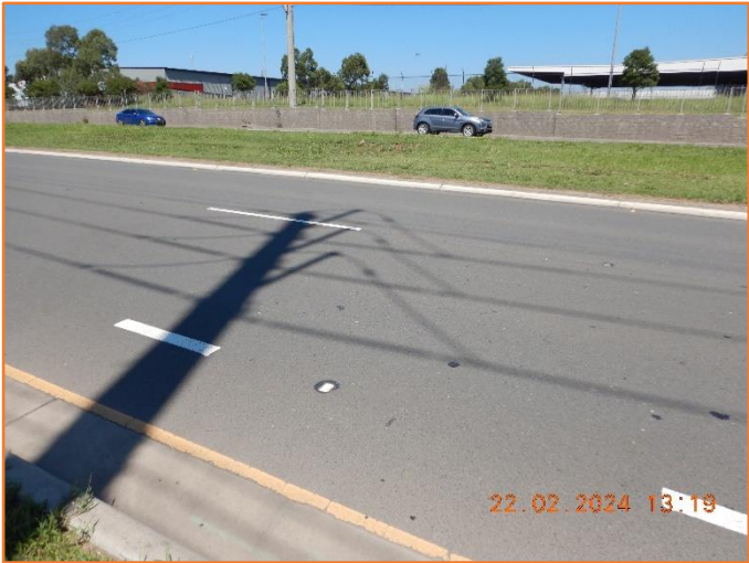
Figure 457: Reasonable - General condition of flexible pavement.
