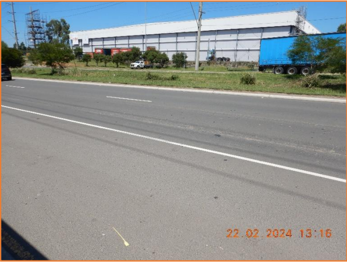
Figure 432: Reasonable - General condition of flexible pavement.
