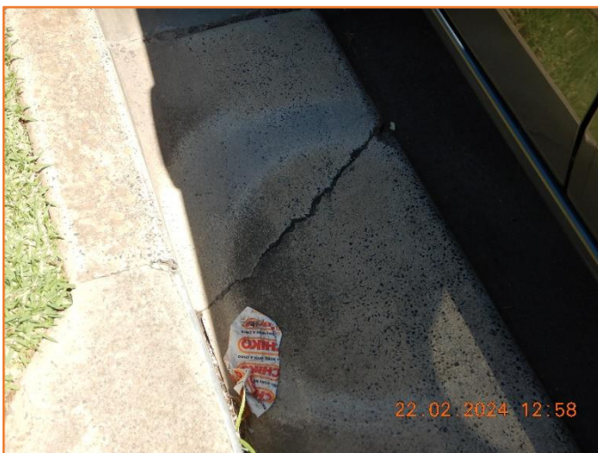
Figure 257: Reasonable - General condition of kerb inlet pit. Moderate cracking observed.
