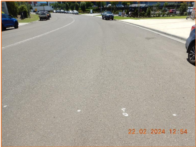
Figure 202: Reasonable - General condition of flexible pavement.
