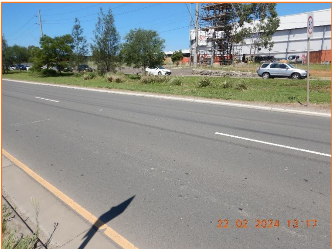
Figure 445: Reasonable - General condition of flexible pavement.
