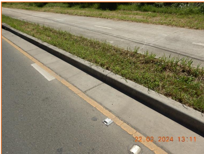
Figure 384: Reasonable - General condition of kerb and gutter.
