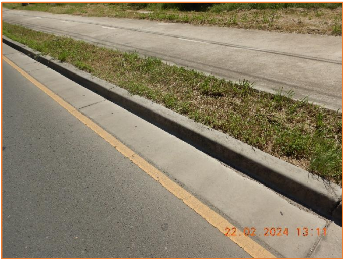
Figure 387: Reasonable - General condition of kerb and gutter.
