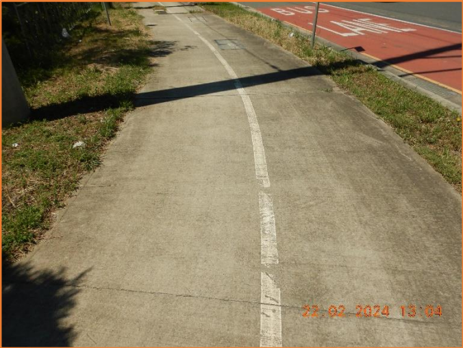
Figure 323: Reasonable - General condition of footpath.
