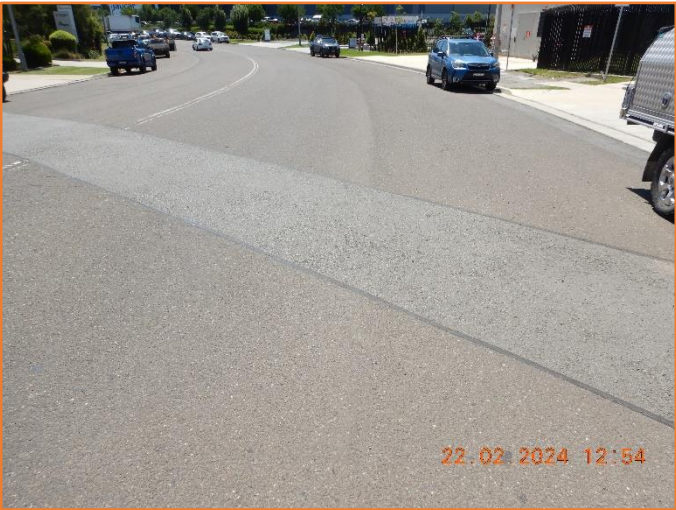
Figure 198: Reasonable - General condition of flexible pavement.
