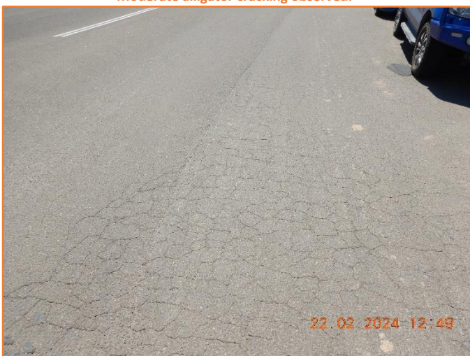
Figure 153: Reasonable - General condition of flexible pavement. Moderate alligator cracking observed.
