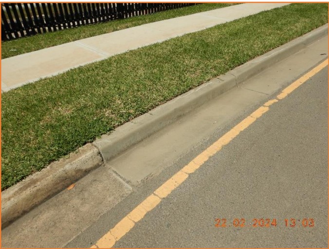
Figure 309: Reasonable - General condition of kerb and gutter.
