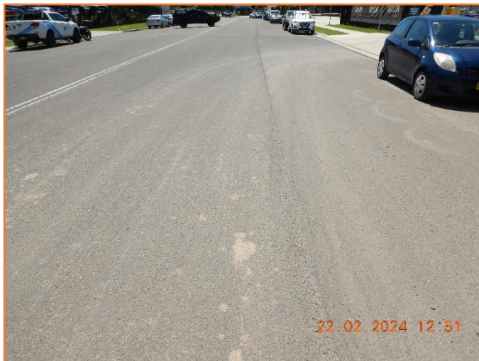
Figure 173: Reasonable - General condition of flexible pavement.
