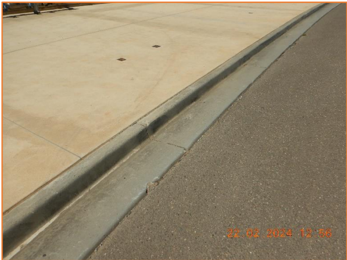
Figure 228: Reasonable - General condition of kerb and gutter.
