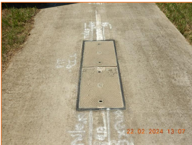
Figure 364: Reasonable - General condition of service pit.
