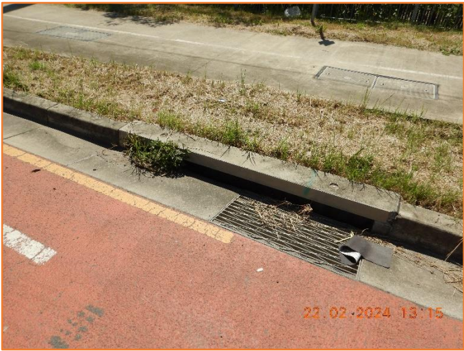
Figure 420: Reasonable - General condition of kerb inlet pit.
