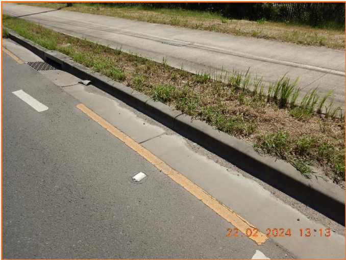
Figure 395: Reasonable - General condition of kerb and gutter.
