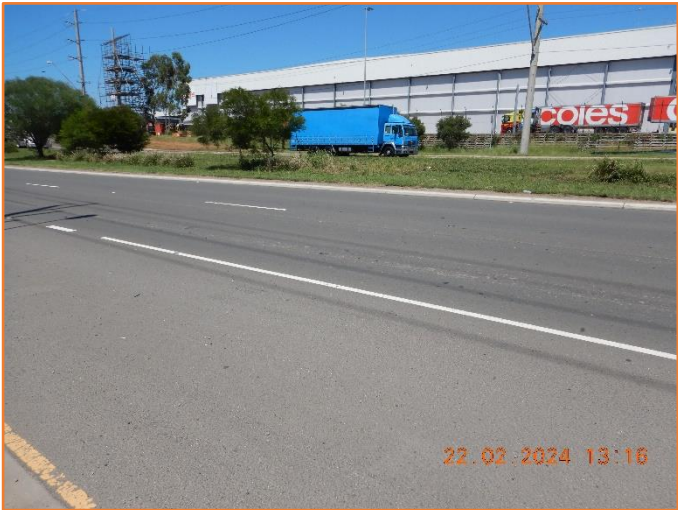
Figure 434: Reasonable - General condition of flexible pavement.
