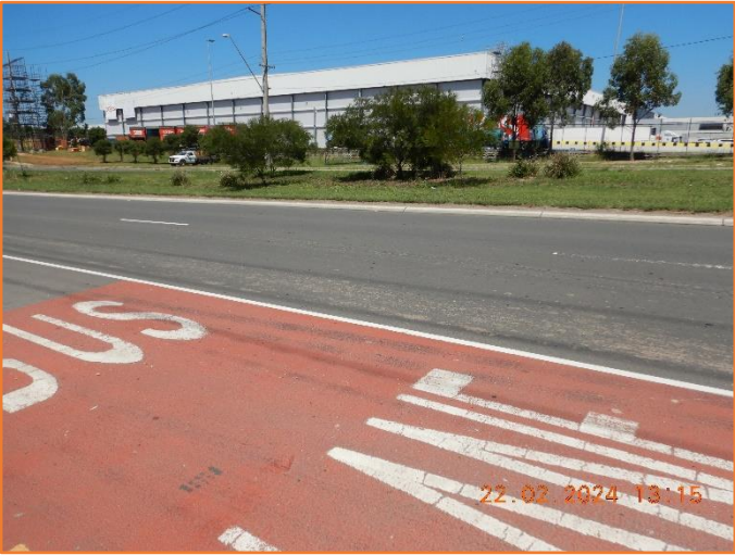
Figure 429: Reasonable - General condition of flexible pavement.
