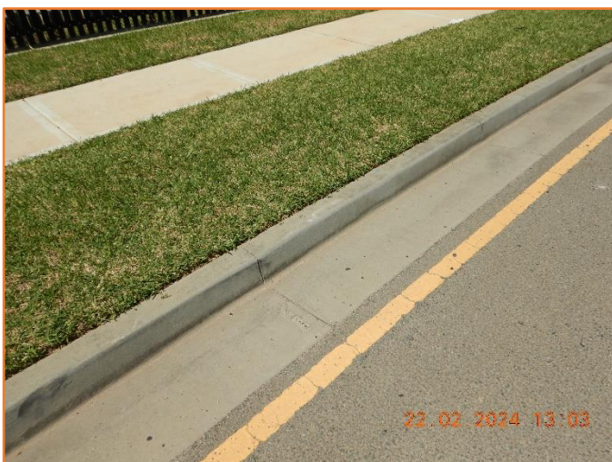
Figure 306: Reasonable - General condition of kerb and gutter.
