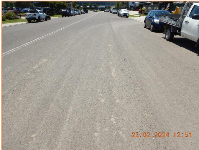
Figure 172: Reasonable - General condition of flexible pavement.
