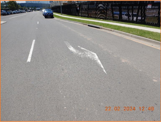
Figure 146: Reasonable - General condition of flexible pavement.
