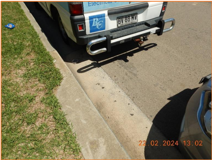
Figure 293: Reasonable - General condition of kerb inlet pit.
