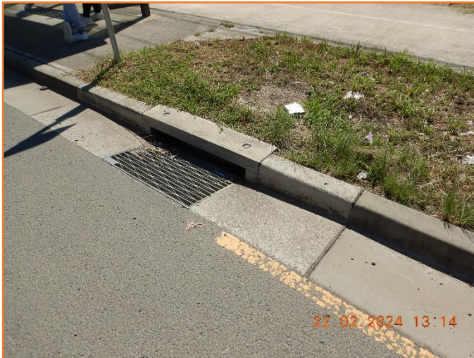
Figure 410: Reasonable - General condition of kerb inlet pit.
