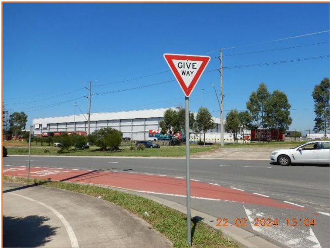
Figure 321: Good - General condition of traffic signage.
