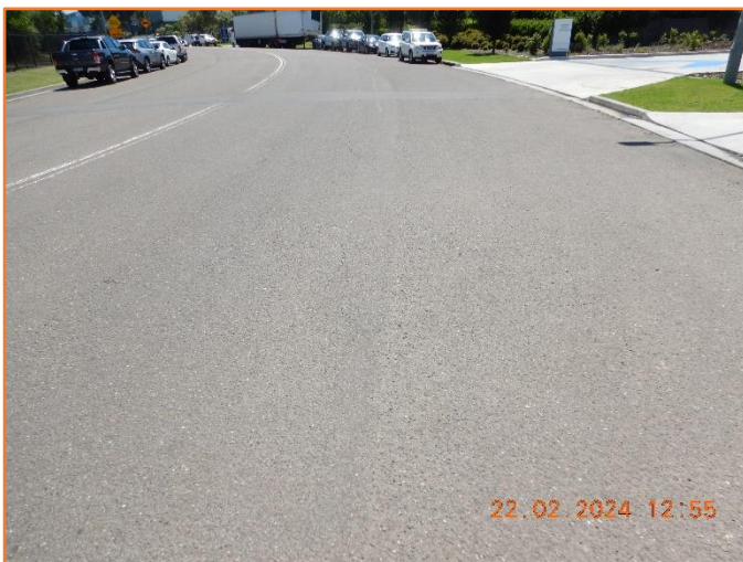
Figure 213: Reasonable - General condition of flexible pavement.
