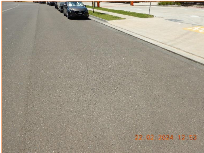
Figure 187: Reasonable - General condition of flexible pavement.
