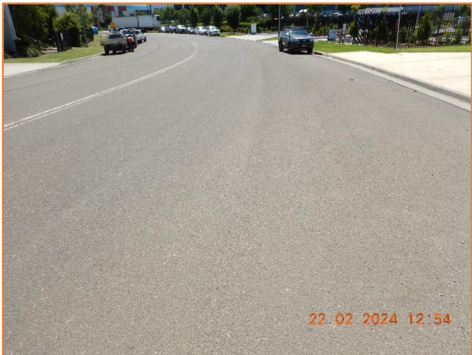
Figure 204: Reasonable - General condition of flexible pavement.
