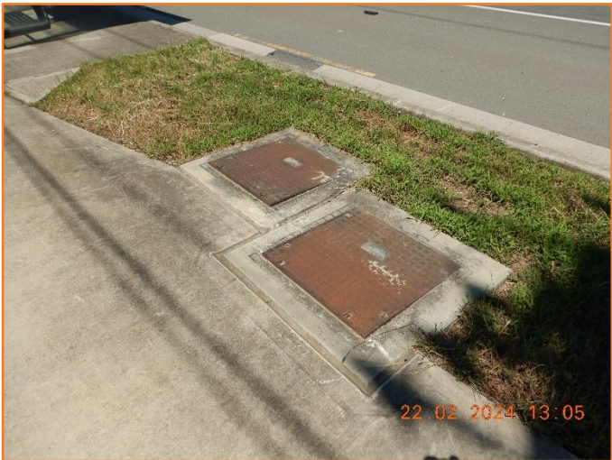
Figure 334: Reasonable - General condition of service pit.
