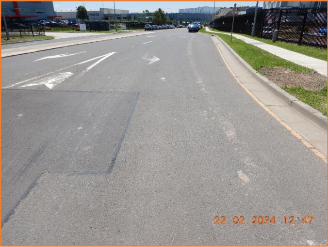
Figure 139: Reasonable - General condition of flexible pavement.
