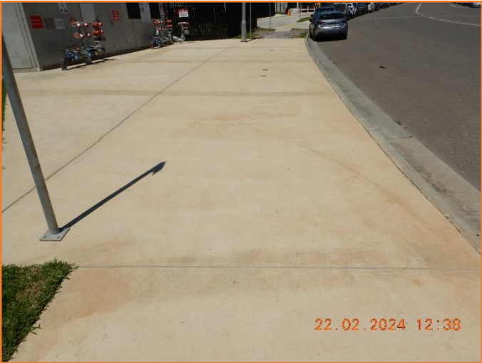
Figure 11: Reasonable - General condition of footpath.
