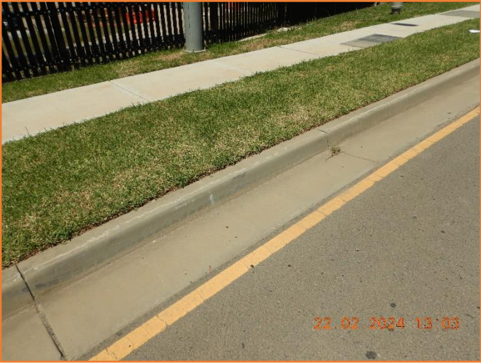
Figure 310: Reasonable - General condition of kerb and gutter.
