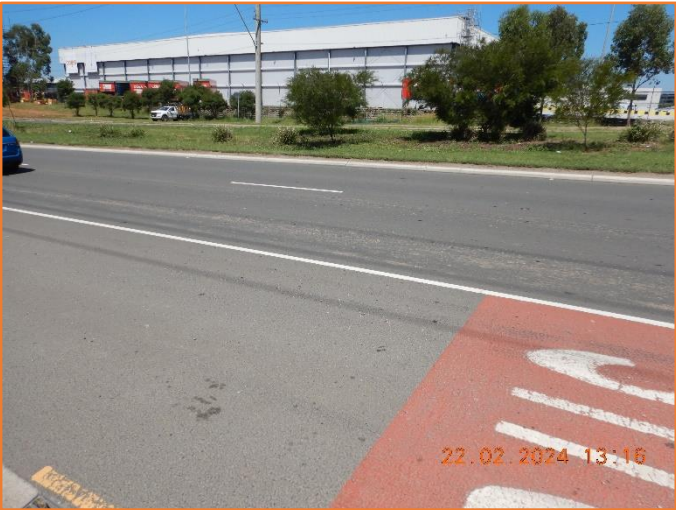
Figure 430: Reasonable - General condition of flexible pavement.
