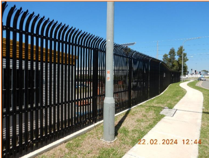
Figure 103: Good - General condition of monopole assembly.
