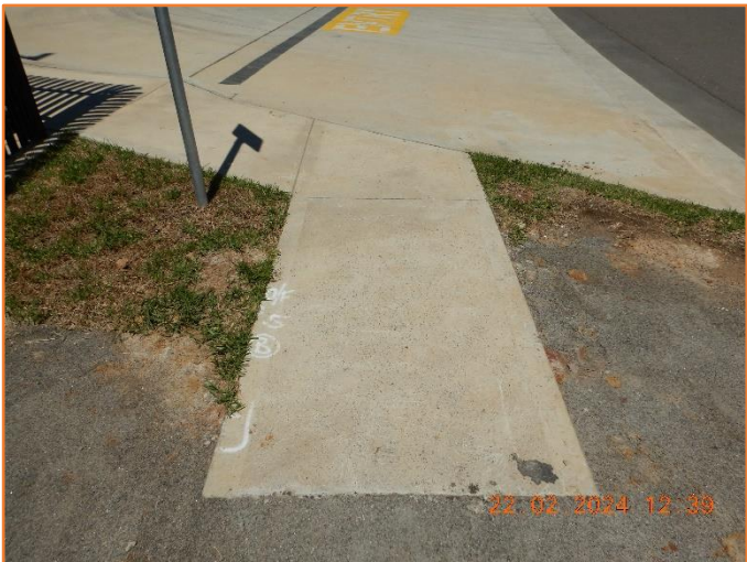
Figure 24: Reasonable - General condition of footpath.
