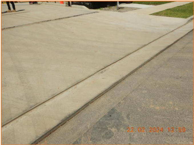
Figure 262: Reasonable - General condition of driveway layback.
