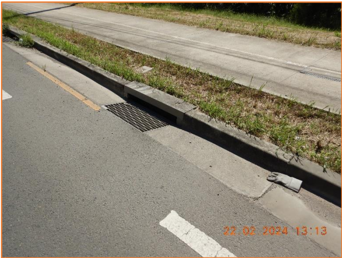
Figure 396: Reasonable - General condition of kerb inlet pit.
