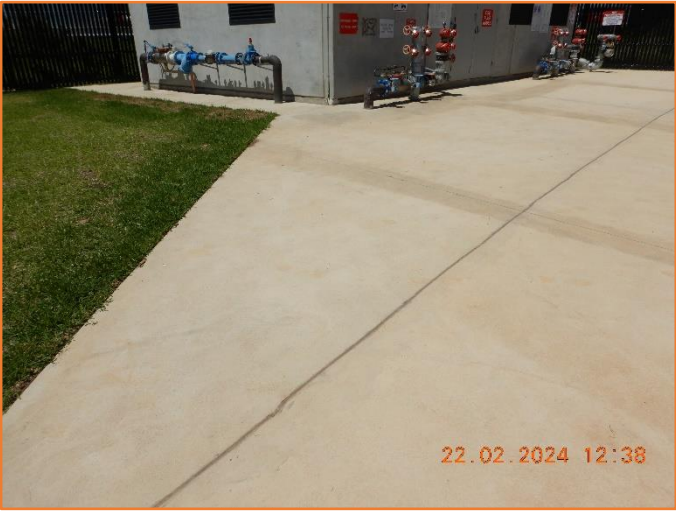
Figure 14: Reasonable - General condition of footpath.
