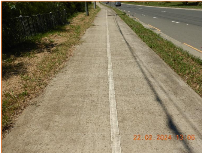
Figure 344: Reasonable - General condition of footpath.
