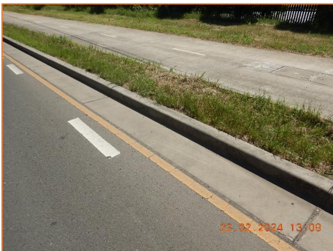
Figure 382: Reasonable - General condition of kerb and gutter.
