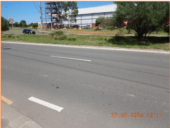
Figure 442: Reasonable - General condition of flexible pavement.
