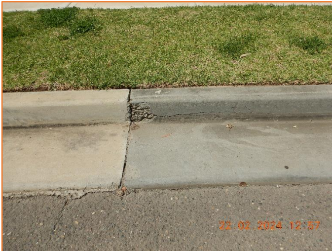
Figure 244: Poor - General condition of kerb and gutter. Moderate cracking and loss of material observed.
