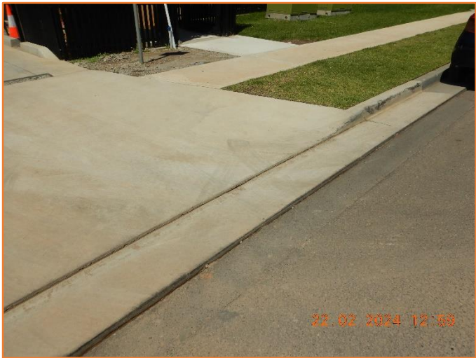
Figure 263: Reasonable - General condition of driveway layback.
