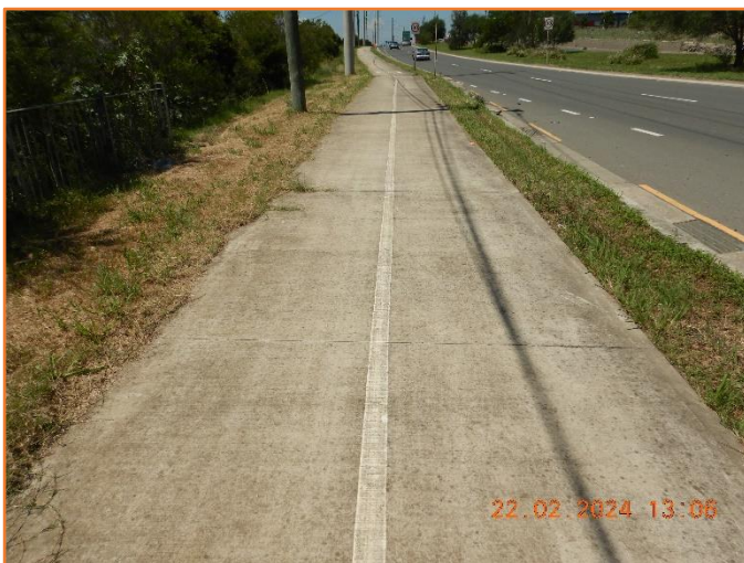
Figure 345: Reasonable - General condition of footpath.
