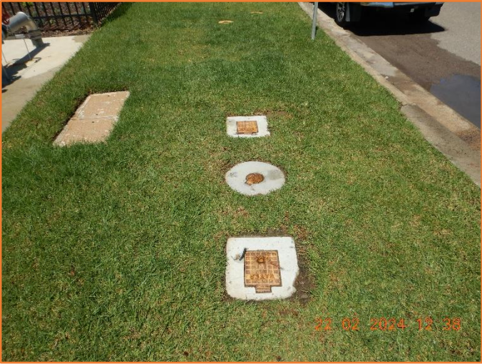
Figure 7: Reasonable - General condition of service pits.
