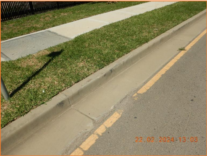
Figure 312: Reasonable - General condition of kerb and gutter.
