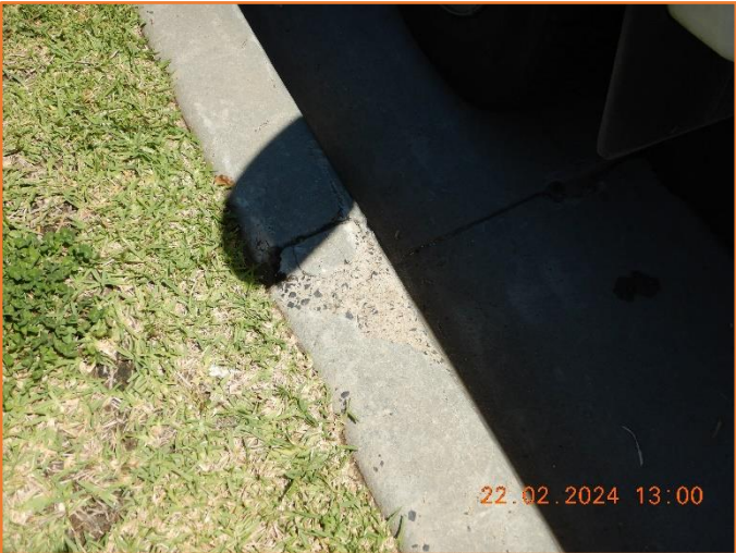
Figure 270: Reasonable - General condition of kerb and gutter. Moderate spalling observed.
