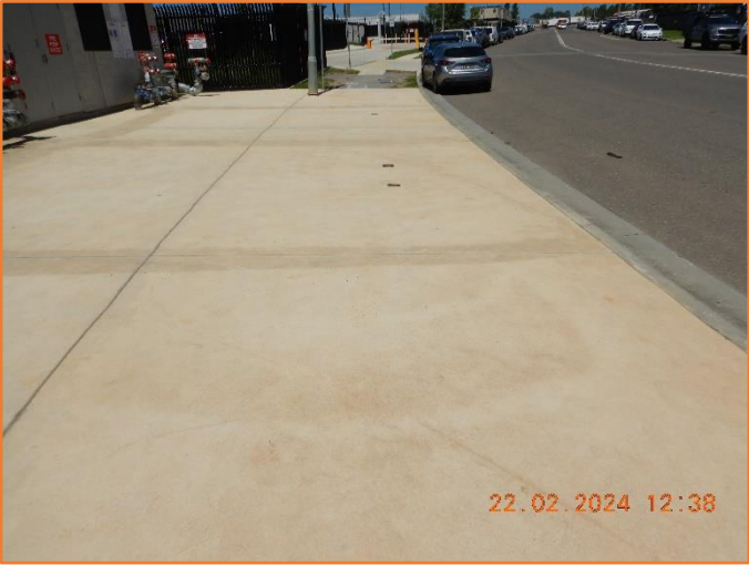
Figure 13: Reasonable - General condition of footpath.
