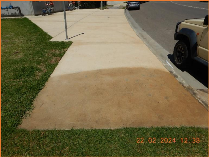
Figure 10: Reasonable - General condition of footpath.
