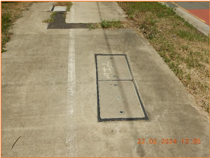
Figure 330: Reasonable - General condition of footpath and service pit.
