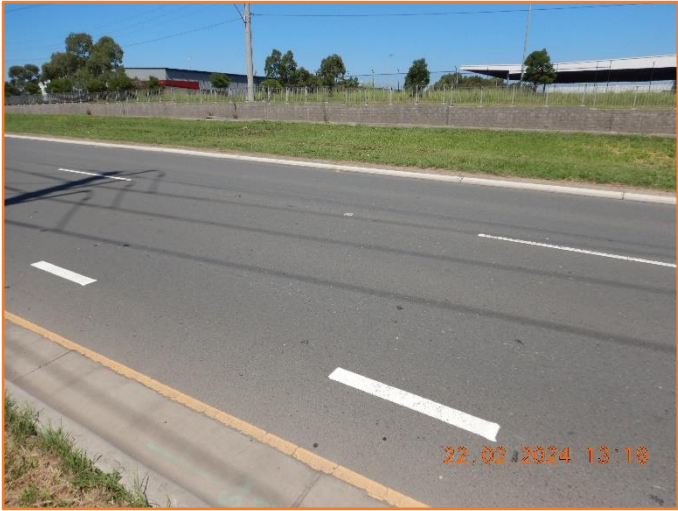
Figure 456: Reasonable - General condition of flexible pavement.
