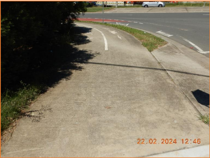
Figure 132: Reasonable - General condition of footpath.
