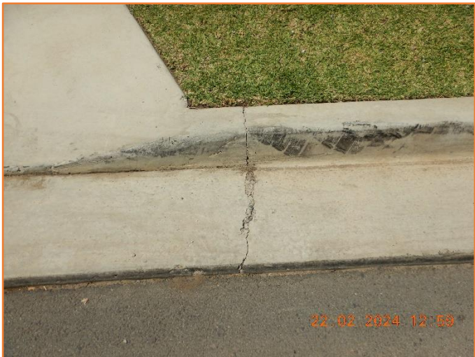
Figure 264: Reasonable - General condition of driveway splay. Moderate hairline cracking observed.
