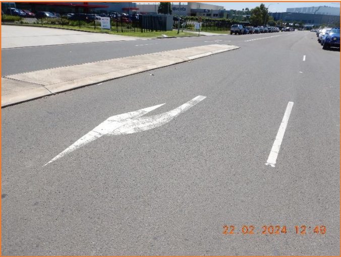
Figure 147: Reasonable - General condition of flexible pavement.
