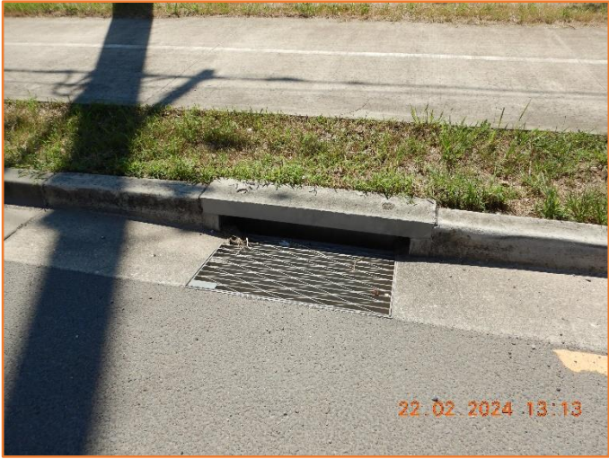
Figure 405: Reasonable - General condition of kerb inlet pit.
