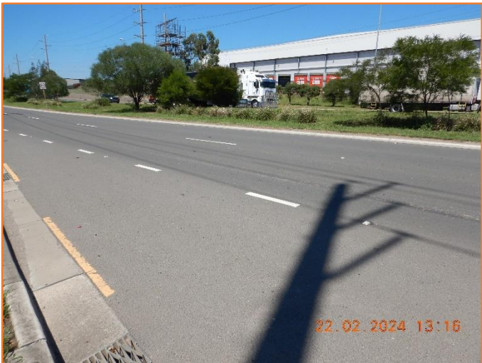
Figure 436: Reasonable - General condition of flexible pavement.
