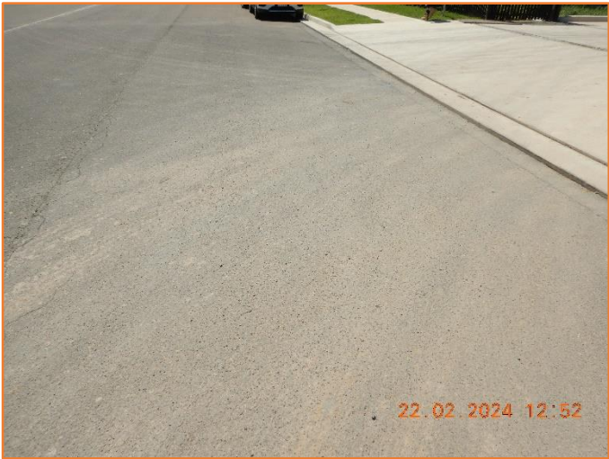
Figure 176: Reasonable - General condition of flexible pavement.
