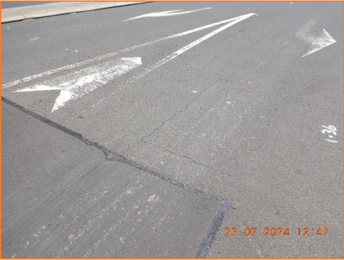
Figure 140: Reasonable - General condition of rigid pavement. Moderate cracking observed.
