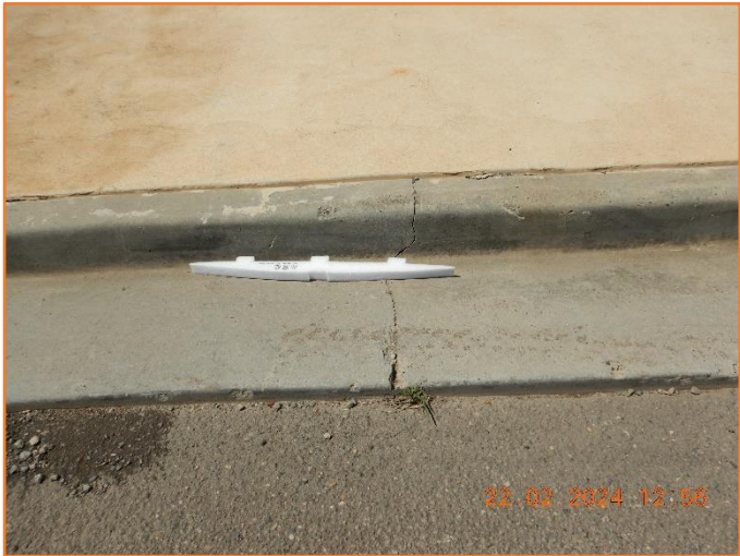
Figure 226: Reasonable - General condition of kerb and gutter. Moderate cracking observed.
