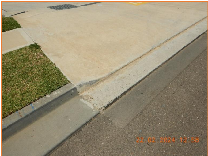
Figure 252: Reasonable - General condition of driveway splay.
