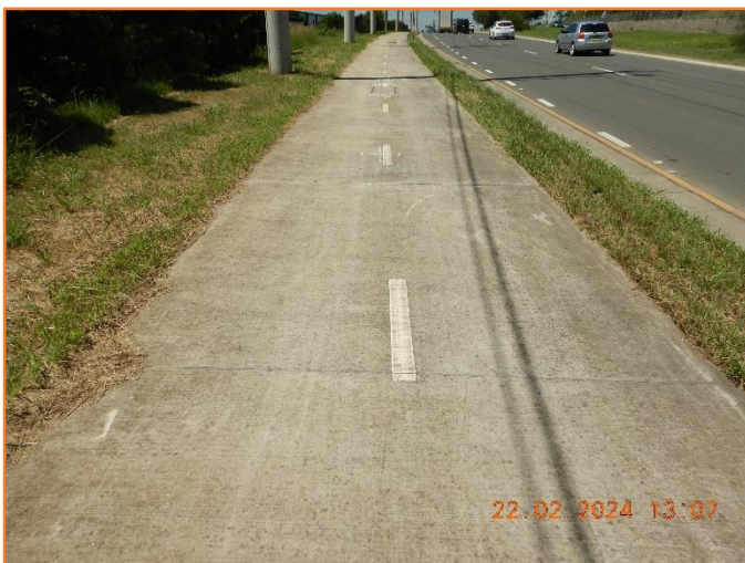
Figure 361: Reasonable - General condition of footpath.
