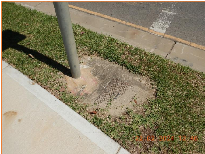
Figure 127: Reasonable - General condition of service pit.
