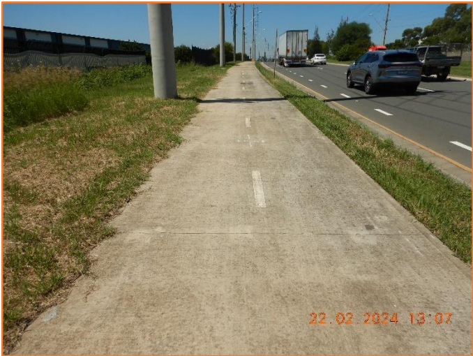
Figure 368: Reasonable - General condition of footpath.
