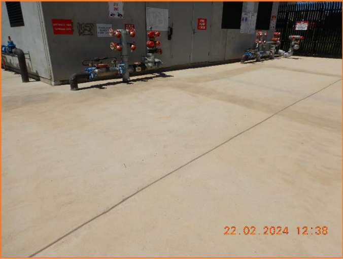
Figure 16: Reasonable - General condition of footpath.
