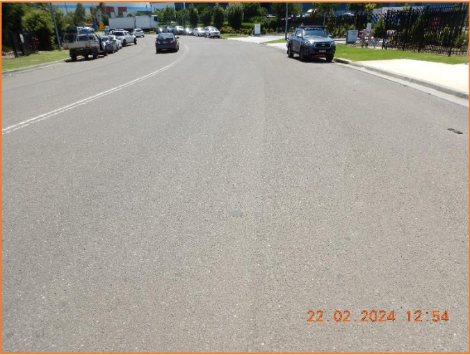
Figure 206: Reasonable - General condition of flexible pavement.
