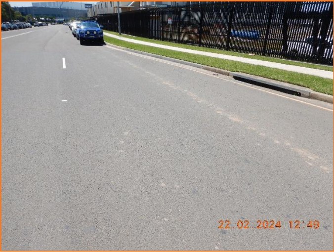
Figure 148: Reasonable - General condition of flexible pavement.
