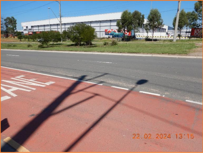
Figure 428: Reasonable - General condition of flexible pavement.
