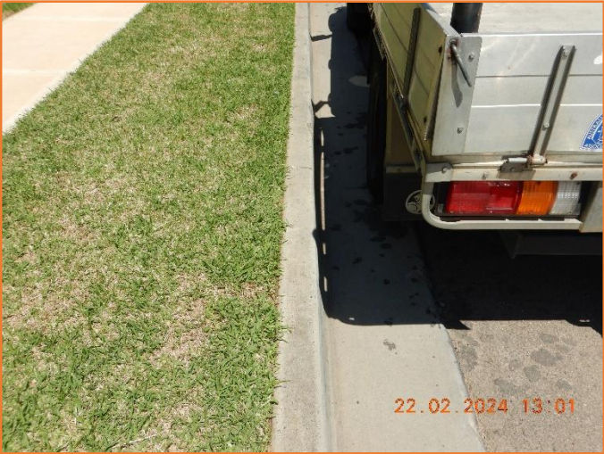
Figure 278: Reasonable - General condition of kerb and gutter.
