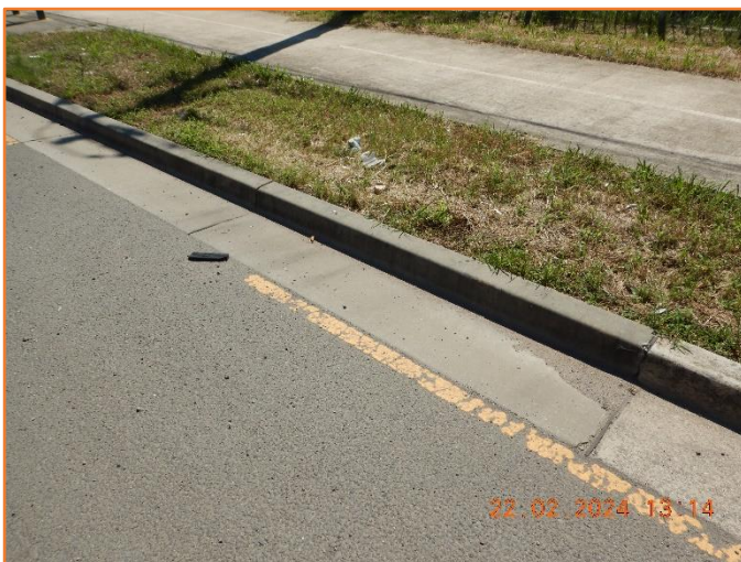
Figure 408: Reasonable - General condition of kerb and gutter.
