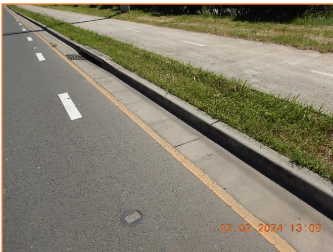
Figure 378: Reasonable - General condition of kerb and gutter.
