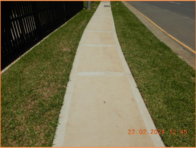
Figure 113: Good - General condition of footpath.
