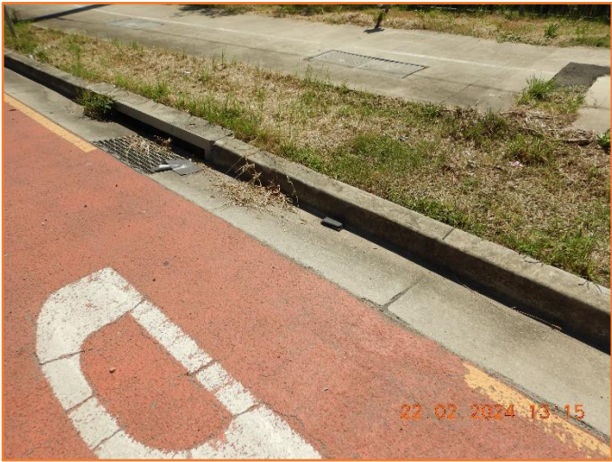
Figure 419: Reasonable - General condition of kerb and gutter.
