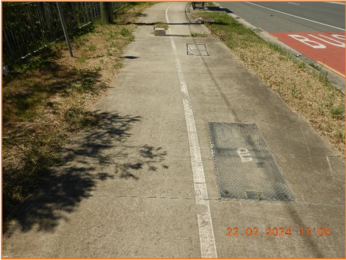
Figure 327: Reasonable - General condition of footpath and service pit.
