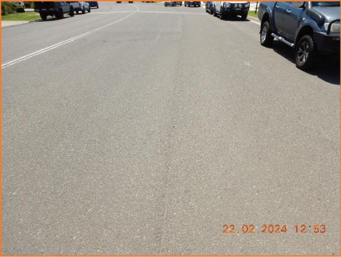
Figure 193: Reasonable - General condition of flexible pavement.
