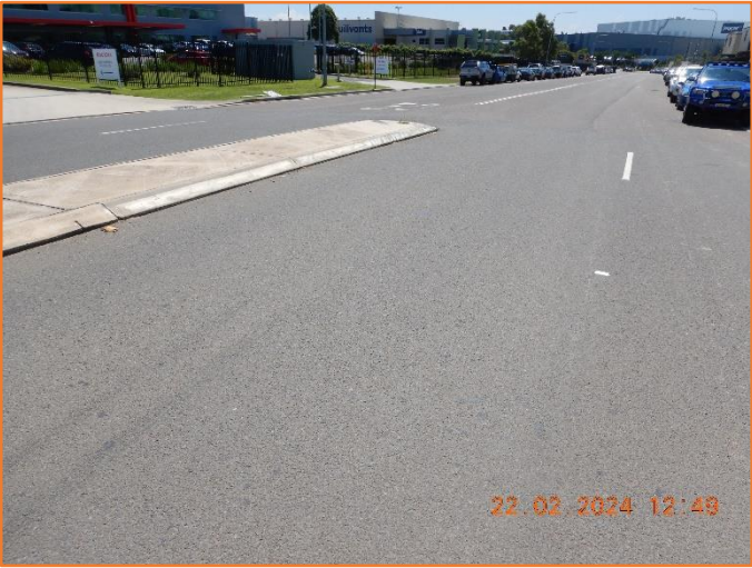
Figure 149: Reasonable - General condition of flexible pavement.
