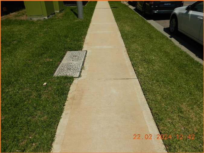
Figure 73: Good - General condition of footpath.
