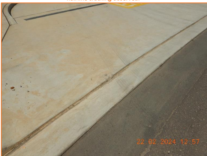
Figure 237: Reasonable - General condition of driveway layback. Minor spalling observed.
