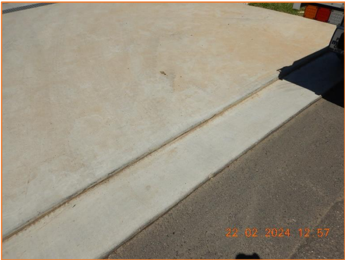
Figure 239: Reasonable - General condition of driveway layback.
