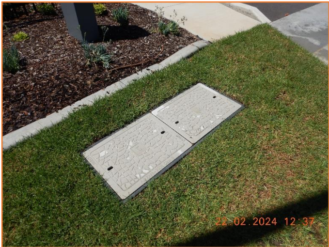
Figure 2: Good - General condition of service pit.
