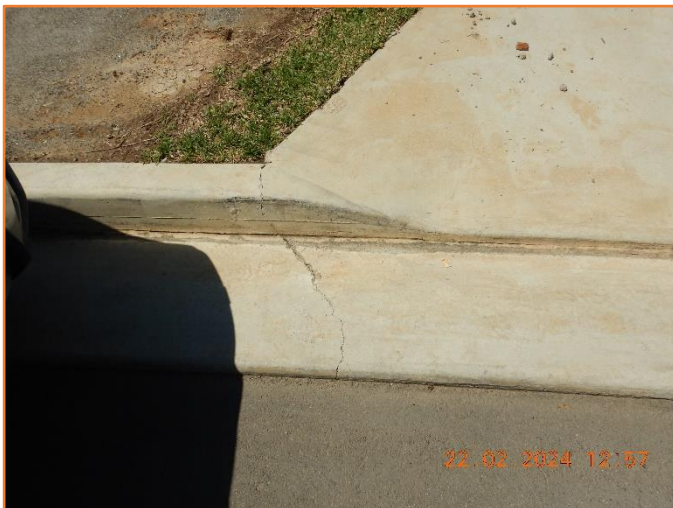
Figure 236: Reasonable - General condition of driveway splay. Moderate hairline cracking observed.
