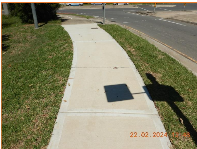
Figure 128: Good - General condition of footpath.
