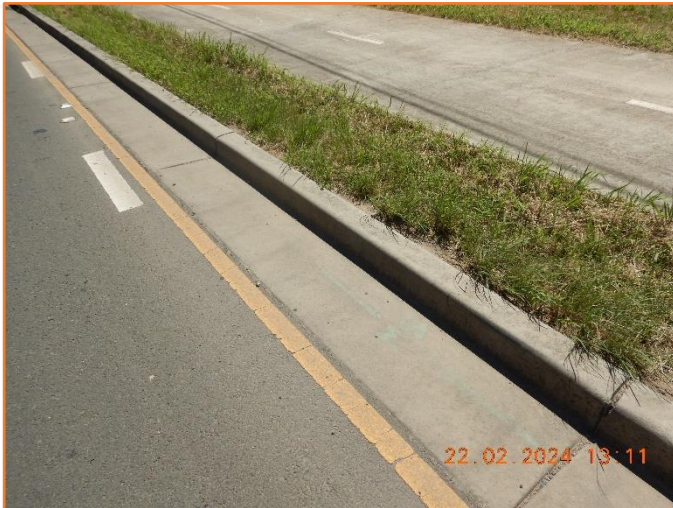
Figure 383: Reasonable - General condition of kerb and gutter.
