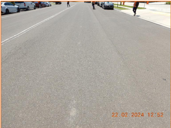
Figure 183: Reasonable - General condition of flexible pavement.
