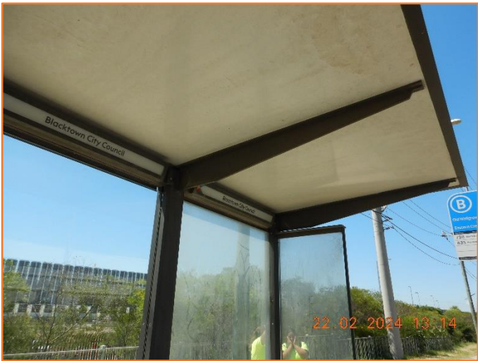
Figure 415: Reasonable - General condition of bus shelter.
