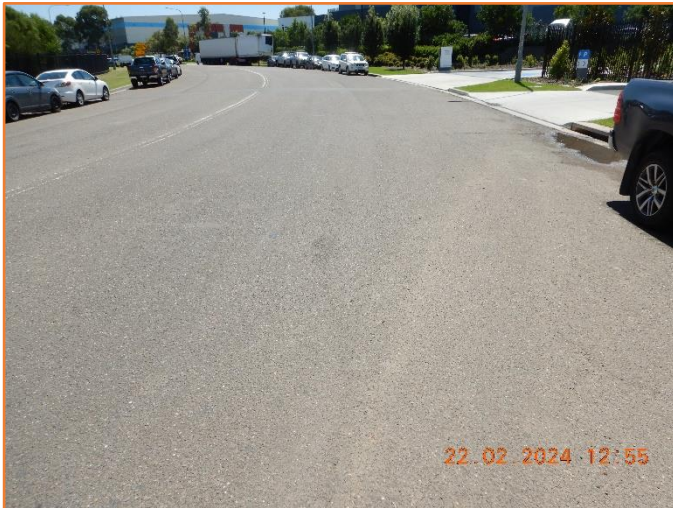
Figure 211: Reasonable - General condition of flexible pavement.
