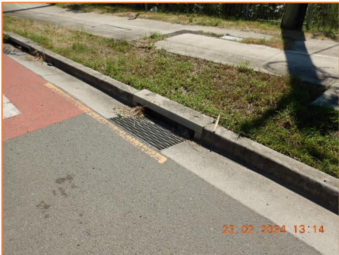
Figure 418: Reasonable - General condition of kerb inlet pit.
