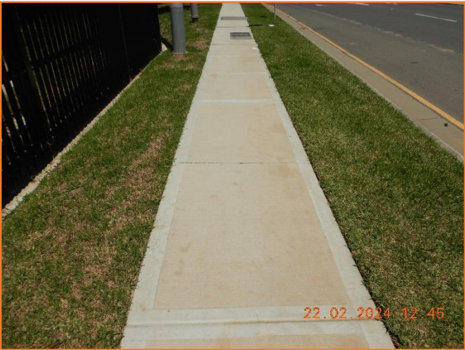
Figure 114: Good - General condition of footpath.
