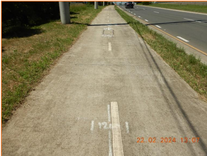
Figure 362: Reasonable - General condition of footpath.
