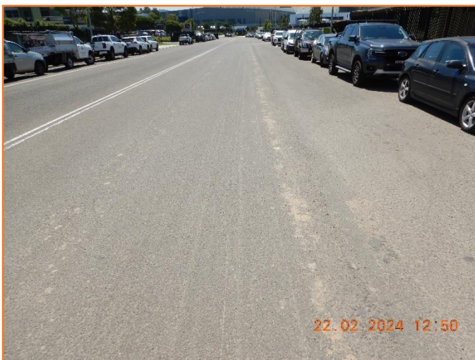
Figure 164: Reasonable - General condition of flexible pavement.
