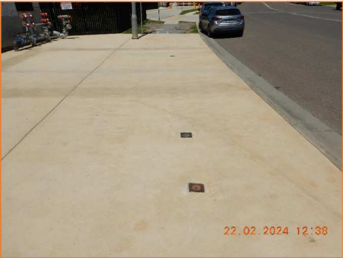
Figure 15: Good - General condition of footpath and service pits.
