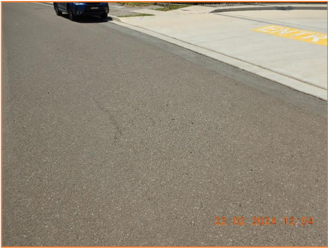
Figure 199: Reasonable - General condition of flexible pavement.
