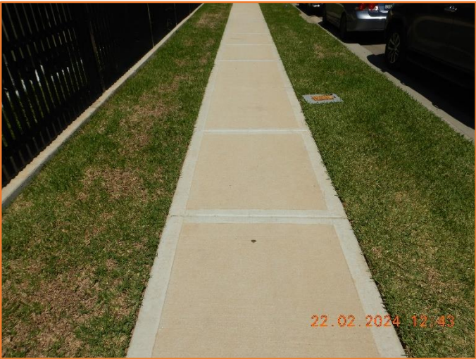
Figure 90: Good - General condition of footpath.
