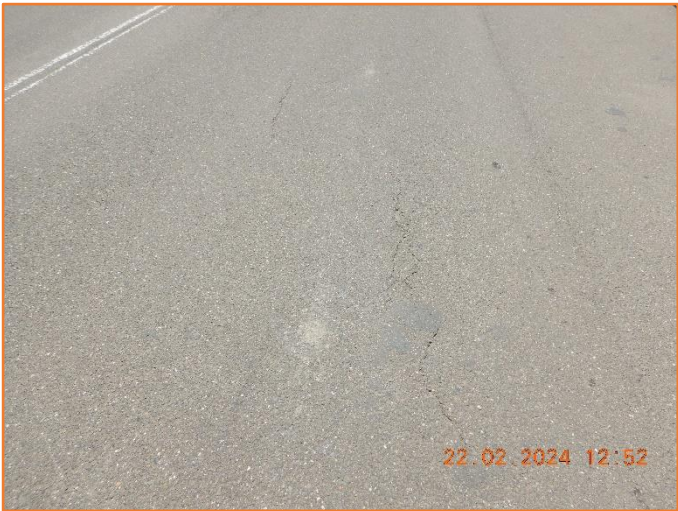
Figure 182: Reasonable - General condition of flexible pavement. Minor cracking observed.
