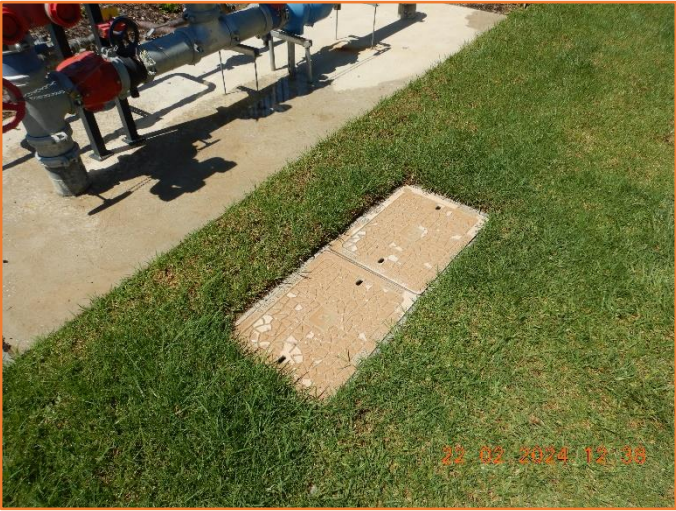
Figure 8: Reasonable - General condition of service pit.
