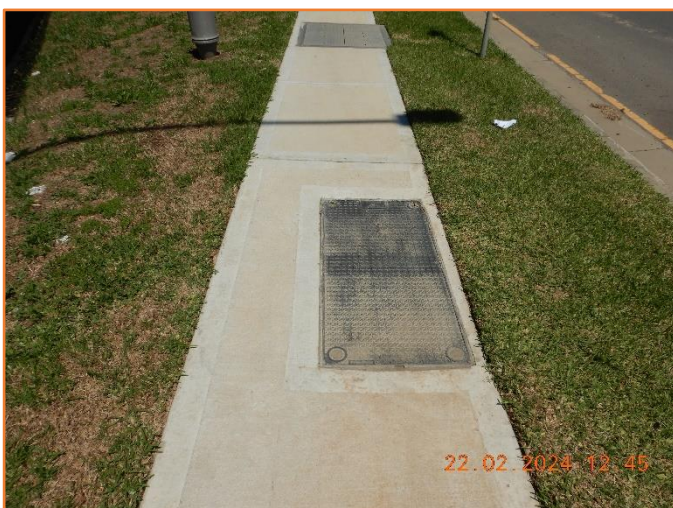
Figure 117: Reasonable - General condition of footpath and service pit.
