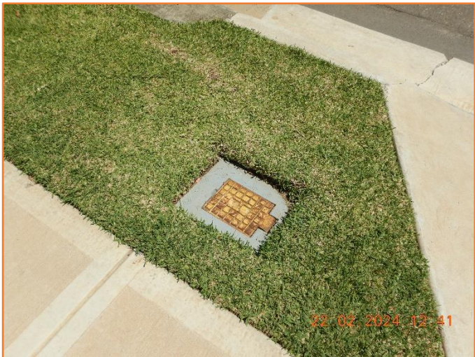
Figure 54: Reasonable - General condition of service pit.
