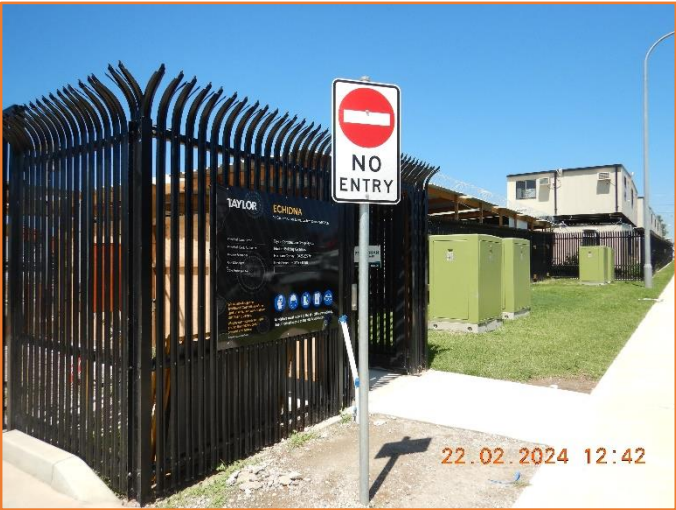
Figure 66: Good - General condition of traffic signage.
