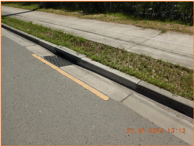
Figure 402: Reasonable - General condition of kerb and gutter and kerb inlet pit.
