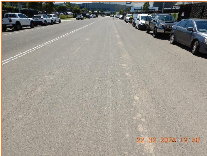
Figure 166: Reasonable - General condition of flexible pavement.
