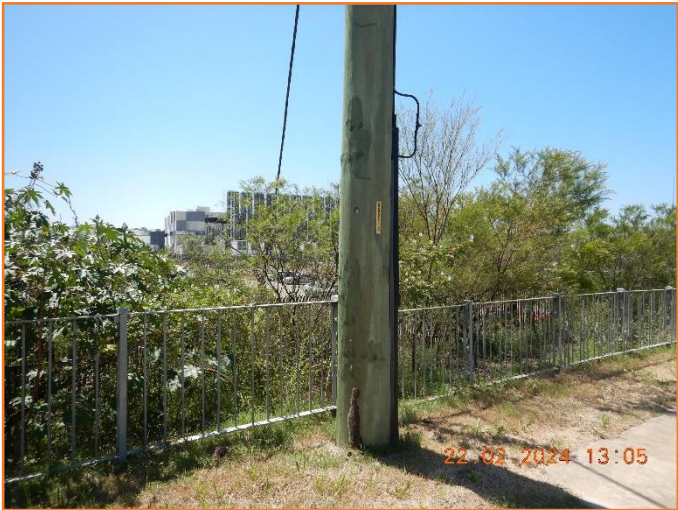
Figure 332: Reasonable - General condition of monopole assembly.
