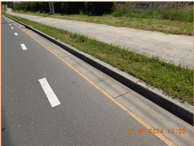
Figure 376: Reasonable - General condition of kerb and gutter.
