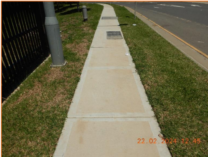
Figure 115: Good - General condition of footpath.
