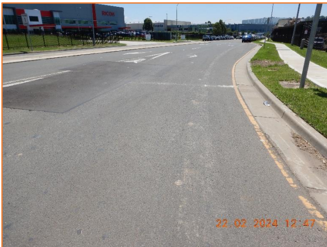
Figure 137: Reasonable - General condition of flexible pavement.
