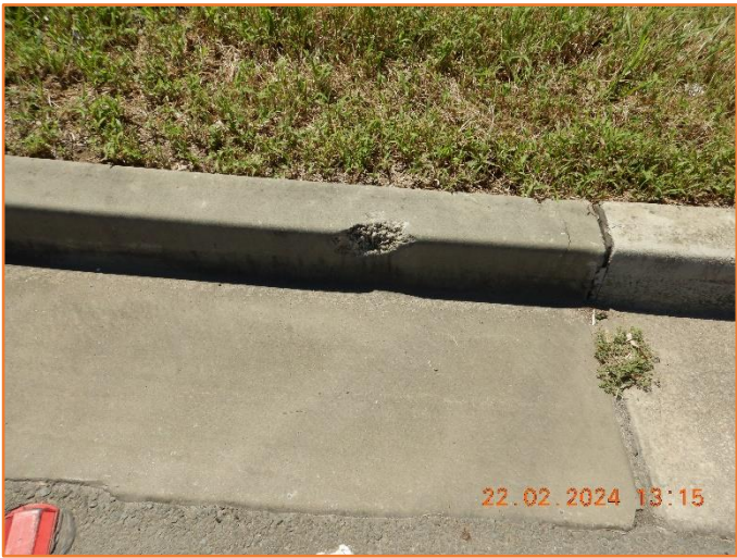
Figure 424: Reasonable - General condition of kerb and gutter. Moderate spalling observed.
