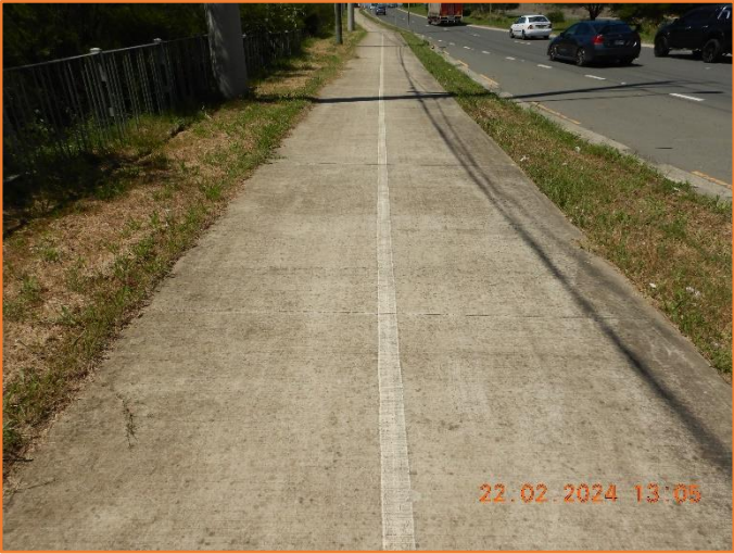
Figure 341: Reasonable - General condition of footpath.
