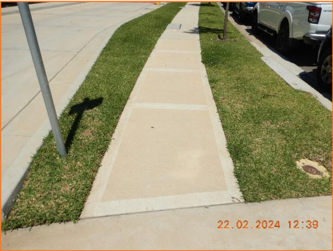
Figure 30: Good - General condition of footpath.
