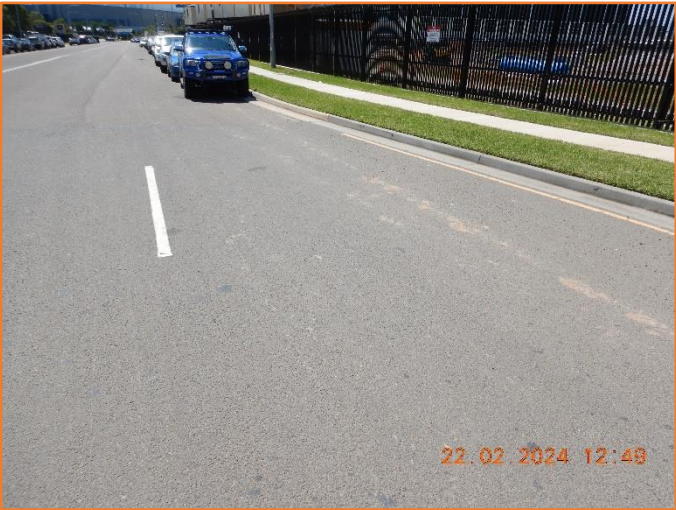
Figure 150: Reasonable - General condition of flexible pavement.
