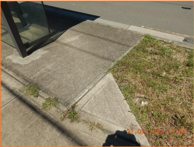
Figure 337: Reasonable - General condition of footpath.
