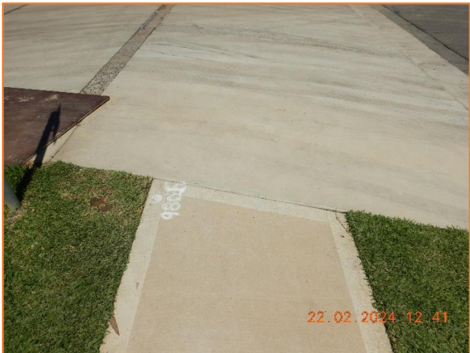
Figure 60: Good - General condition of footpath.
