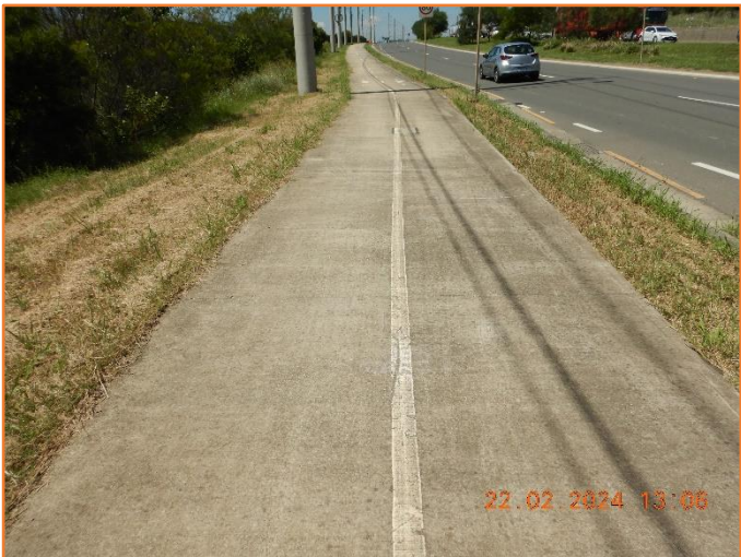
Figure 349: Reasonable - General condition of footpath.
