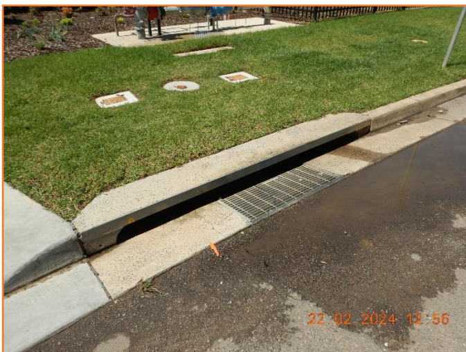
Figure 219: Reasonable - General condition of kerb inlet pit.
