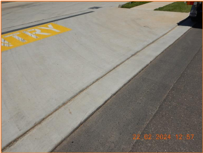
Figure 238: Reasonable - General condition of driveway layback.
