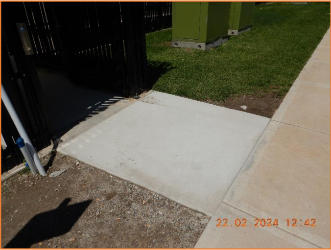
Figure 68: Good - General condition of footpath.
