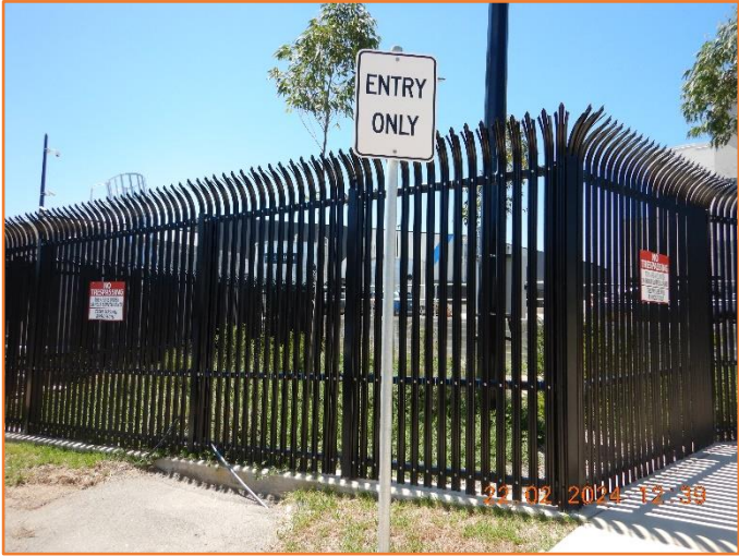
Figure 25: Good - General condition of traffic signage.
