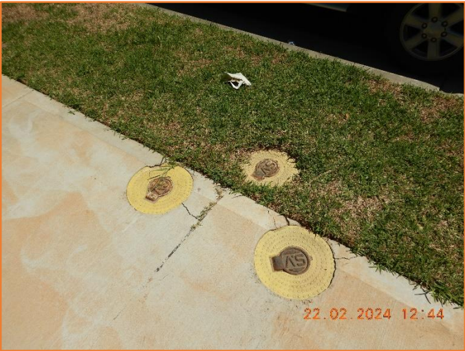
Figure 102: Reasonable - General condition of service pits. Moderate cracking observed.
