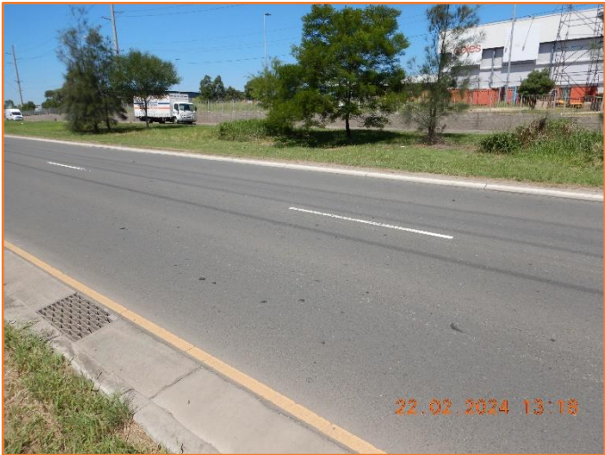
Figure 449: Reasonable - General condition of flexible pavement.
