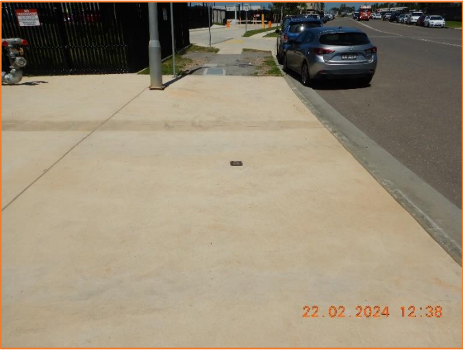
Figure 17: Reasonable - General condition of footpath.
