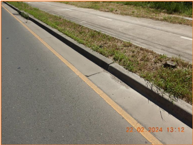
Figure 389: Reasonable - General condition of kerb and gutter.
