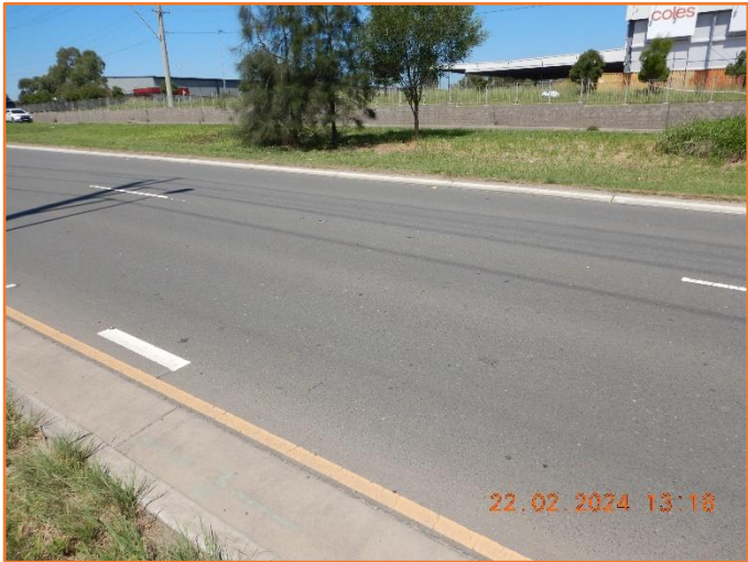
Figure 452: Reasonable - General condition of flexible pavement.
