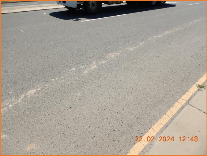
Figure 142: Reasonable - General condition of flexible pavement.
