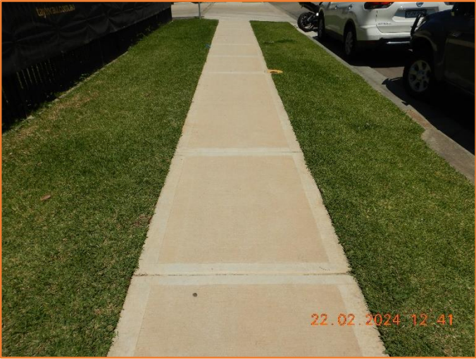
Figure 55: Good - General condition of footpath.
