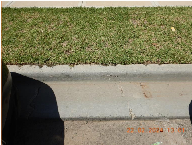
Figure 286: Reasonable - General condition of kerb and gutter. Moderate cracking observed.
