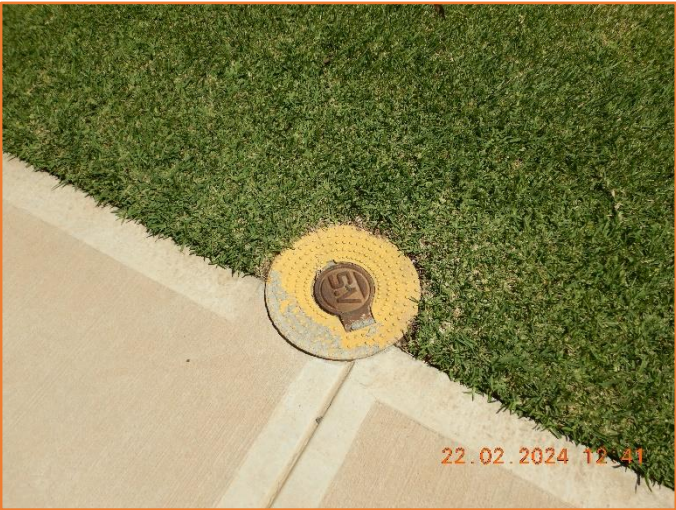
Figure 57: Good - General condition of service pit.
