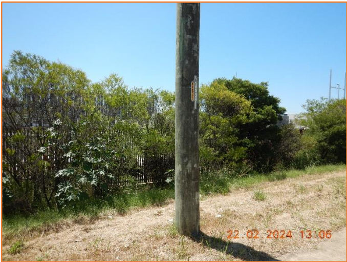
Figure 348: Reasonable - General condition of monopole assembly.
