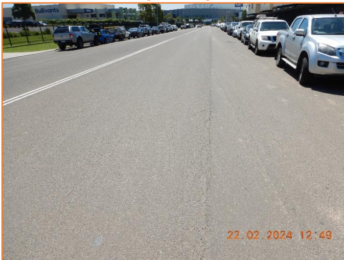
Figure 155: Reasonable - General condition of flexible pavement.
