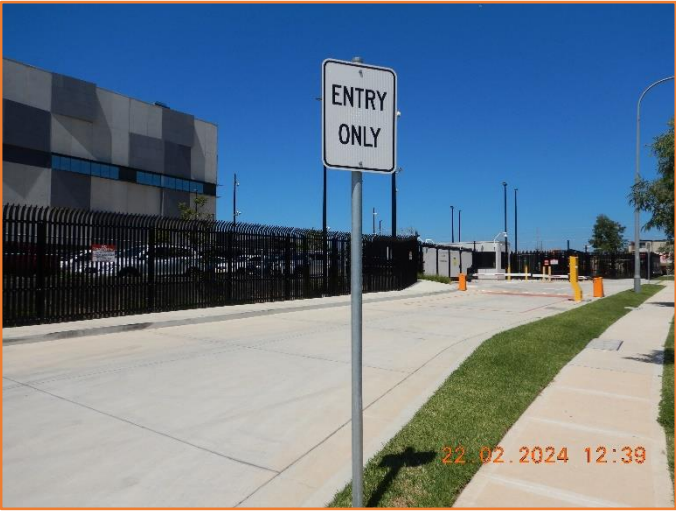
Figure 29: Good - General condition of traffic signage.
