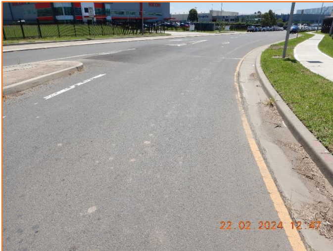
Figure 136: Reasonable - General condition of flexible pavement.
