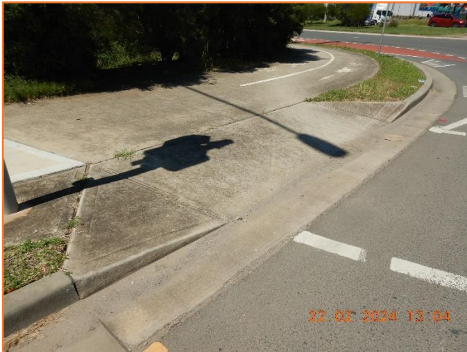
Figure 319: Reasonable - General condition of pram ramp.
