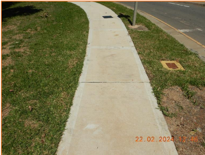
Figure 124: Good - General condition of footpath.
