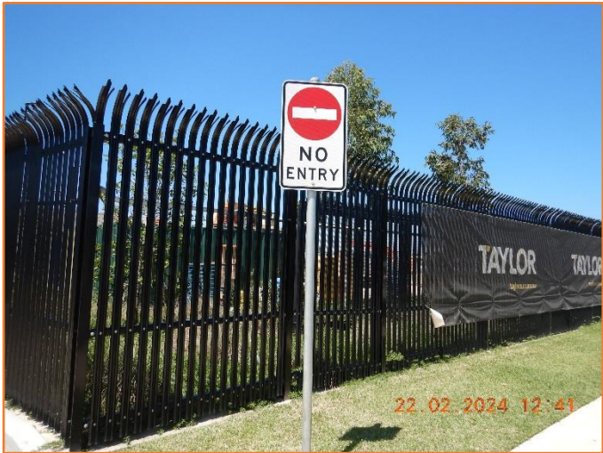
Figure 52: Good - General condition of traffic signage.
