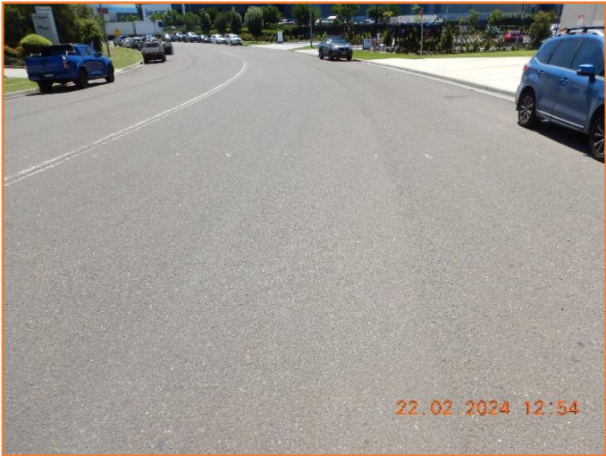
Figure 201: Reasonable - General condition of flexible pavement.
