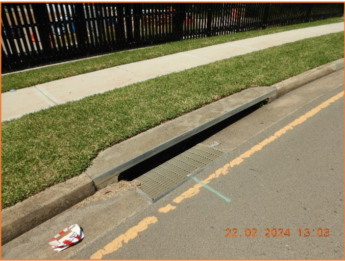
Figure 308: Reasonable - General condition of kerb inlet pit.
