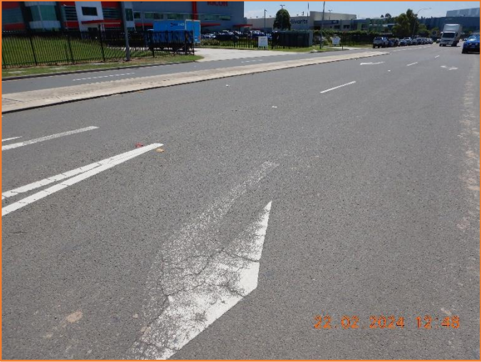
Figure 141: Reasonable - General condition of flexible pavement.
