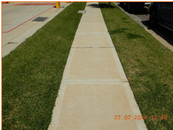
Figure 35: Good - General condition of footpath.
