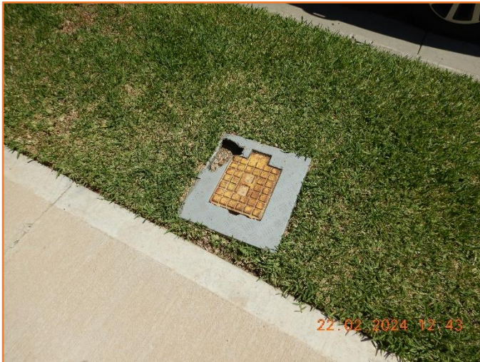
Figure 91: Good - General condition of service pit.
