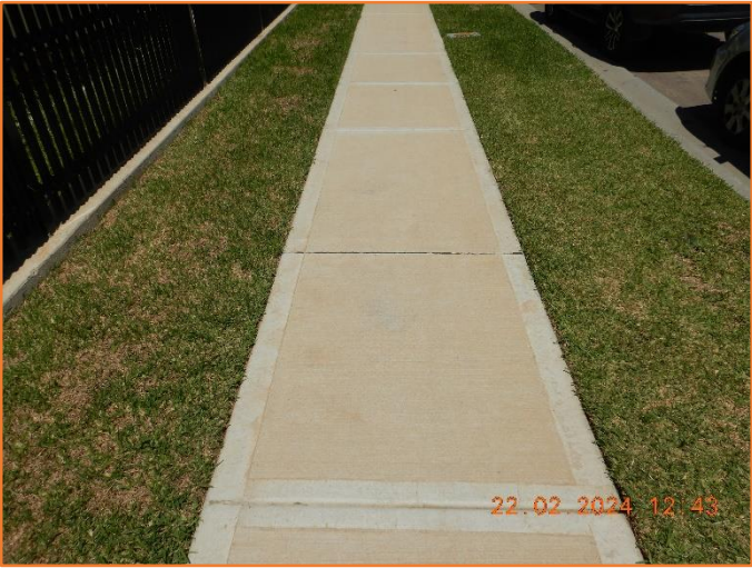
Figure 89: Good - General condition of footpath.
