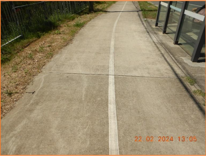
Figure 336: Reasonable - General condition of footpath.
