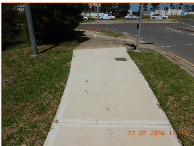
Figure 129: Good - General condition of footpath.
