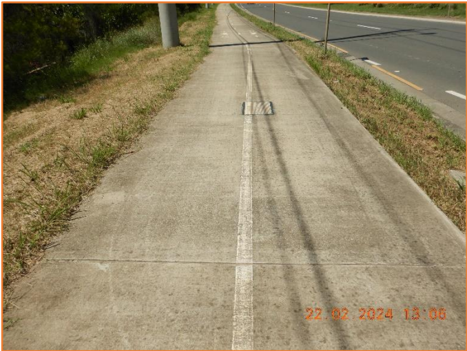
Figure 350: Reasonable - General condition of footpath.
