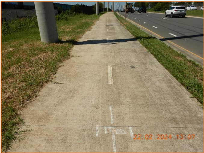
Figure 369: Reasonable - General condition of footpath.
