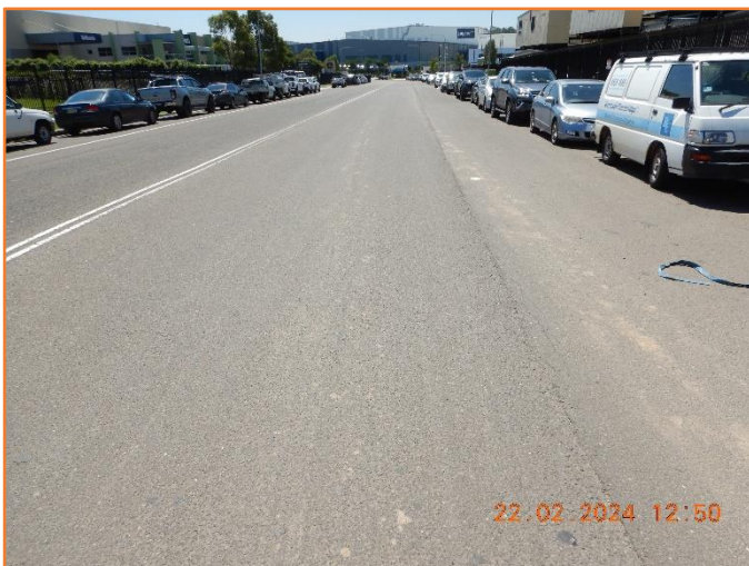
Figure 159: Reasonable - General condition of flexible pavement.
