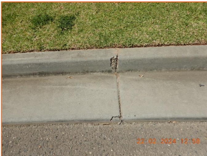
Figure 245: Reasonable - General condition of kerb and gutter. Minor spalling observed.
