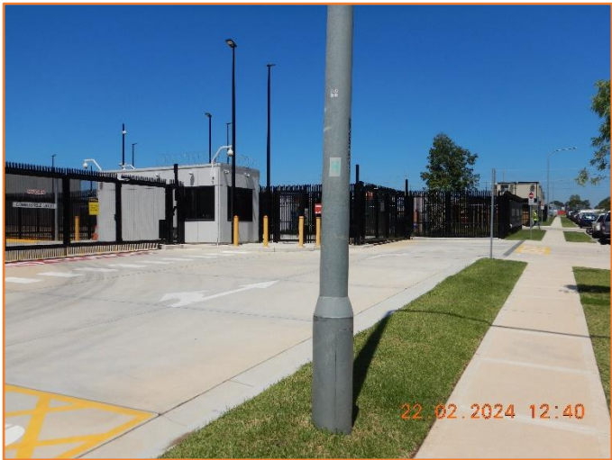
Figure 41: Good - General condition of monopole assembly.
