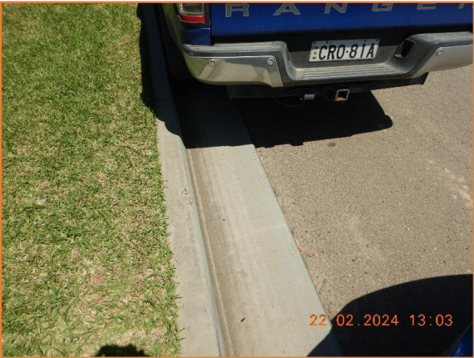
Figure 303: Reasonable - General condition of kerb and gutter.
