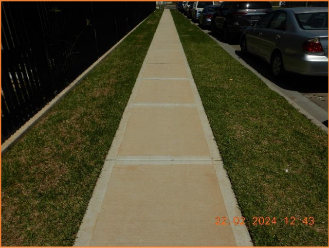
Figure 88: Good - General condition of footpath.
