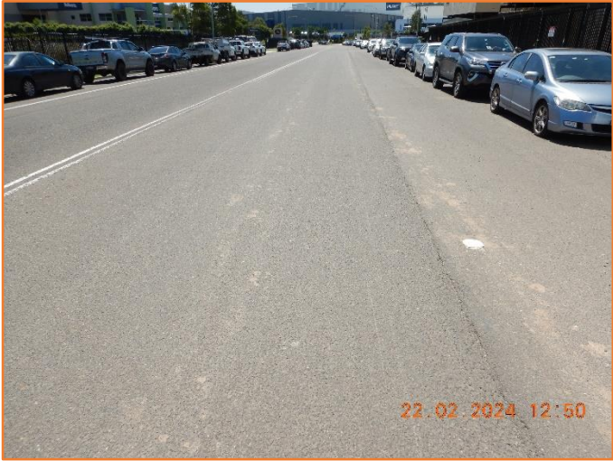
Figure 160: Reasonable - General condition of flexible pavement.
