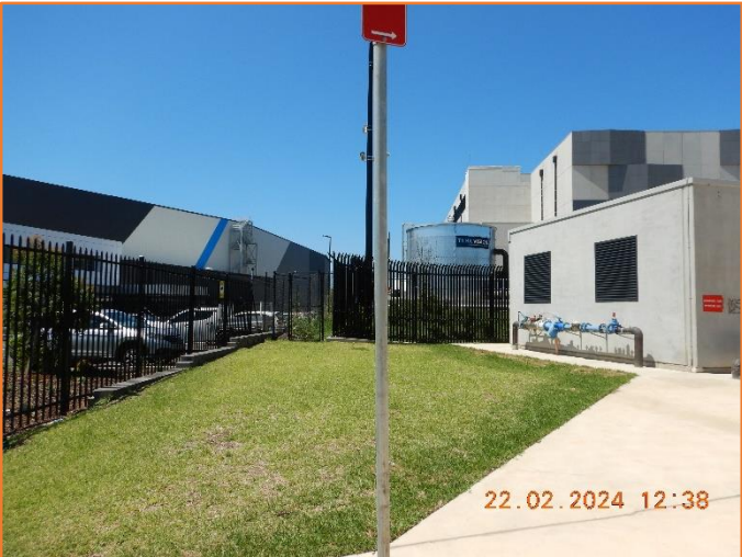
Figure 12: Good - General condition of traffic signage.
