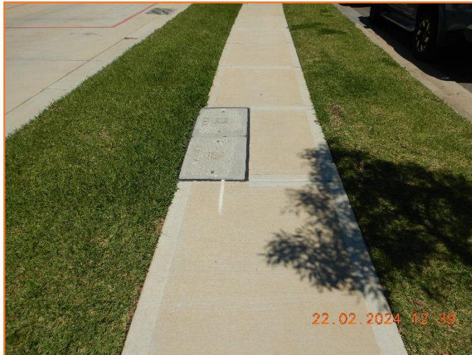
Figure 34: Good - General condition of footpath and service pits.
