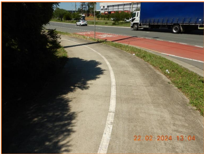
Figure 322: Reasonable - General condition of footpath.
