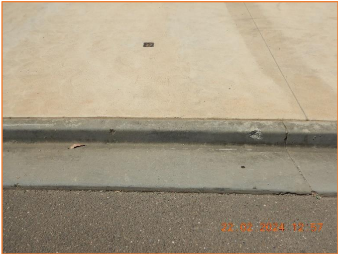
Figure 232: Reasonable - General condition of kerb and gutter. Minor spalling observed.
