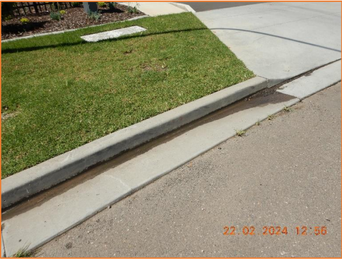
Figure 216: Reasonable - General condition of kerb and gutter.
