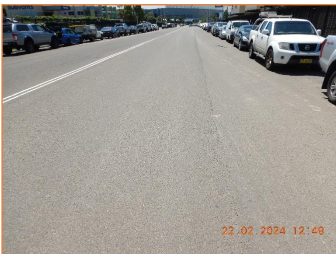
Figure 156: Reasonable - General condition of flexible pavement.
