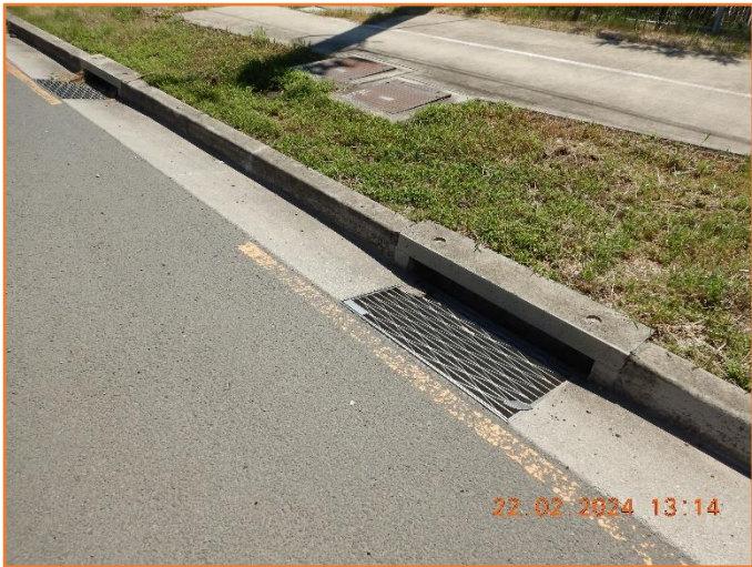
Figure 417: Reasonable - General condition of kerb inlet pit.
