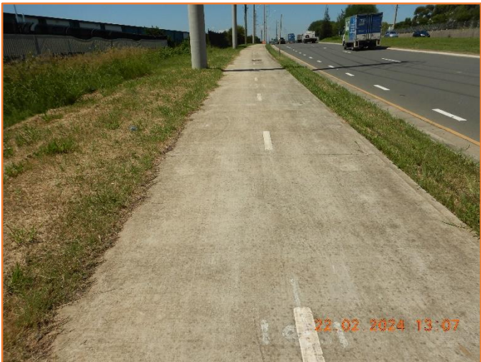
Figure 367: Reasonable - General condition of footpath.
