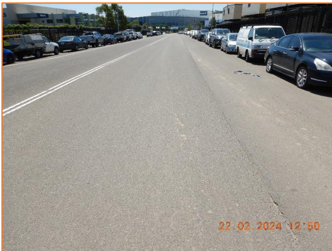
Figure 158: Reasonable - General condition of flexible pavement.
