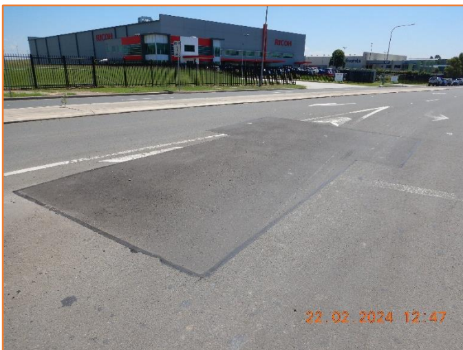
Figure 138: Reasonable - General condition of flexible pavement. Previous repair observed.
