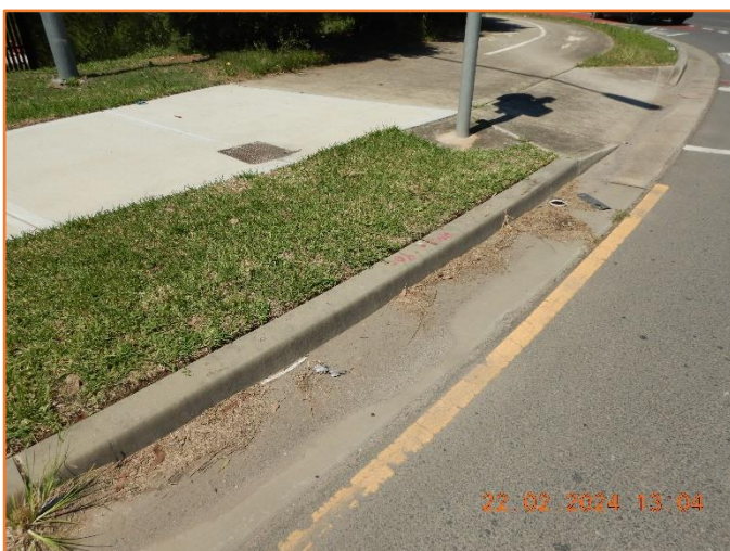
Figure 318: Reasonable - General condition of kerb and gutter.
