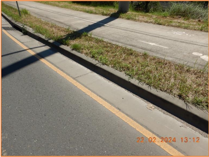
Figure 393: Reasonable - General condition of kerb and gutter.
