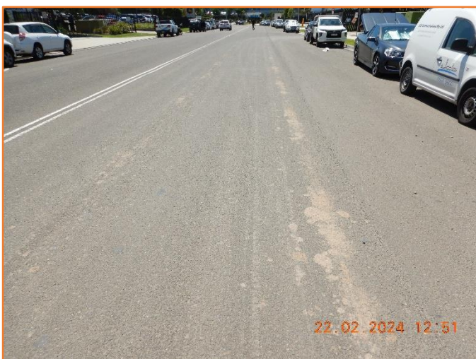
Figure 168: Reasonable - General condition of flexible pavement.
