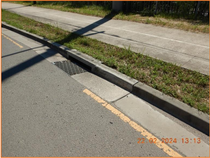
Figure 404: Reasonable - General condition of kerb and gutter and kerb inlet pit.
