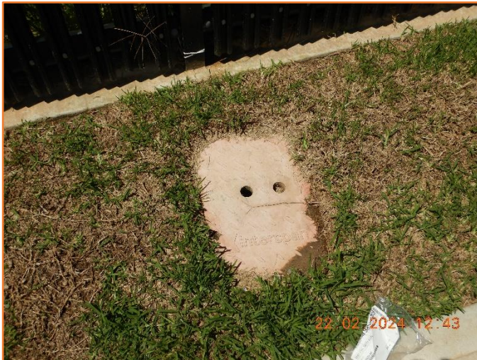
Figure 85: Reasonable - General condition of service pit. Moderate cracking observed.
