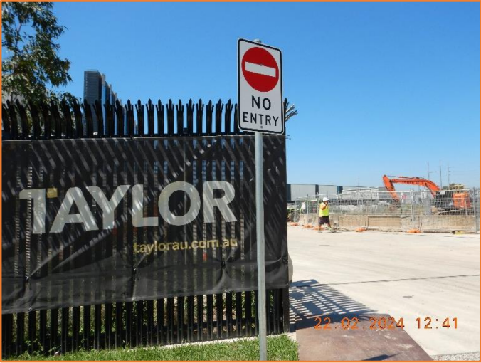
Figure 61: Good - General condition of traffic signage.
