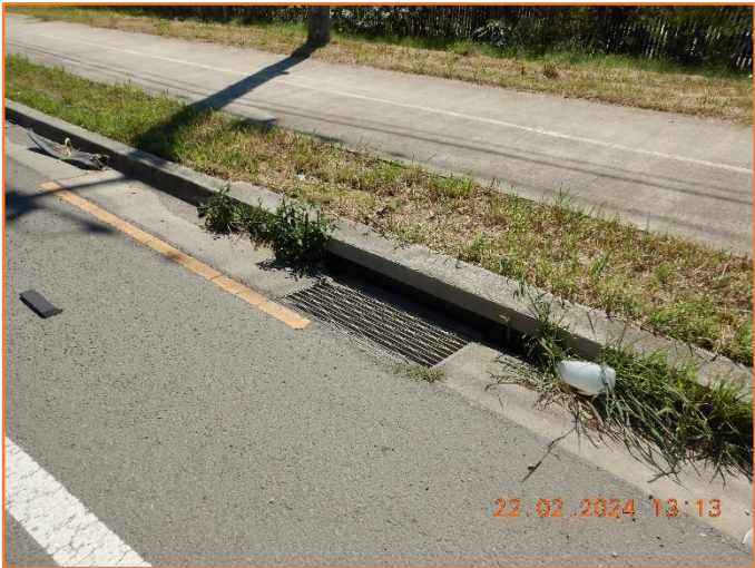
Figure 398: Reasonable - General condition of kerb inlet pit.
