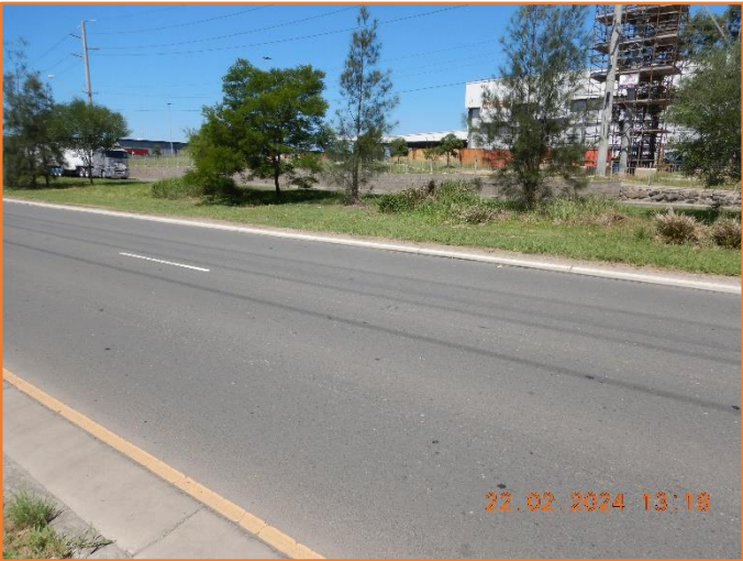
Figure 448: Reasonable - General condition of flexible pavement.
