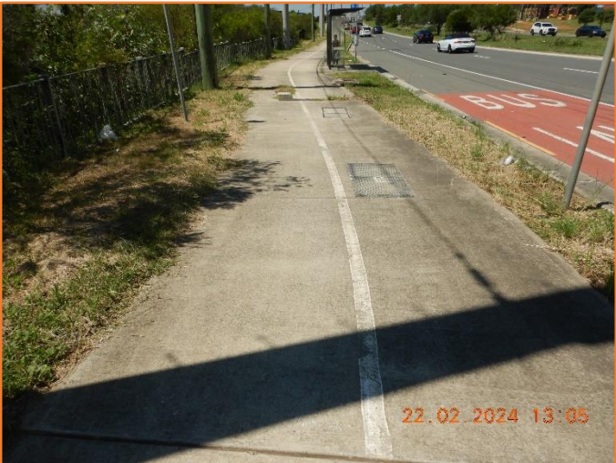
Figure 325: Reasonable - General condition of footpath.
