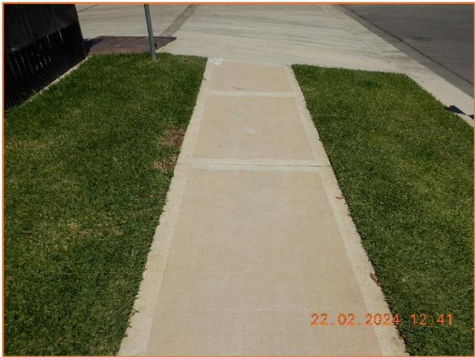
Figure 59: Good - General condition of footpath.
