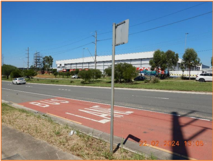
Figure 326: Good - General condition of traffic signage.
