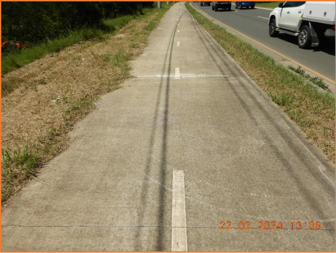
Figure 356: Reasonable - General condition of footpath.
