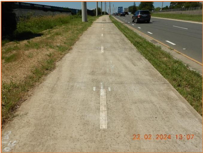
Figure 366: Reasonable - General condition of footpath.
