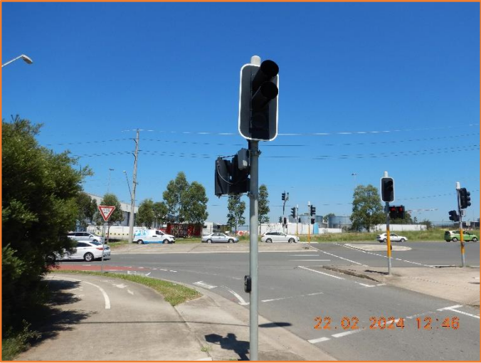
Figure 130: Good - General condition of traffic signage.
