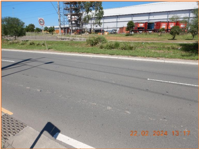
Figure 443: Reasonable - General condition of flexible pavement.
