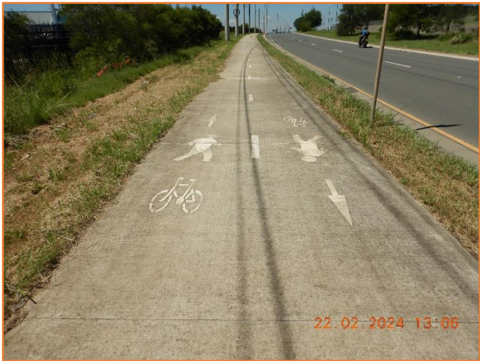
Figure 354: Reasonable - General condition of footpath.
