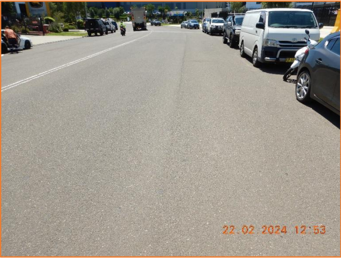
Figure 191: Reasonable - General condition of flexible pavement.
