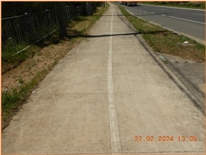
Figure 338: Reasonable - General condition of footpath.
