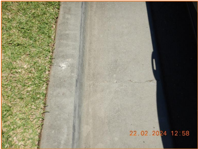
Figure 250: Reasonable - General condition of kerb and gutter. Minor cracking observed.
