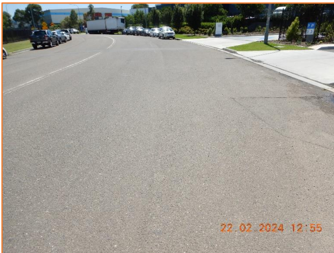
Figure 212: Reasonable - General condition of flexible pavement.
