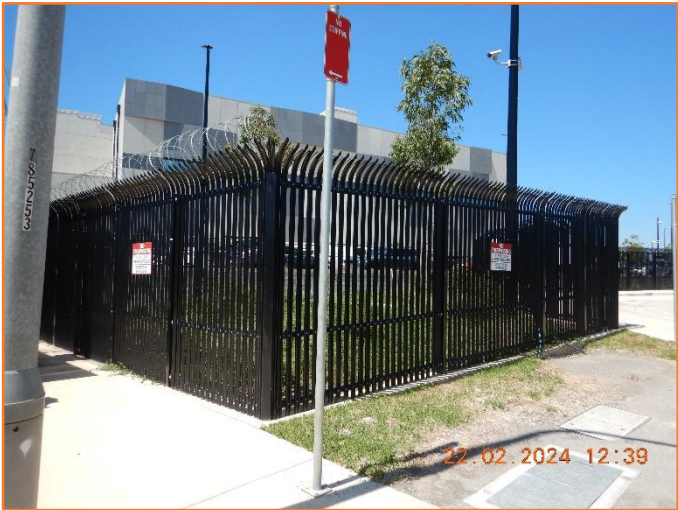
Figure 22: Good - General condition of traffic signage.
