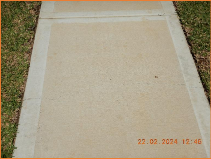
Figure 121: Reasonable - General condition of footpath. Moderate hairline cracking observed.
