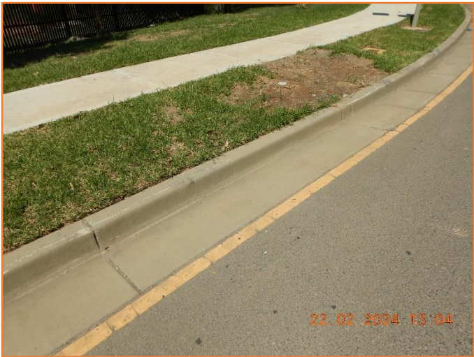
Figure 314: Reasonable - General condition of kerb and gutter.
