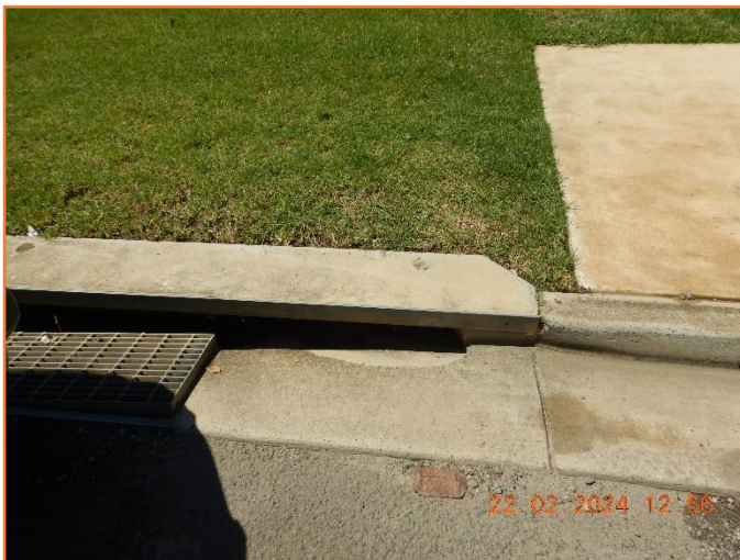
Figure 224: Reasonable - General condition of kerb inlet pit.
