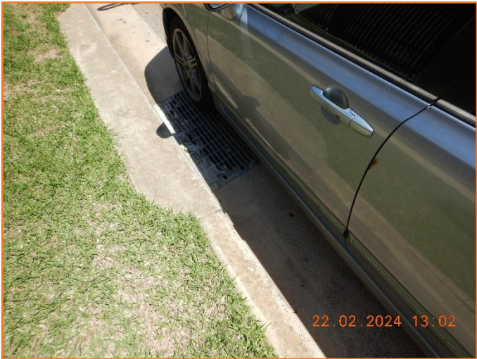
Figure 292: Reasonable - General condition of kerb inlet pit.
