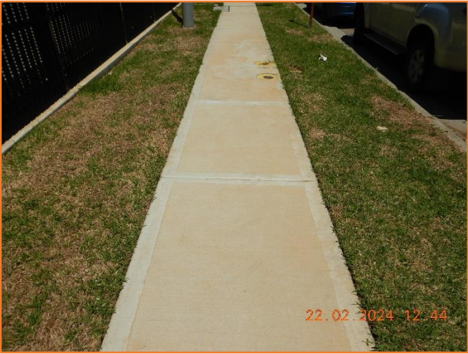
Figure 101: Good - General condition of footpath.
