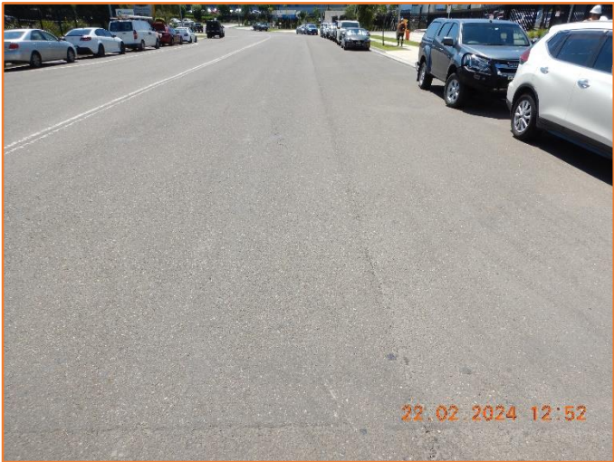
Figure 181: Reasonable - General condition of flexible pavement.
