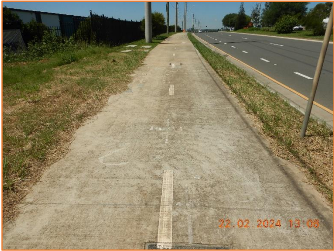
Figure 373: Reasonable - General condition of footpath.
