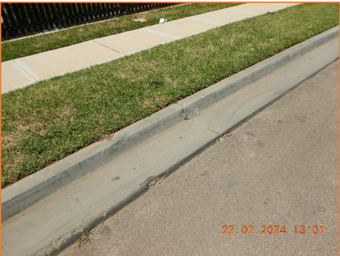
Figure 282: Reasonable - General condition of kerb and gutter.
