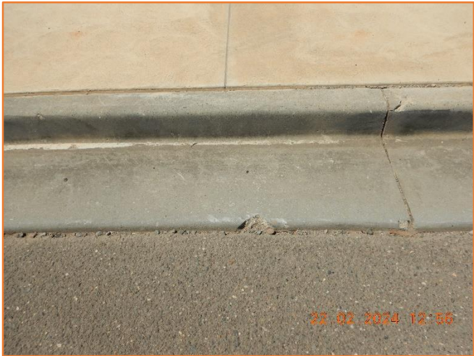
Figure 229: Reasonable - General condition of kerb and gutter. Minor spalling observed.
