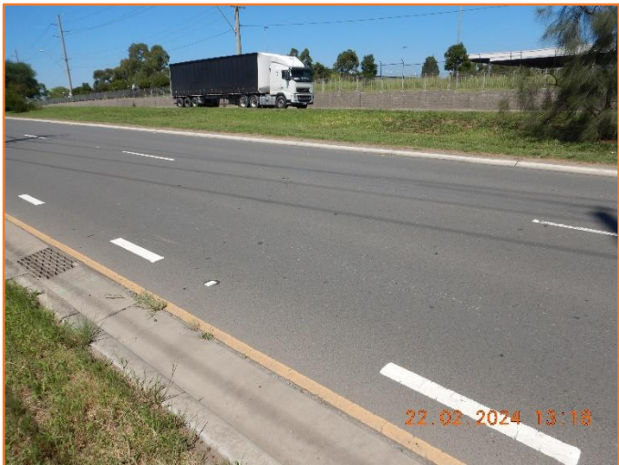
Figure 454: Reasonable - General condition of flexible pavement.
