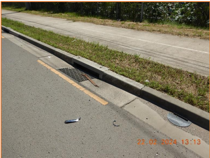
Figure 400: Reasonable - General condition of kerb and gutter and kerb inlet pit.
