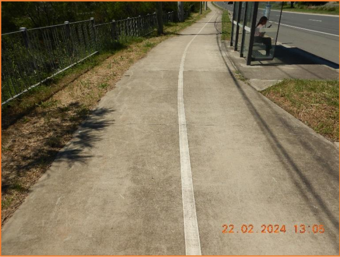
Figure 335: Reasonable - General condition of footpath.
