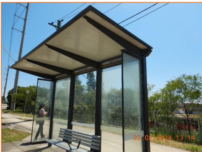
Figure 412: Reasonable - General condition of bus shelter.
