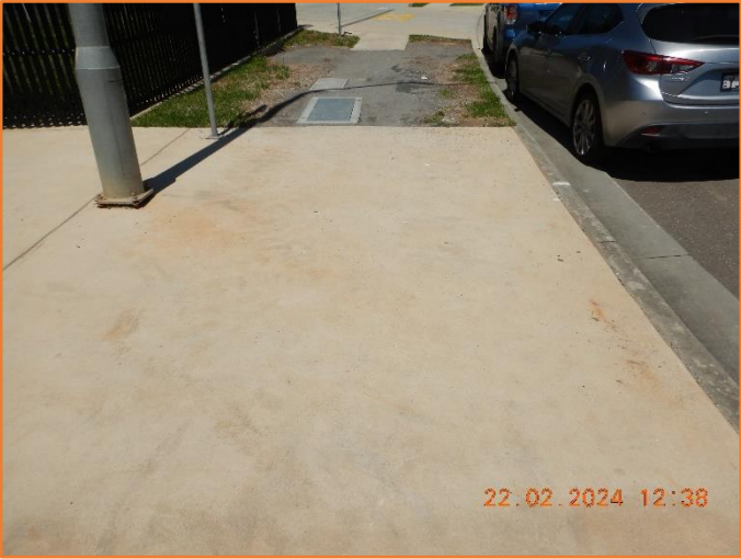
Figure 19: Reasonable - General condition of footpath.
