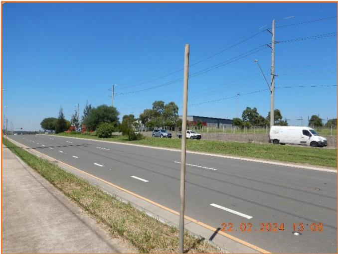
Figure 374: Defective - General condition of signage.
