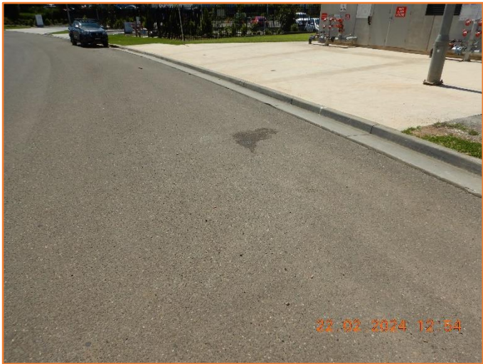
Figure 203: Reasonable - General condition of flexible pavement.
