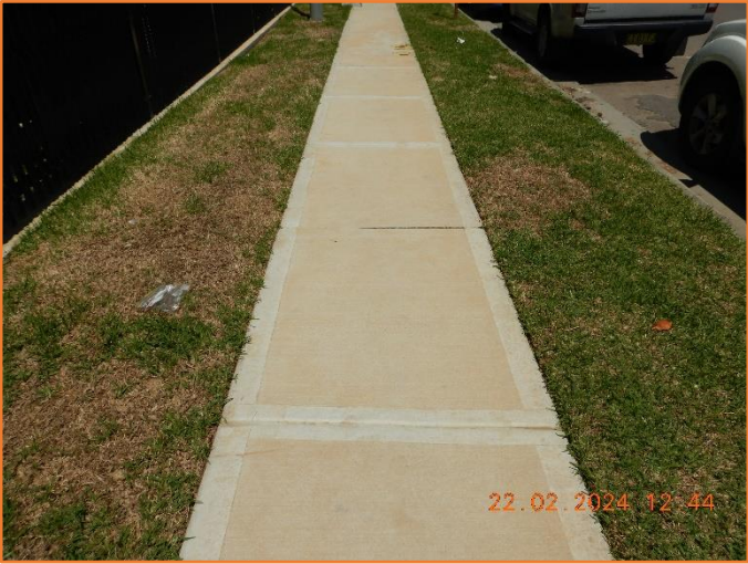
Figure 100: Good - General condition of footpath.
