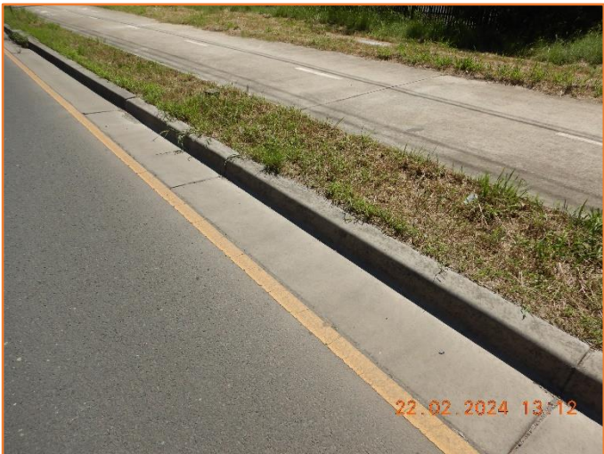
Figure 388: Reasonable - General condition of kerb and gutter.
