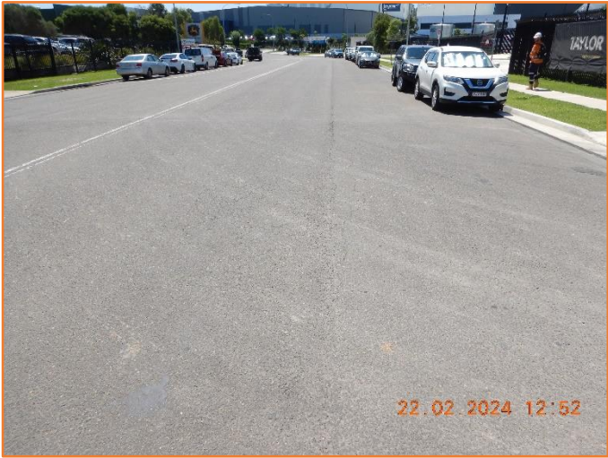
Figure 177: Reasonable - General condition of flexible pavement.
