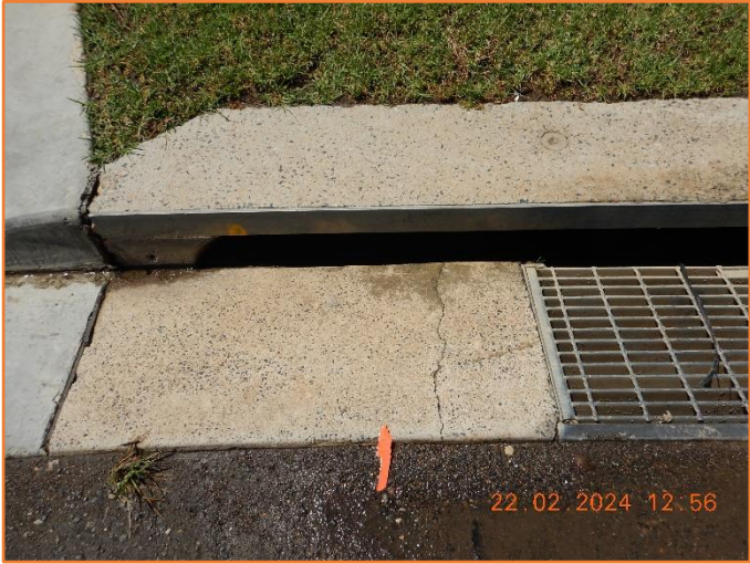
Figure 220: Reasonable - General condition of kerb inlet pit. Minor cracking observed.
