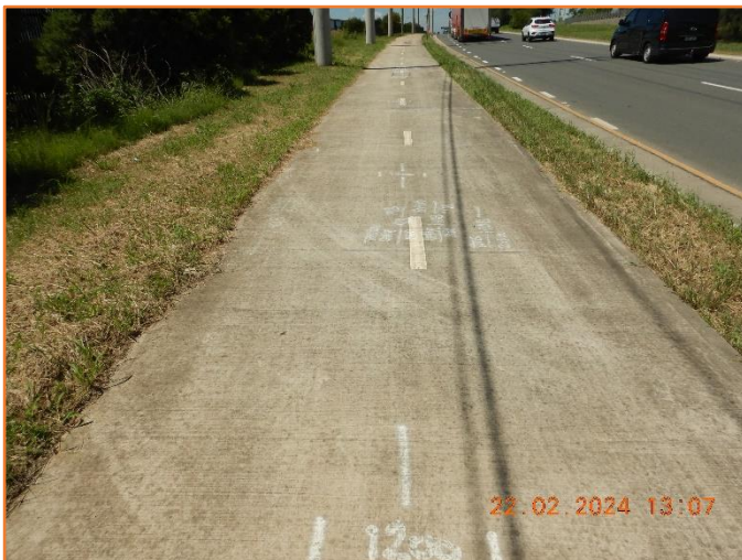
Figure 360: Reasonable - General condition of footpath.
