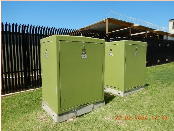
Figure 70: Good - General condition of substations.
