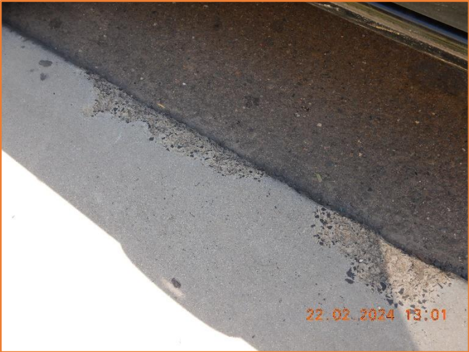
Figure 280: Reasonable - General condition of kerb and gutter. Minor spalling observed.
