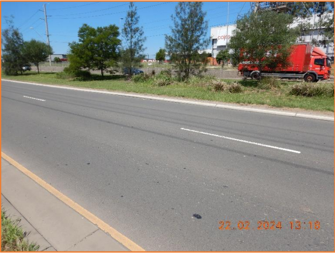
Figure 447: Reasonable - General condition of flexible pavement.
