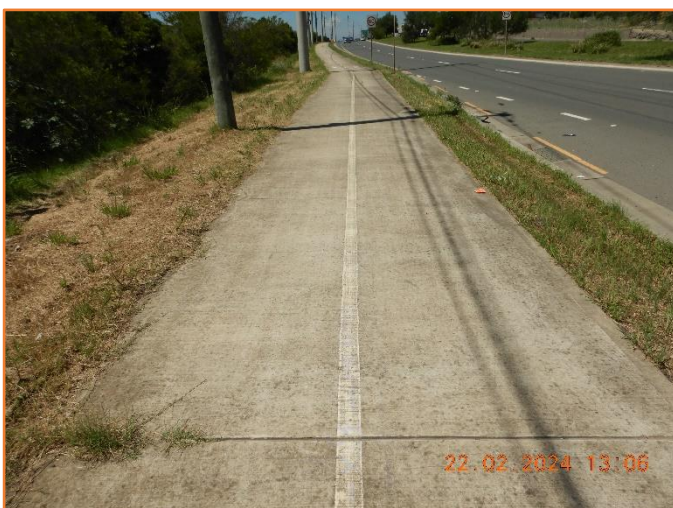
Figure 346: Reasonable - General condition of footpath.
