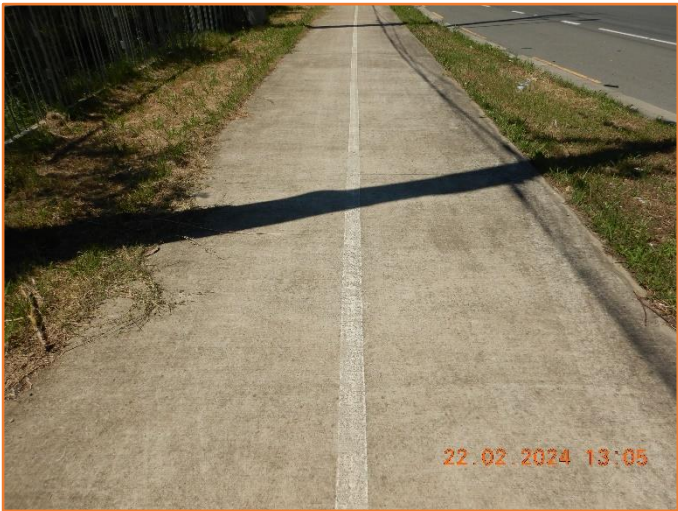
Figure 339: Reasonable - General condition of footpath.
