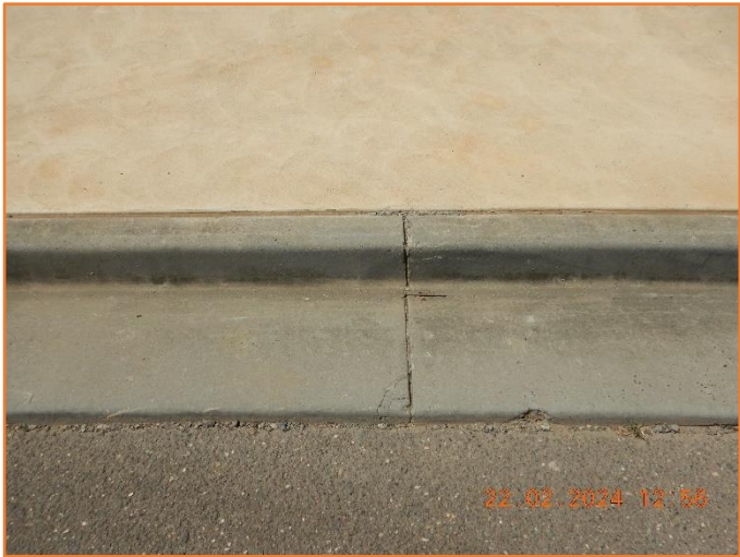
Figure 230: Reasonable - General condition of kerb and gutter. Minor hairline cracking observed.
