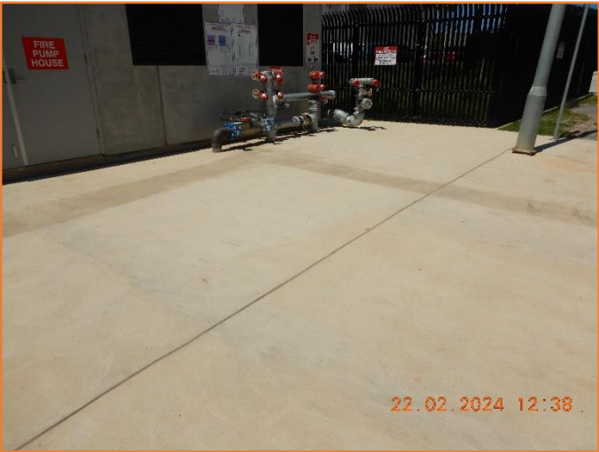
Figure 18: Reasonable - General condition of footpath.
