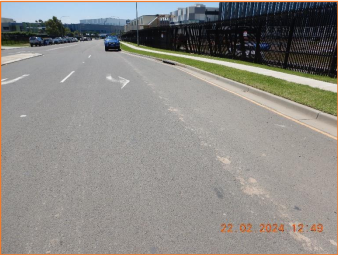
Figure 144: Reasonable - General condition of flexible pavement.
