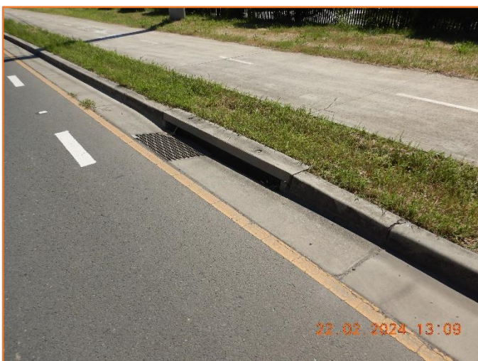
Figure 379: Reasonable - General condition of kerb inlet pit.
