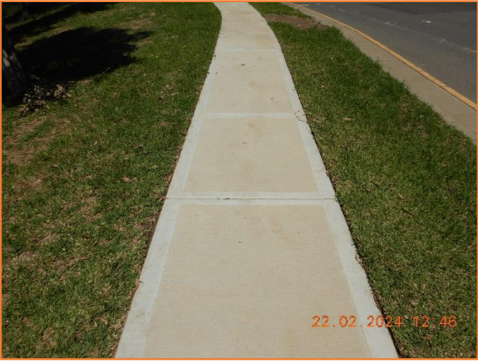
Figure 122: Good - General condition of footpath.
