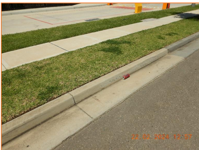
Figure 243: Reasonable - General condition of kerb and gutter.
