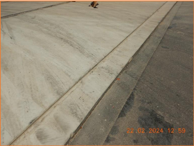
Figure 261: Reasonable - General condition of driveway layback.
