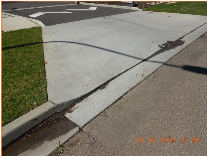
Figure 217: Reasonable - General condition of driveway layback.
