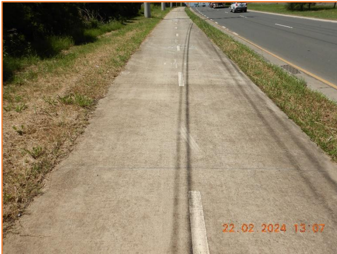
Figure 359: Reasonable - General condition of footpath.
