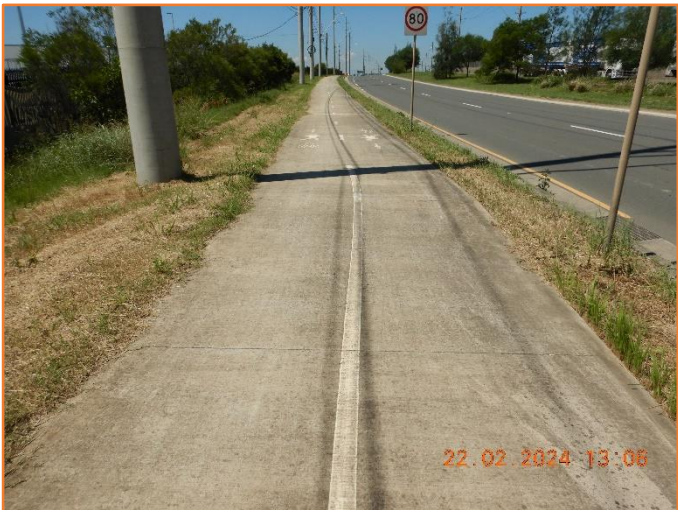
Figure 352: Reasonable - General condition of footpath.
