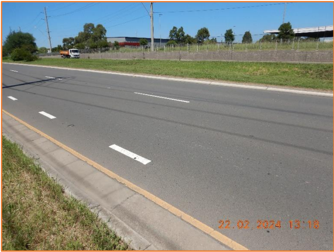
Figure 455: Reasonable - General condition of flexible pavement.
