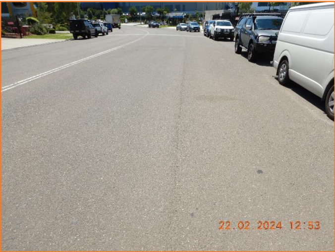
Figure 192: Reasonable - General condition of flexible pavement.
