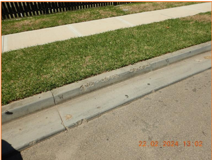
Figure 297: Poor - General condition of kerb and gutter. Moderate spalling observed.
