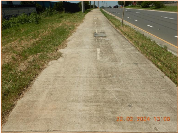
Figure 371: Reasonable - General condition of footpath.
