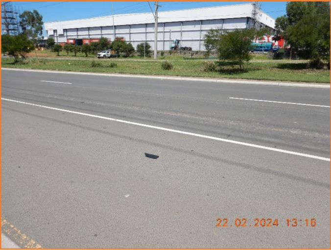
Figure 431: Reasonable - General condition of flexible pavement.
