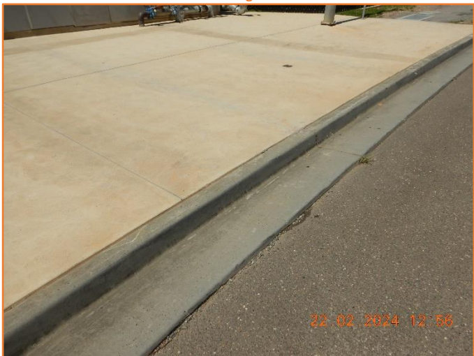
Figure 231: Reasonable - General condition of kerb and gutter.
