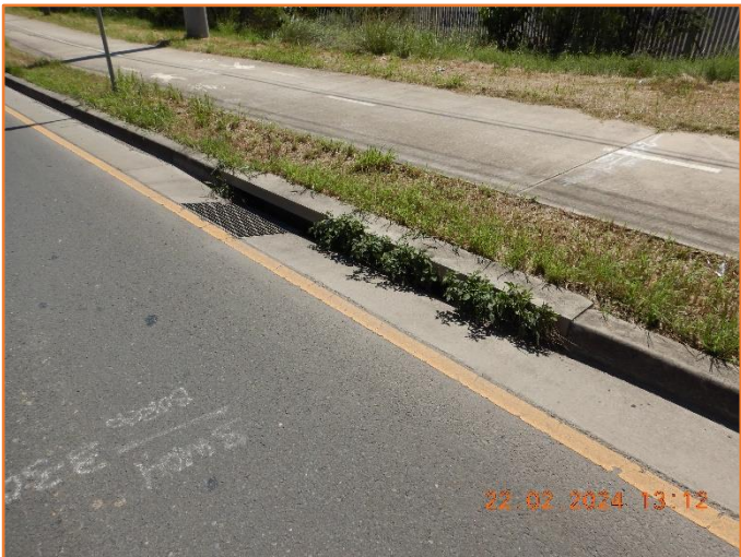
Figure 391: Reasonable - General condition of kerb inlet pit.
