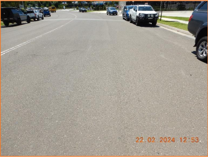
Figure 194: Reasonable - General condition of flexible pavement.
