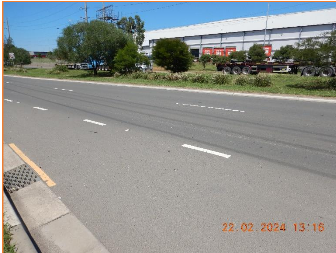
Figure 437: Reasonable - General condition of flexible pavement.
