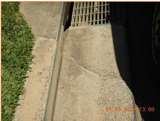
Figure 275: Reasonable - General condition of kerb inlet pit. Moderate cracking observed.
