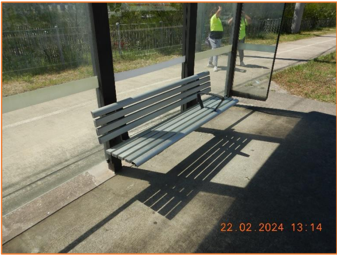
Figure 414: Reasonable - General condition of bus shelter.
