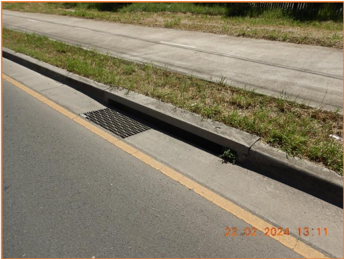
Figure 386: Reasonable - General condition of kerb inlet pit.
