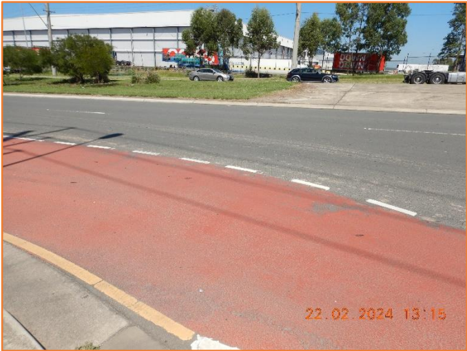
Figure 427: Reasonable - General condition of flexible pavement.
