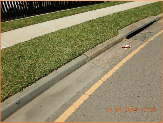
Figure 307: Reasonable - General condition of kerb and gutter.
