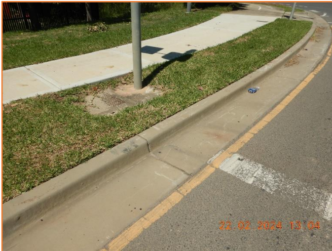
Figure 316: Reasonable - General condition of kerb and gutter.
