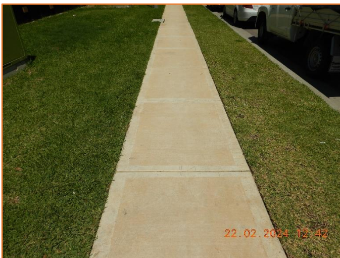
Figure 71: Good - General condition of footpath.
