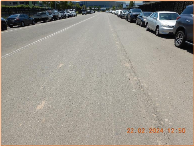
Figure 162: Reasonable - General condition of flexible pavement.
