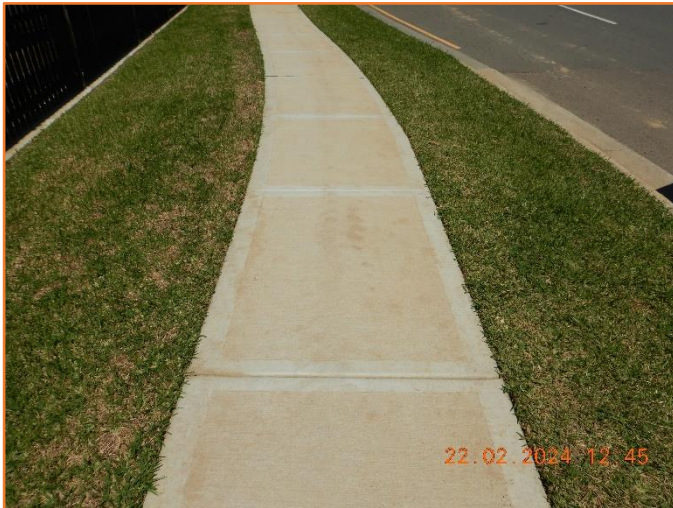
Figure 109: Good - General condition of footpath.
