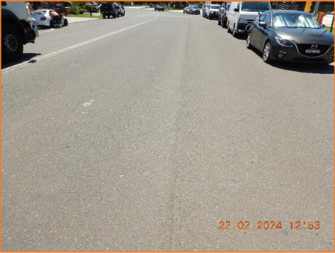
Figure 190: Reasonable - General condition of flexible pavement.
