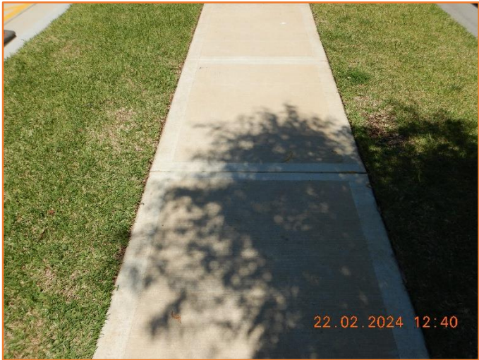
Figure 40: Good - General condition of footpath.
