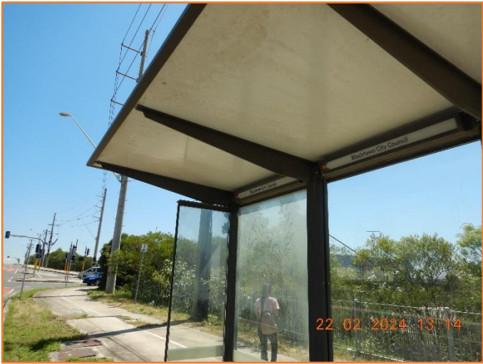
Figure 413: Reasonable - General condition of bus shelter.
