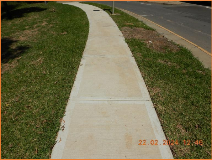
Figure 123: Good - General condition of footpath.
