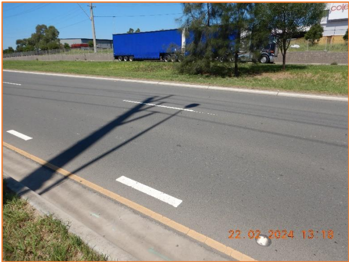
Figure 453: Reasonable - General condition of flexible pavement.
