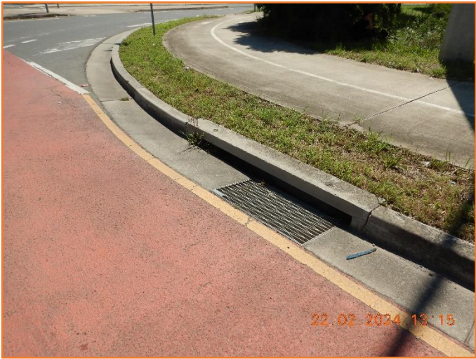
Figure 422: Reasonable - General condition of kerb inlet pit.
