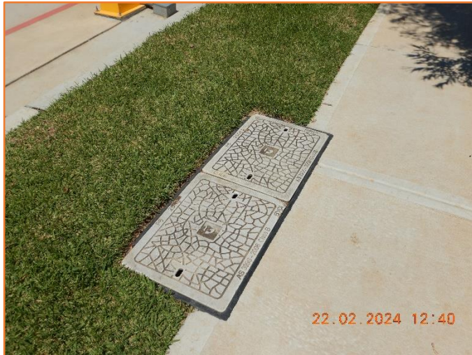
Figure 37: Good - General condition of service pits.
