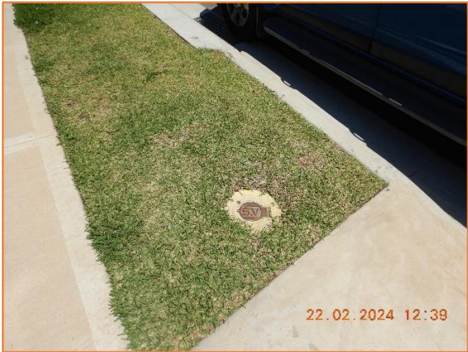
Figure 31: Reasonable - General condition of service pit.
