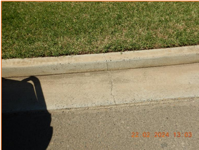
Figure 304: Reasonable - General condition of kerb and gutter. Moderate hairline cracking observed.
