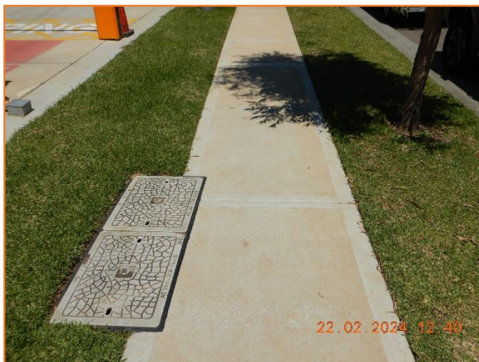
Figure 38: Good - General condition of footpath.
