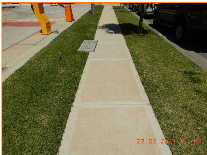
Figure 36: Good - General condition of footpath.
