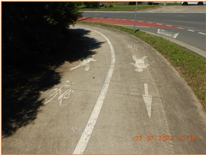
Figure 320: Reasonable - General condition of footpath.
