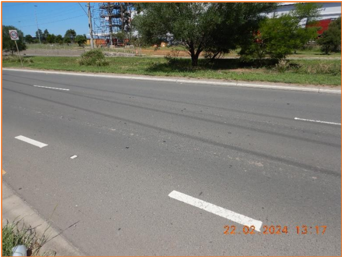
Figure 440: Reasonable - General condition of flexible pavement.
