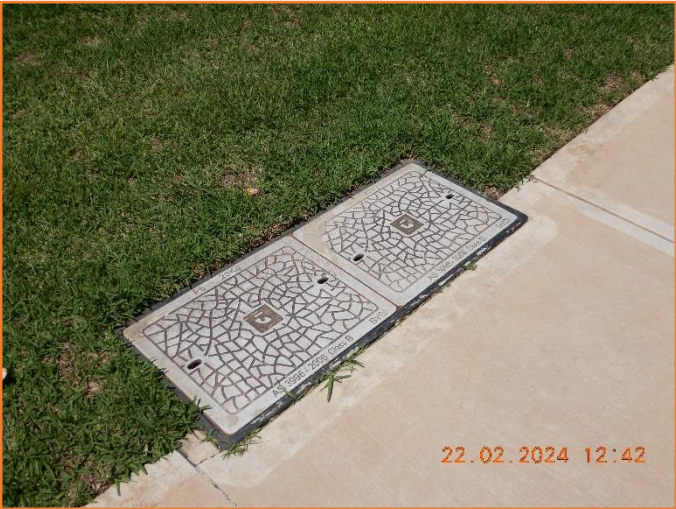
Figure 74: Reasonable - General condition of service pit. Moderate cracking observed.
