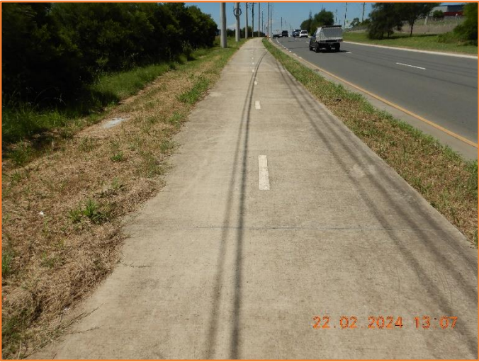
Figure 357: Reasonable - General condition of footpath.
