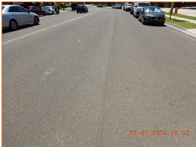
Figure 188: Reasonable - General condition of flexible pavement.
