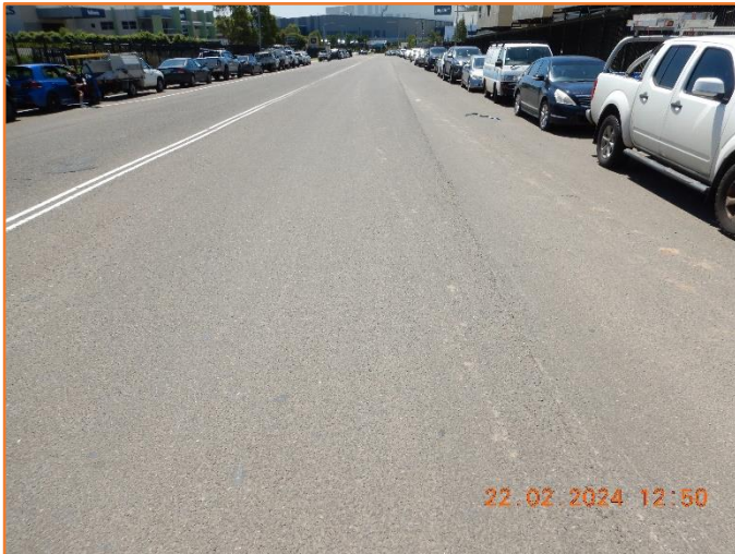
Figure 157: Reasonable - General condition of flexible pavement.
