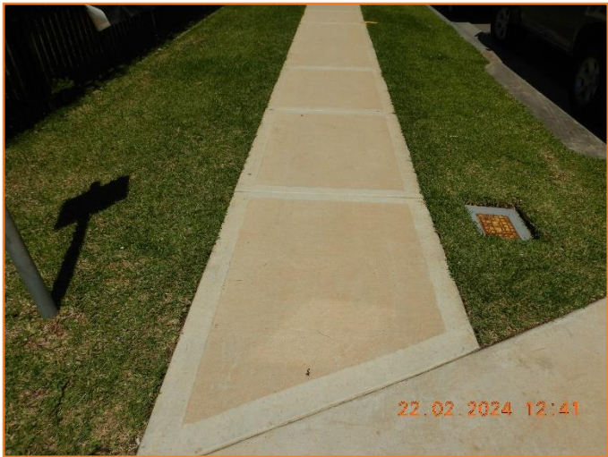
Figure 53: Good - General condition of footpath.
