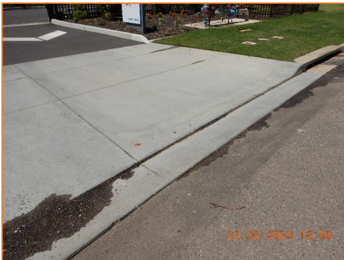
Figure 218: Reasonable - General condition of driveway layback.
