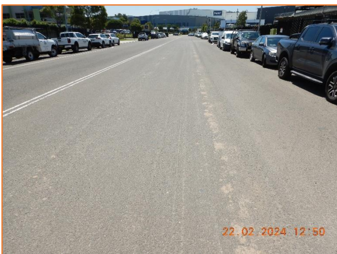
Figure 165: Reasonable - General condition of flexible pavement.
