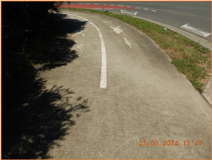
Figure 135: Reasonable - General condition of footpath.
