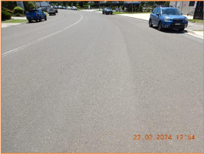
Figure 200: Reasonable - General condition of flexible pavement.
