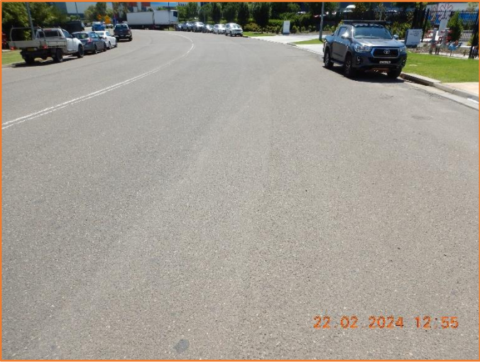
Figure 208: Reasonable - General condition of flexible pavement.
