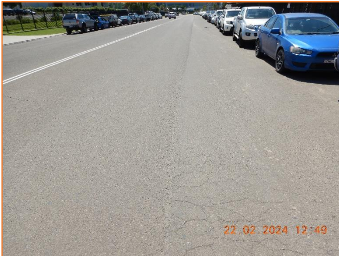
Figure 154: Reasonable - General condition of flexible pavement. Moderate alligator cracking observed.
