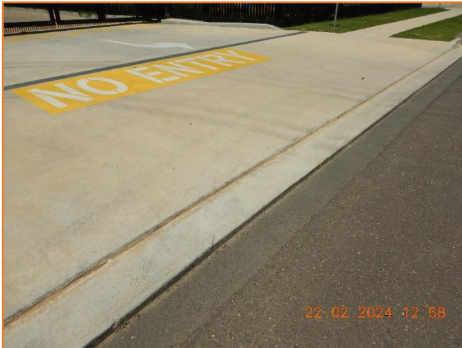
Figure 253: Reasonable - General condition of driveway layback.
