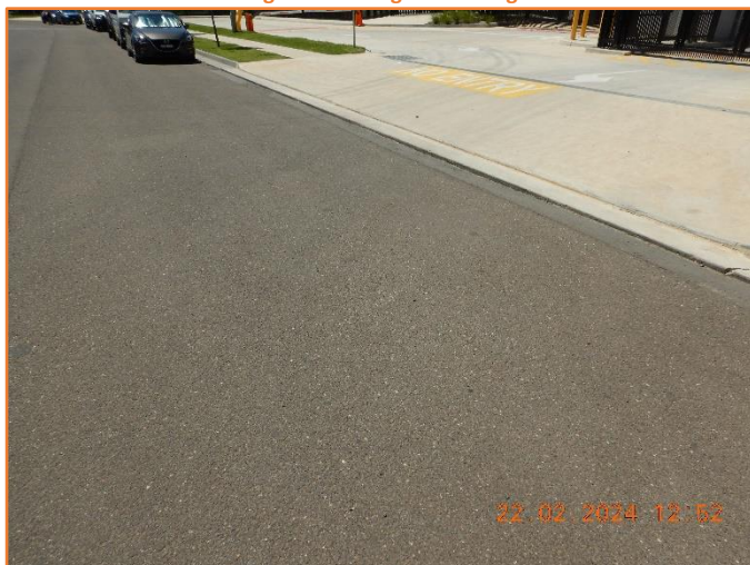
Figure 185: Reasonable - General condition of flexible pavement.
