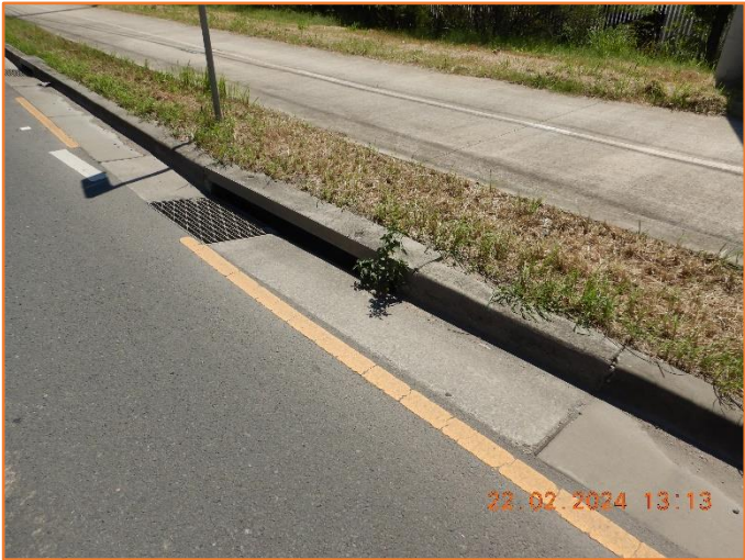
Figure 394: Reasonable - General condition of kerb inlet pit.
