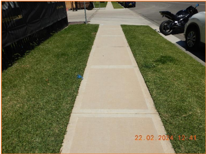
Figure 58: Good - General condition of footpath.
