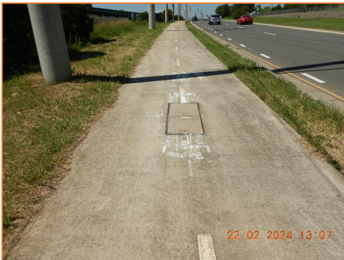
Figure 363: Reasonable - General condition of footpath.
