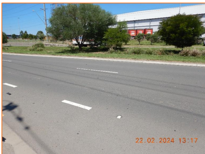
Figure 439: Reasonable - General condition of flexible pavement.
