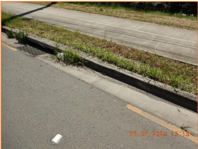
Figure 397: Reasonable - General condition of kerb and gutter.
