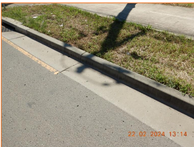
Figure 409: Reasonable - General condition of kerb and gutter.
