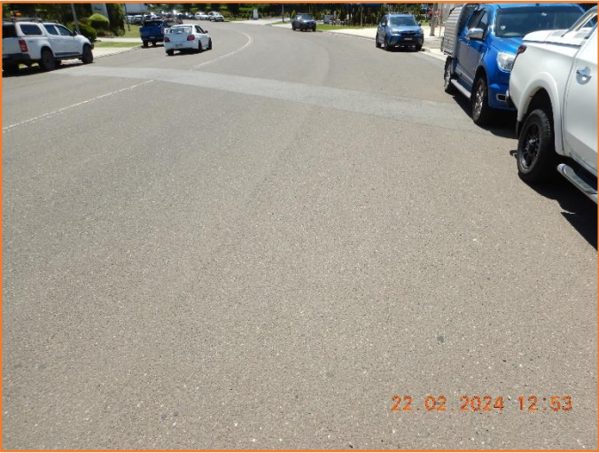
Figure 197: Reasonable - General condition of flexible pavement.
