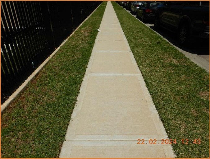
Figure 83: Good - General condition of footpath.
