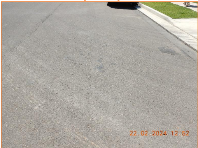
Figure 180: Reasonable - General condition of flexible pavement.
