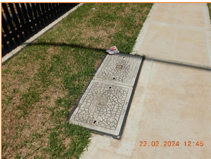
Figure 107: Reasonable - General condition of service pits.
