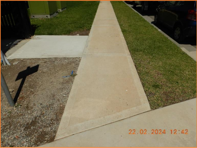
Figure 67: Good - General condition of footpath.
