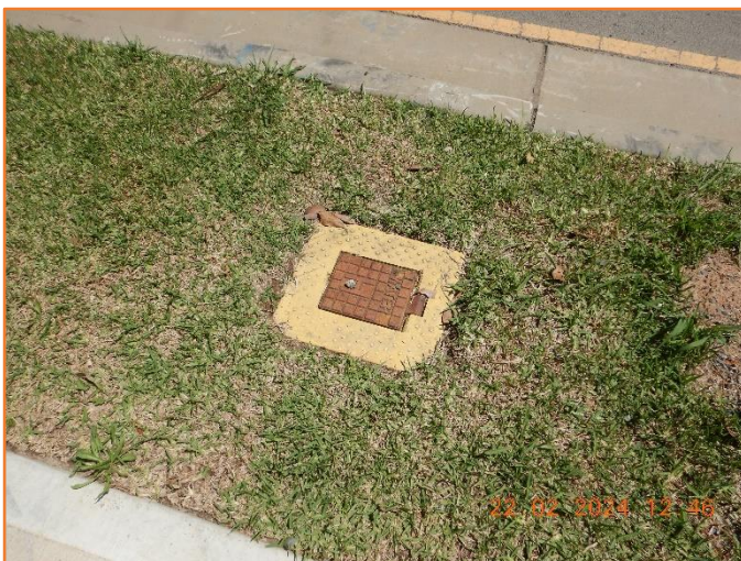
Figure 125: Good - General condition of service pit.
