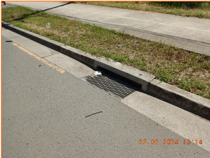
Figure 407: Reasonable - General condition of kerb inlet pit.
