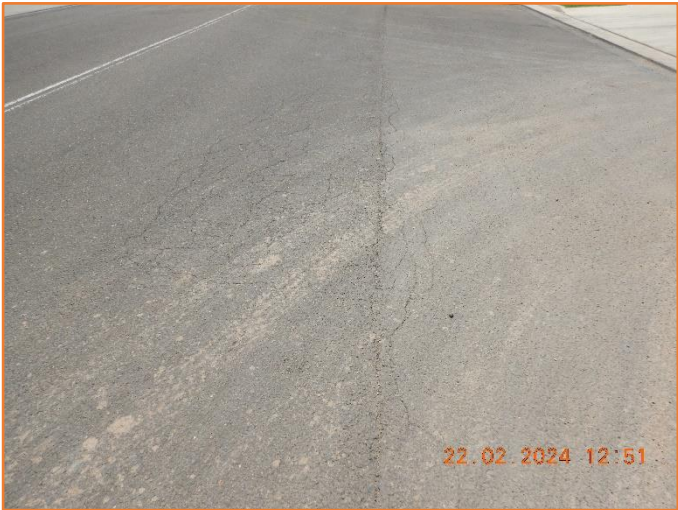
Figure 175: Reasonable - General condition of flexible pavement. Moderate alligator cracking observed.
