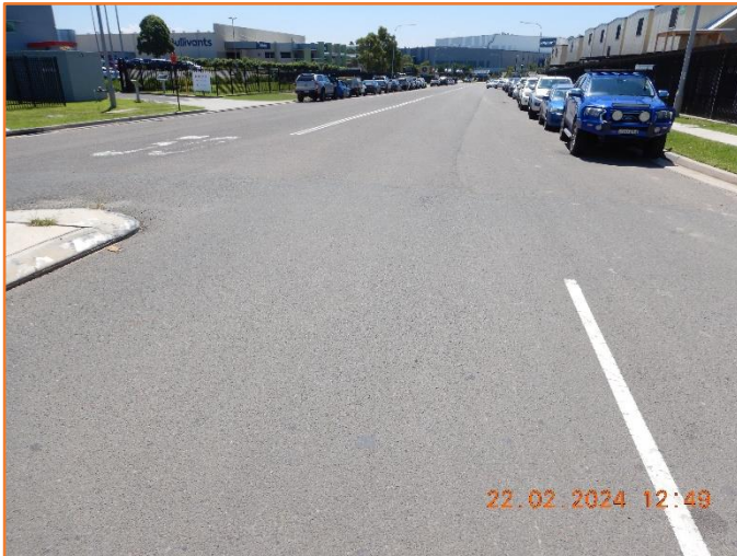
Figure 151: Reasonable - General condition of flexible pavement.
