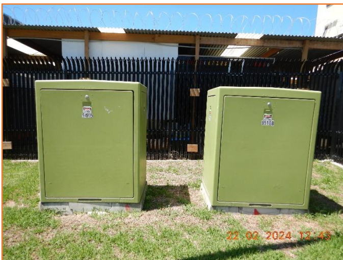
Figure 78: Good - General condition of substations.
