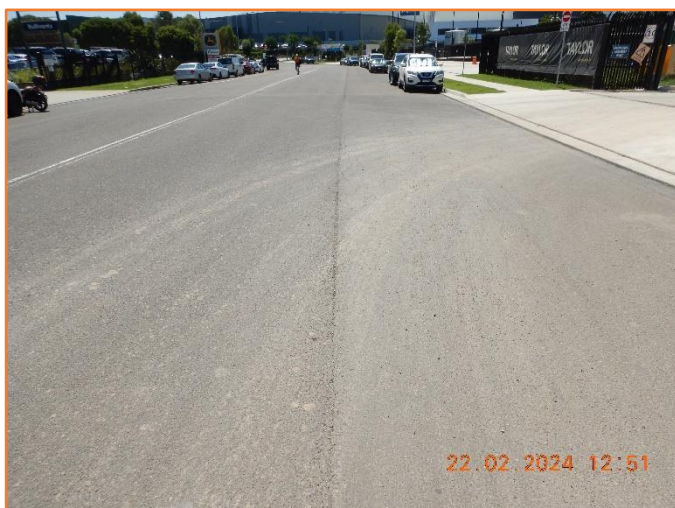
Figure 174: Reasonable - General condition of flexible pavement.
