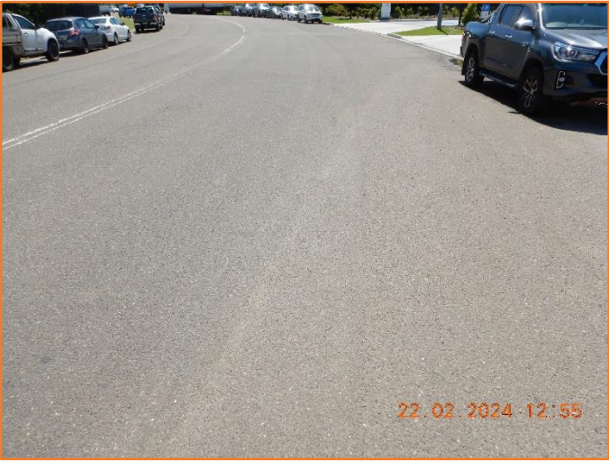
Figure 209: Reasonable - General condition of flexible pavement.
