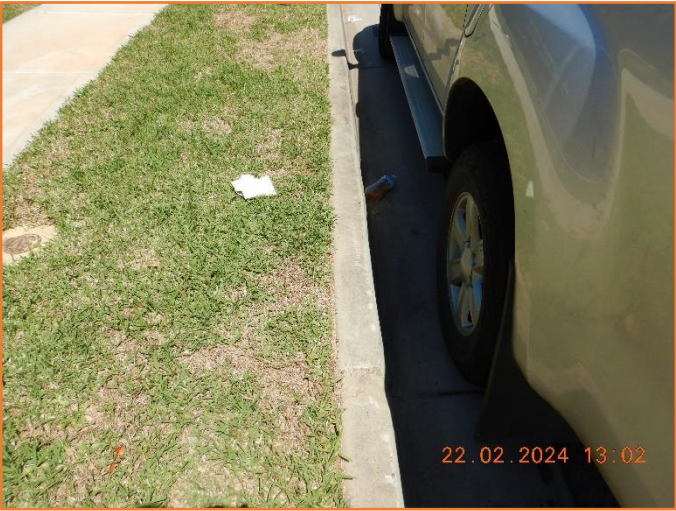
Figure 300: Reasonable - General condition of kerb and gutter.
