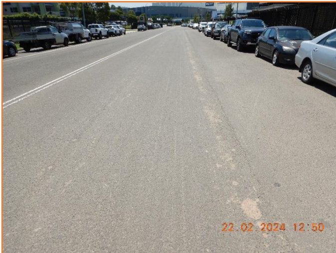
Figure 163: Reasonable - General condition of flexible pavement.
