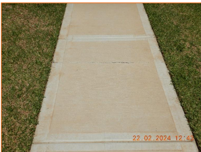
Figure 87: Reasonable - General condition of footpath. Moderate cracking observed.
