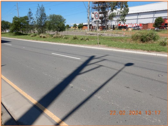
Figure 444: Reasonable - General condition of flexible pavement.
