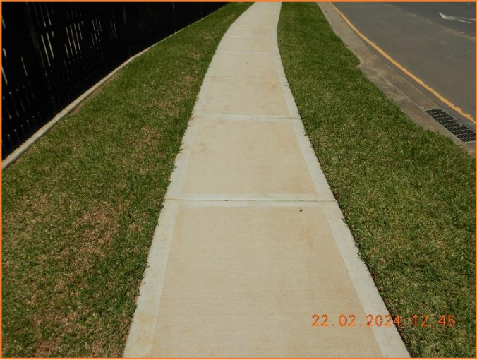
Figure 112: Good - General condition of footpath.
