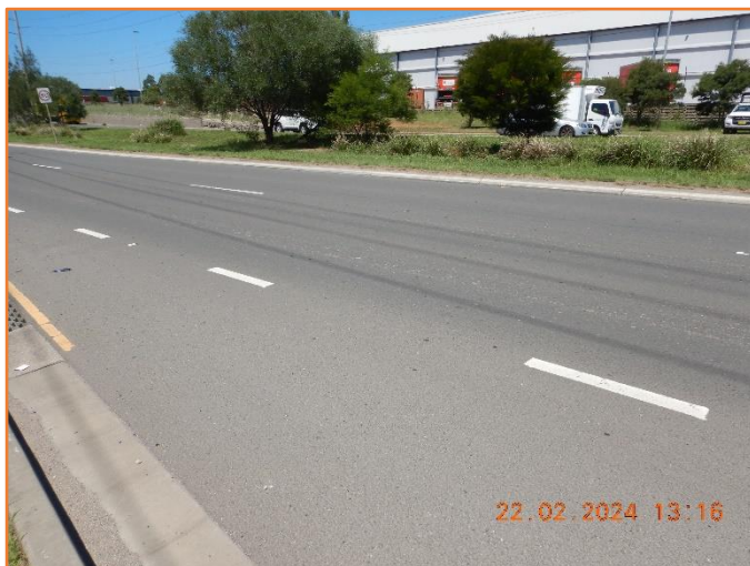
Figure 438: Reasonable - General condition of flexible pavement.
