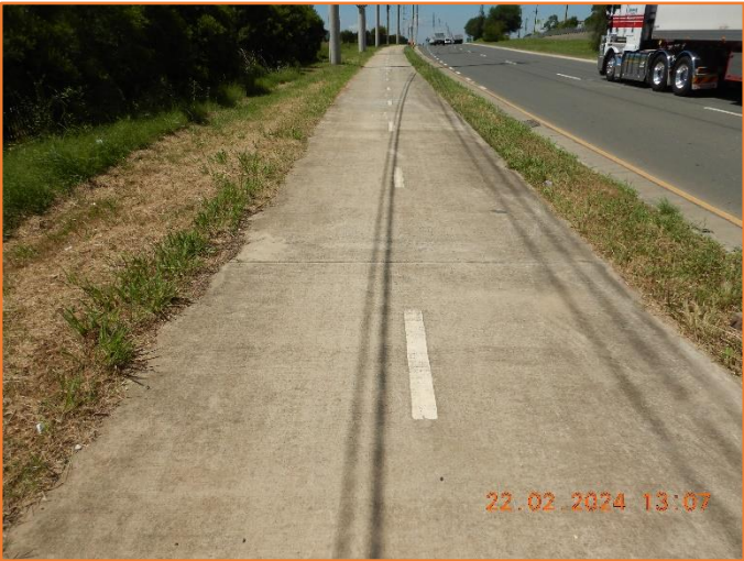
Figure 358: Reasonable - General condition of footpath.
