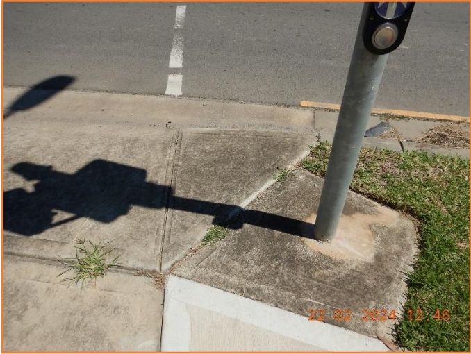
Figure 133: Reasonable - General condition of footpath.
