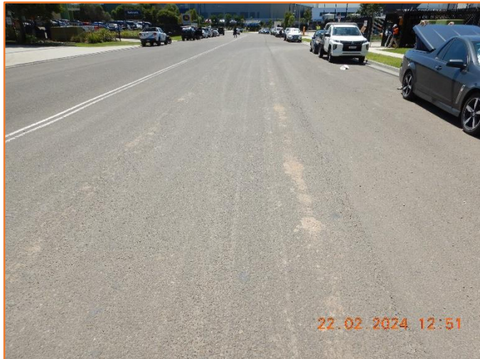
Figure 169: Reasonable - General condition of flexible pavement.
