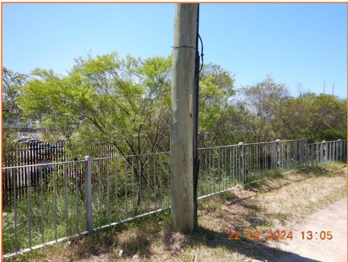
Figure 340: Reasonable - General condition of monopole assembly.
