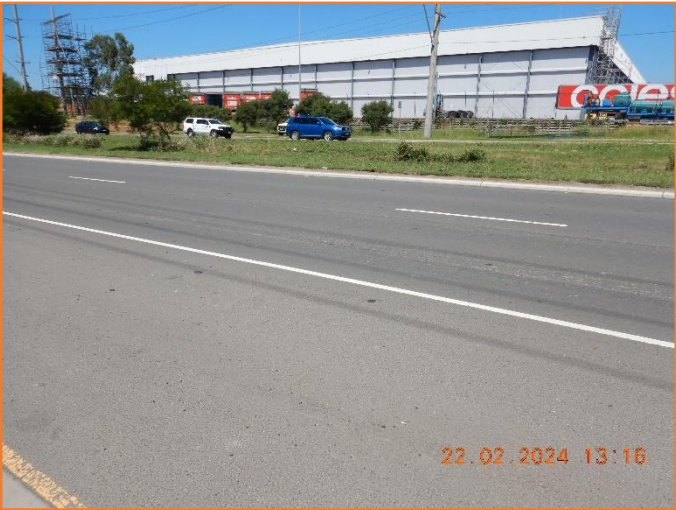
Figure 433: Reasonable - General condition of flexible pavement.
