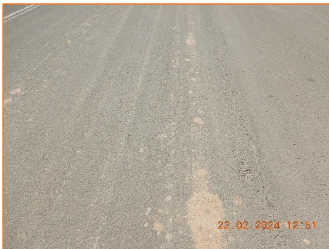
Figure 170: Reasonable - General condition of flexible pavement. Moderate alligator cracking observed.
