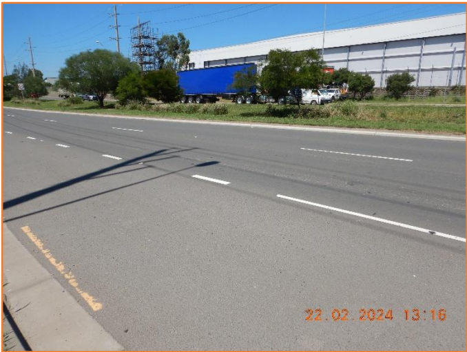
Figure 435: Reasonable - General condition of flexible pavement.
