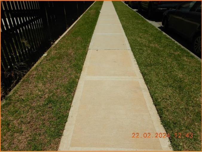
Figure 82: Good - General condition of footpath.
