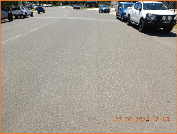
Figure 196: Reasonable - General condition of flexible pavement.
