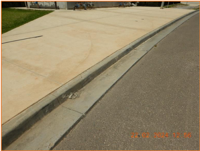
Figure 227: Reasonable - General condition of kerb and gutter.
