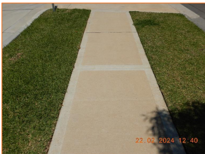
Figure 45: Good - General condition of footpath.
