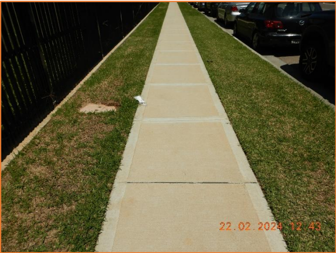
Figure 84: Good - General condition of footpath.
