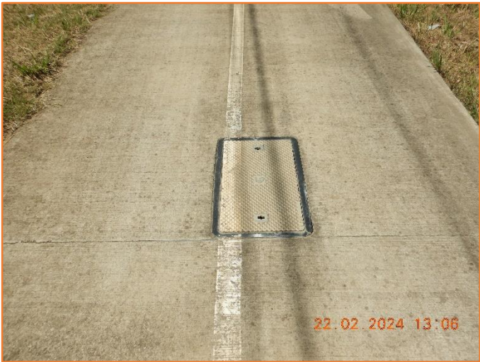
Figure 351: Reasonable - General condition of service pit.
