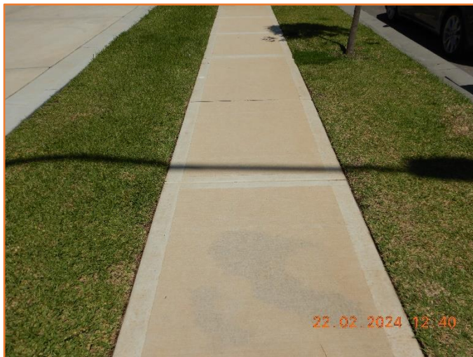
Figure 43: Good - General condition of footpath.
