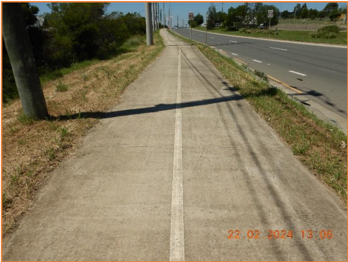
Figure 347: Reasonable - General condition of footpath.
