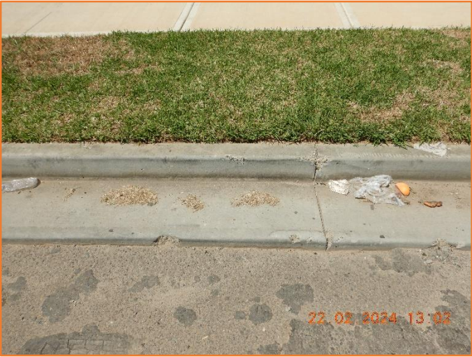
Figure 299: Reasonable - General condition of kerb and gutter. Moderate spalling observed.
