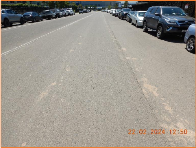
Figure 161: Reasonable - General condition of flexible pavement.
