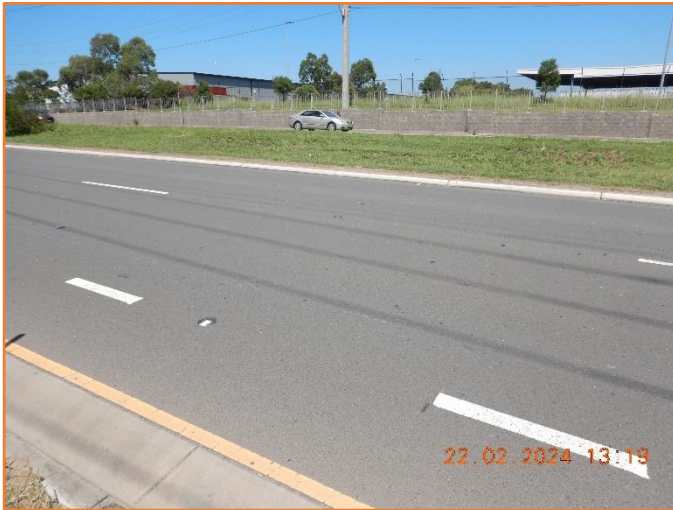
Figure 458: Reasonable - General condition of flexible pavement.
