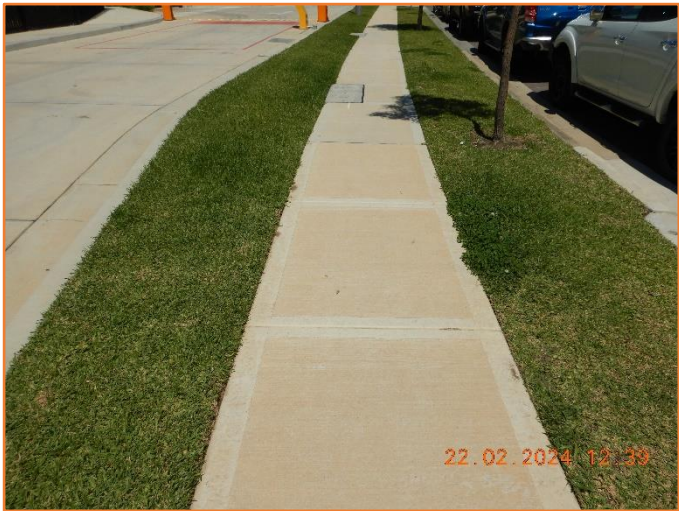
Figure 32: Good - General condition of footpath.
