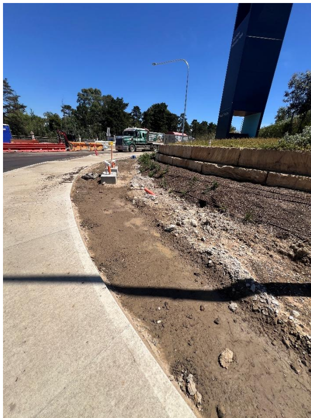
Figure 22 – General condition of the footpath.
