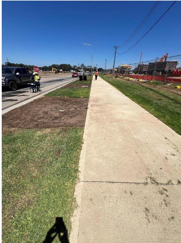
Figure 87 – General condition of the footpath.
