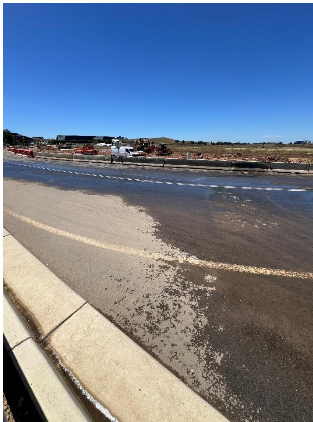
Figure 132 – General condition of the road.
