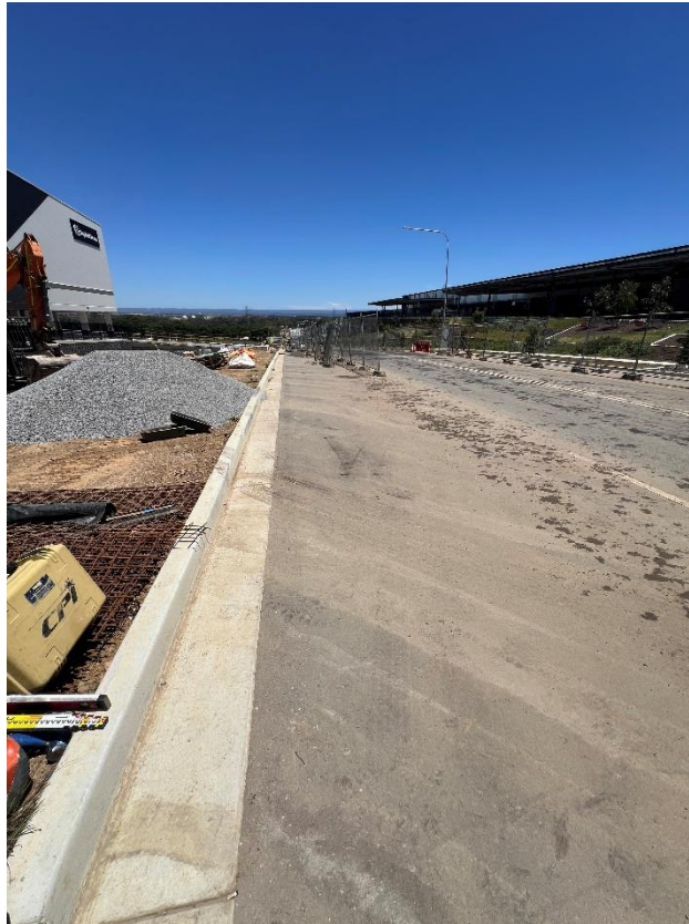
Figure 269 – General condition of the road.
