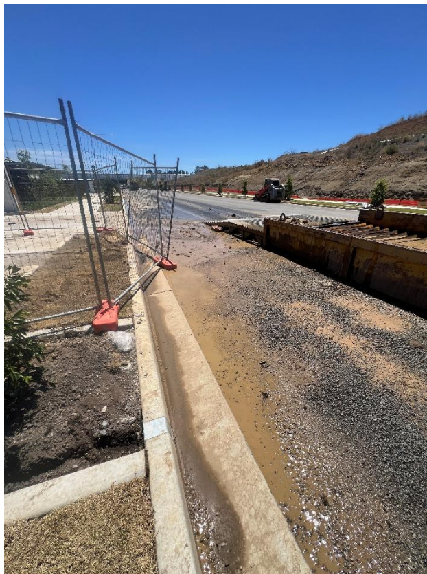
Figure 216 – General condition of the road.
