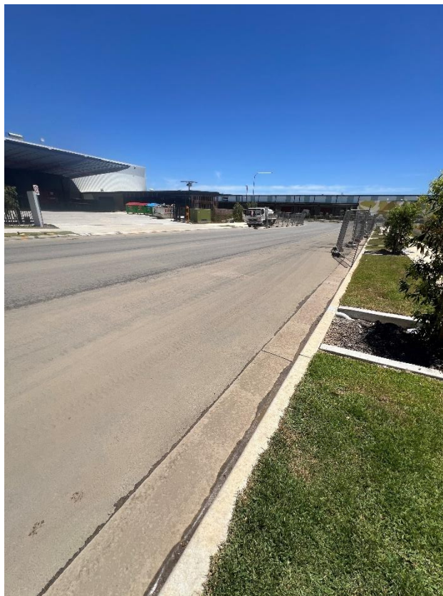
Figure 190 – General condition of the road.
