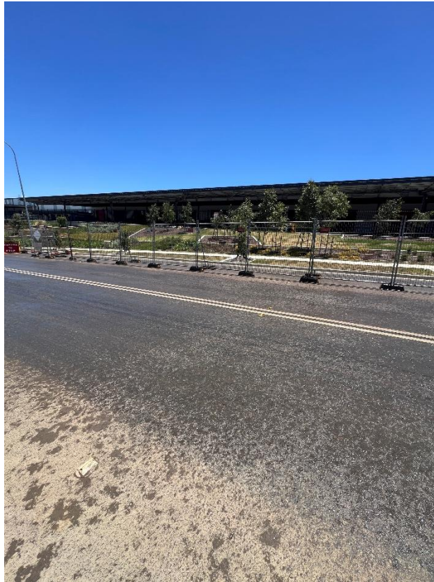
Figure 273 – General condition of the road.
