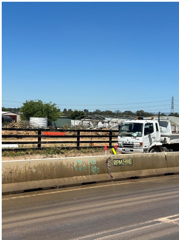
Figure 52 – General condition of the road.
