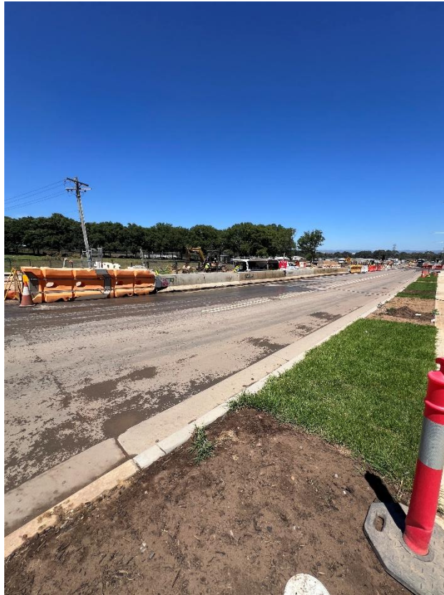
Figure 1 – General condition of the road.
