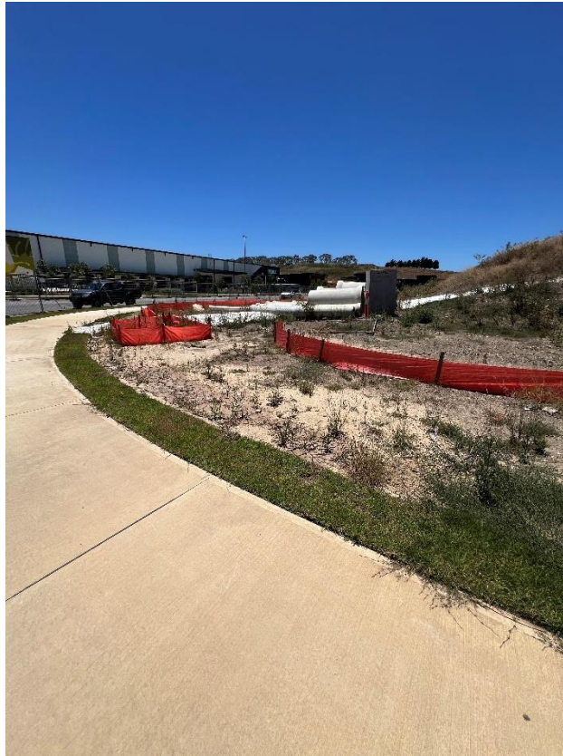
Figure 179 – General condition of the footpath.
