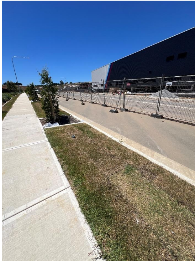
Figure 157 – General condition of the footpath.
