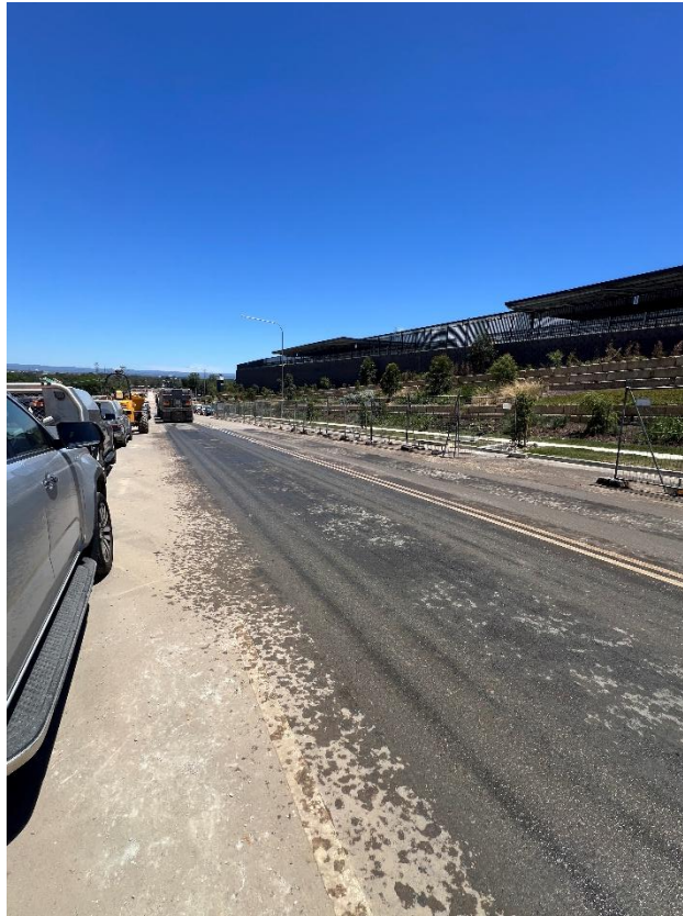
Figure 277 – General condition of the road.
