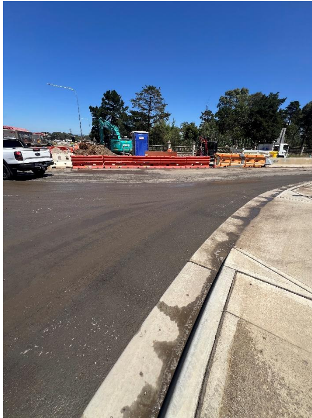
Figure 25 – General condition of the road.
