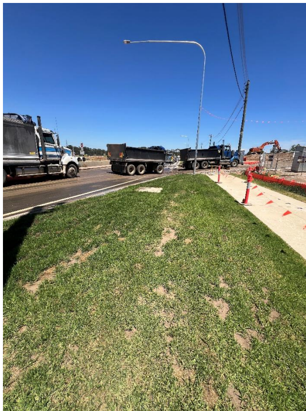
Figure 72 – General condition of the ground area.
