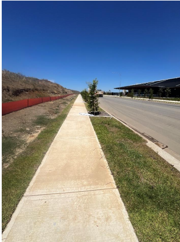
Figure 191 – General condition of the footpath.
