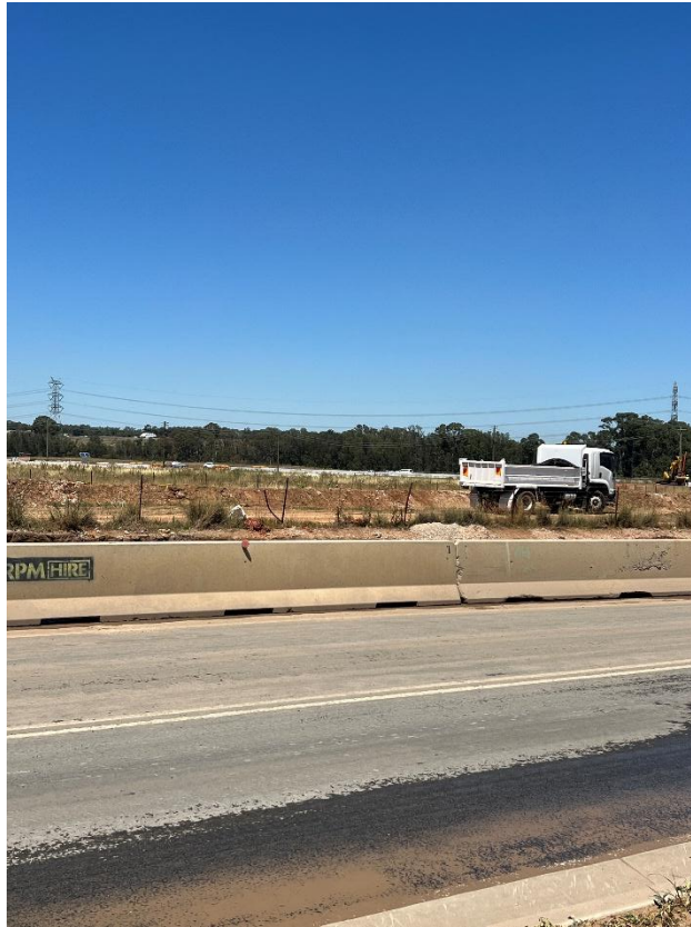
Figure 101 – General condition of the road.
