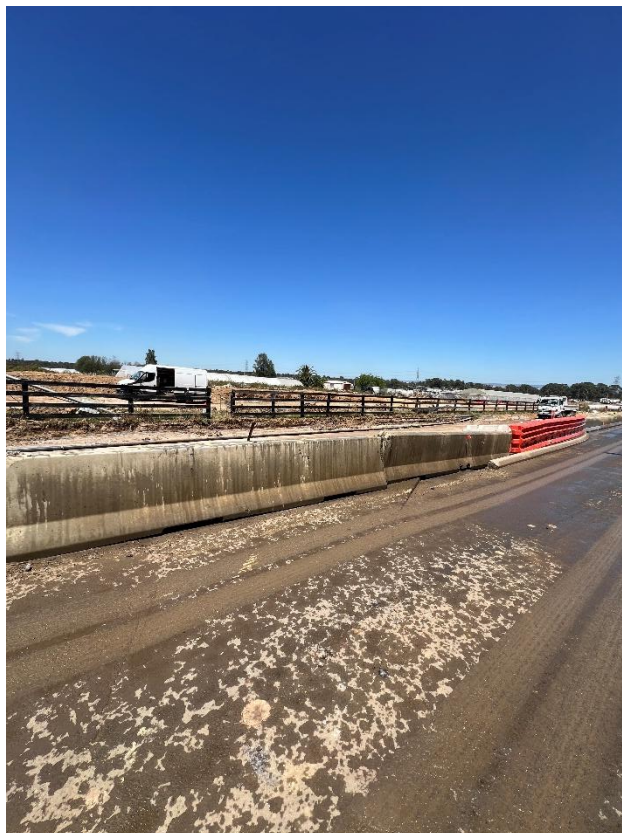
Figure 44 – General condition of the road.
