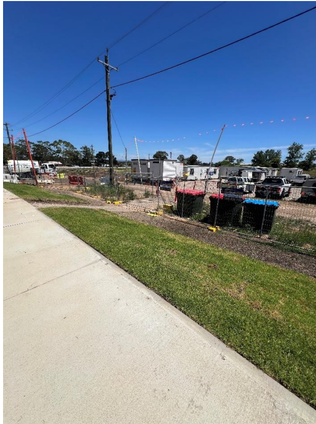
Figure 127 – General condition of the fence.
