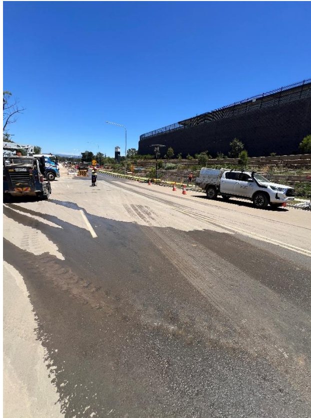
Figure 287 – General condition of the road.
