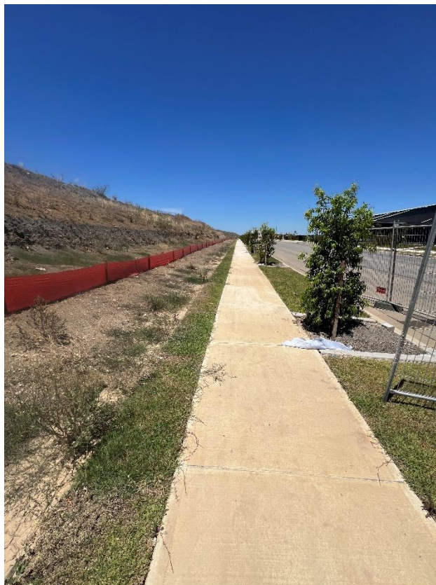
Figure 186 – General condition of the footpath.
