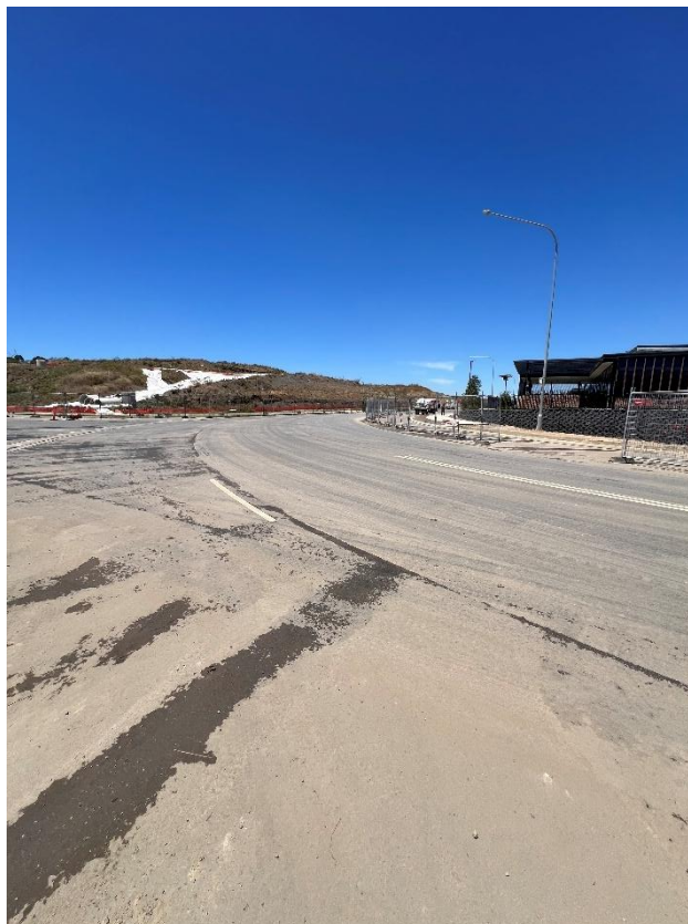
Figure 170 – General condition of the road.
