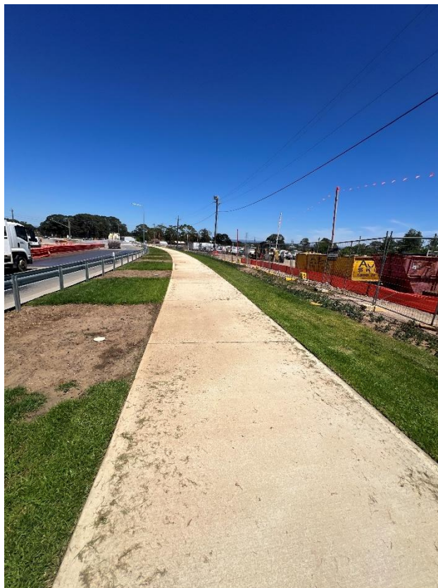
Figure 112 – General condition of the footpath.
