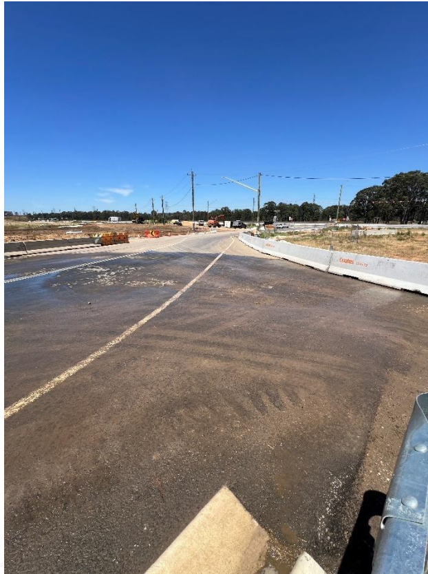
Figure 131 – General condition of the road.
