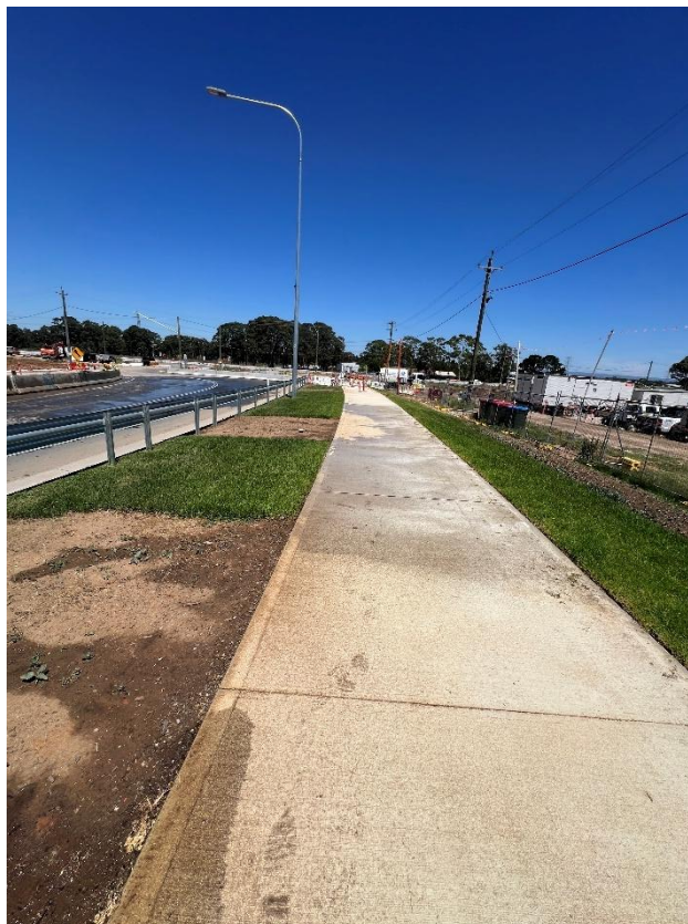
Figure 118 – General condition of the footpath.
