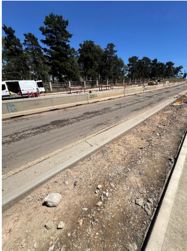
Figure 35 – General condition of the road.
