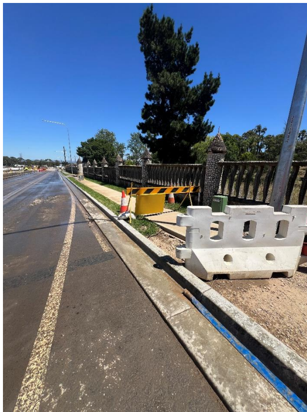
Figure 46 – General condition of the road.
