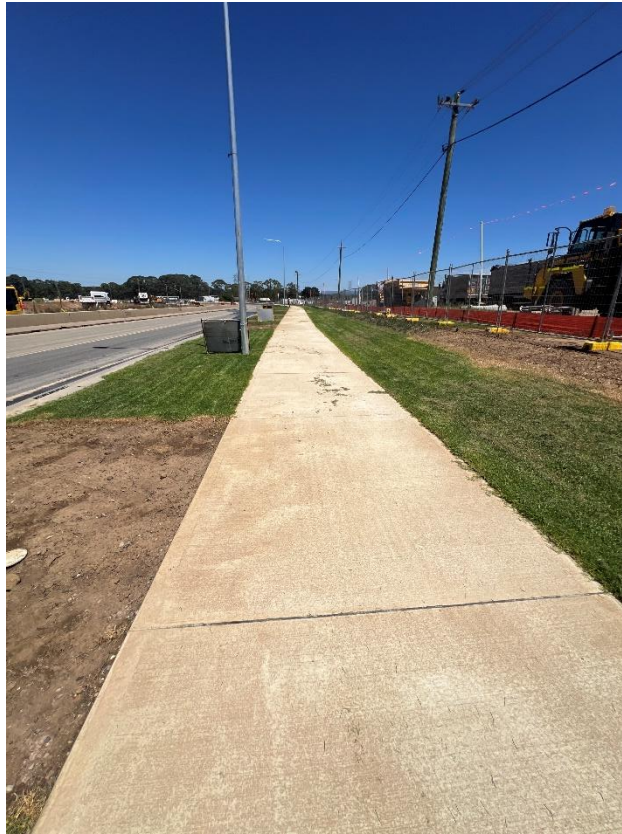
Figure 93 – General condition of the footpath.
