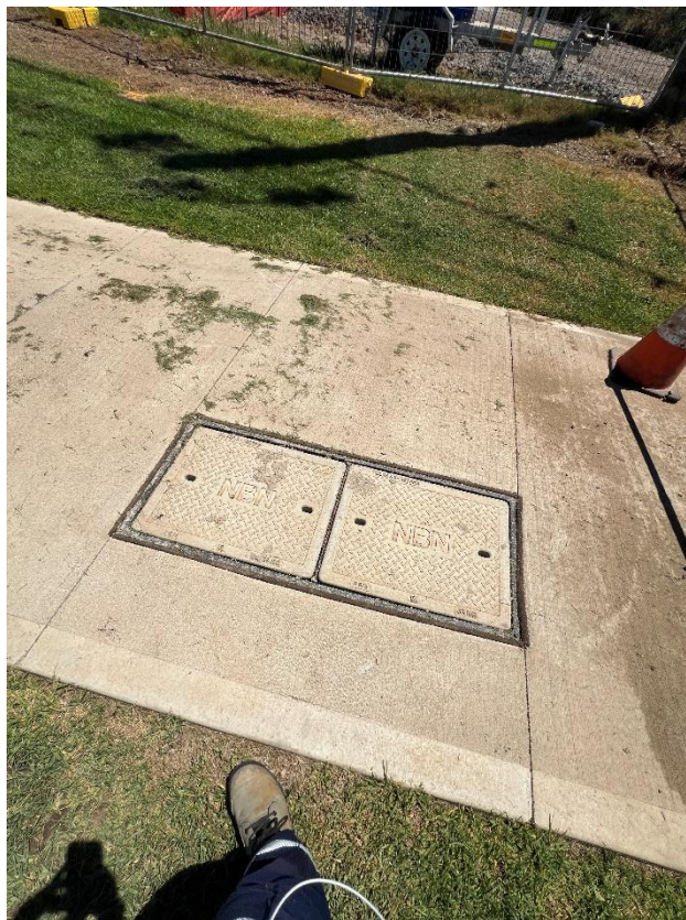
Figure 88 – General condition of the utility lid.
