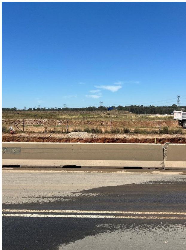
Figure 106 – General condition of the road.
