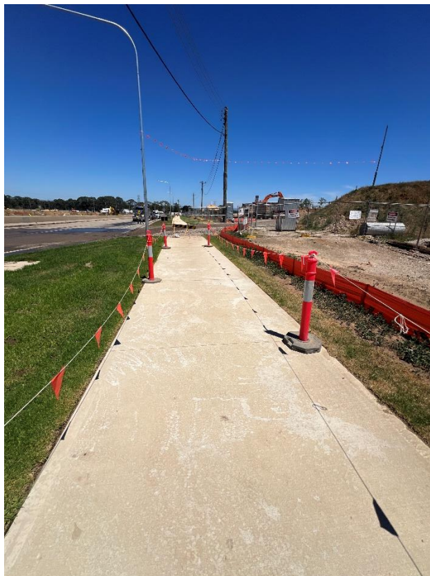
Figure 78 – General condition of the footpath.
