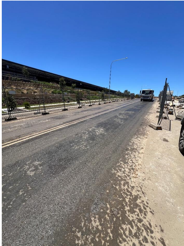
Figure 279 – General condition of the road.
