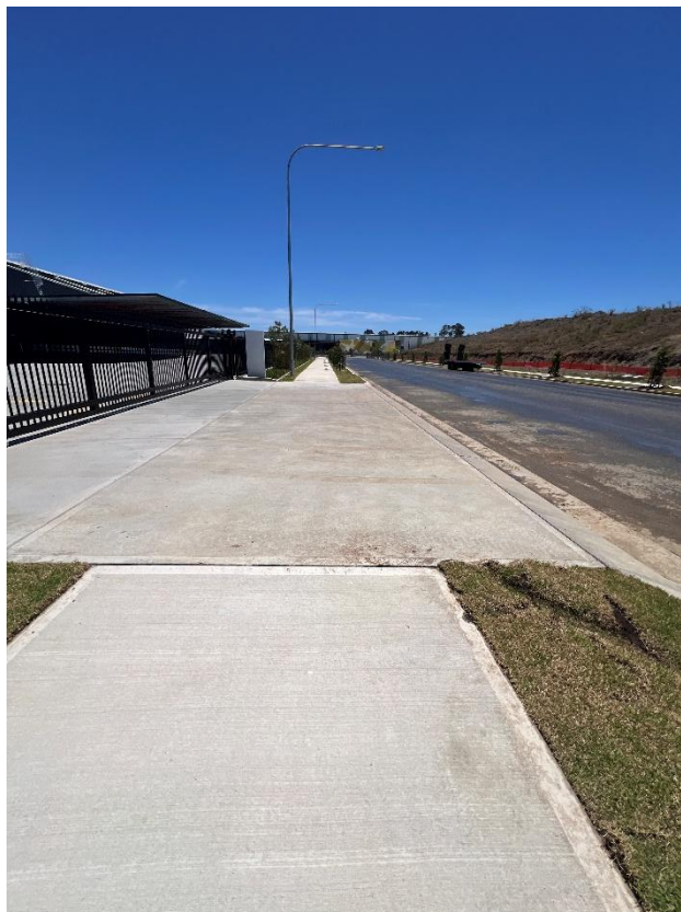
Figure 224 – General condition of the driveway.
