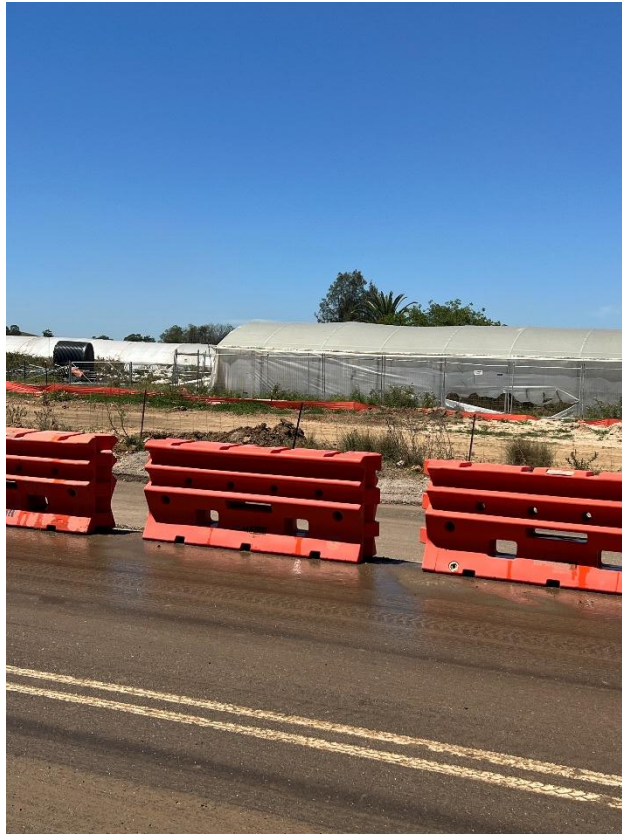
Figure 77 – General condition of the road.
