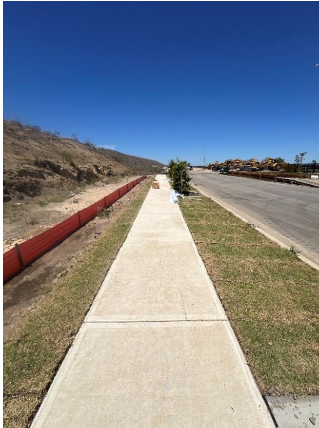
Figure 207 – General condition of the footpath.
