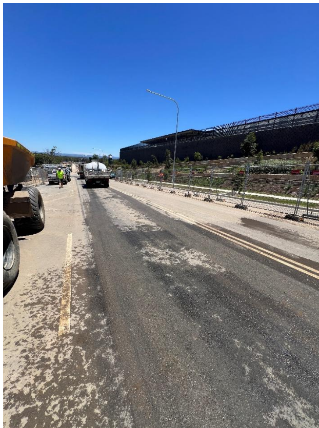
Figure 280 – General condition of the road.
