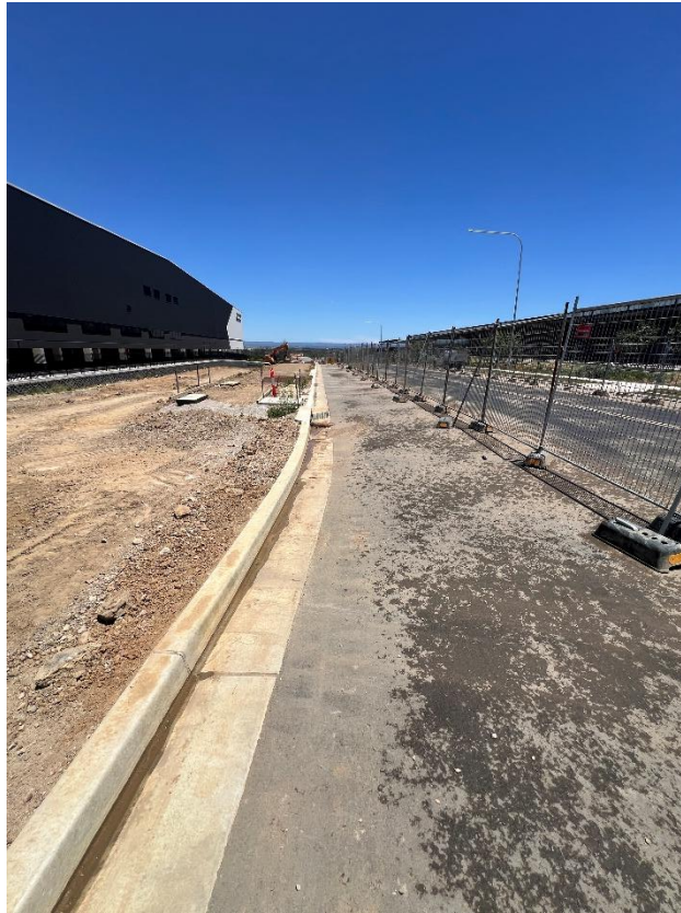
Figure 259 – General condition of the road.
