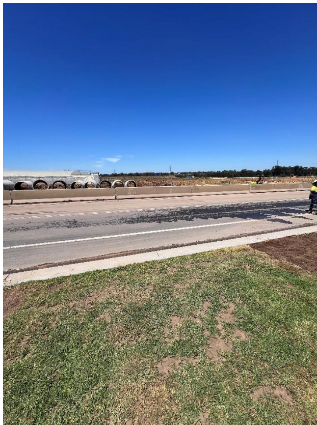
Figure 84 – General condition of the road.
