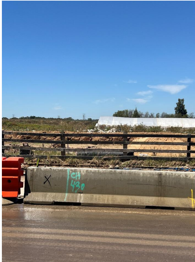
Figure 51 – General condition of the road.
