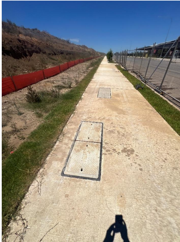
Figure 181 – General condition of the footpath.
