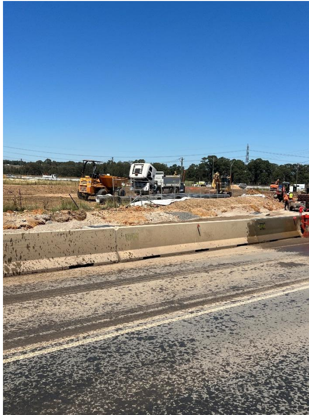
Figure 117 – General condition of the road.
