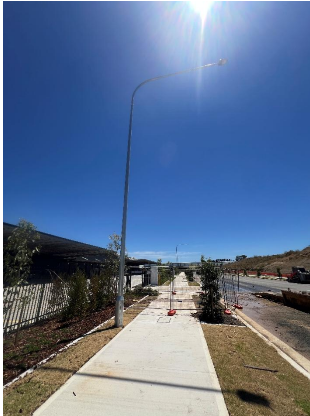
Figure 215 – General condition of the electrical light post.
