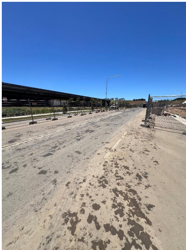
Figure 272 – General condition of the road.
