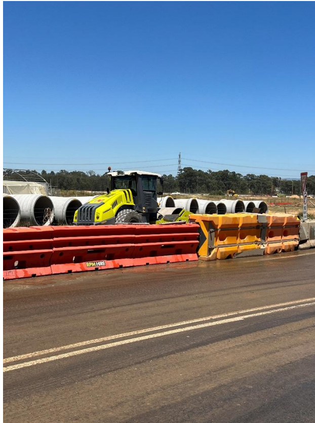
Figure 75 – General condition of the road.
