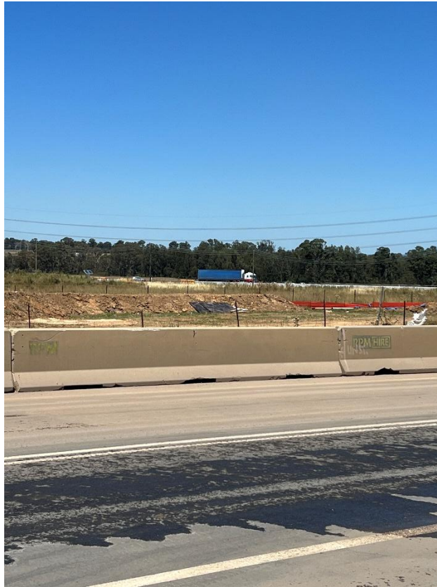
Figure 85 – General condition of the road.
