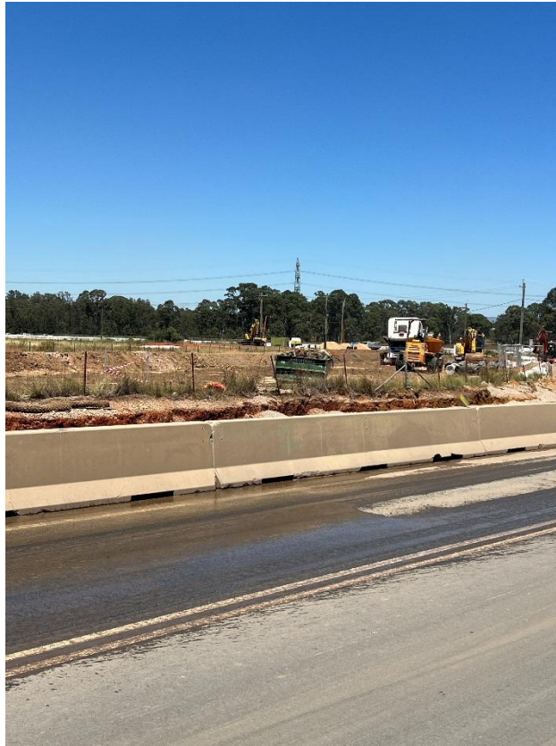
Figure 107 – General condition of the road.
