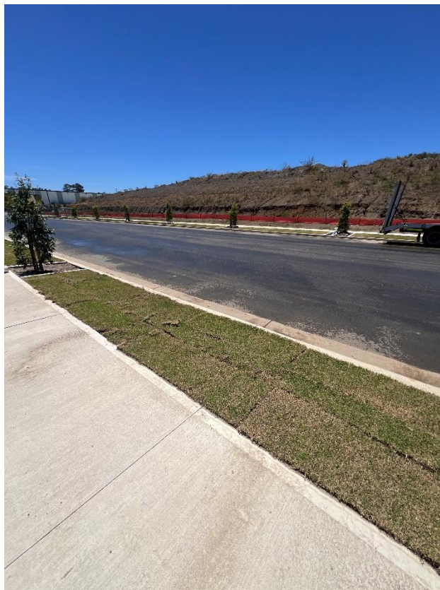
Figure 232 – General condition of the road.
