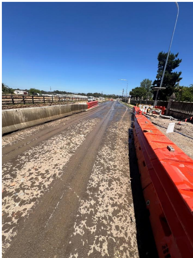
Figure 42 – General condition of the road.
