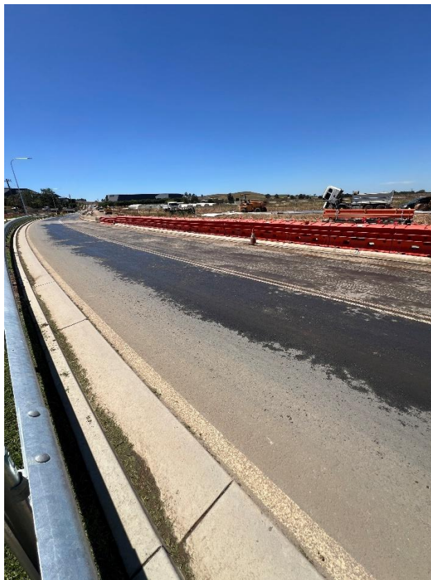
Figure 122 – General condition of the road.
