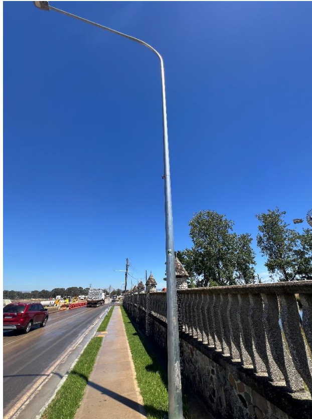
Figure 59 – General condition of the electrical light post.
