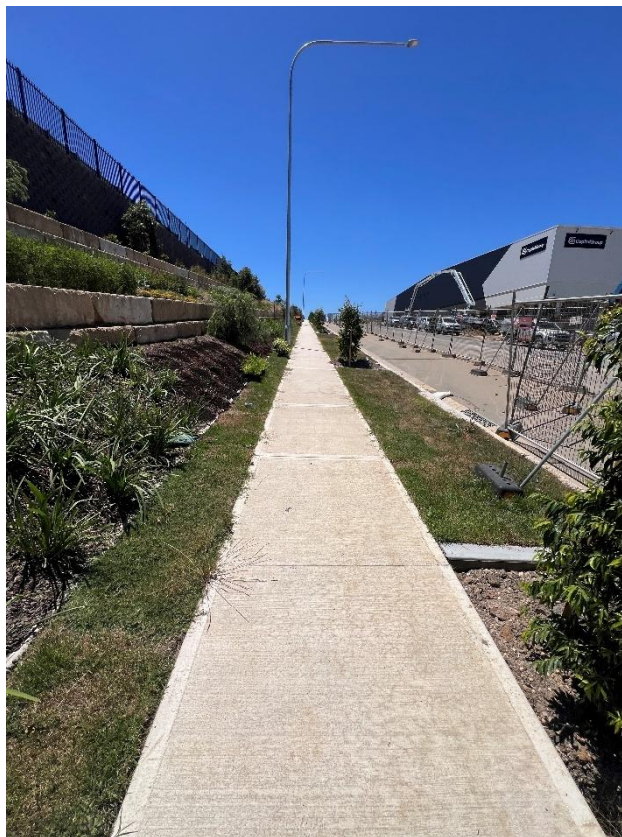
Figure 140 – General condition of the footpath.
