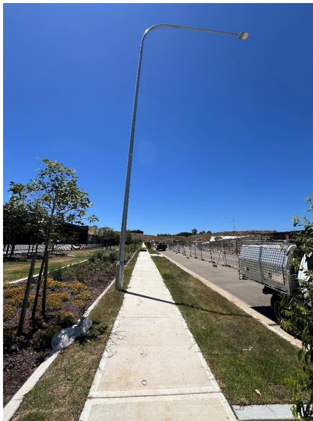
Figure 162 – General condition of the electrical light post.
