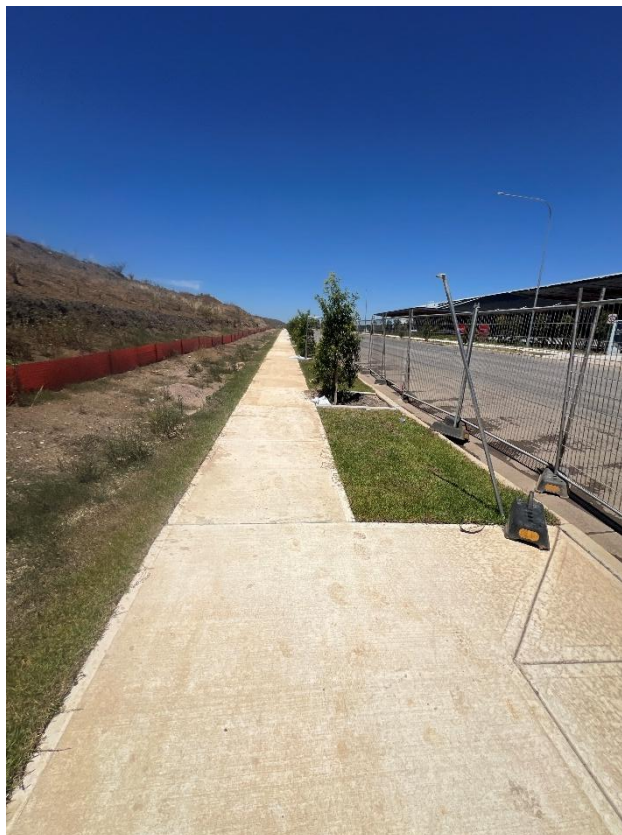
Figure 184 – General condition of the footpath.
