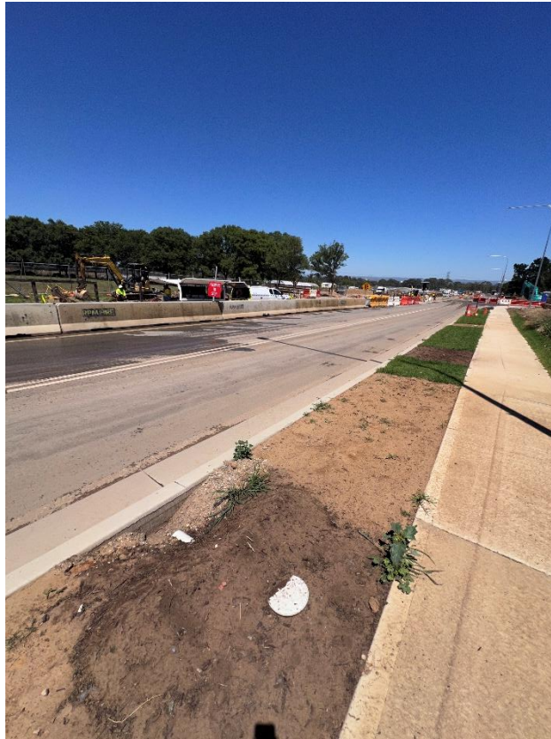
Figure 5 – General condition of the road.
