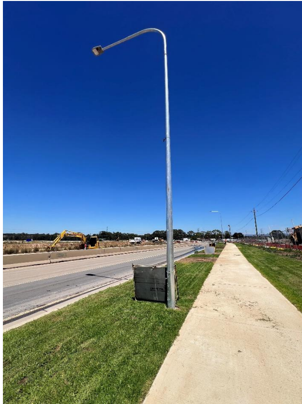
Figure 95 – General condition of the electrical light post.
