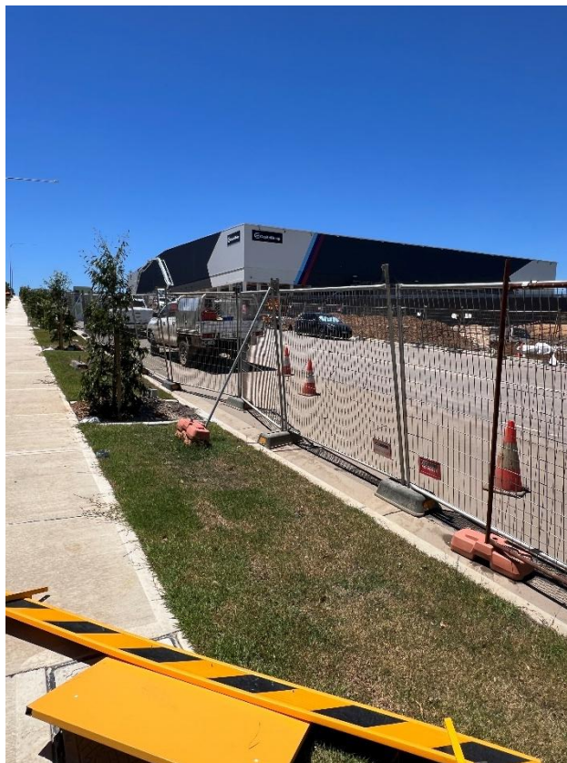
Figure 136 – General condition of the fence.
