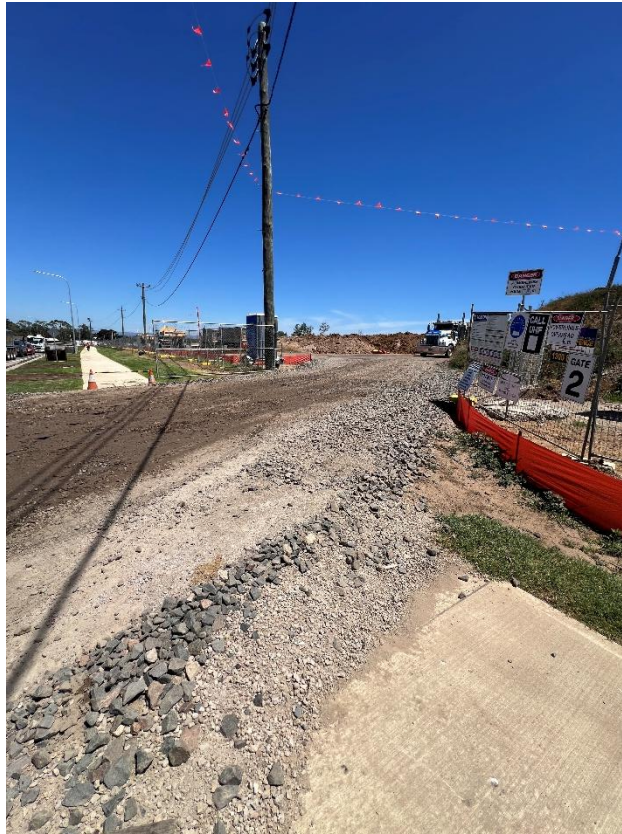
Figure 83 – General condition of the driveway.
