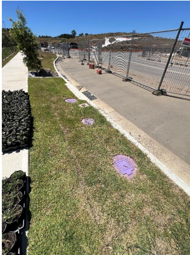
Figure 167 – General condition of the utility lid.
