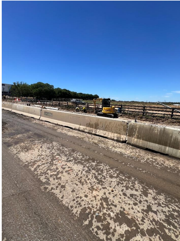
Figure 43 – General condition of the road.
