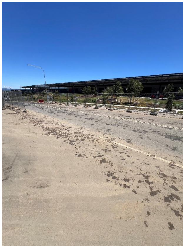
Figure 270 – General condition of the road.
