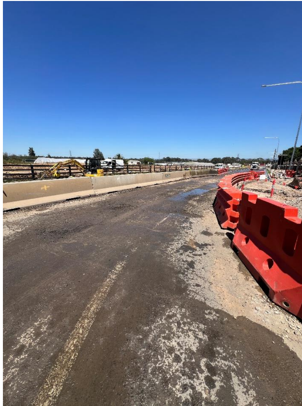
Figure 39 – General condition of the road.
