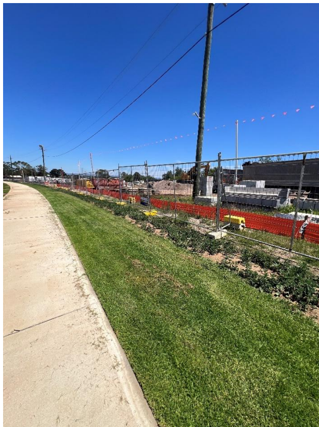
Figure 110 – General condition of the fence.
