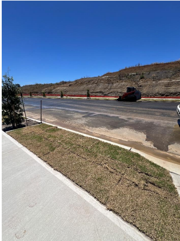
Figure 219 – General condition of the road.
