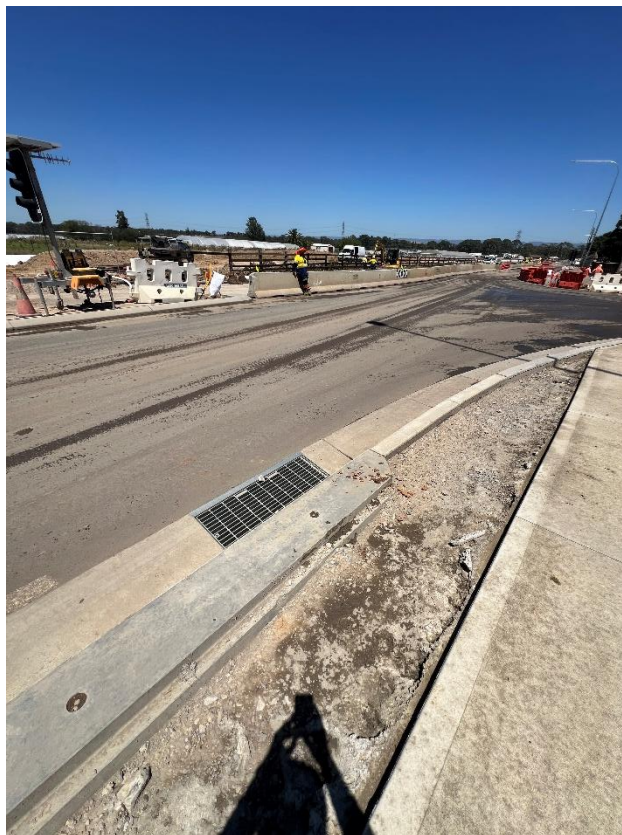
Figure 20 – General condition of the road.
