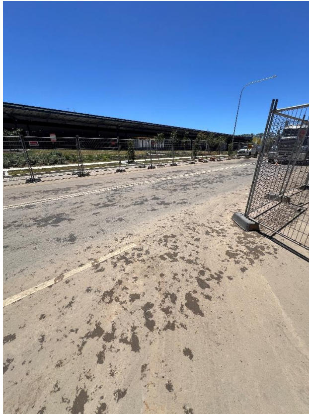
Figure 271 – General condition of the road.
