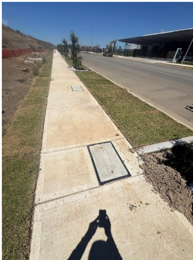
Figure 196 – General condition of the utility lid.
