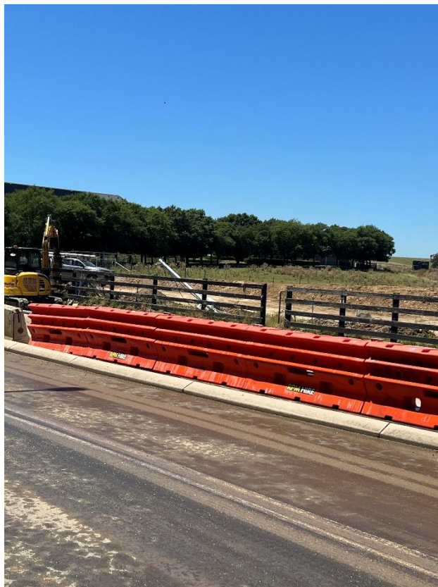
Figure 50 – General condition of the road.
