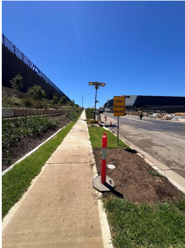
Figure 3 – General condition of the footpath.
