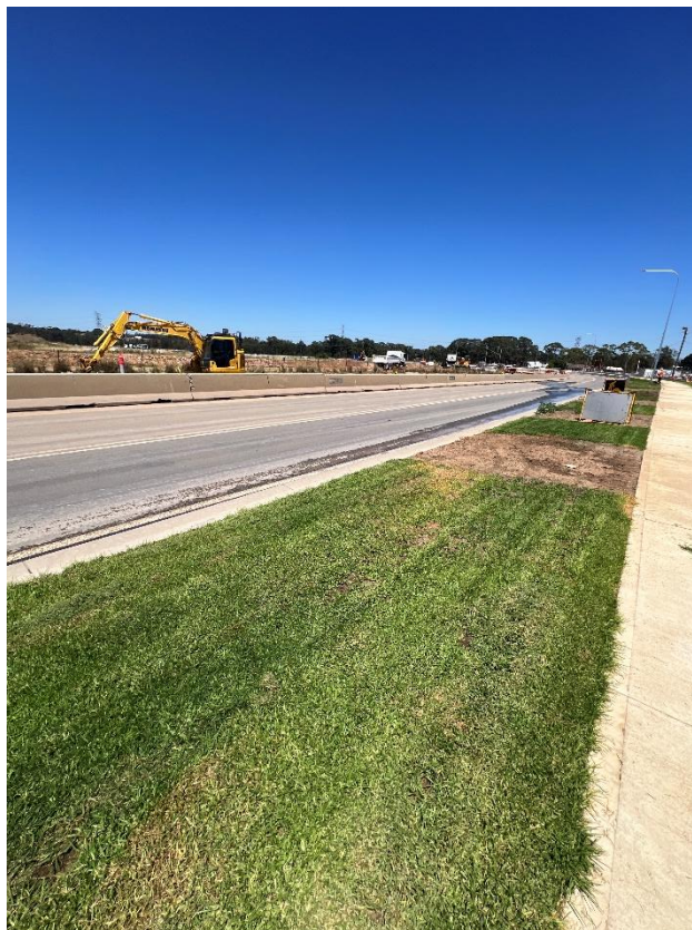
Figure 96 – General condition of the ground area.
