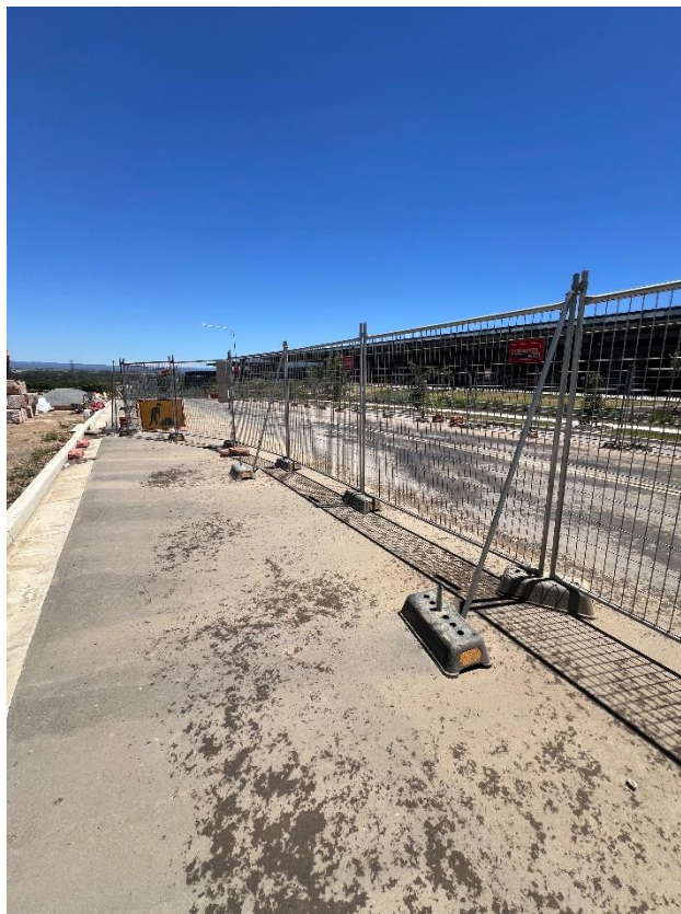
Figure 266 – General condition of the road.
