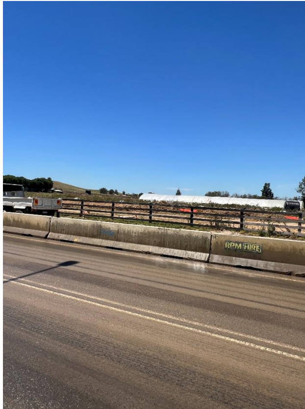
Figure 63 – General condition of the road.
