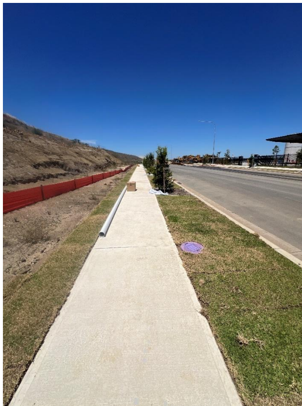
Figure 202 – General condition of the footpath.
