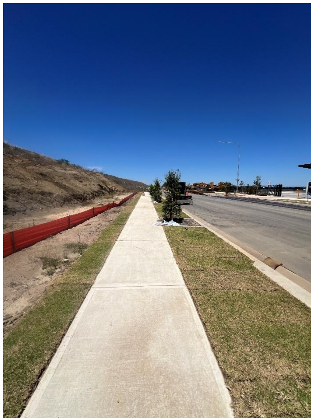
Figure 204 – General condition of the footpath.
