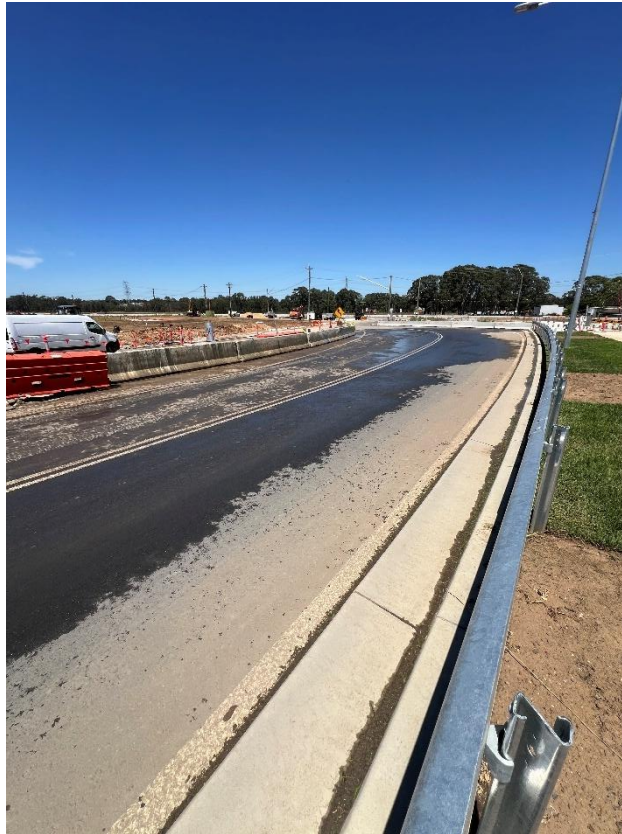
Figure 121 – General condition of the road.
