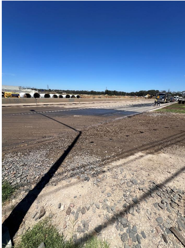
Figure 81 – General condition of the road.
