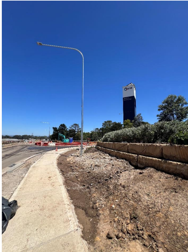
Figure 17 – General condition of the electrical light post.
