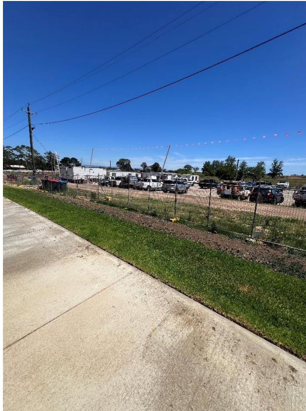
Figure 119 – General condition of the fence.
