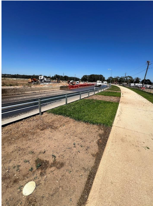
Figure 113 – General condition of the ground area.
