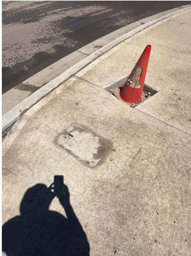
Figure 23 – General condition of the utility lid.
