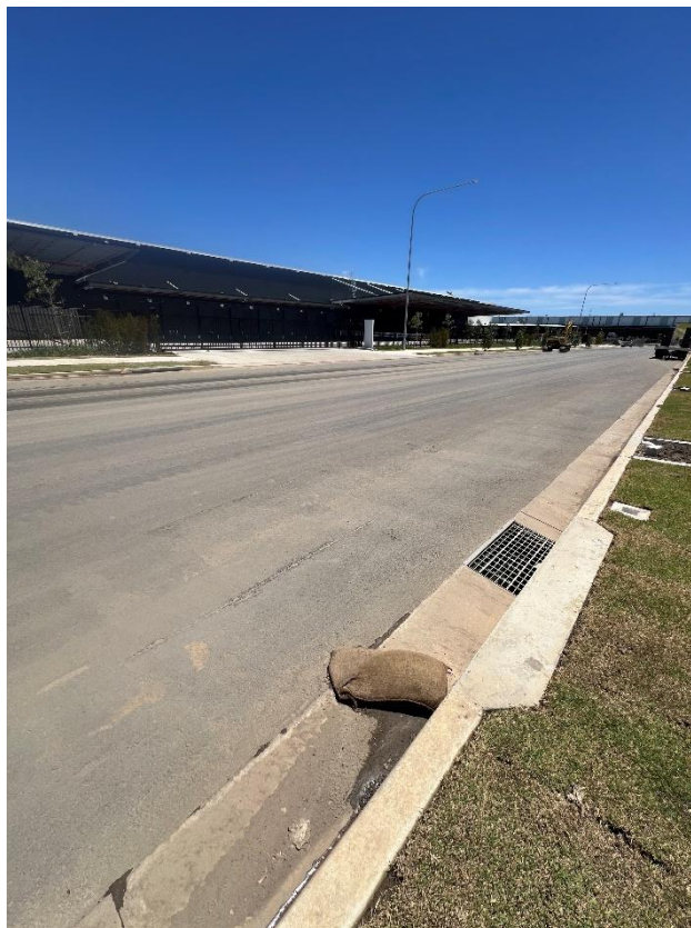
Figure 206 – General condition of the road.
