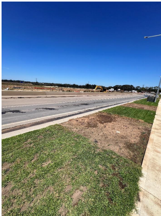
Figure 92 – General condition of the ground area.
