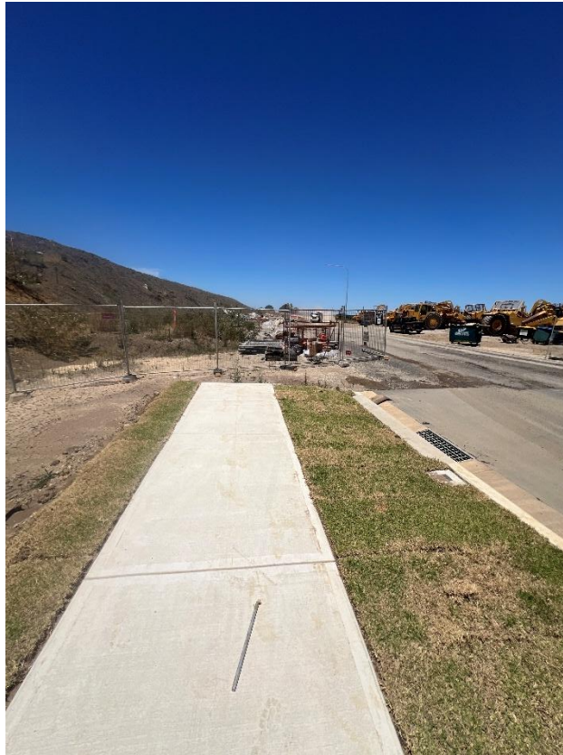
Figure 211 – General condition of the footpath.
