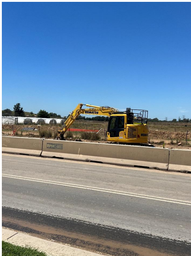
Figure 100 – General condition of the road.
