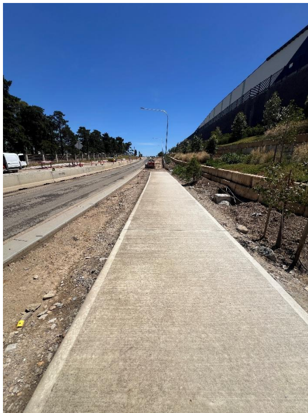
Figure 32 – General condition of the footpath.
