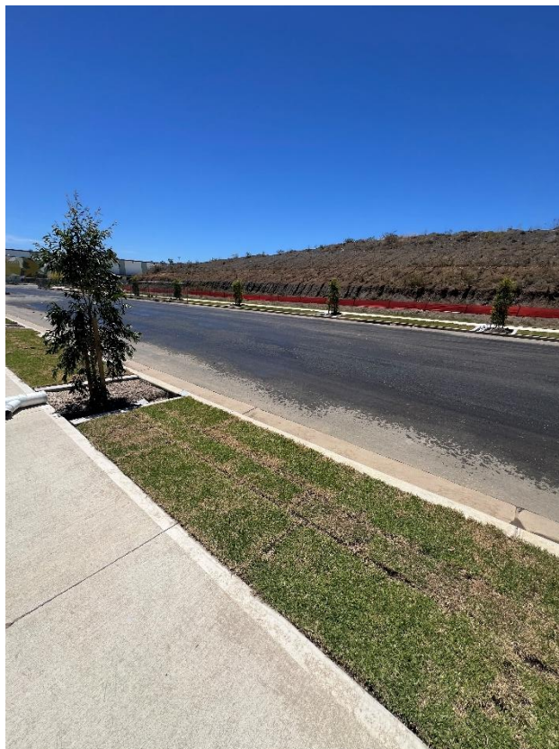
Figure 236 – General condition of the road.
