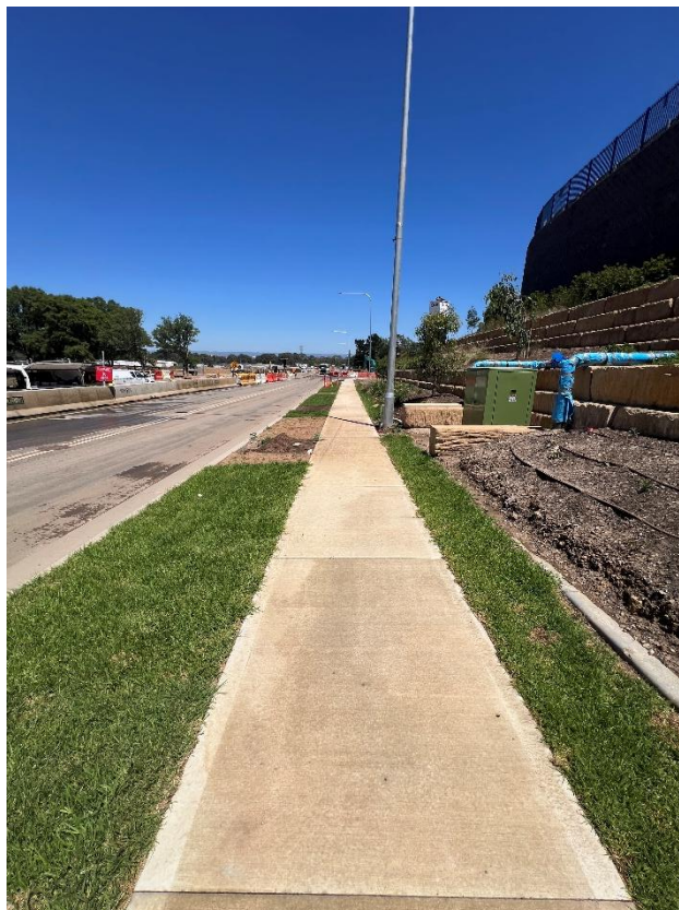
Figure 2 – General condition of the footpath.
