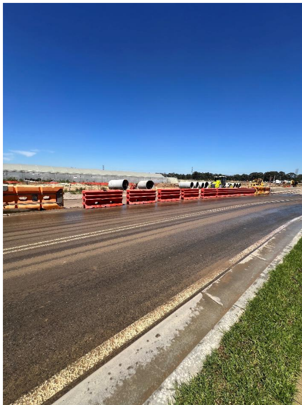
Figure 68 – General condition of the road.
