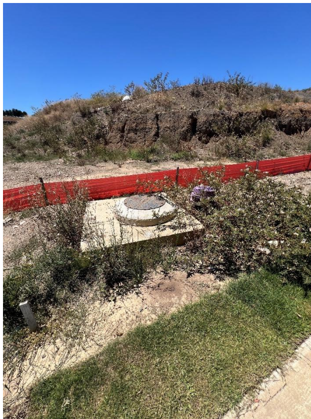
Figure 180 – General condition of the utility lid.
