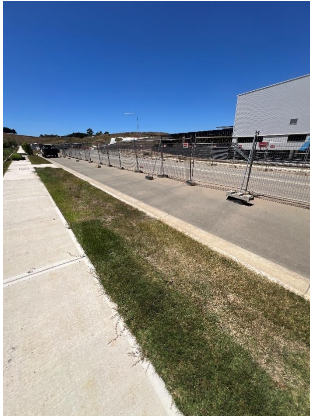
Figure 163 – General condition of the footpath.
