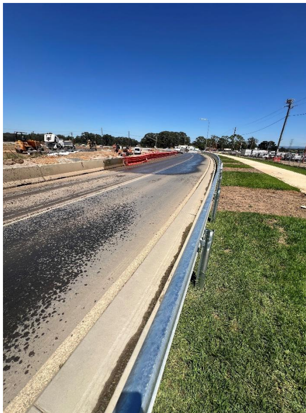
Figure 114 – General condition of the road.
