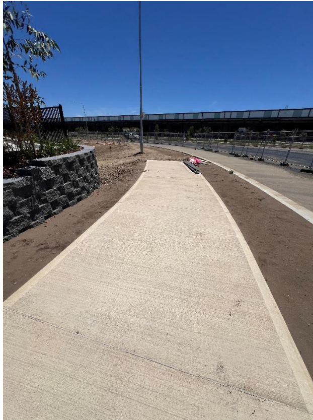
Figure 251 – General condition of the footpath.
