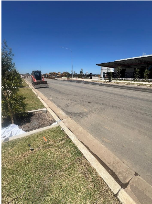
Figure 205 – General condition of the road.
