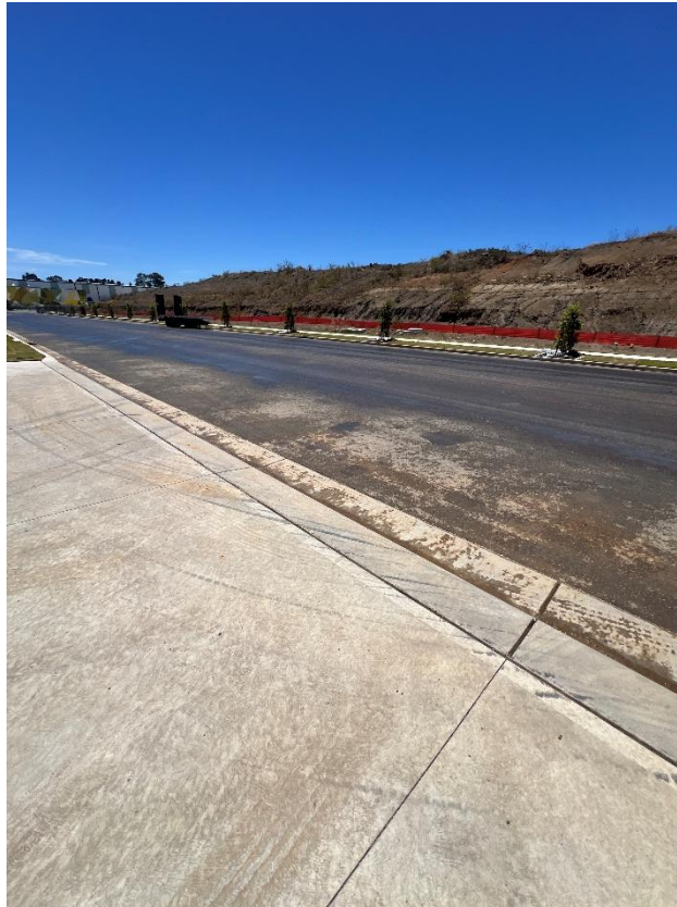
Figure 225 – General condition of the driveway.
