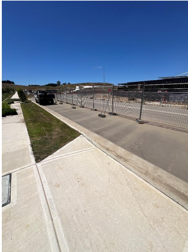
Figure 165 – General condition of the footpath.
