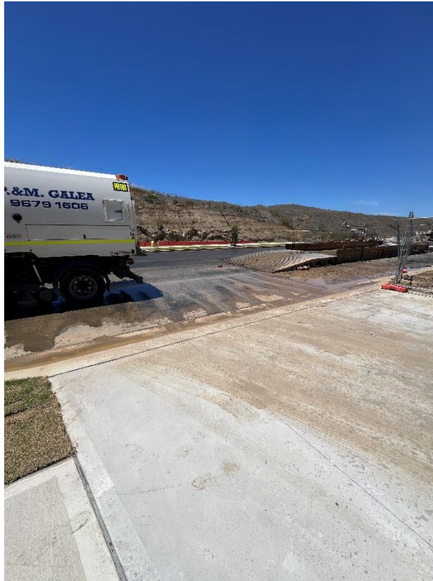
Figure 217 – General condition of the driveway.
