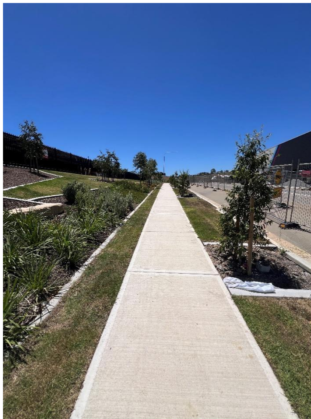
Figure 154 – General condition of the footpath.
