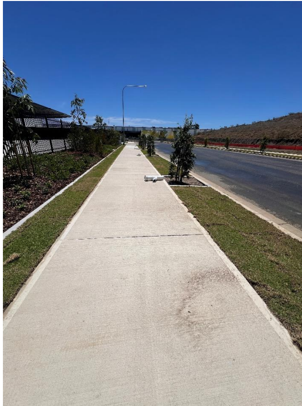
Figure 233 – General condition of the footpath.
