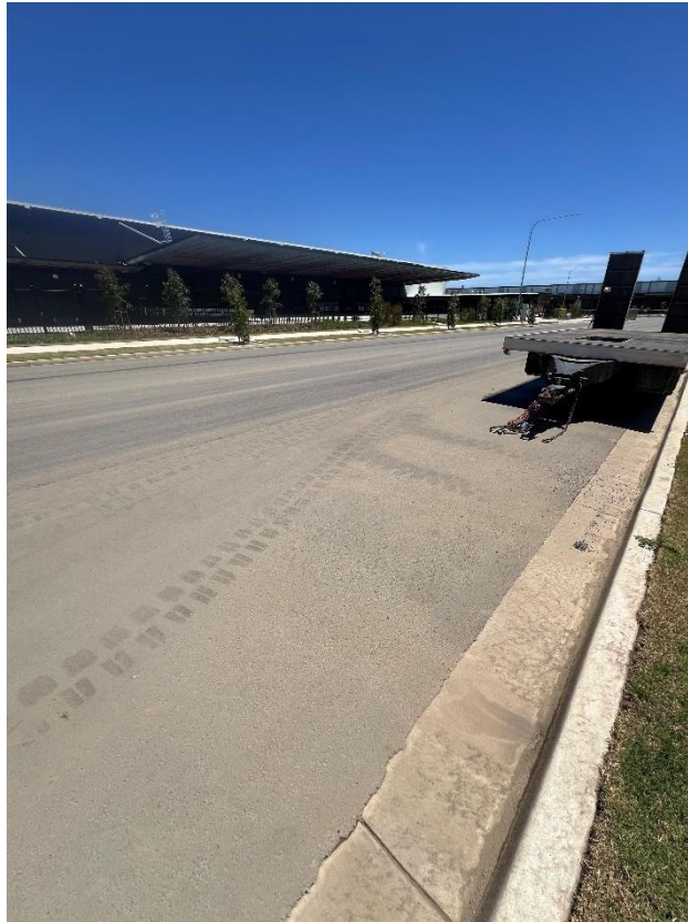
Figure 199 – General condition of the road.
