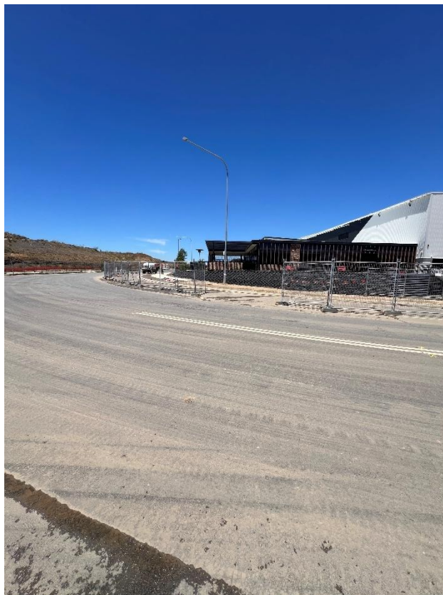
Figure 172 – General condition of the road.
