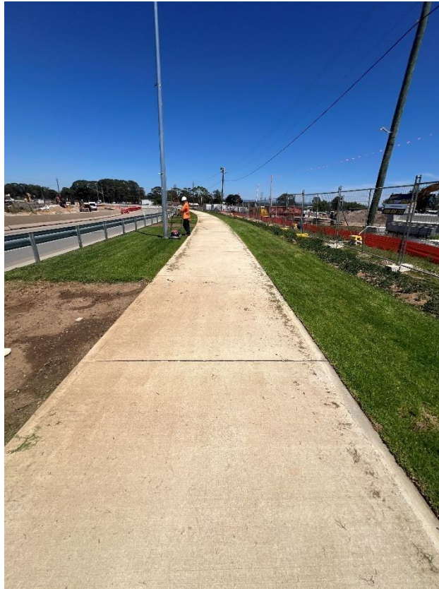
Figure 109 – General condition of the footpath.
