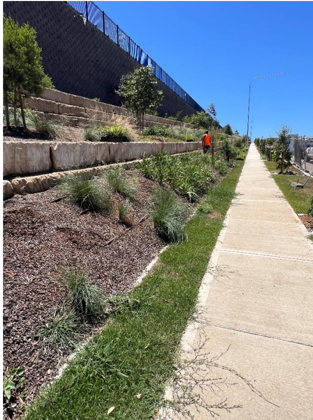
Figure 137 – General condition of the footpath.
