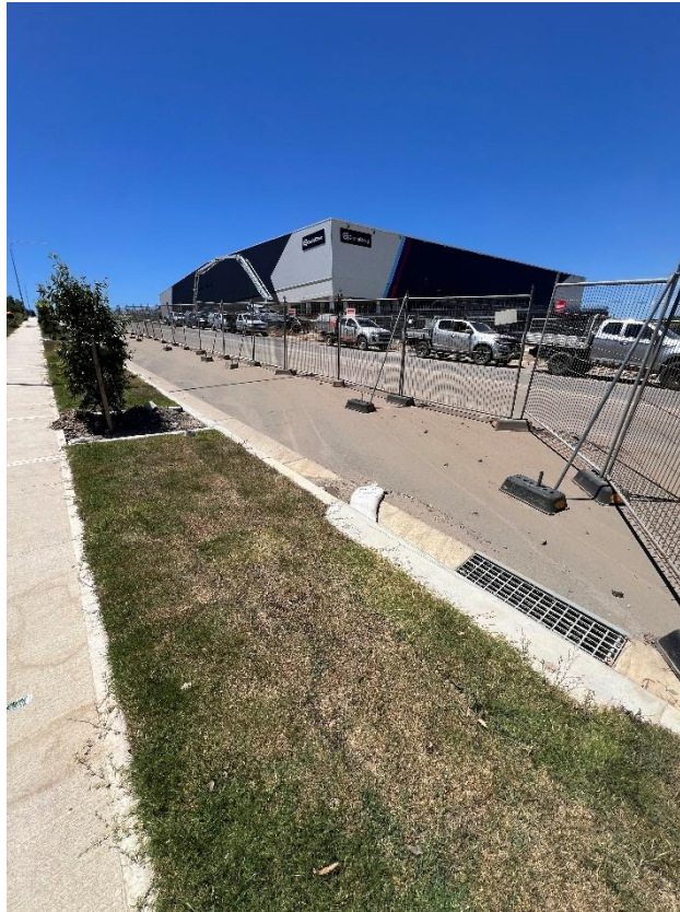
Figure 141 – General condition of the fence.
