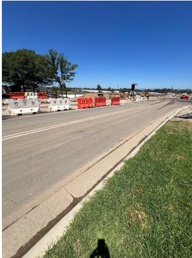
Figure 15 – General condition of the road.
