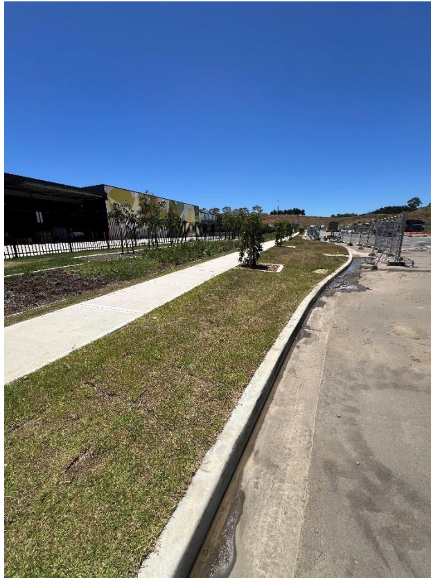
Figure 169 – General condition of the footpath.
