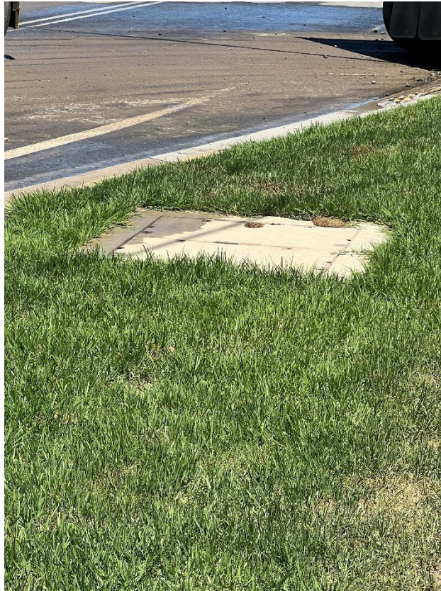
Figure 73 – General condition of the utility lid.
