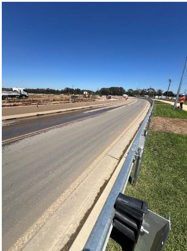
Figure 104 – General condition of the metal barrier.
