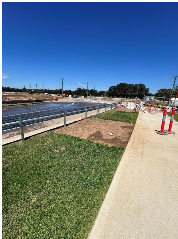
Figure 128 – General condition of the ground area.
