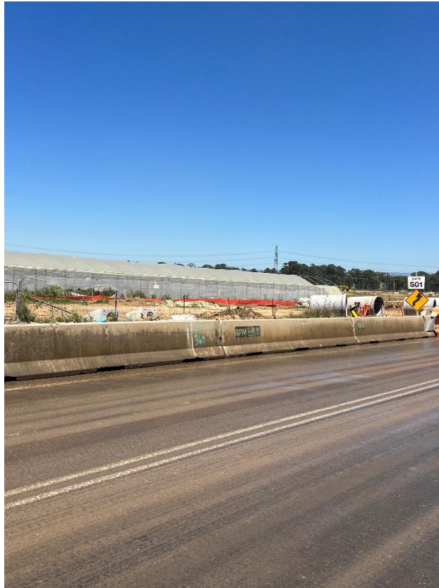
Figure 65 – General condition of the road.
