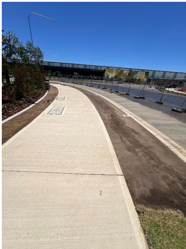
Figure 248 – General condition of the footpath.
