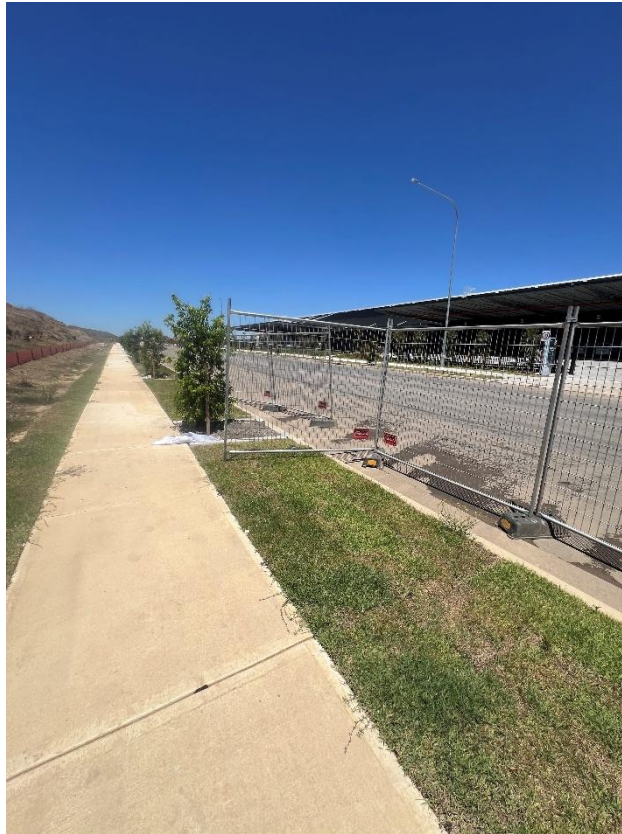
Figure 185 – General condition of the footpath.
