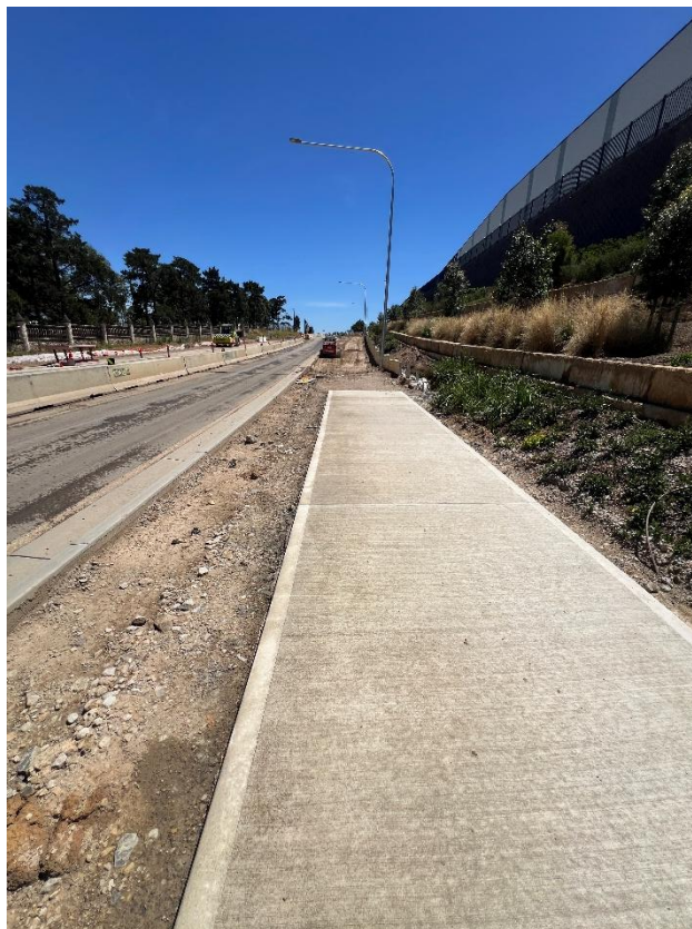
Figure 34 – General condition of the footpath.
