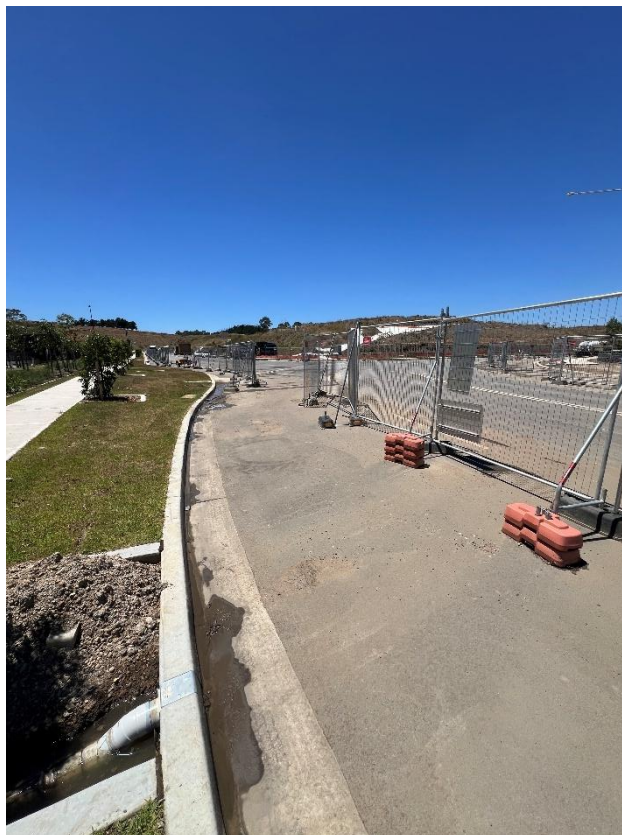
Figure 168 – General condition of the road.
