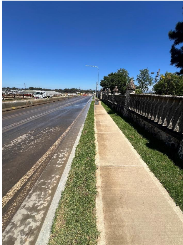
Figure 47 – General condition of the footpath.
