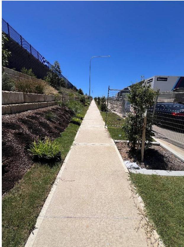
Figure 139 – General condition of the footpath.
