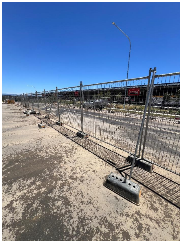
Figure 264 – General condition of the fence.
