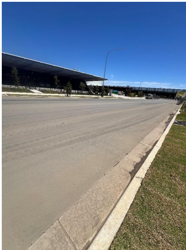
Figure 194 – General condition of the road.
