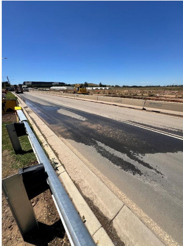
Figure 105 – General condition of the road.
