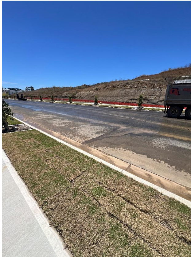
Figure 221 – General condition of the road.
