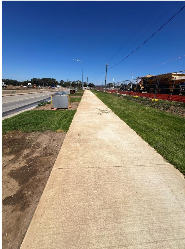
Figure 97 – General condition of the footpath.
