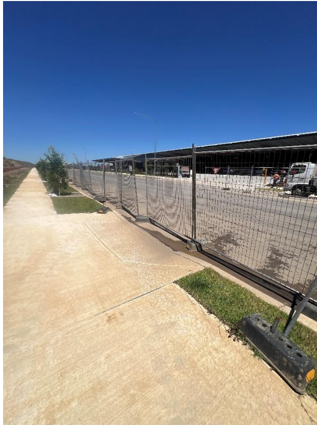
Figure 183 – General condition of the footpath.
