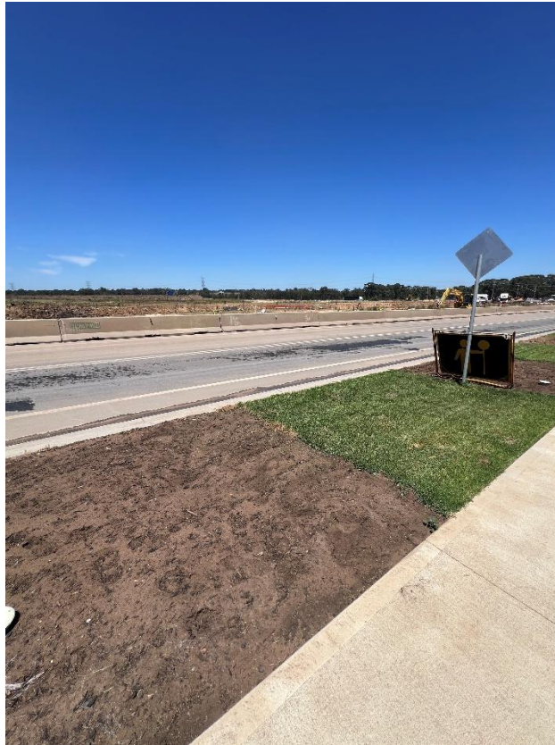
Figure 89 – General condition of the road.
