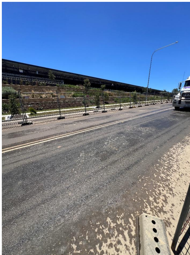
Figure 278 – General condition of the road.
