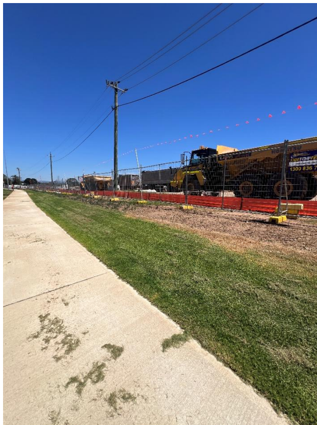
Figure 94 – General condition of the electrical post.
