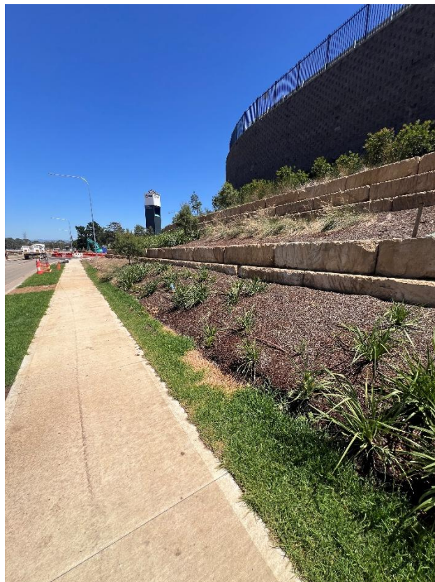
Figure 10 – General condition of the footpath.
