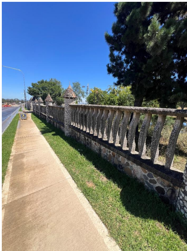
Figure 48 – General condition of the footpath.
