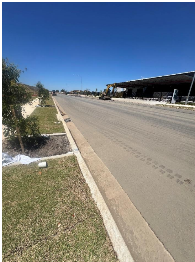
Figure 198 – General condition of the road.
