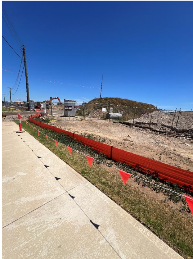
Figure 79 – General condition of the footpath.
