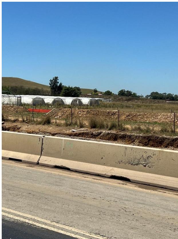
Figure 108 – General condition of the road.
