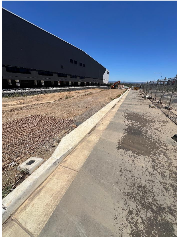
Figure 263 – General condition of the road.
