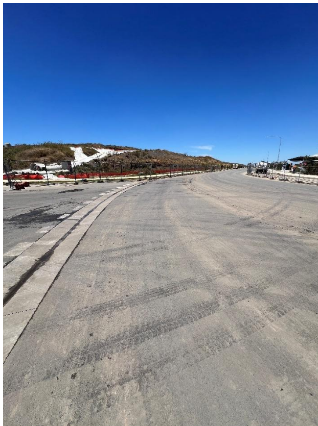
Figure 174 – General condition of the road.
