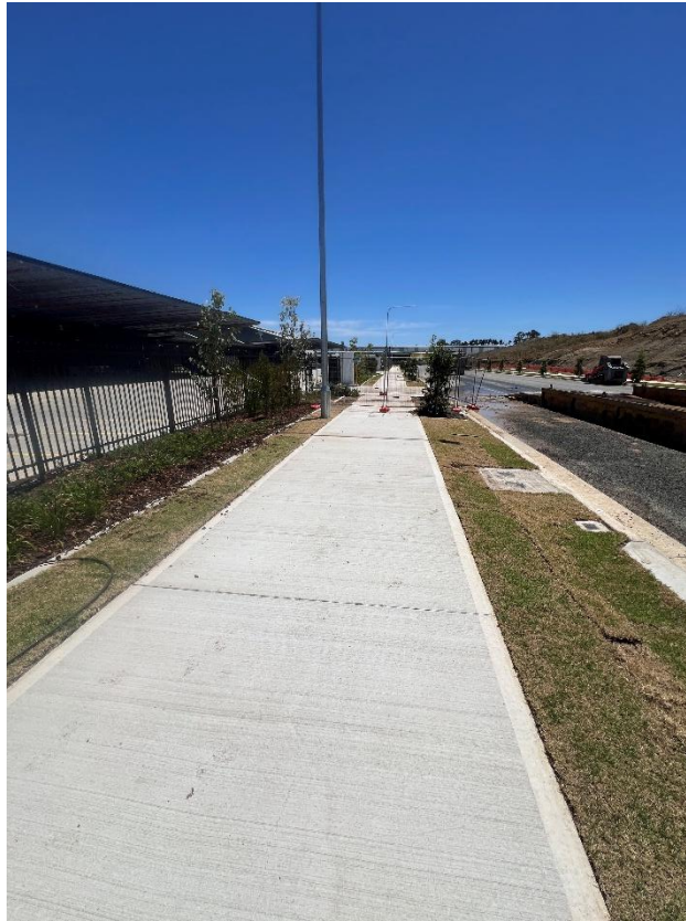
Figure 213 – General condition of the footpath.
