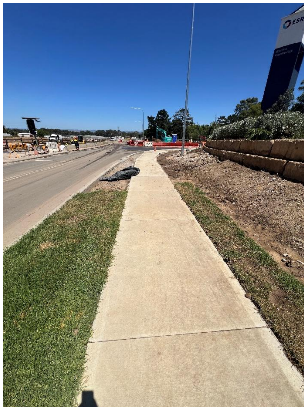
Figure 16 – General condition of the footpath.
