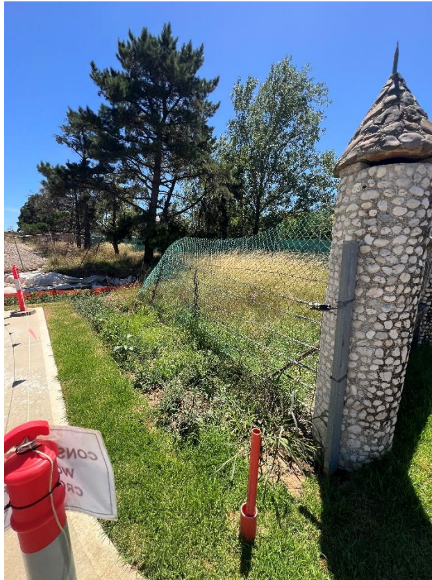
Figure 71 – General condition of the fence.
