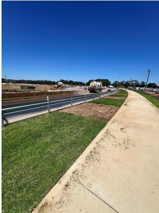
Figure 111 – General condition of the ground area.
