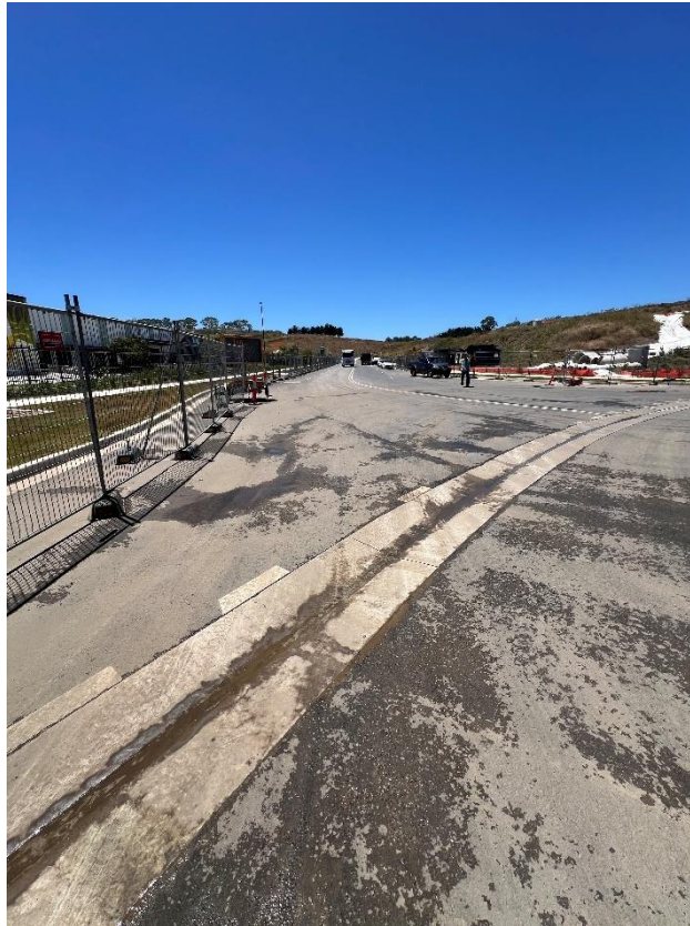
Figure 173 – General condition of the road.
