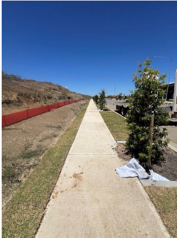
Figure 195 – General condition of the footpath.
