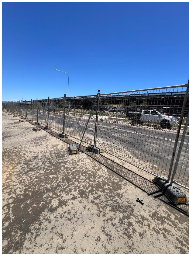
Figure 260 – General condition of the fence.
