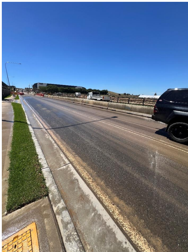
Figure 62 – General condition of the road.
