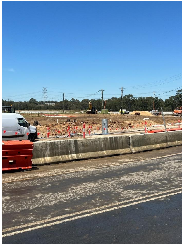
Figure 123 – General condition of the road.
