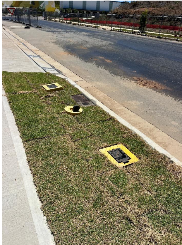
Figure 241 – General condition of the utility lid.
