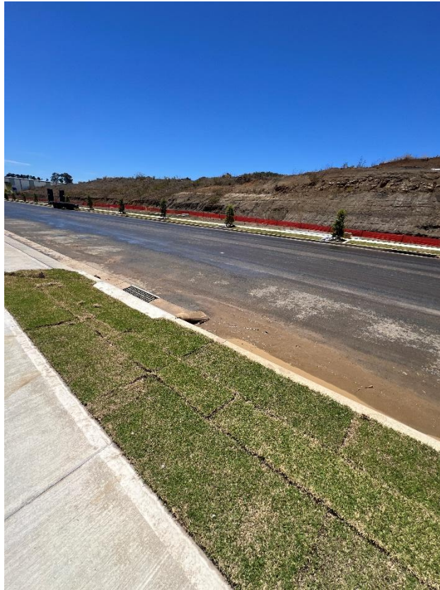
Figure 223 – General condition of the road.
