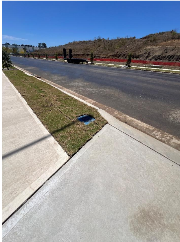
Figure 227 – General condition of the utility lid.
