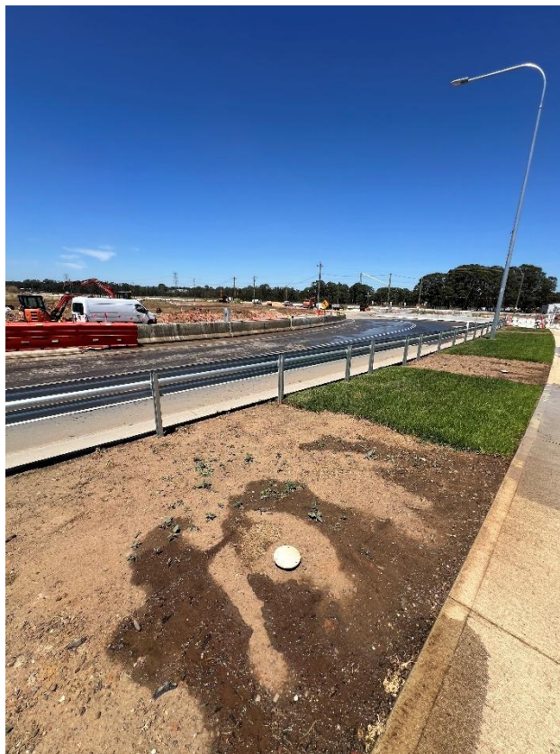
Figure 120 – General condition of the ground area.
