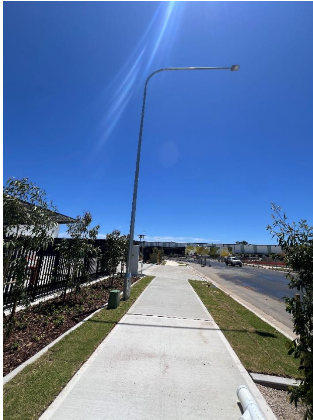
Figure 239 – General condition of the electrical light post.
