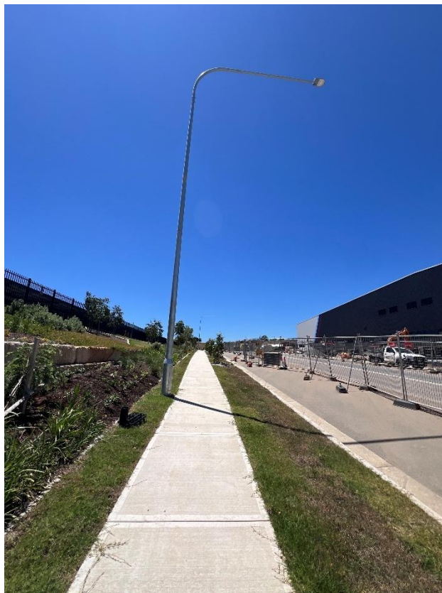
Figure 152 – General condition of the electrical light post.
