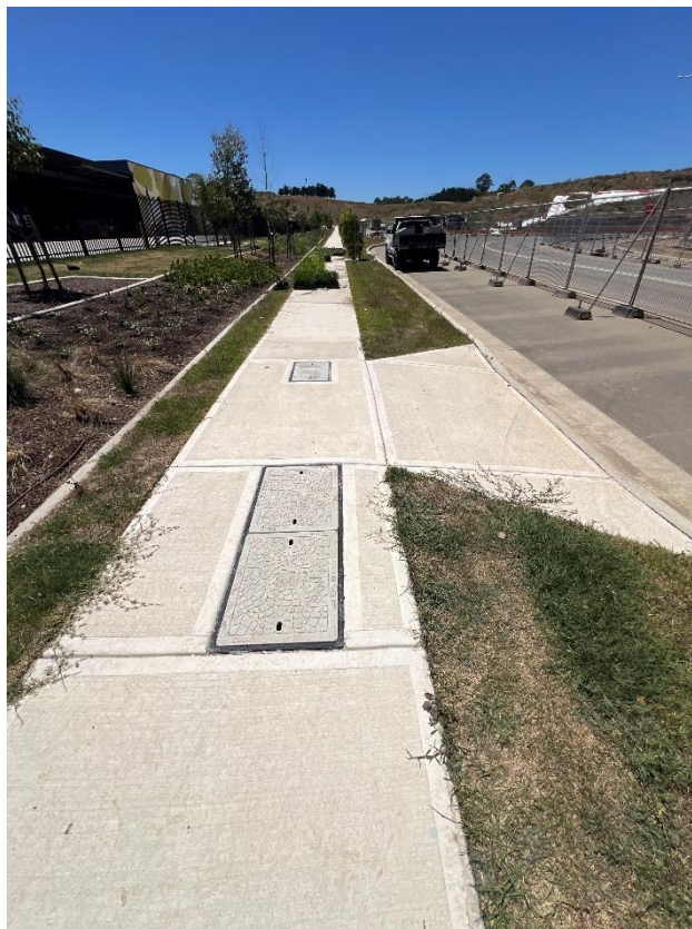
Figure 164 – General condition of the footpath.
