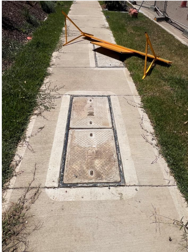
Figure 135 – General condition of the utility lid.
