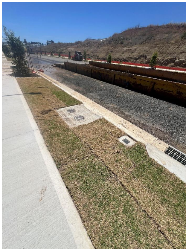
Figure 214 – General condition of the utility lid.
