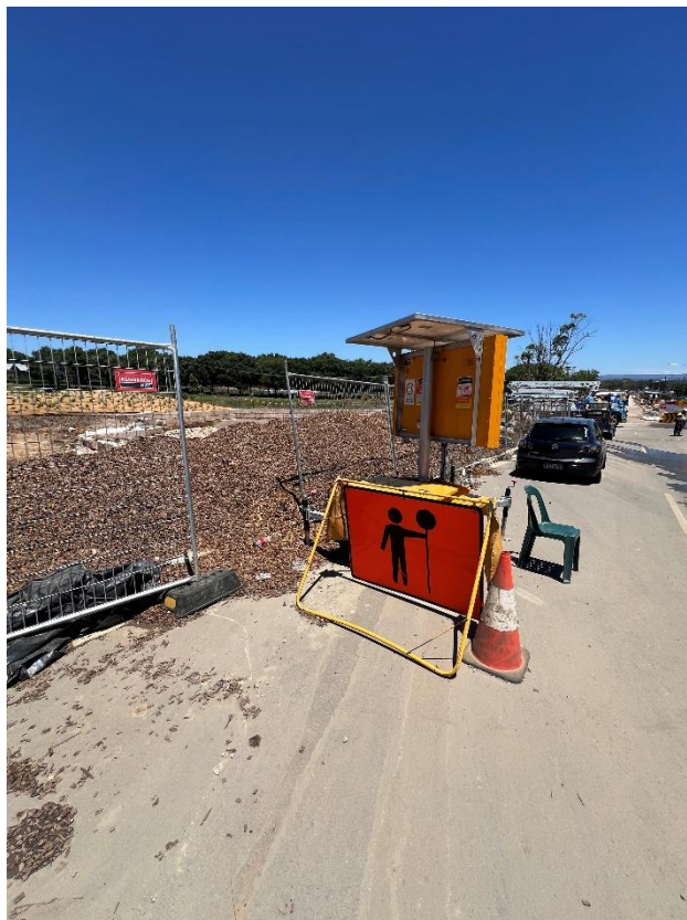
Figure 284 – General condition of the road signpost.
