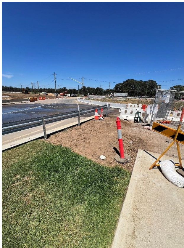
Figure 130 – General condition of the ground area.
