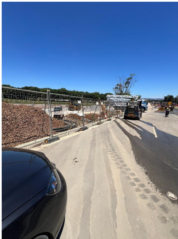
Figure 286 – General condition of the road.
