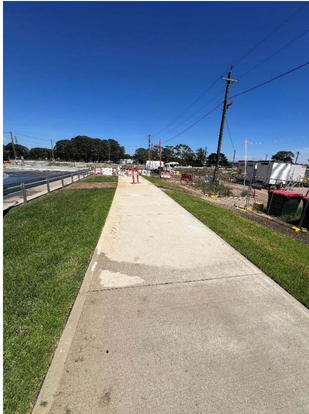
Figure 125 – General condition of the footpath.
