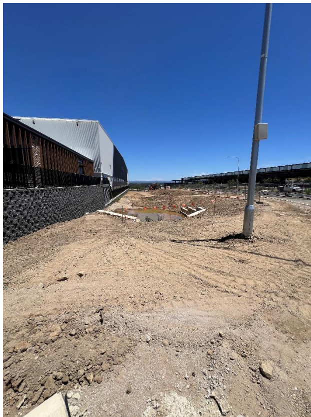
Figure 254 – General condition of the ground area.
