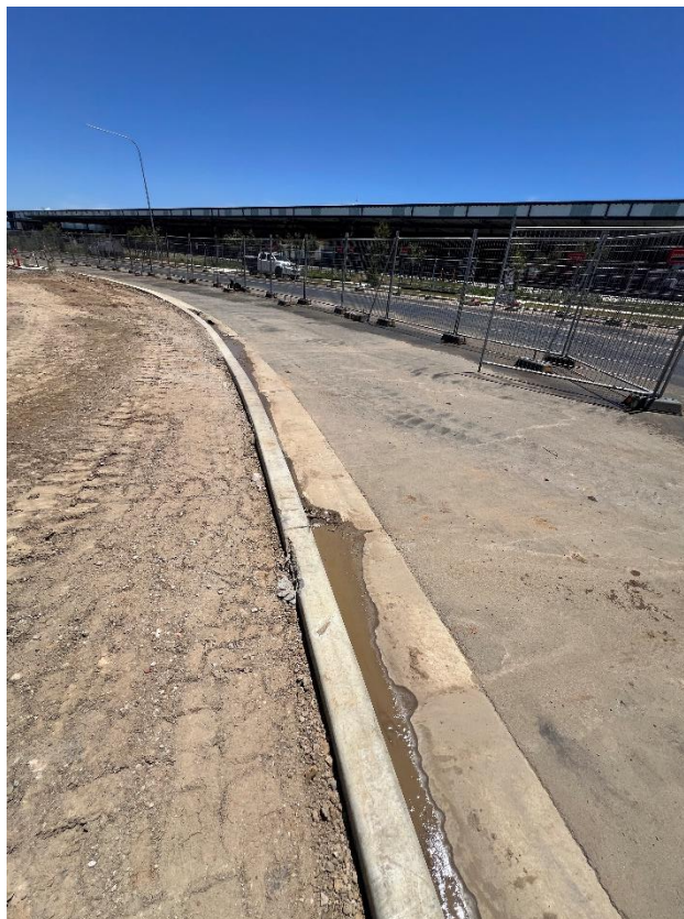
Figure 256 – General condition of the kerb.
