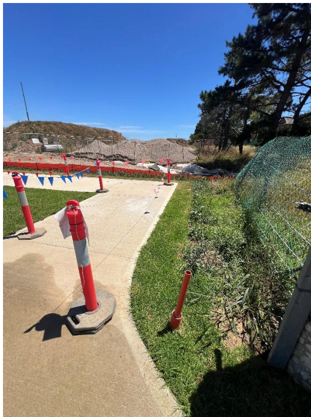
Figure 70 – General condition of the footpath.
