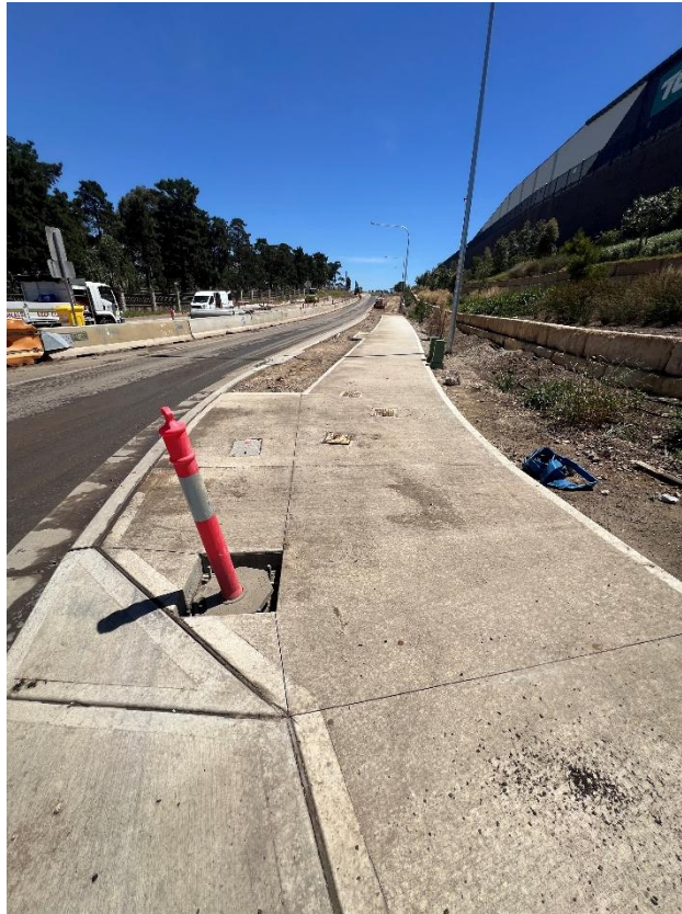
Figure 27 – General condition of the footpath.
