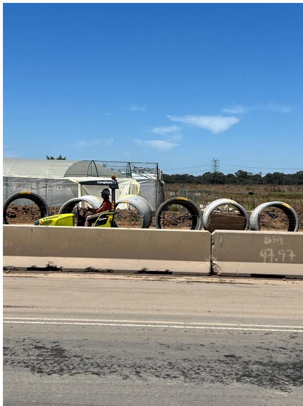
Figure 86 – General condition of the road.
