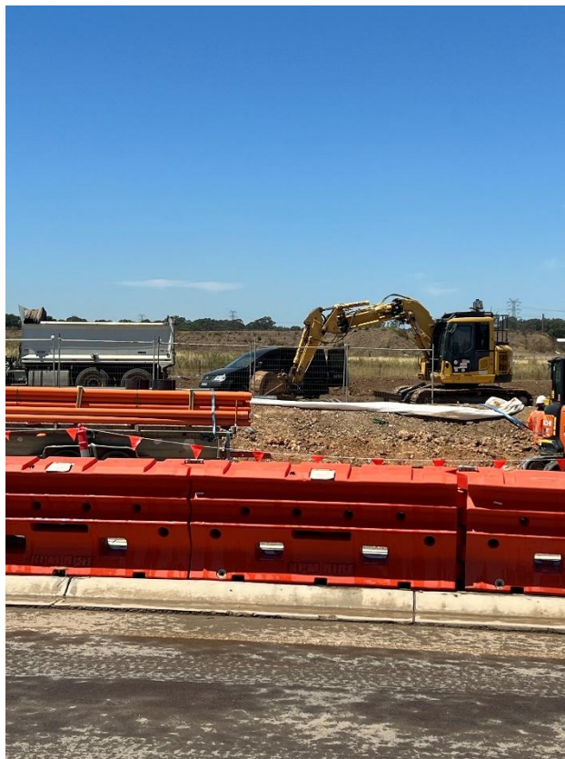
Figure 124 – General condition of the road barrier.
