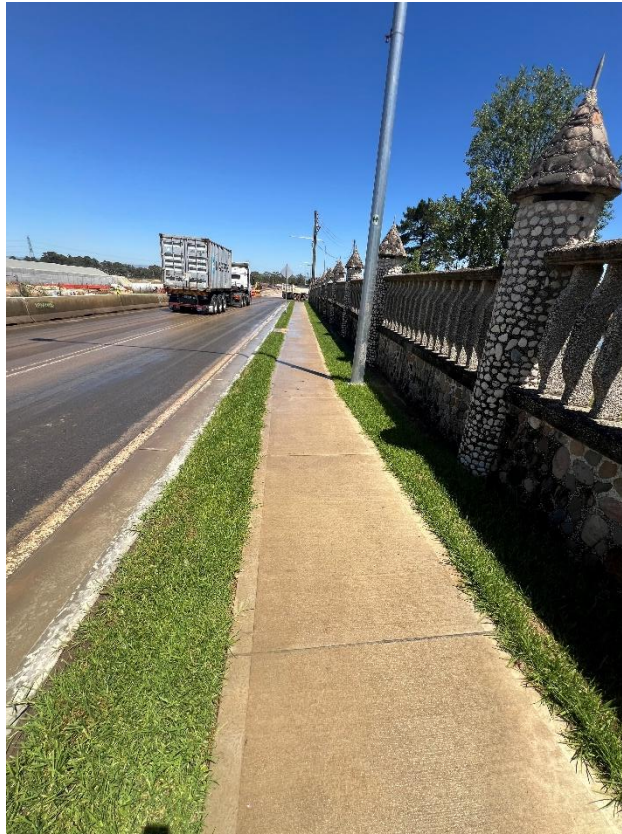
Figure 57 – General condition of the footpath.
