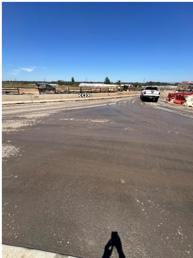
Figure 26 – General condition of the road.
