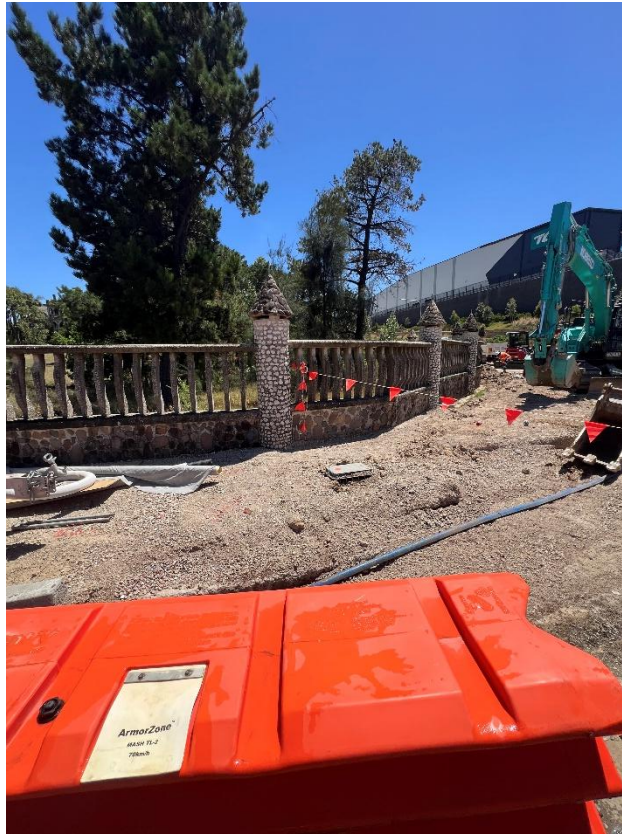
Figure 45 – General condition of the fence.
