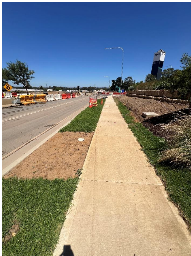
Figure 12 – General condition of the road.
