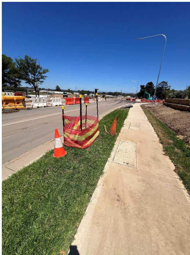
Figure 14 – General condition of the footpath.
