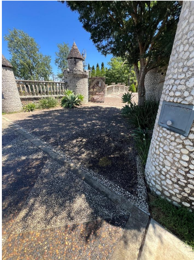
Figure 55 – General condition of the driveway.
