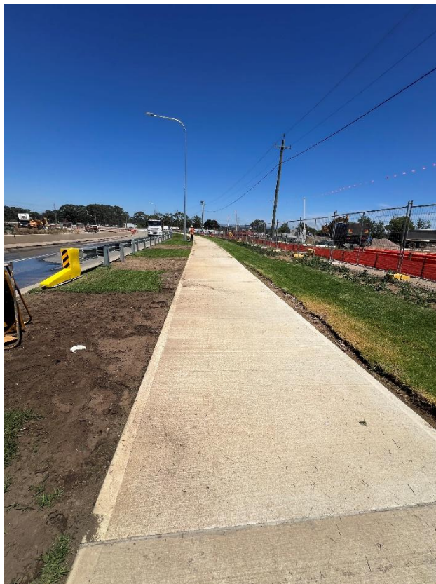
Figure 102 – General condition of the footpath.
