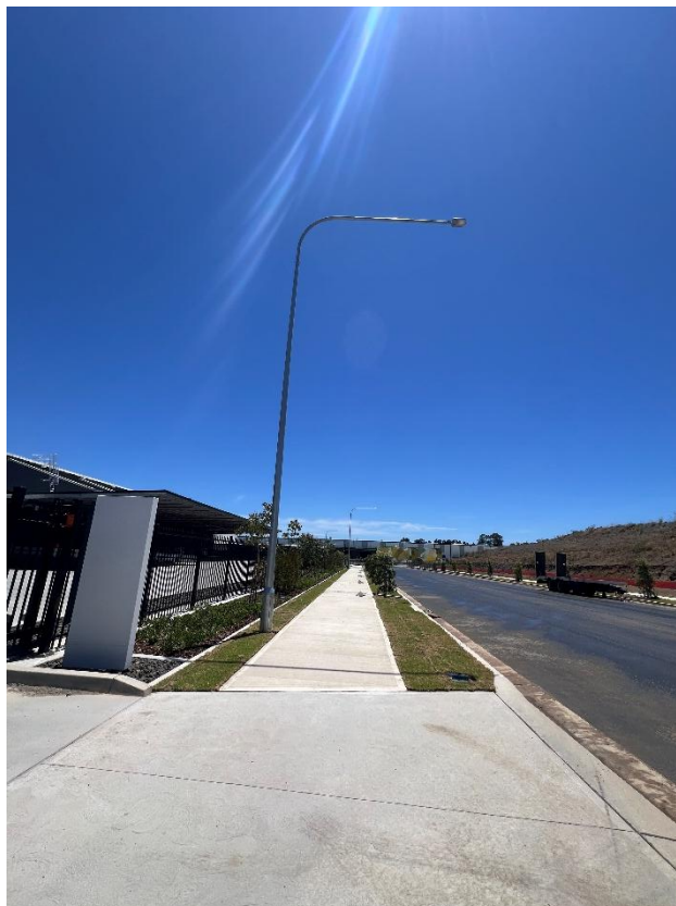
Figure 226 – General condition of the electrical light post.
