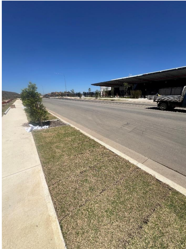
Figure 201 – General condition of the road.
