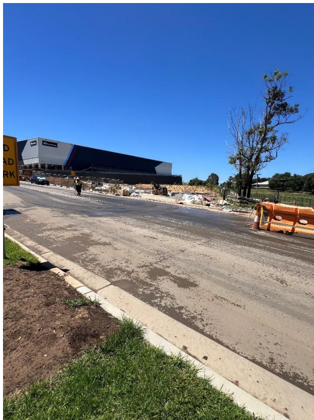
Figure 4 – General condition of the road.
