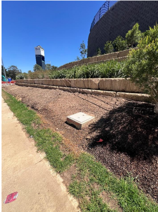
Figure 13 – General condition of the utility lid.
