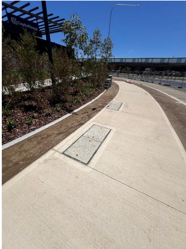
Figure 249 – General condition of the footpath.
