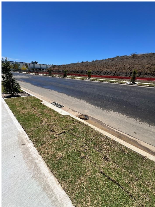
Figure 238 – General condition of the road.
