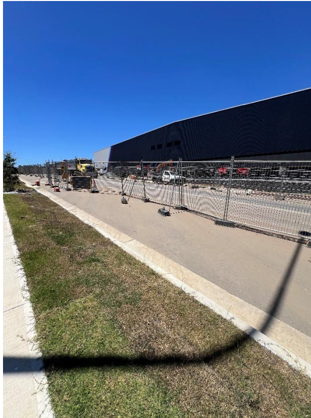
Figure 153 – General condition of the fence.
