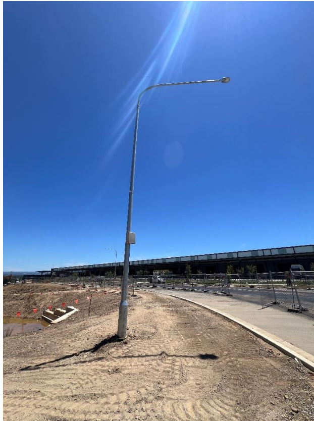
Figure 253 – General condition of the electrical light post.
