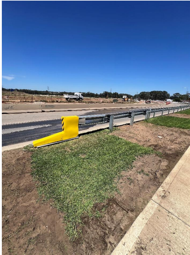
Figure 103 – General condition of the ground area.
