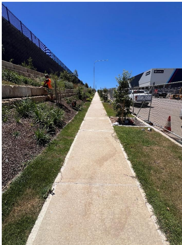
Figure 138 – General condition of the footpath.
