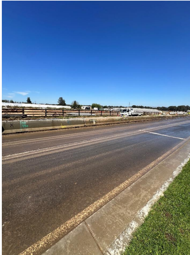
Figure 49 – General condition of the road.
