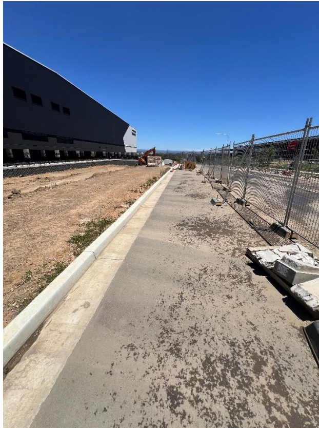
Figure 265 – General condition of the road.
