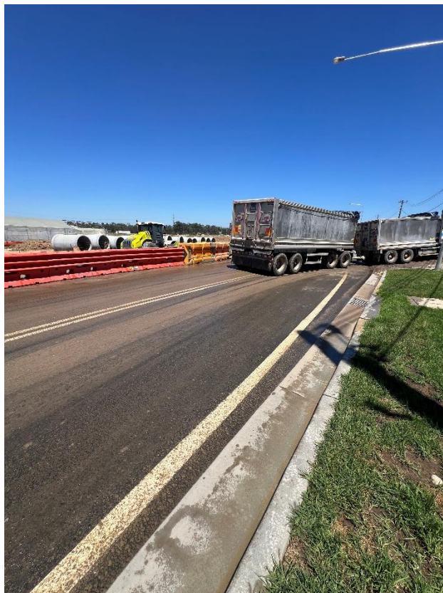
Figure 74 – General condition of the road.
