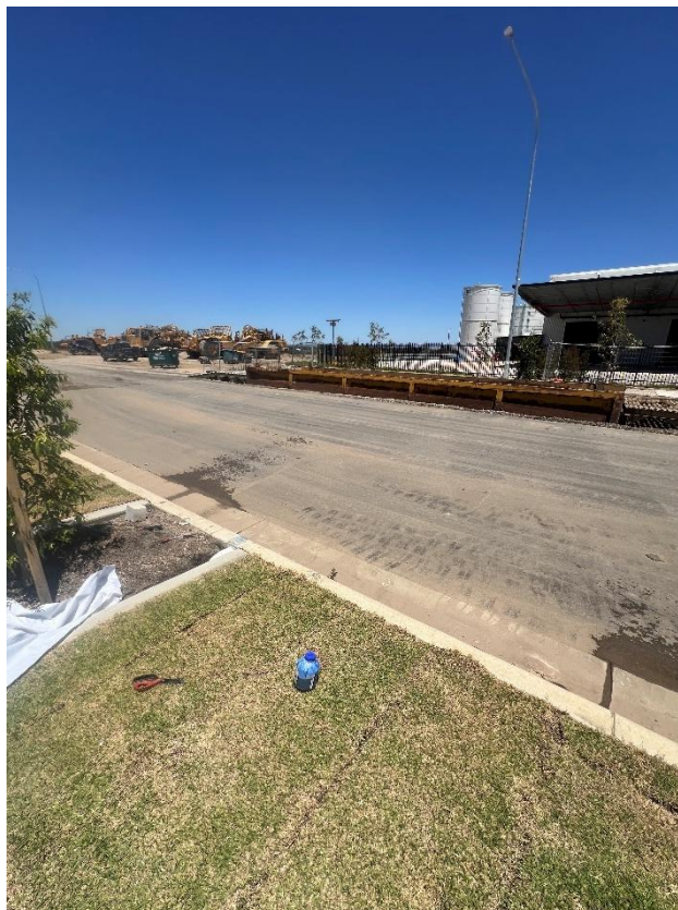
Figure 210 – General condition of the road.
