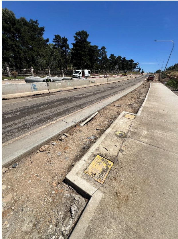
Figure 31 – General condition of the utility lid.
