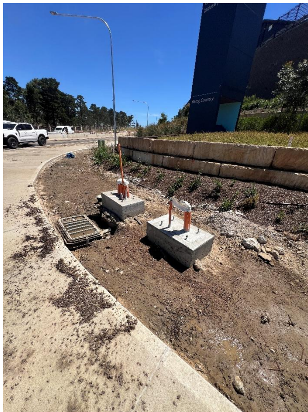
Figure 24 – General condition of the utility lid.
