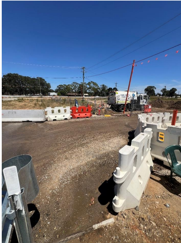
Figure 133 – General condition of the road barrier.
