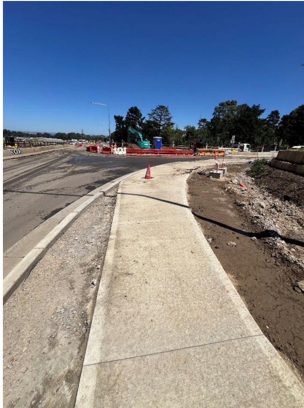
Figure 21 – General condition of the footpath.
