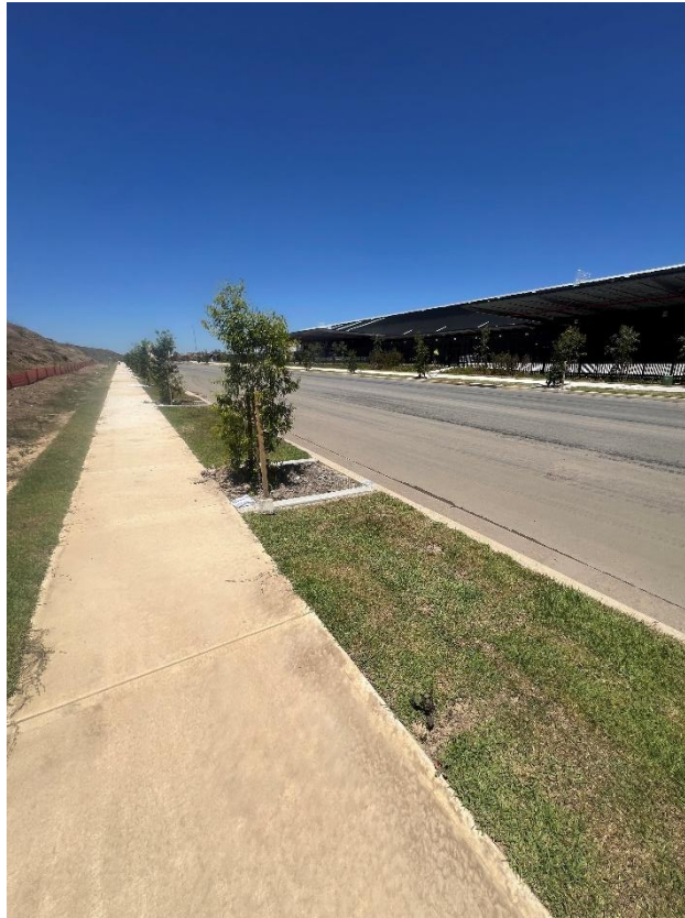
Figure 187 – General condition of the footpath.
