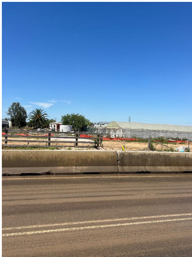
Figure 64 – General condition of the road.
