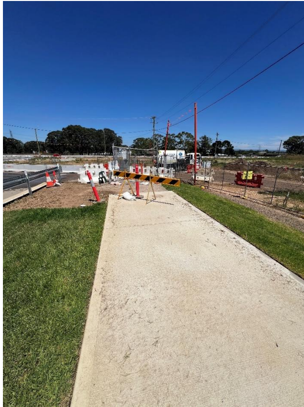
Figure 129 – General condition of the footpath.
