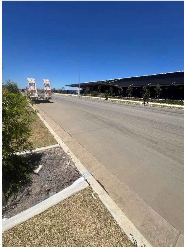
Figure 193 – General condition of the road.
