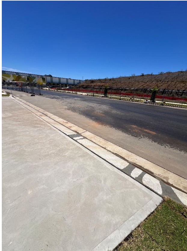
Figure 243 – General condition of the driveway.
