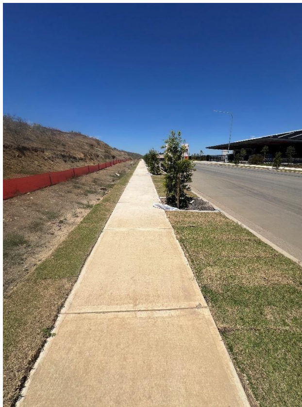
Figure 192 – General condition of the footpath.
