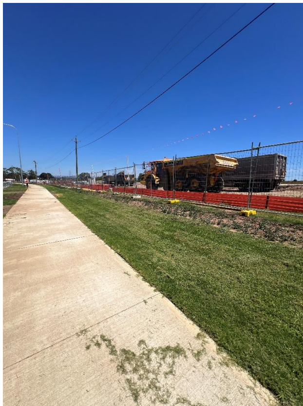
Figure 98 – General condition of the footpath.
