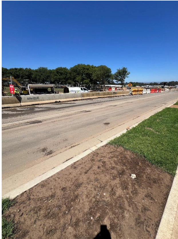
Figure 11 – General condition of the road.
