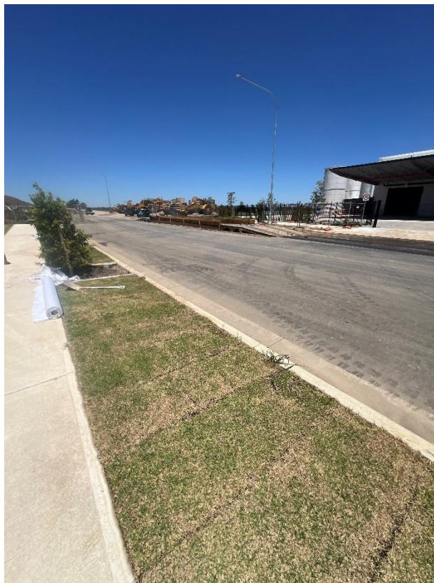
Figure 208 – General condition of the road.
