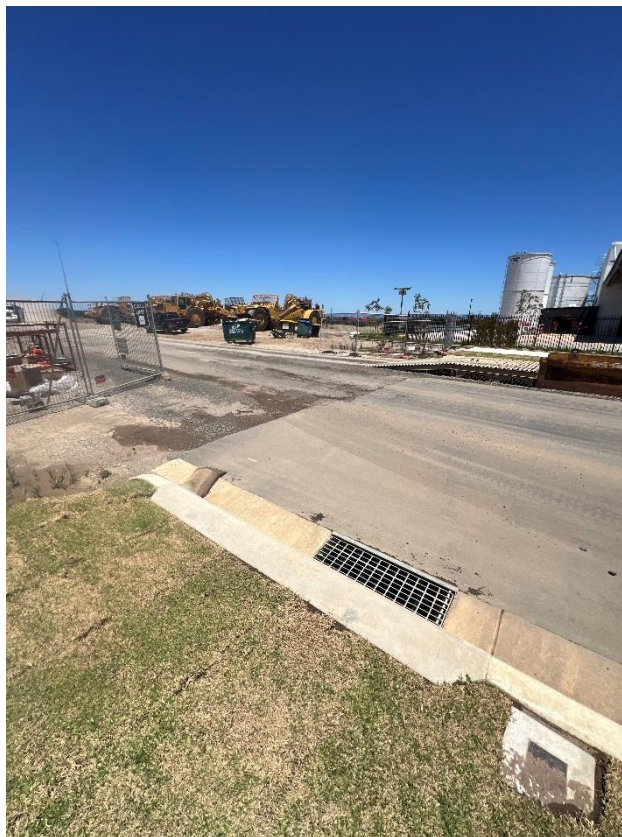
Figure 212 – General condition of the road.
