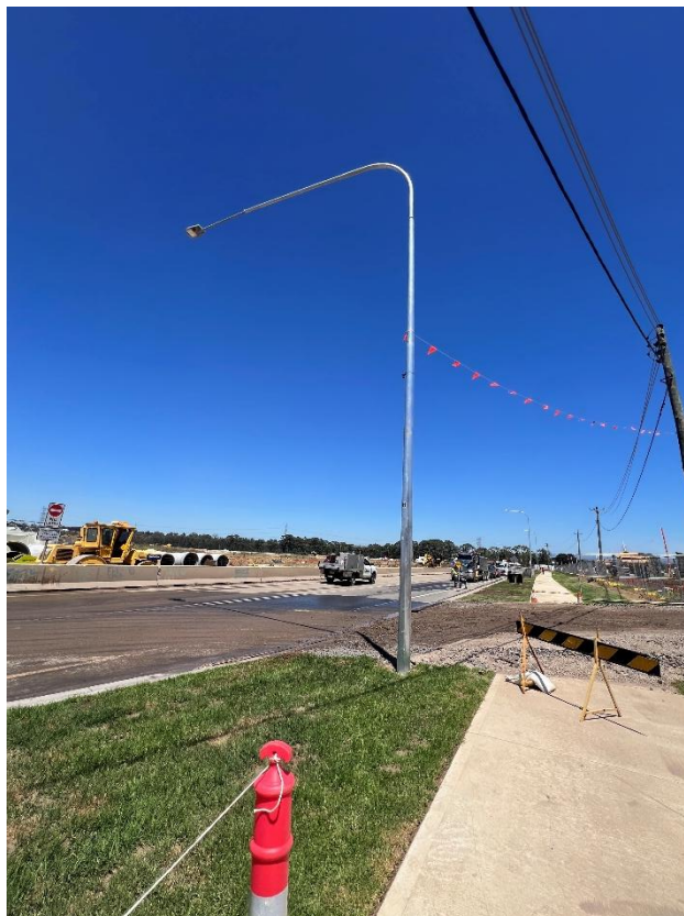
Figure 80 – General condition of the electrical light post.
