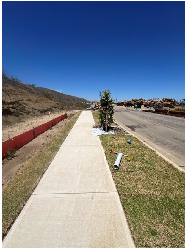
Figure 209 – General condition of the footpath.
