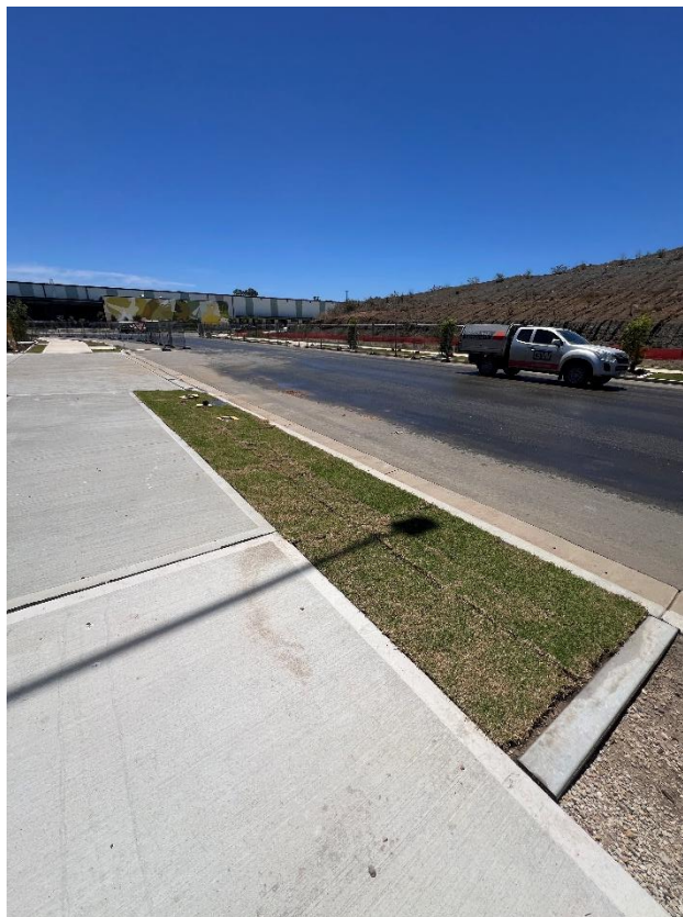
Figure 240 – General condition of the road.
