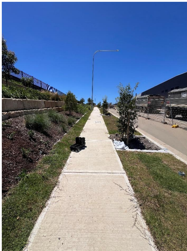
Figure 150 – General condition of the footpath.
