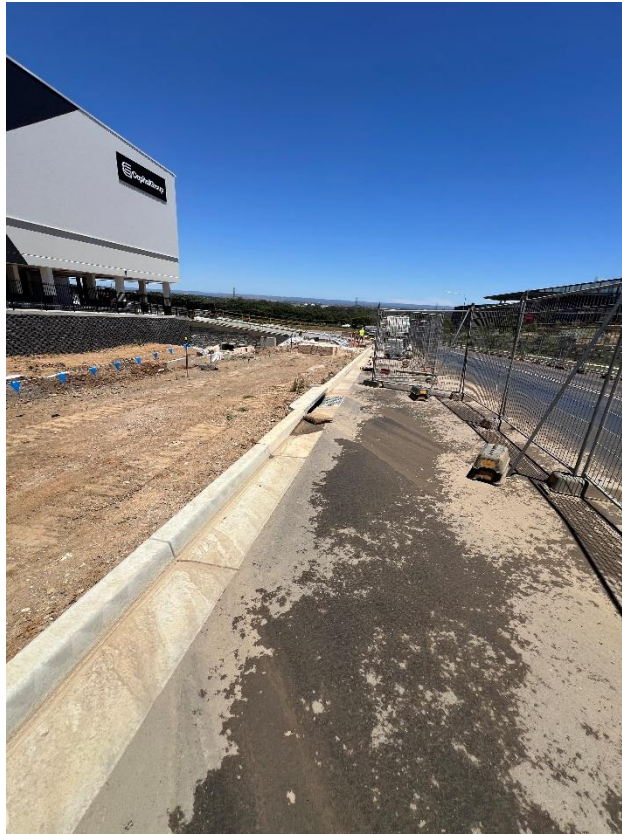
Figure 275 – General condition of the road.
