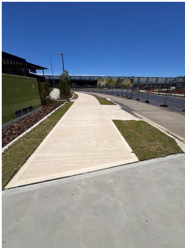
Figure 244 – General condition of the footpath.
