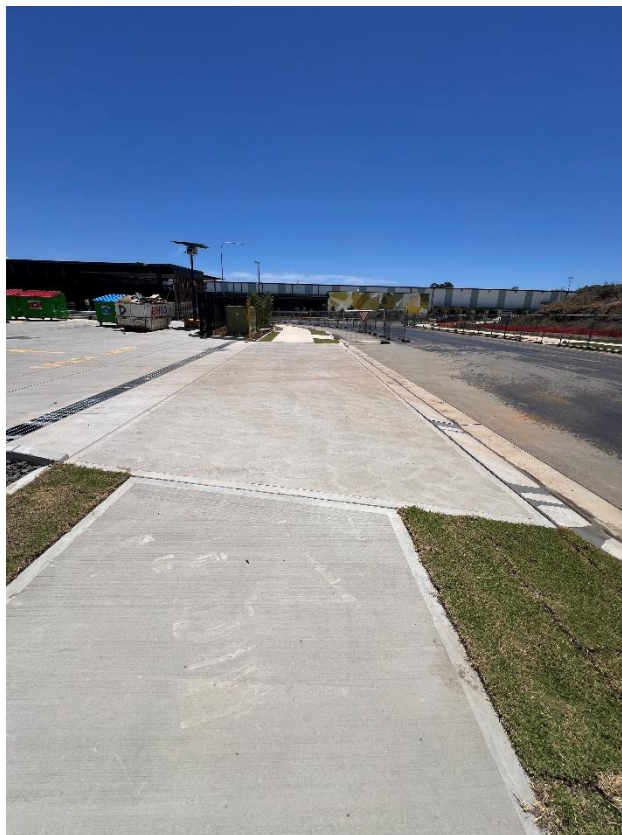
Figure 242 – General condition of the driveway.
