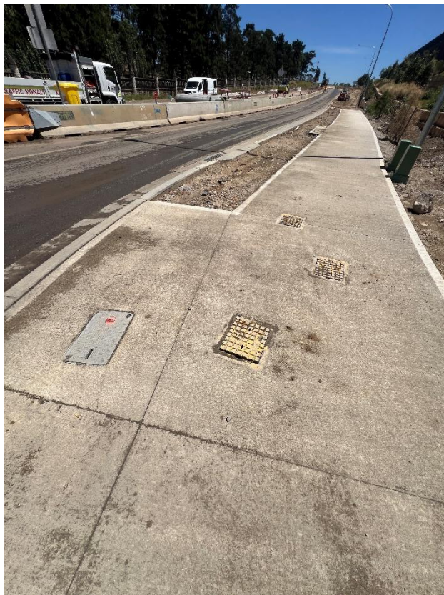
Figure 28 – General condition of the utility lid.
