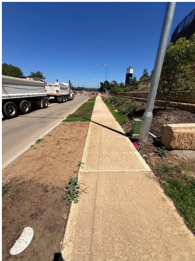
Figure 6 – General condition of the footpath.
