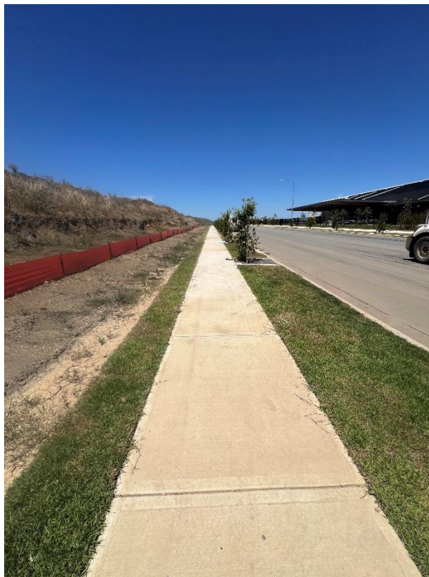
Figure 188 – General condition of the footpath.
