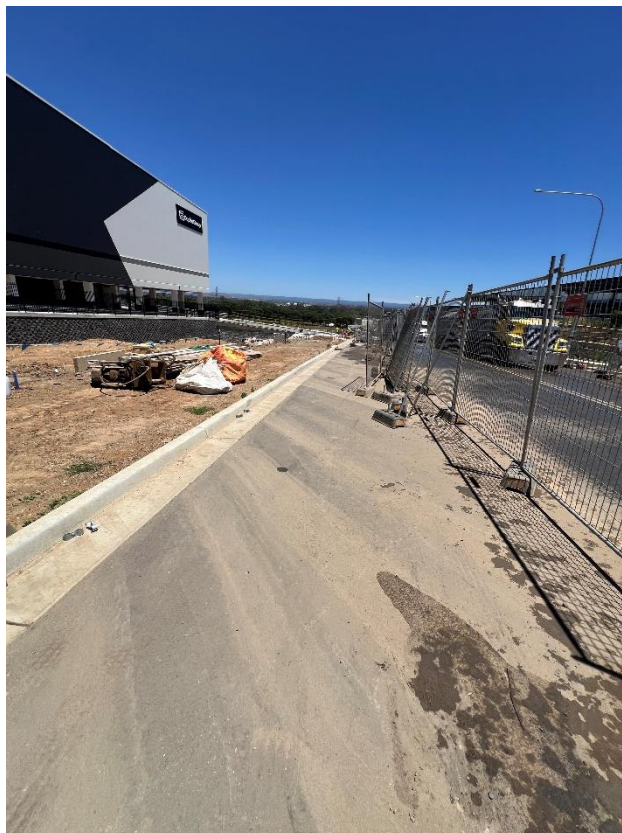
Figure 274 – General condition of the road.
