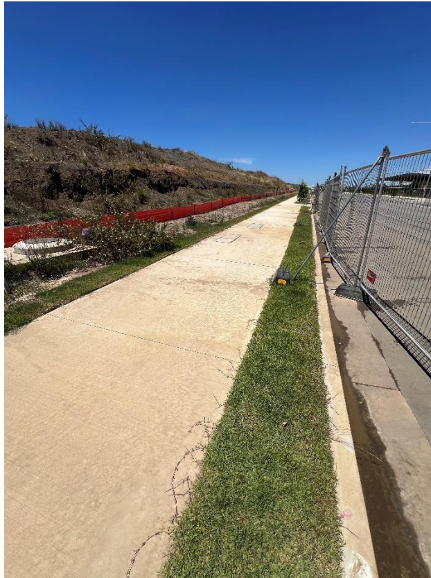
Figure 177 – General condition of the footpath.
