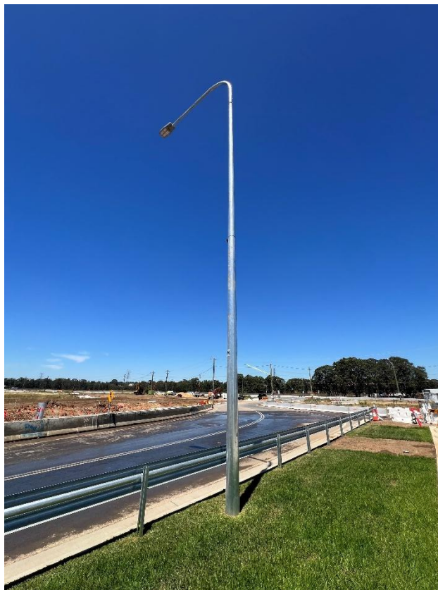
Figure 126 – General condition of the electrical light post.
