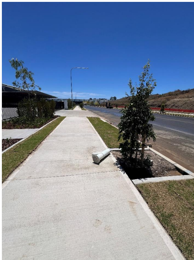
Figure 222 – General condition of the footpath.
