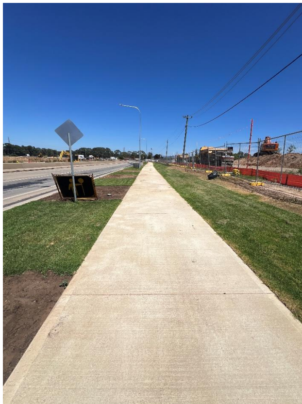
Figure 90 – General condition of the footpath.
