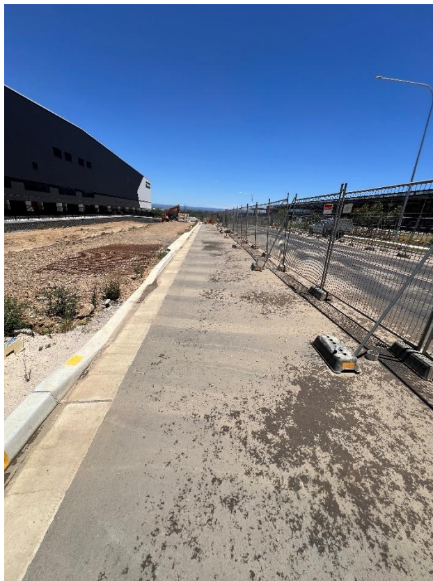
Figure 262 – General condition of the road.
