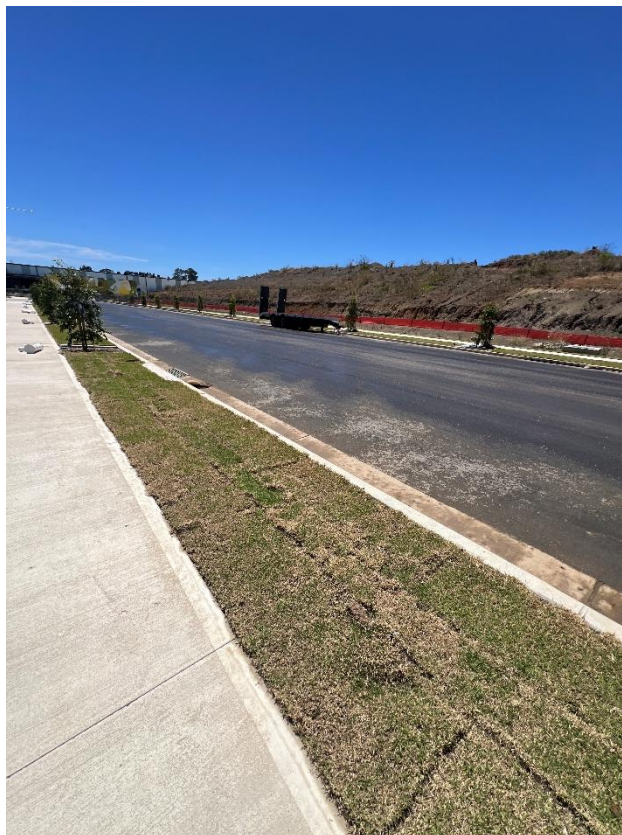
Figure 228 – General condition of the road.
