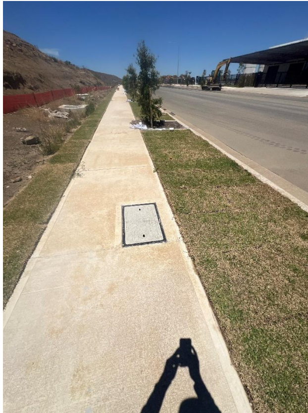
Figure 197 – General condition of the footpath.
