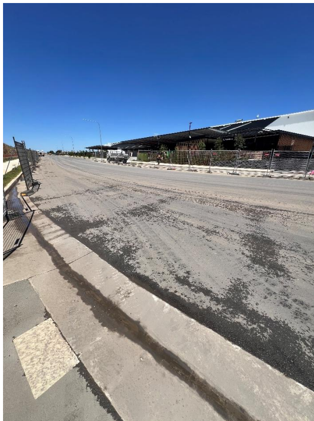
Figure 176 – General condition of the road.
