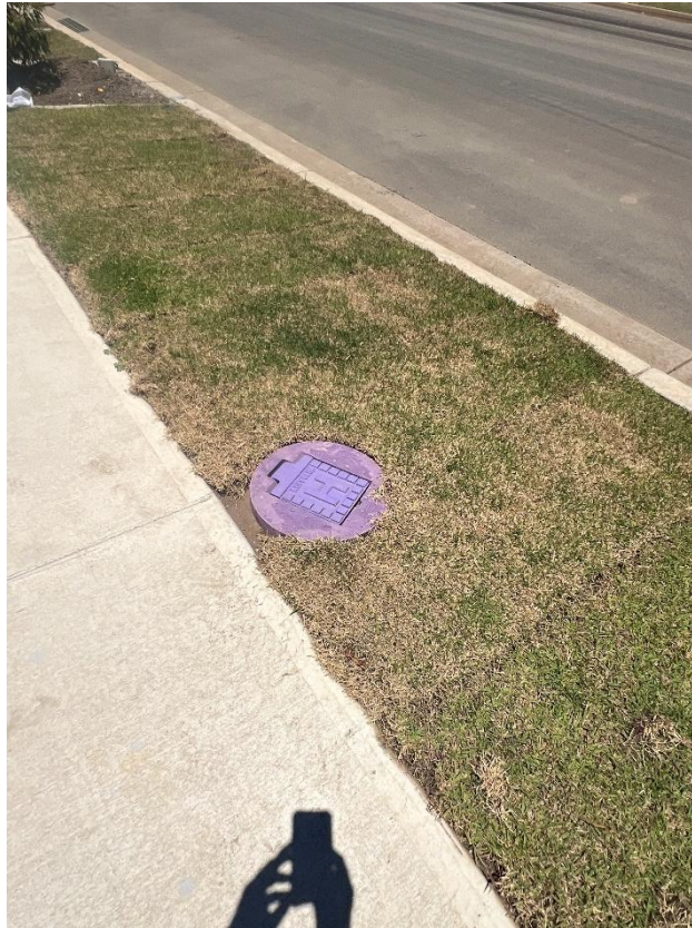
Figure 203 – General condition of the utility lid.
