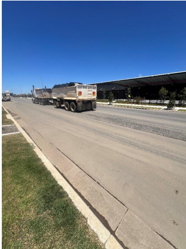
Figure 189 – General condition of the road.
