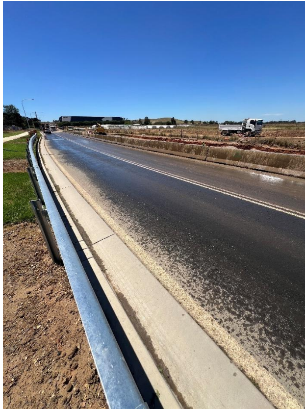
Figure 115 – General condition of the road.
