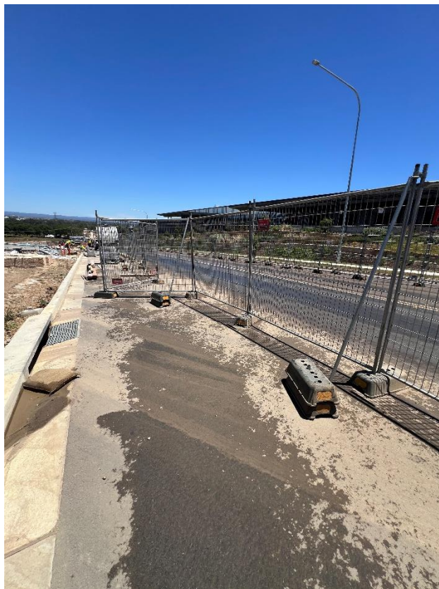
Figure 276 – General condition of the road.
