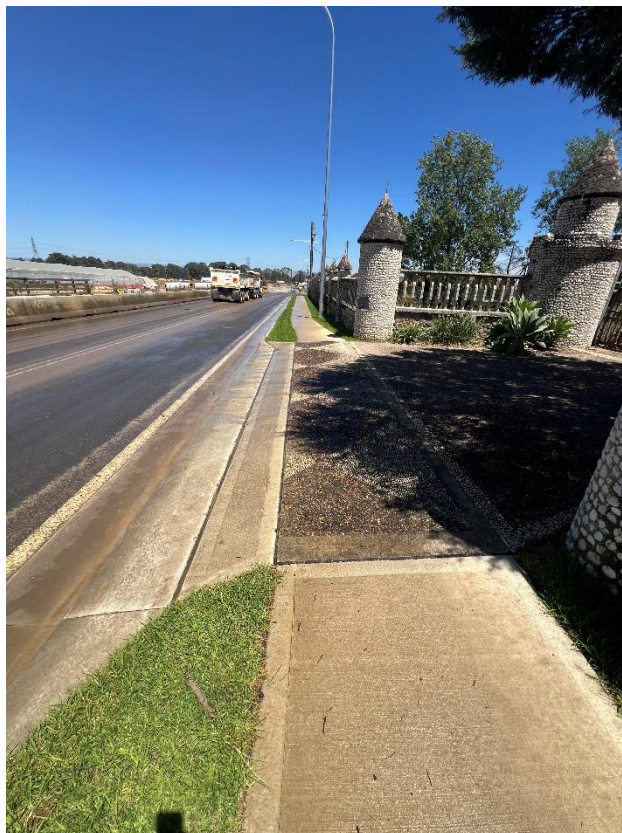
Figure 54 – General condition of the driveway.
