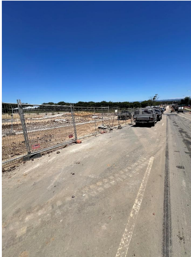
Figure 281 – General condition of the road.
