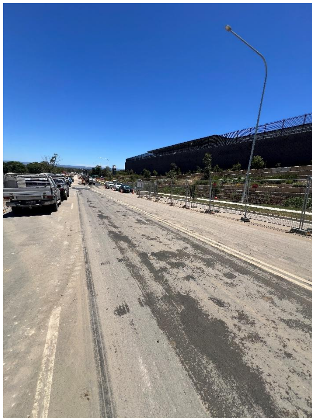
Figure 282 – General condition of the road.
