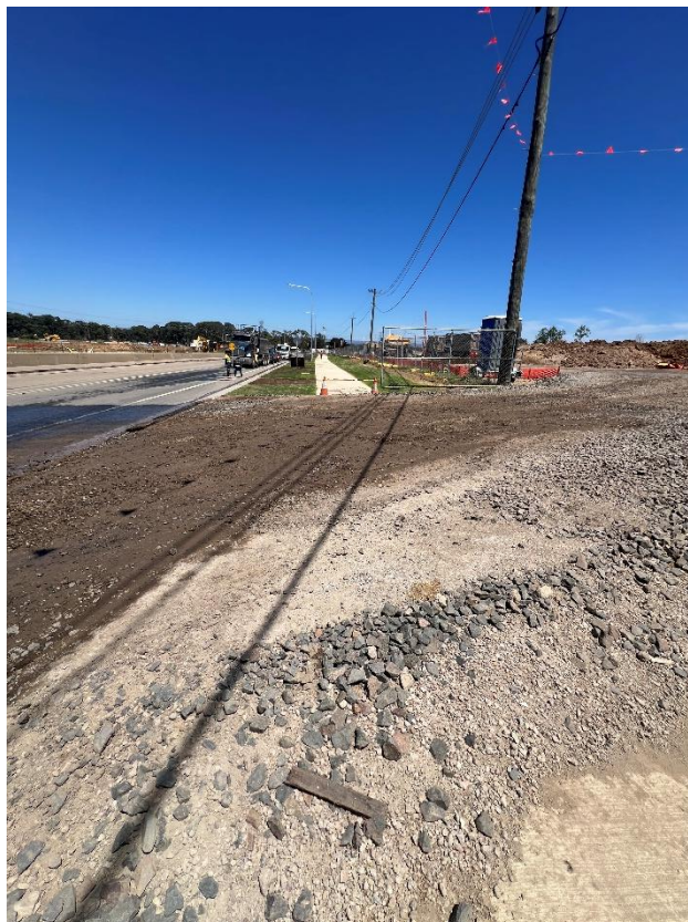
Figure 82 – General condition of the driveway.
