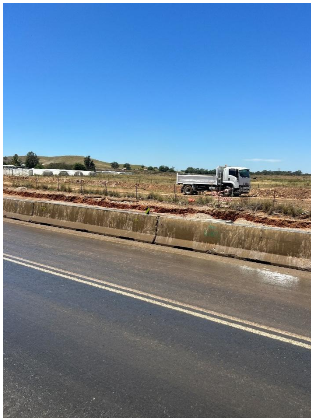
Figure 116 – General condition of the road.
