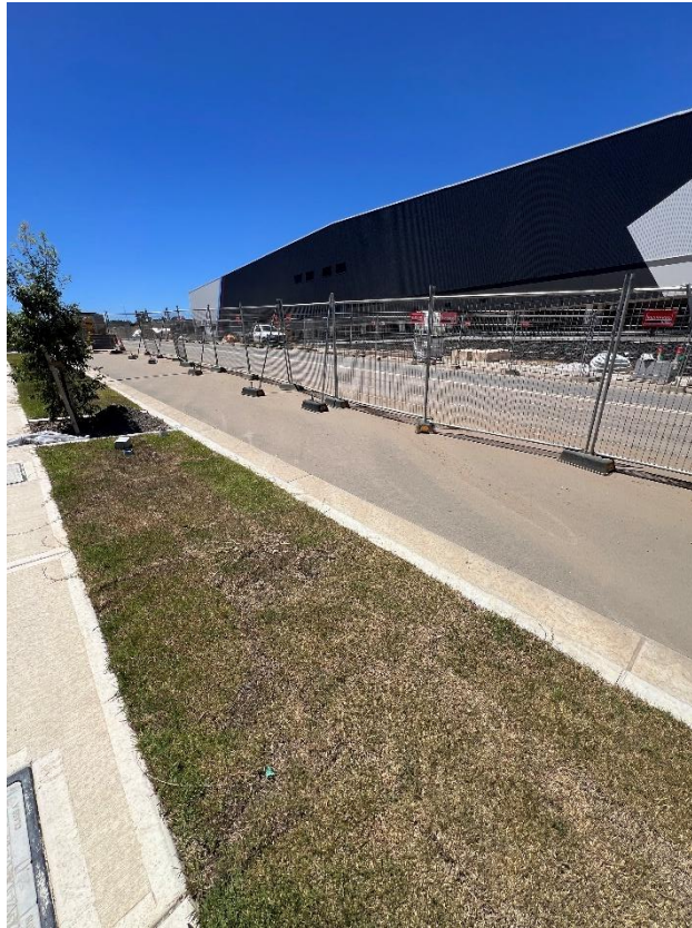
Figure 151 – General condition of the fence.
