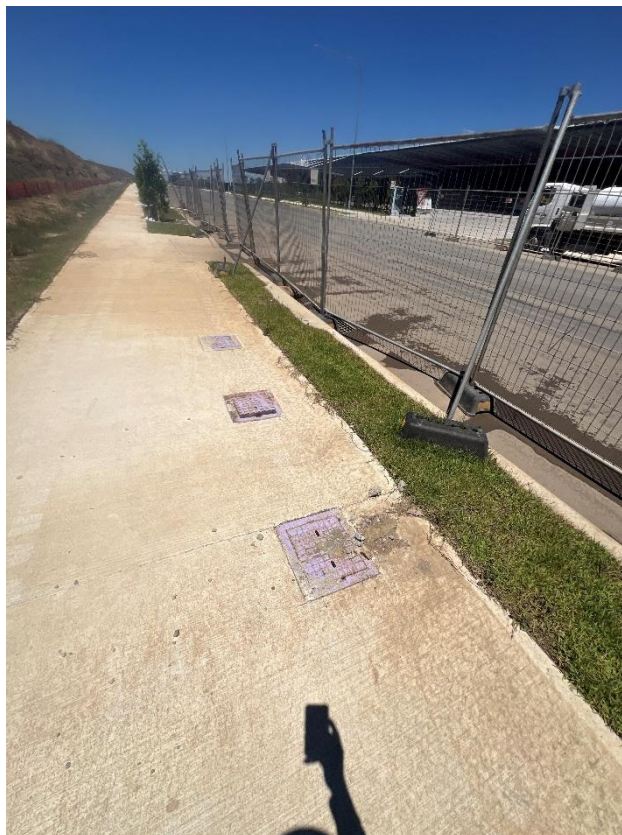
Figure 182 – General condition of the footpath.
