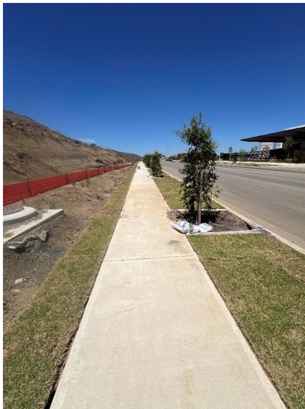
Figure 200 – General condition of the footpath.
