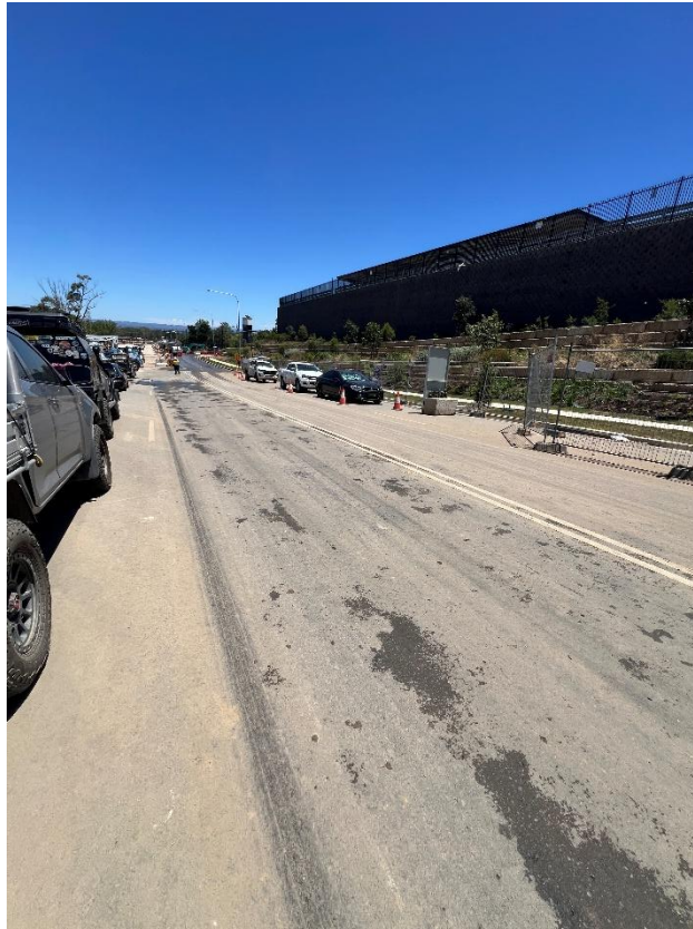
Figure 283 – General condition of the road.
