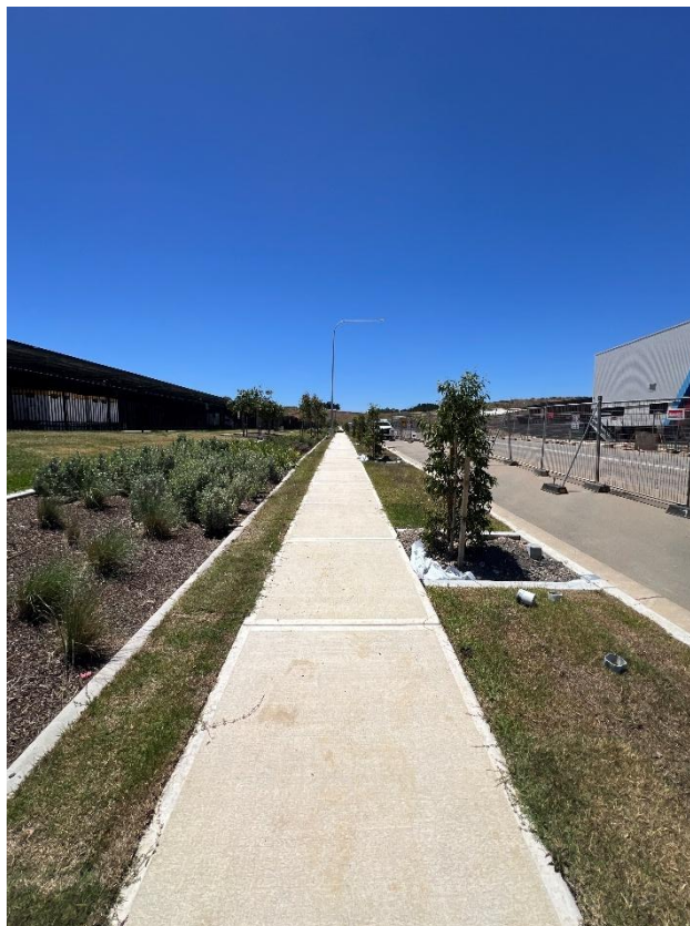
Figure 158 – General condition of the footpath.
