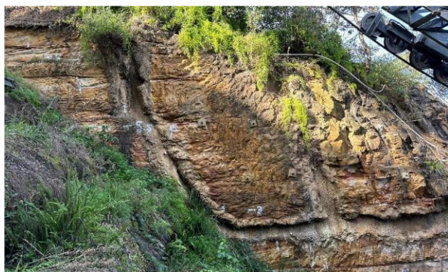
Picture 15 Existing excavation at the existing Lower Station showing the sub-vertical joints and bolts observed within the exposed rock face
