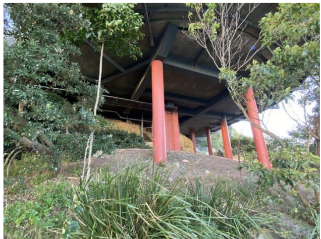
Picture 8 Supporting pylons and sandstone under the existing Lower Station
