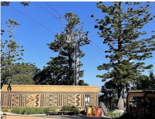
Picture 3 View of existing cableway route from inside the Zoo
