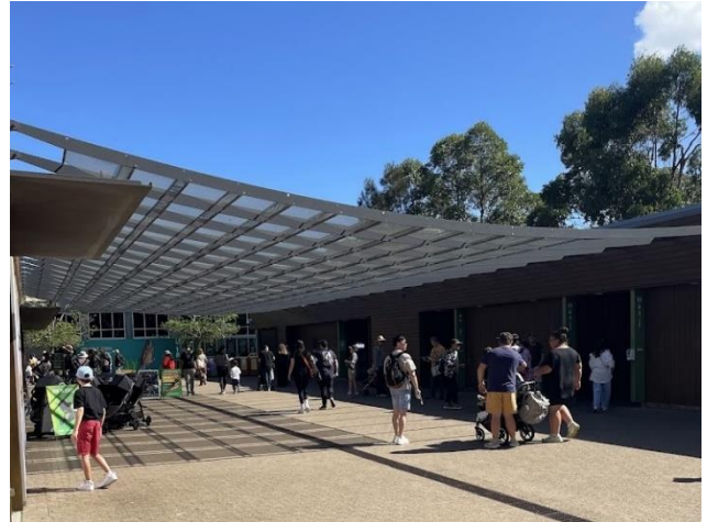
Picture 2 View of existing upper station entrance from the Plaza
