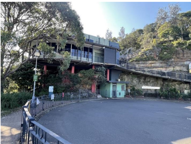
Picture 5 View of existing lower station at Athol Wharf Road
