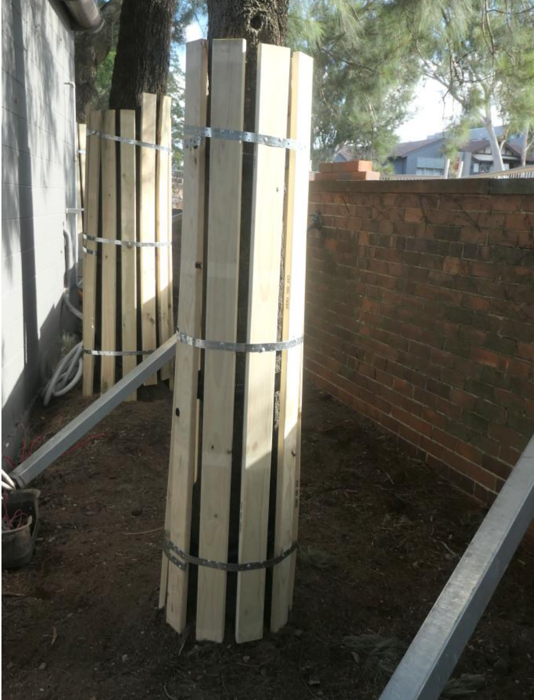
Figure 3.2 – Example of acceptable Trunk Protection batten installation. (Photo: Arterra)
