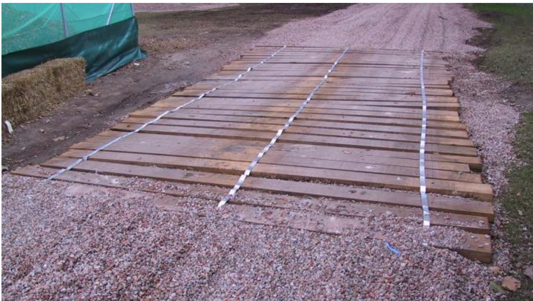
Figure 3.1 – Example of acceptable Tree Protection Area ground protection (Photo: Arterra)
