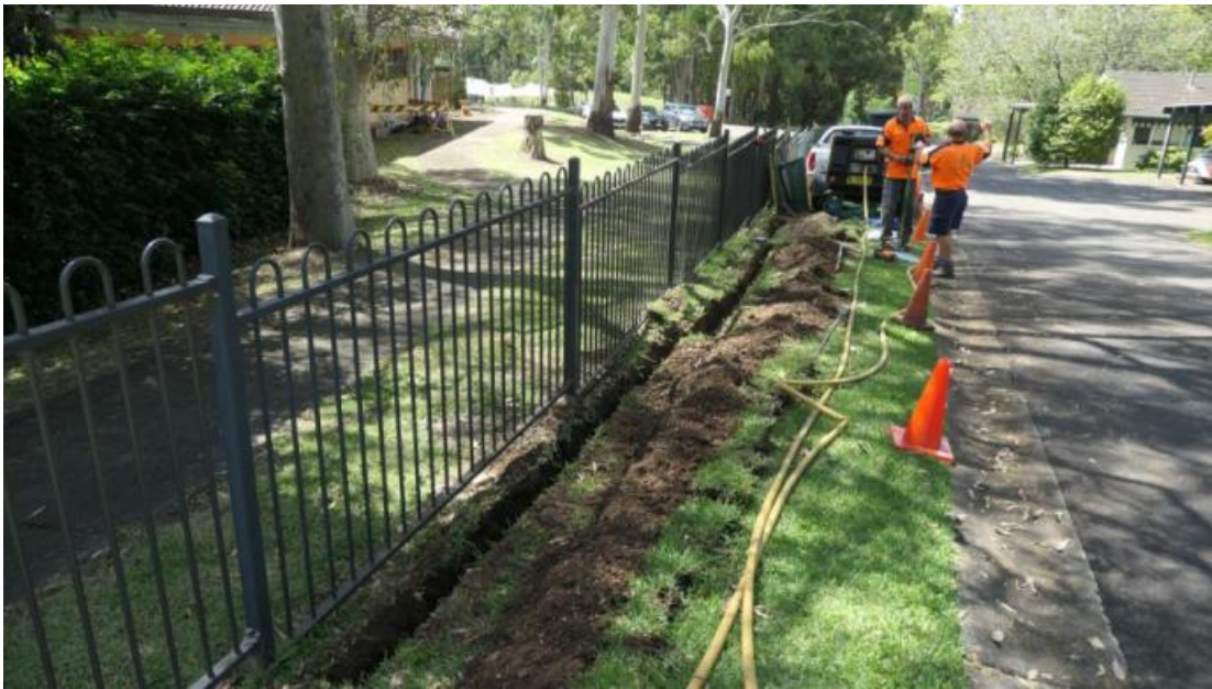
Figure 4 – Photo of the area where root investigations were carried out, with trenching completed. (Photo: Arterra 16/2/22)
