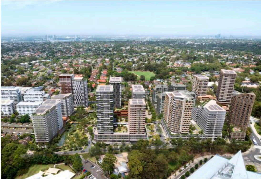
Figure 2.1 –Overview render of the proposed Master Plan development when viewed from the northern side. Regrading is required to resurface the creek line within the proposed open space and excavation is required to accommodate the proposed buildings and basement levels (Source: Arterra - BVN)
