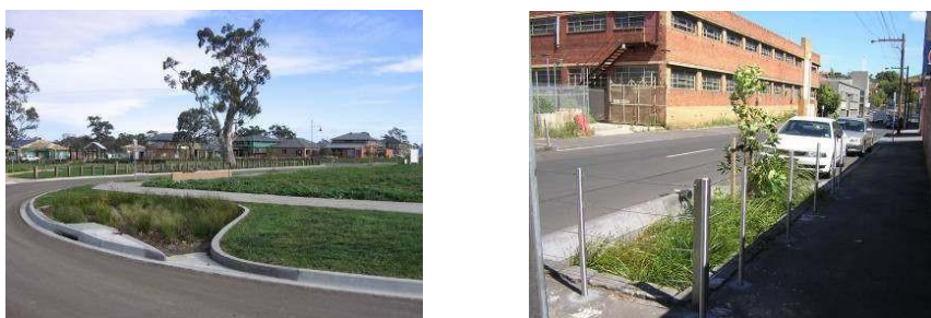
Figure 18: Examples of bioretention raingardens
