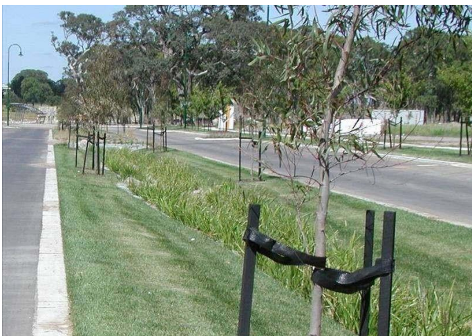
Figure 10: Typical swale and buffer strip configuration
