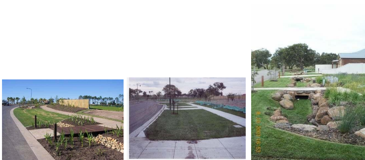
Figure 11 - Examples of different types of swale crossings
