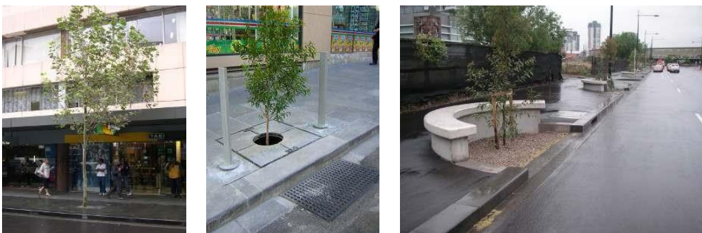
Figure 17 - Example street tree bioretention systems
