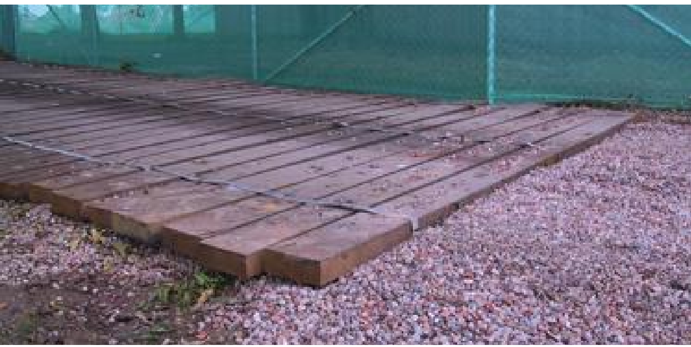
Example image of acceptable ground protection rumble boards
