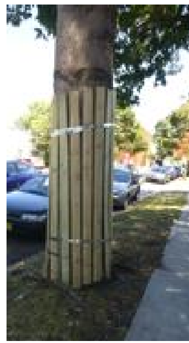
Example image of acceptable tree protection tree protection battens
