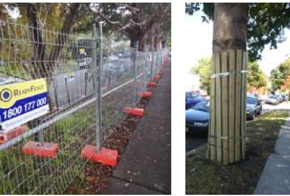
Example image of acceptable tree protection fencing measures to be applied.
