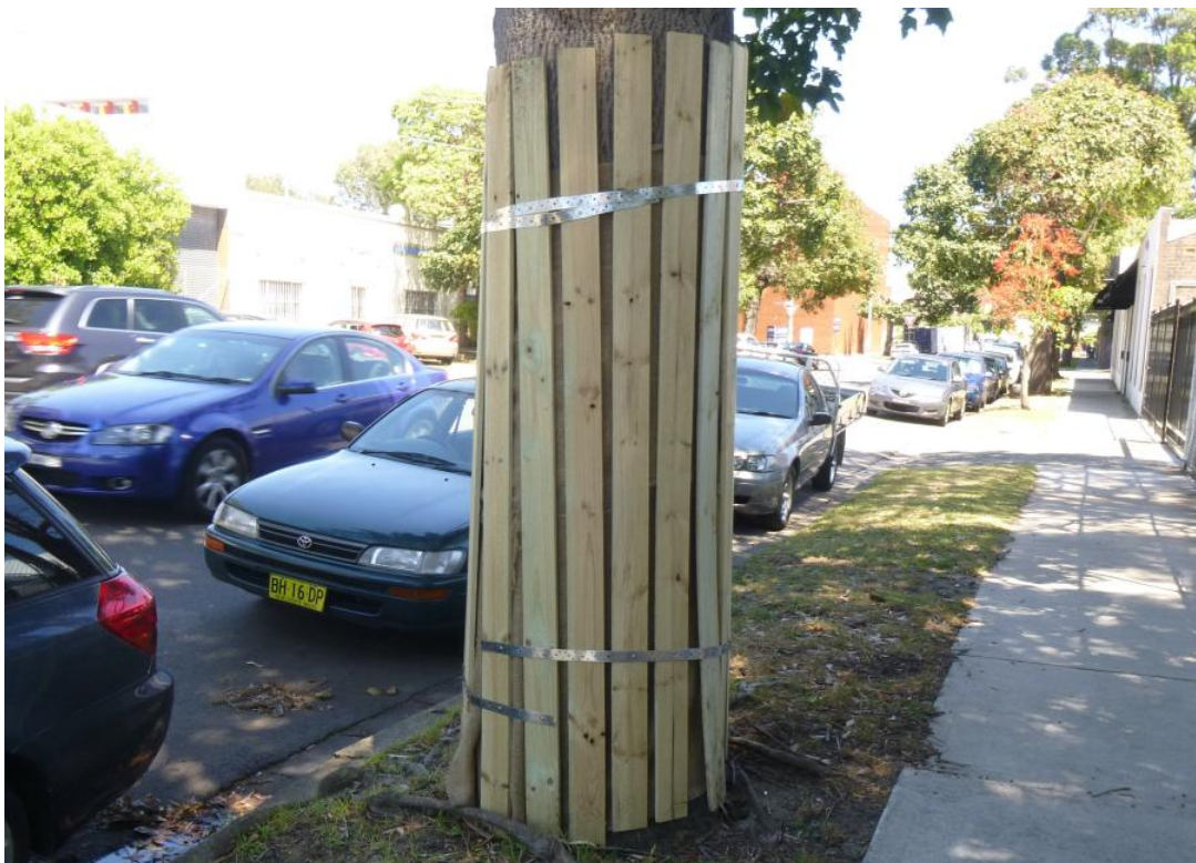
Figure 3.2 – Example of acceptable Trunk Protection batten installation. (Photo: Arterra)
