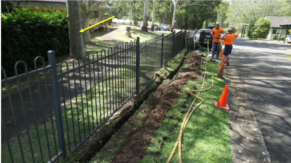
Figure 2.9 – Photo of subsurface root investigations, with trench completed. T05 arrowed at left. (Photo: Arterra 16/2/22)
