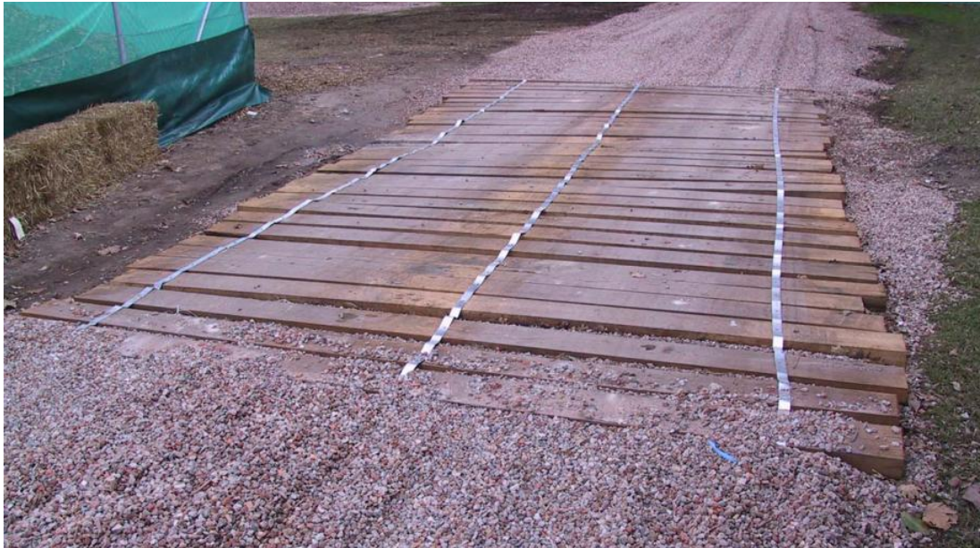
Figure 3.1 – Example of acceptable Tree Protection Area ground protection (Photo: Arterra)
