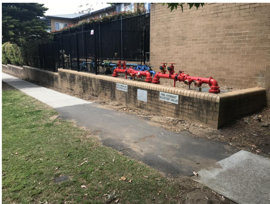
Figure 13 –Existing booster assemblies
