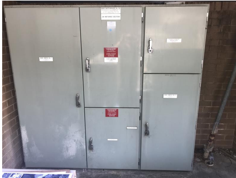
Figure 6 – Existing western main switchboard
