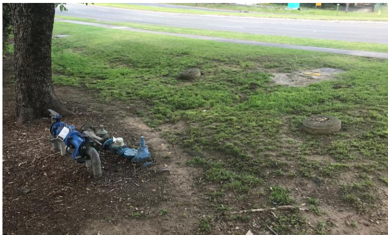
Figure 15 –Existing water meter
