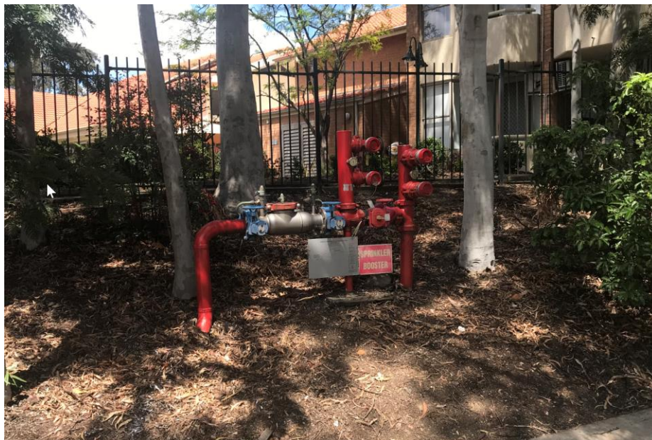
Figure 17 –Existing booster assemblies
