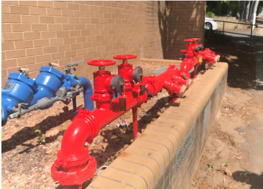
Figure 16 –Existing booster assemblies
