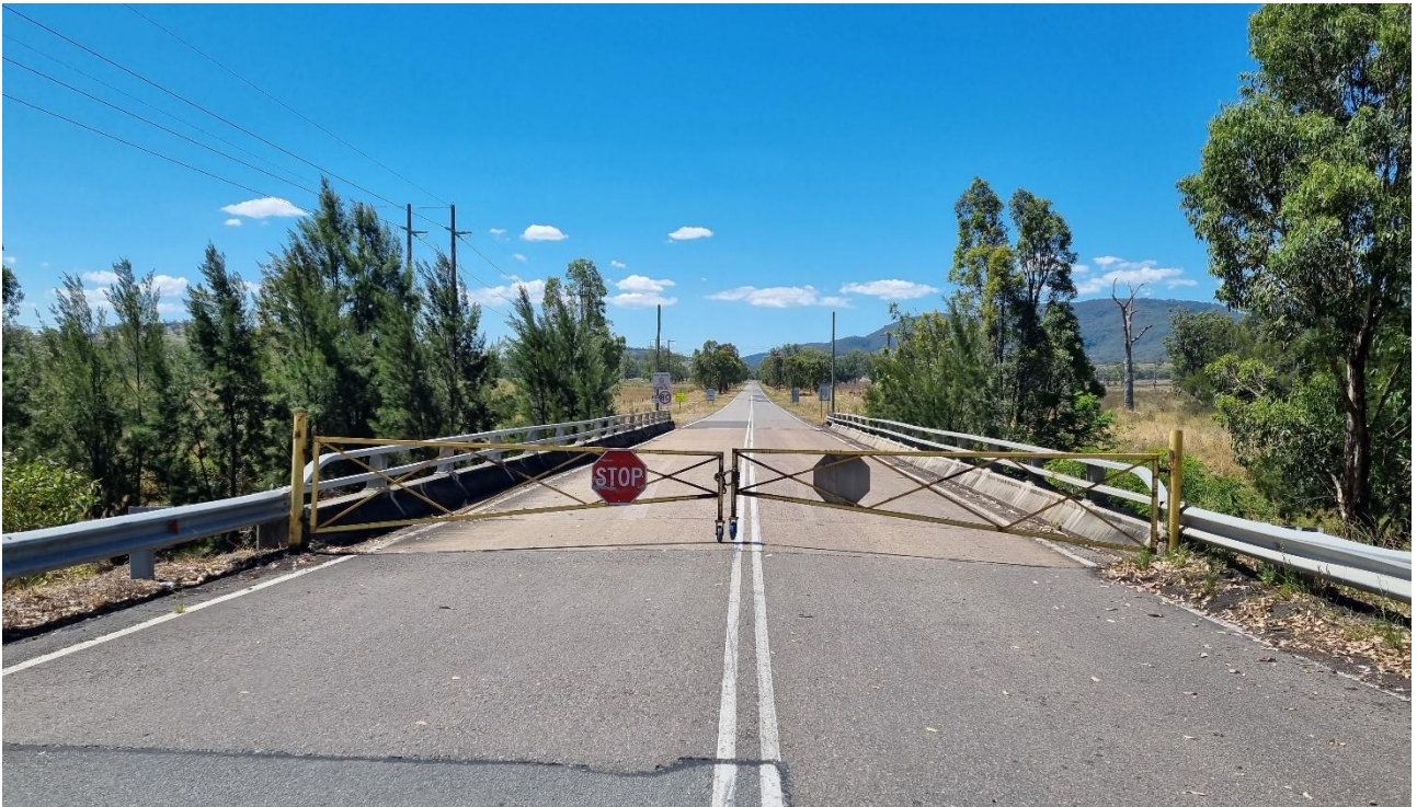
Photograph 6.1 Southern site access
