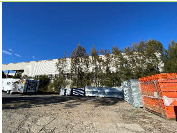
Photo plate 13: PCT 1800 viewed from the north
