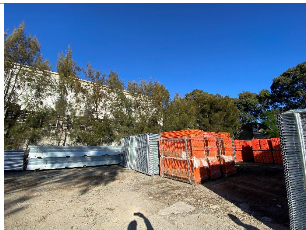
Photo plate 14: PCT 1800 viewed from the northeast
