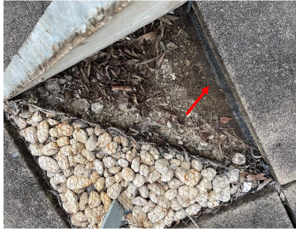
Photo 20: Roof – Assumed asbestos containing waterproofing membrane
