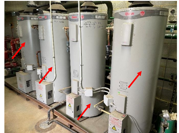
Photo 24: Roof – Assumed SMF insulation core to hot water heater
