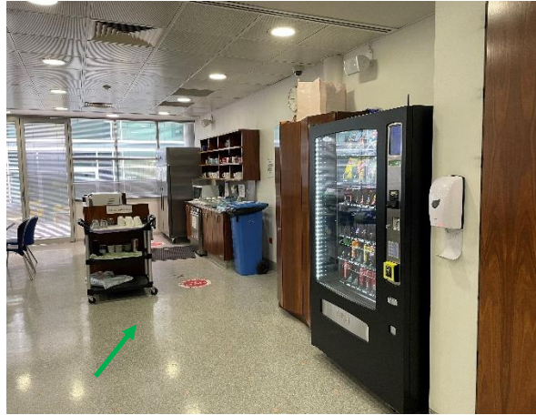
Photo 8: Non-asbestos containing light grey speckled vinyl floor
