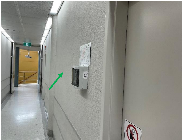
Photo 16: Level 1 – Non-asbestos containing or Lead based textured paint to the walls
