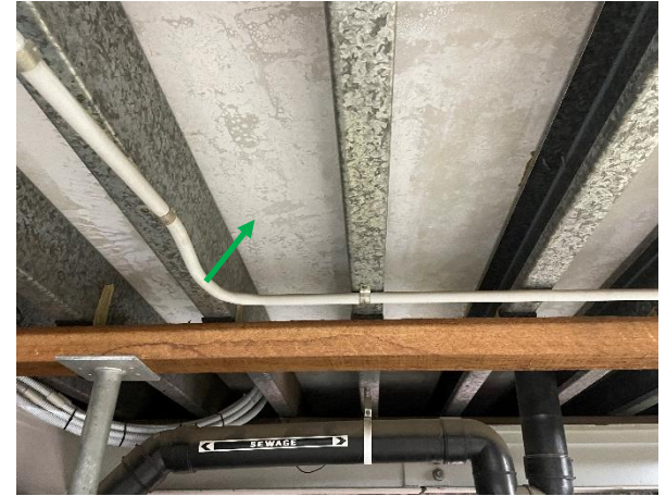
Photo 9: Basement – Non-asbestos containing compressed fibre cement to the ceiling
