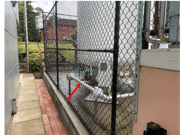
Photo 6: External – Assumed SMF insulation to nitrogen tank pipework
