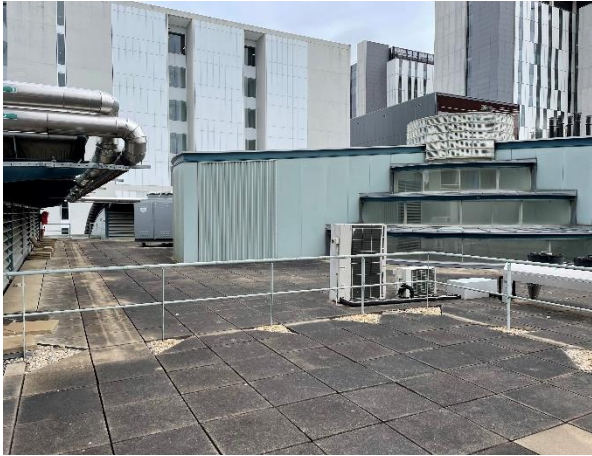
Photo 19: Overview of the roof and associated plant rooms
