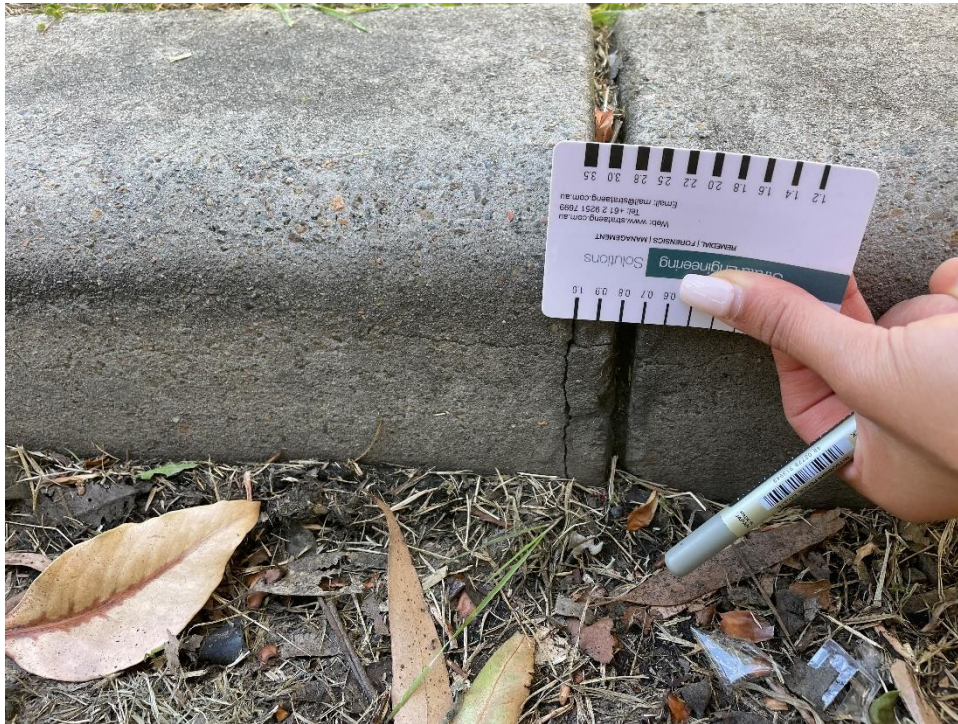
PHOTO 5 WESTERN ROAD CH 00-10m
