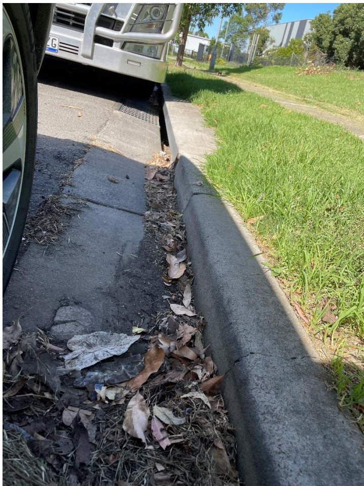
PHOTO 6 WESTERN ROAD CH 00-10m
