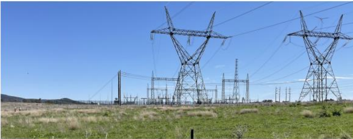
Figure 6-14 Views of the existing substation from the Development Site
