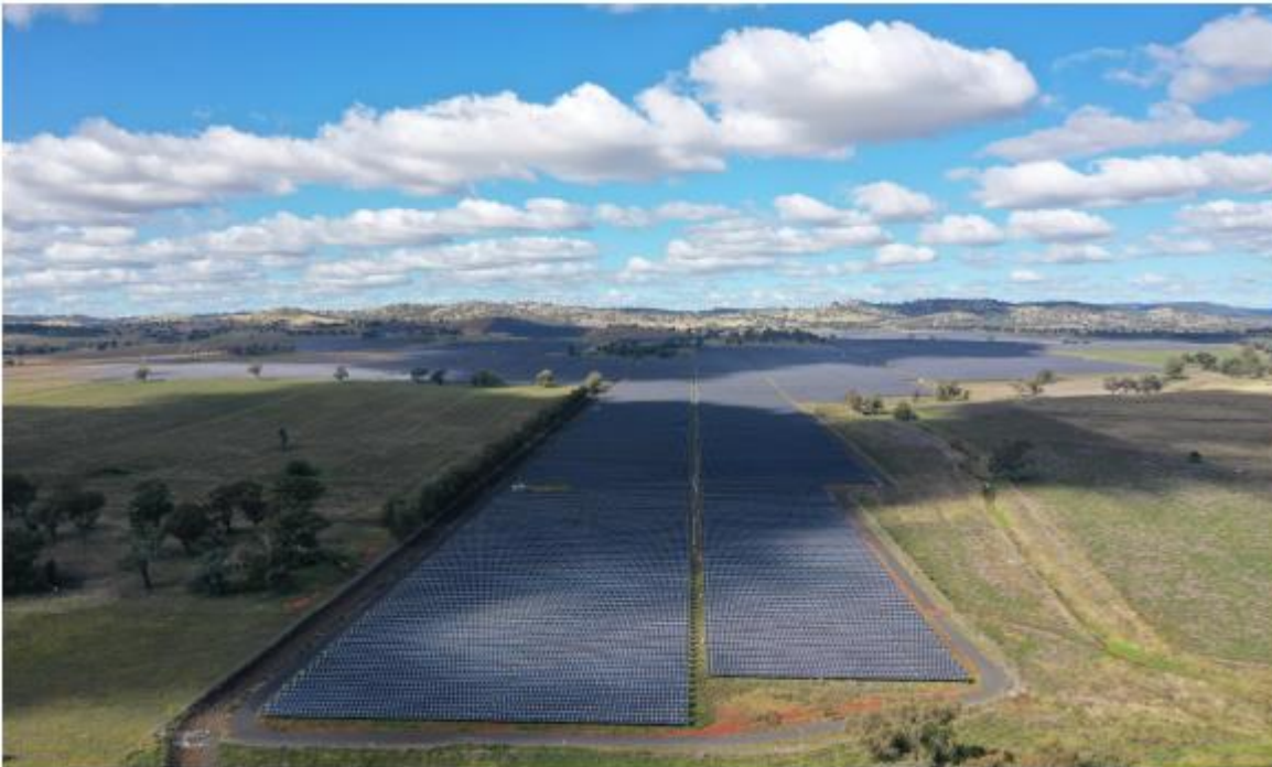
Figure 6-15 Views of Wellington Solar Farm (Source: Moir LA drone photograph)
