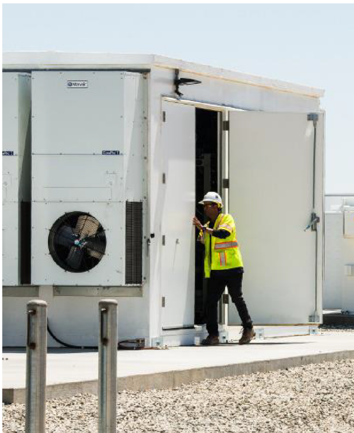
Example of a typical BESS
