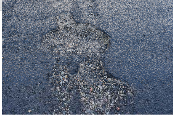
Figure 16: Imported rubble fill beneath bitumen paving
