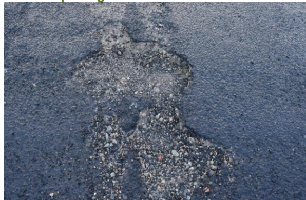
Figure 16: Imported rubble fill beneath bitumen paving
