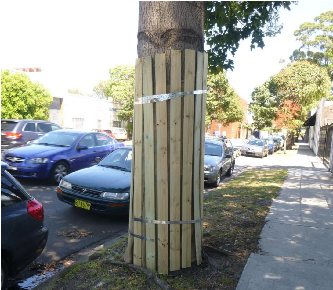
Figure 23 – Example of acceptable Trunk Protection batten installation. (Photo: Arterra)
