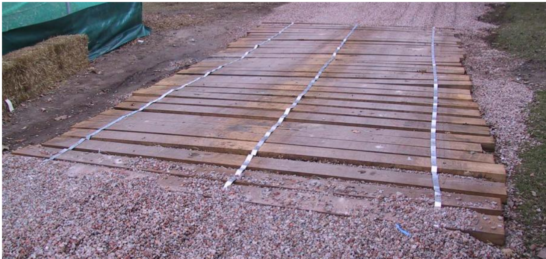
Figure 22 – Example of acceptable Tree Protection Area ground protection (Photo: Arterra)
