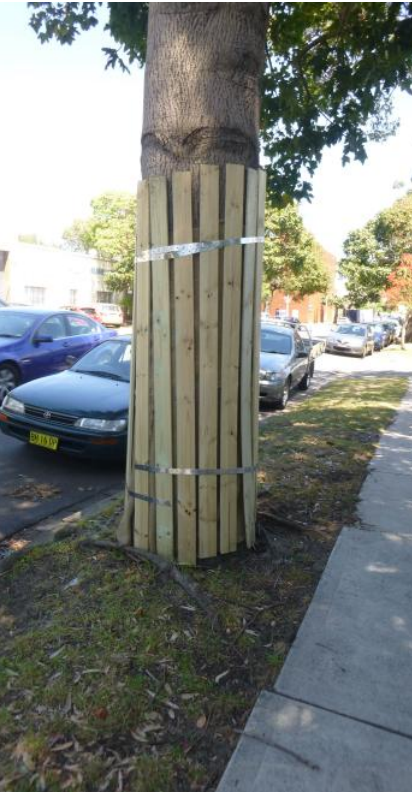
Example image of acceptable tree tree protection battens
