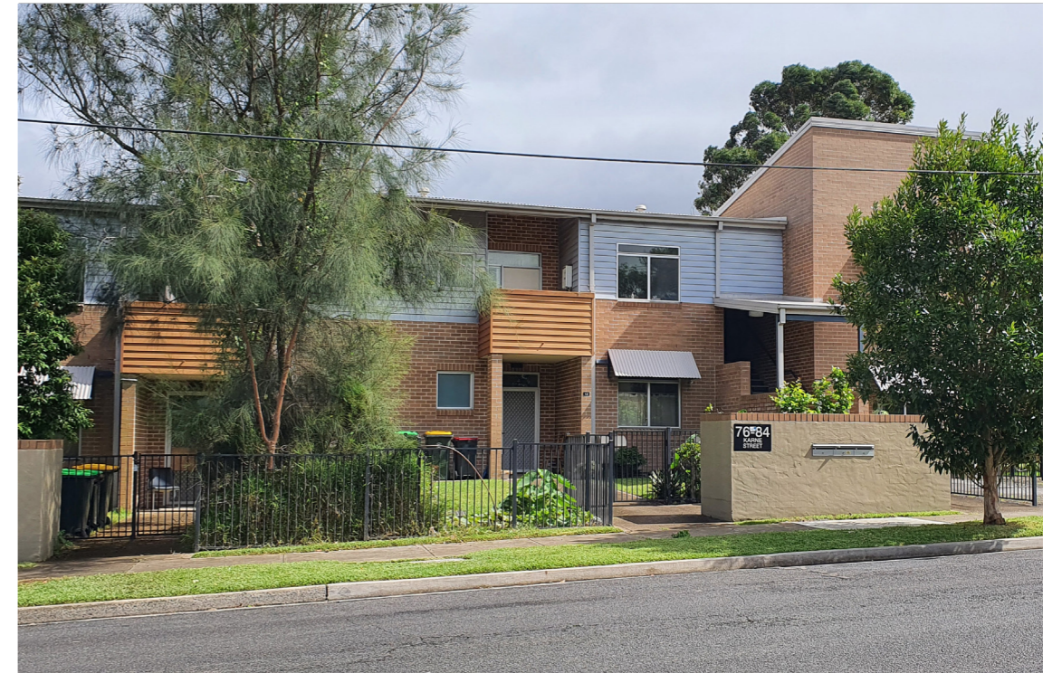
2. Residential development in the immediate proximity consists of single dwellings and medium-density multi-dwellings.
