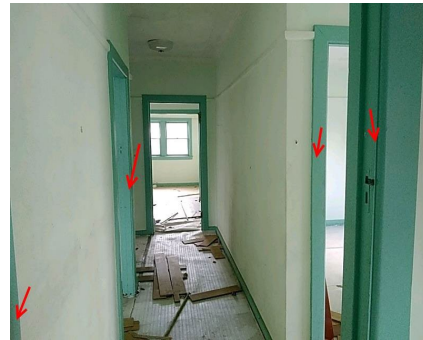
Photo No: 221107-101755 Result: Lead in Paint - Negative Location-Level: Interior - Ground Floor Room-Location: All elevation of the floor - walls Feature-Material: Lower colour paint system
