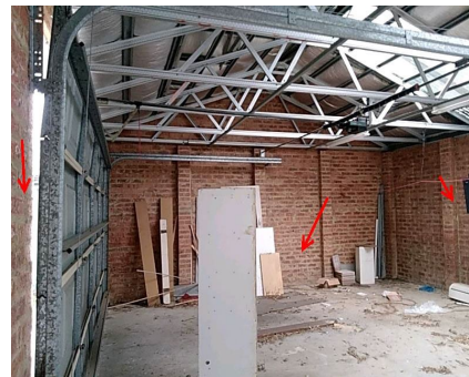
Photo No: 221107-104314 Result: Asbestos - Negative Location-Level: Interior and Exterior - Ground Floor Room-Location: All elevation of the building - walls Feature-Material: Brick
