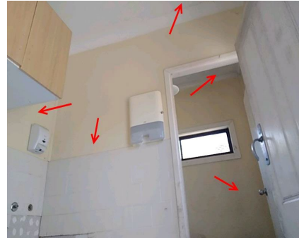
Photo No: 221107-133927 Result: Asbestos - Negative Location-Level: Interior - Ground Floor Room-Location: Laundry and toilet - internal walls and ceilings Feature-Material: FC sheeting
