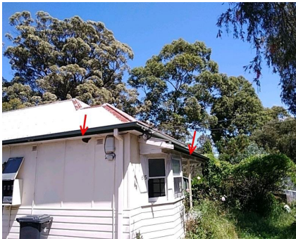
Photo No: 221107-141046 Result: Lead in Paint - Positive Location-Level: Exterior - Ground Floor Room-Location: All elevation of the building - roof Feature-Material: Lower colour paint system Item No - Risk Rating: 11 - Low
