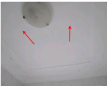
Photo No: 221107-094933 Result: Asbestos - Presumed Negative Location-Level: Interior - Ground Floor Room-Location: Kitchen - ceiling Feature-Material: Plaster-like material
