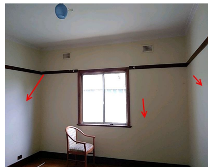
Photo No: 221107-135200 Result: Asbestos - Presumed Negative Location-Level: Interior - Ground Floor Room-Location: Western bedroom - internal walls Feature-Material: Plaster-like material
