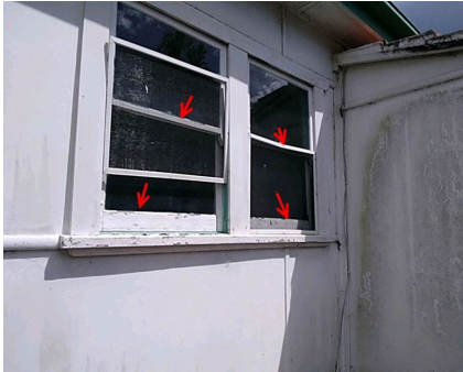
Photo No: 221107-104044 Result: Asbestos - Negative Location-Level: Exterior - Ground Floor Room-Location: All elevation of the building - windows frames sealant Feature-Material: Mastic-like material
