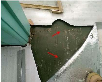
Photo No: 221107-094049 Result: Asbestos - Negative Location-Level: Interior - Ground Floor Room-Location: All elevation of the building - flooring Feature-Material: Timber
