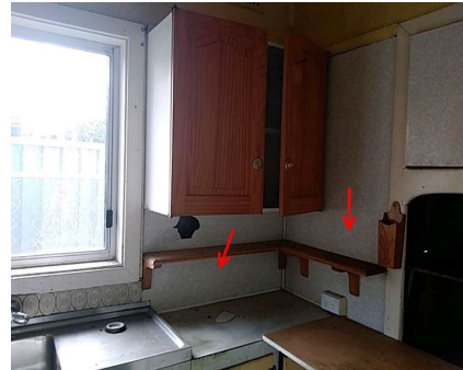
Photo No: 221107-094153 Result: Asbestos - Negative Location-Level: Interior - Ground Floor Room-Location: Kitchen - splashback Feature-Material: FC sheeting
