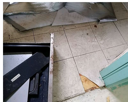
Photo No: 221107-095248 Result: Asbestos - Negative Location-Level: Interior - Ground Floor Room-Location: Kitchen - flooring Feature-Material: Vinyl tiles, backing material and adhesive
