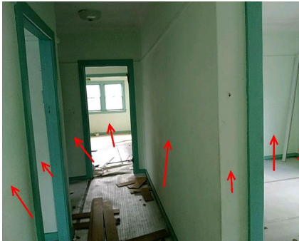
Photo No: 221107-093107 Result: Asbestos - Negative Location-Level: Interior - Ground Floor Room-Location: Northern bedroom, living area and lobby - internal walls Feature-Material: Plaster-like material
