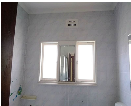
Photo No: 221107-134830 Result: Asbestos - Negative Location-Level: Interior - Ground Floor Room-Location: Bathroom - walls (behind tiles) Feature-Material: FC sheeting
