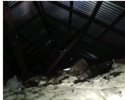
Photo No: 221107-142113 Result: Lead in Dust - Negative Location-Level: Interior - Roof Room-Location: Roof cavity - settled dust Feature-Material: Settled dust
