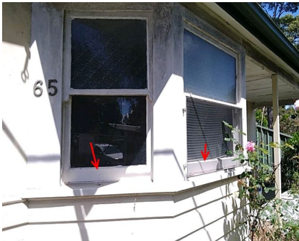
Photo No: 221107-140154 Result: Asbestos - Negative Location-Level: Exterior - Ground Floor Room-Location: All elevation of the building - windows frames sealant Feature-Material: Mastic-like material
