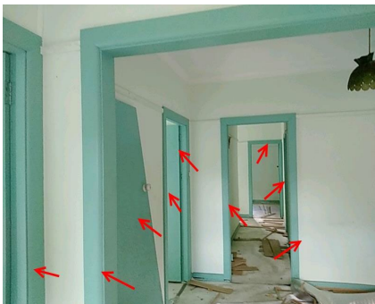
Photo No: 221107-101956 Result: Lead in Paint - Negative Location-Level: Interior - Ground Floor Room-Location: All elevation of the building - doors and door frames Feature-Material: Lower colour paint system
