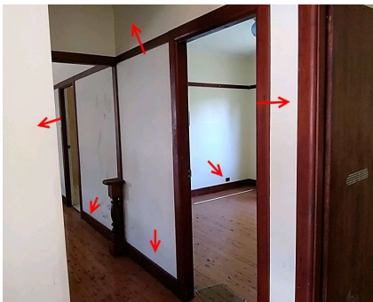
Photo No: 221107-142549 Result: Lead in Paint - Negative Location-Level: Interior - Ground Floor Room-Location: All elevation of the floor - walls and ceilings Feature-Material: Lower colour paint system
