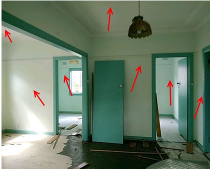
Photo No: 221107-095513 Result: Asbestos - Presumed Negative Location-Level: Interior - Ground Floor Room-Location: Dining area and southern bedrooms - internal walls and ceilings Feature-Material: Plaster-like material
