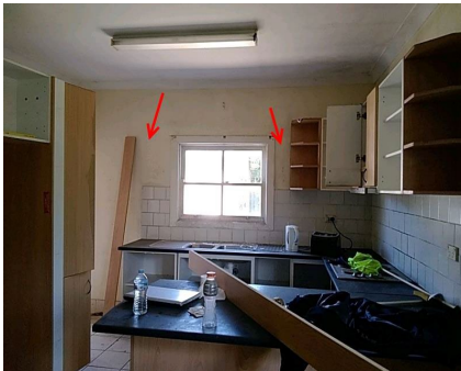
Photo No: 221107-134217 Result: Asbestos - Negative Location-Level: Interior - Ground Floor Room-Location: Kitchen - Eastern wall Feature-Material: FC sheeting
