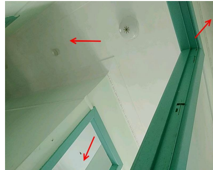
Photo No: 221107-093712 Result: Asbestos - Presumed Negative Location-Level: Interior - Ground Floor Room-Location: Northern bedroom, living area and lobby - ceilings Feature-Material: Plaster-like material
