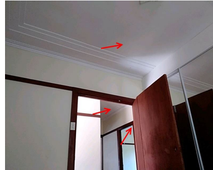
Photo No: 221107-135250 Result: Asbestos - Presumed Negative Location-Level: Interior - Ground Floor Room-Location: Bedrooms and lobby - ceilings Feature-Material: Plaster-like material
