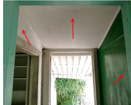
Photo No: 221107-095625 Result: Asbestos - Presumed Negative Location-Level: Interior - Ground Floor Room-Location: Rear entrance - internal walls and ceiling Feature-Material: FC sheeting
