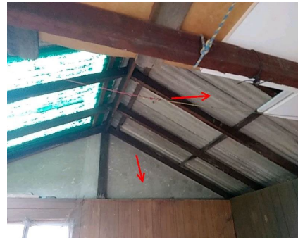
Photo No: 221107-103727 Result: Asbestos - Presumed Positive Location-Level: Exterior - Ground Floor Room-Location: All elevation of the garage - gable Feature-Material: FC sheeting Item No - Risk Rating: 1 - Low
