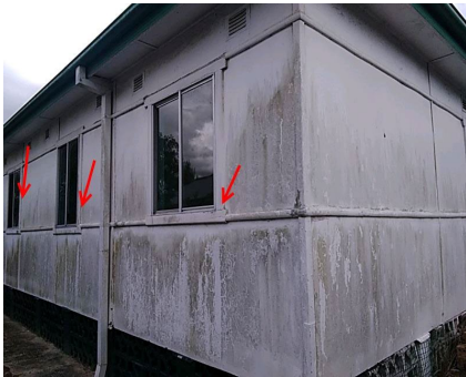
Photo No: 221107-101517 Result: Lead in Paint - Negative Location-Level: Exterior - Ground Floor Room-Location: All elevation of the building - windows frames Feature-Material: Lower colour paint system
