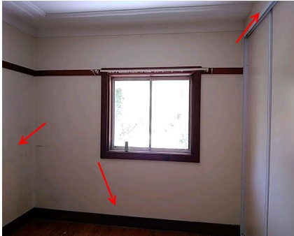
Photo No: 221107-135213 Result: Asbestos - Presumed Negative Location-Level: Interior - Ground Floor Room-Location: Southern bedroom - internal walls Feature-Material: Plaster-like material
