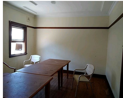
Photo No: 221107-134817 Result: Asbestos - Presumed Negative Location-Level: Interior - Ground Floor Room-Location: Dining area and living area - internal walls and ceiling Feature-Material: Plaster-like material
