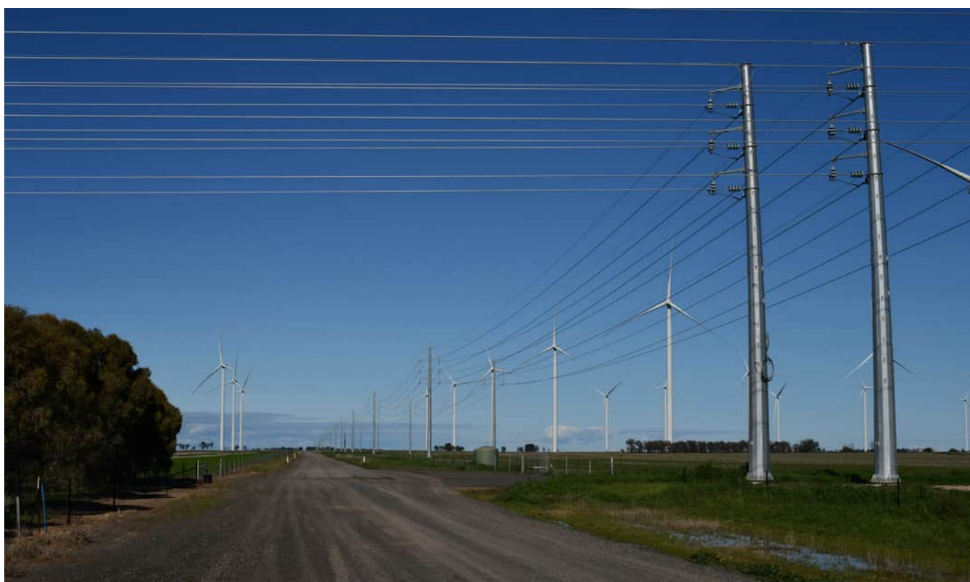
Plate 11 – Internal access road at Murra Warra Wind Farm VIC (Image: ©GBD Pty Ltd 2022)
