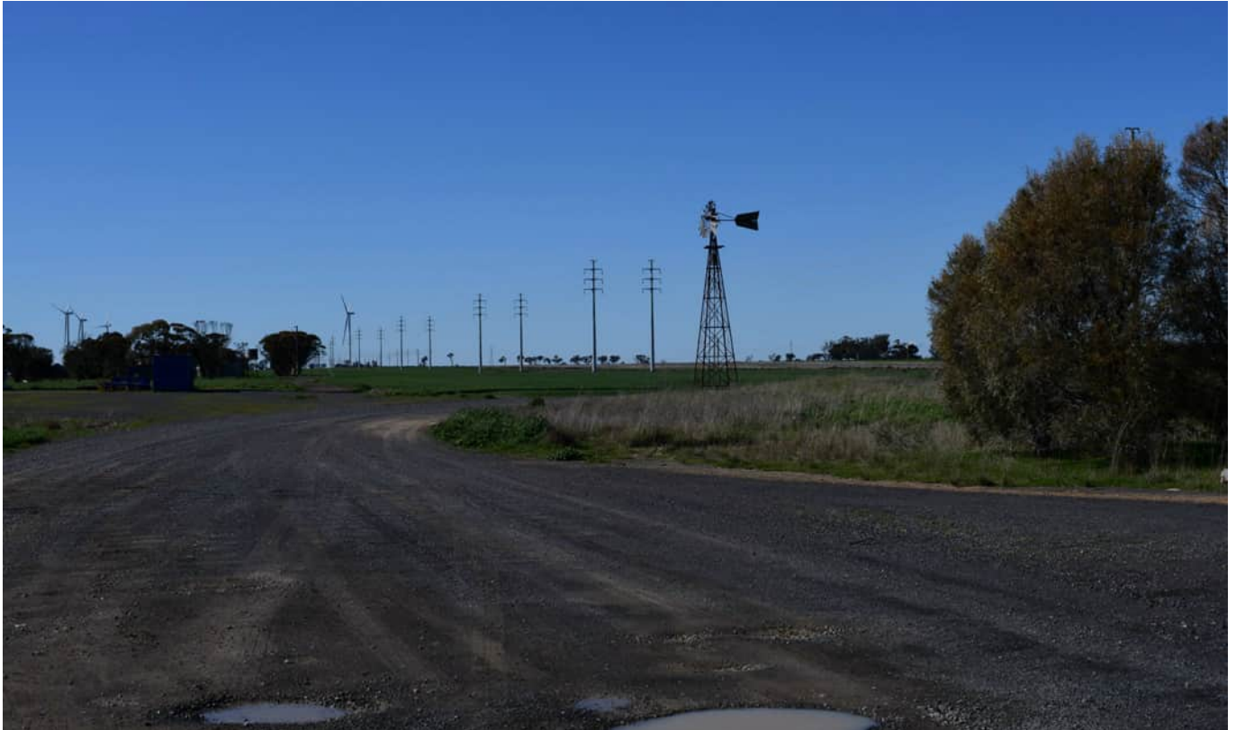
Plate 12 – 330kV transmission line structure at Murra Warra Wind Farm VIC (Image: ©GBD Pty Ltd 2022)
