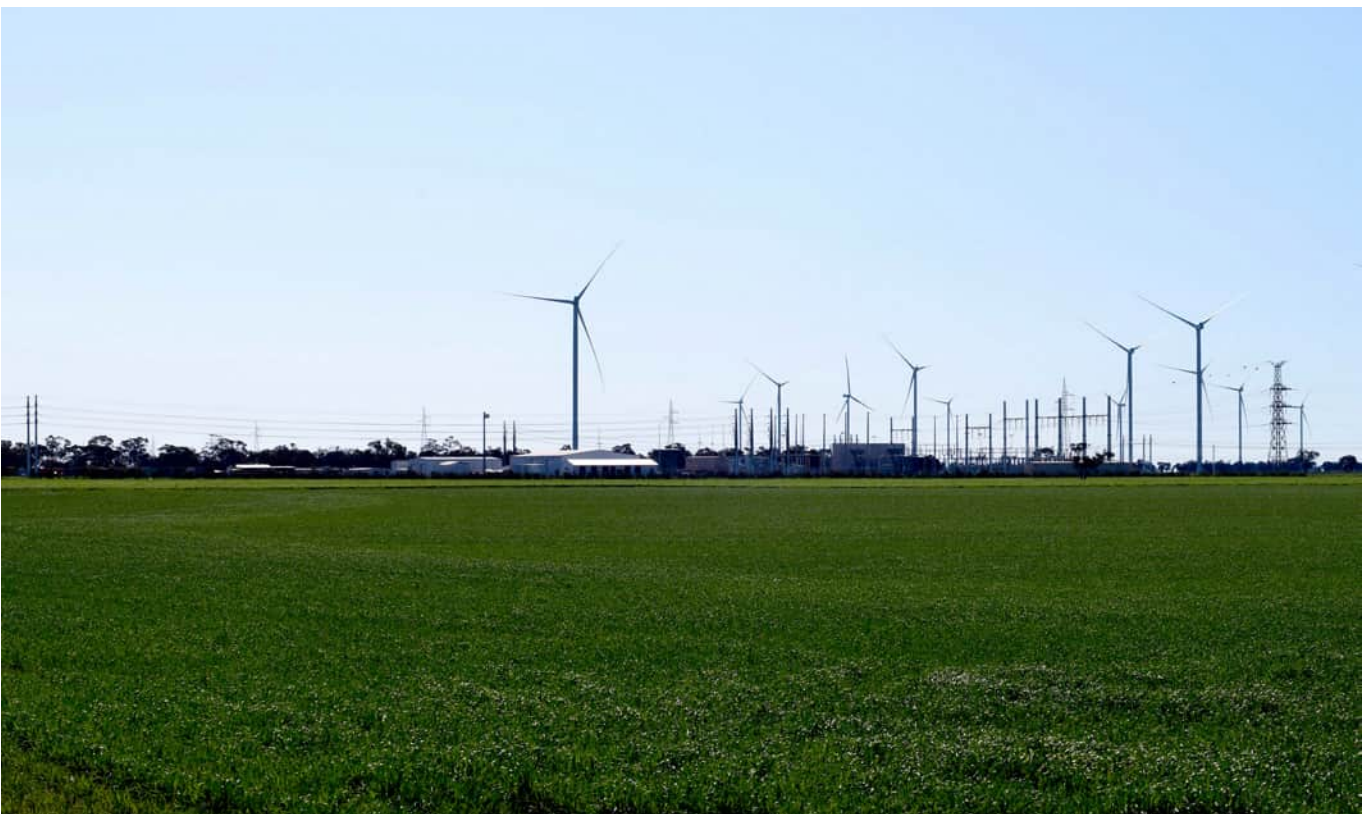
Plate 3 – Typical O&M/substation facility, Murra Warra Wind Farm VIC (Image: ©GBD Pty Ltd 2022)
