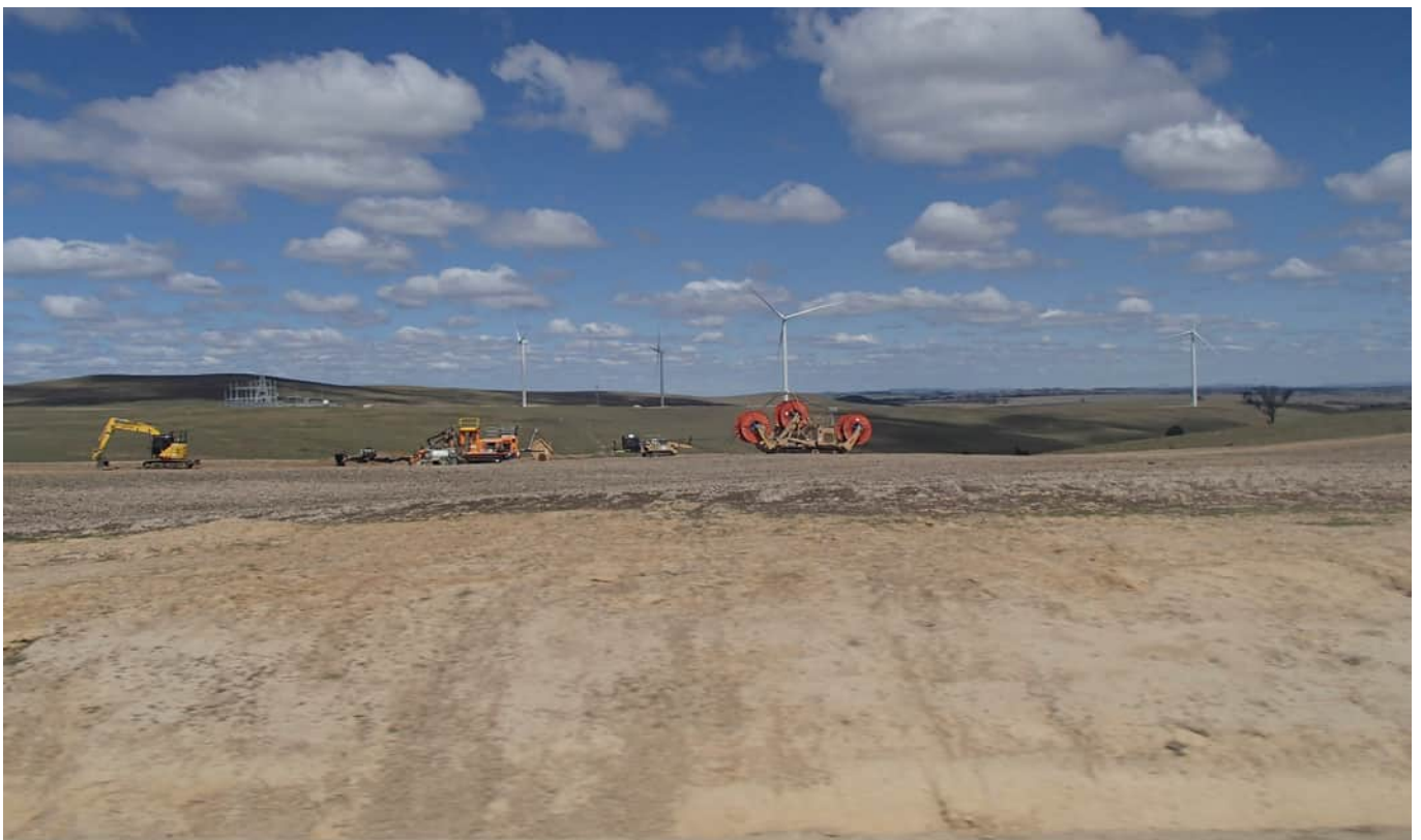
Plate 9 – Cable laying, Crookwell 2 Wind Farm NSW (Image: ©GBD Pty Ltd 2018)
