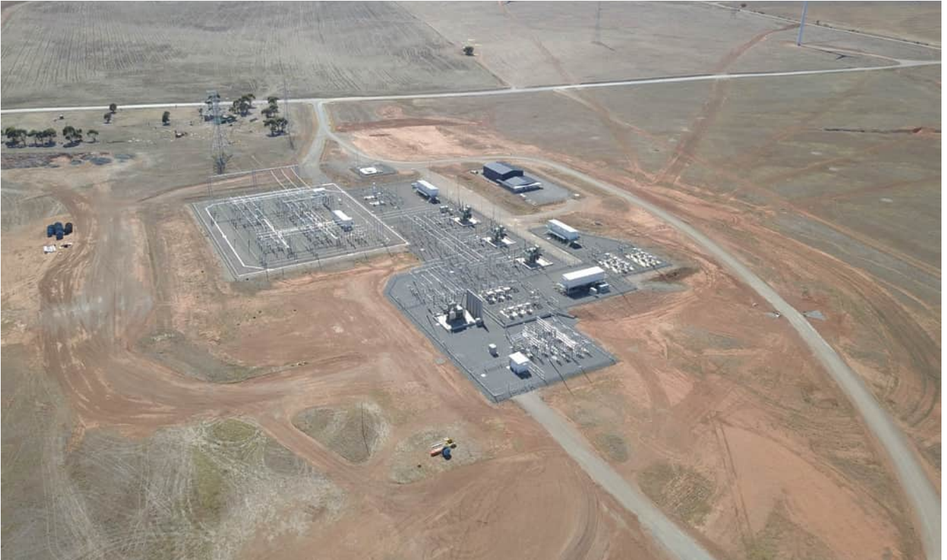
Plate 2 – Typical substation facility, Hornsdale SA (Image: ©GBD Pty Ltd 2018)
