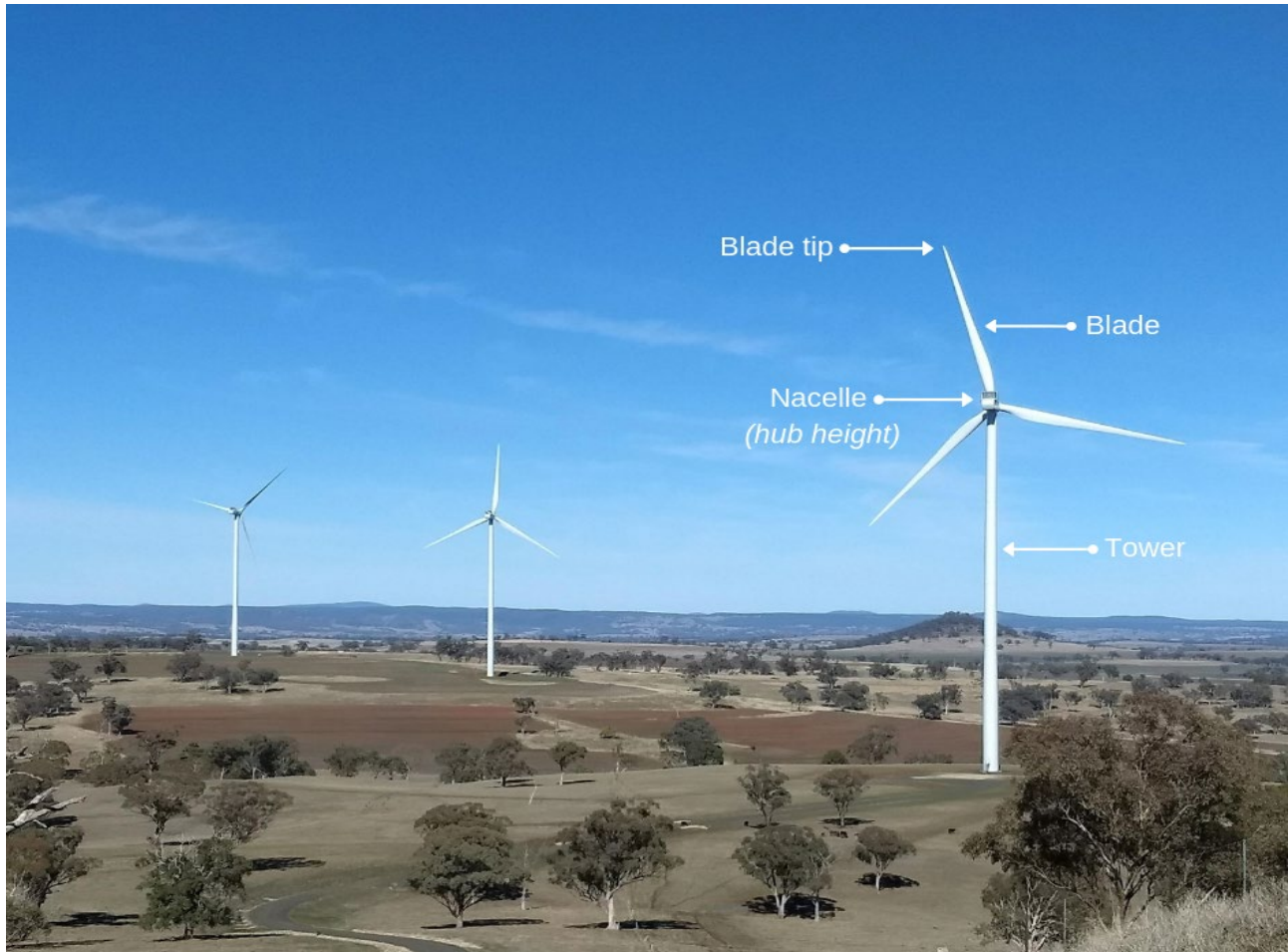
Figure 3.2 Example Components of a WTG (Sapphire Wind Farm)
