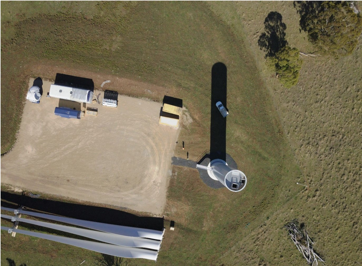
Figure 3.7 Hardstand, tower footing and blade laydown area (Sapphire Wind Farm)
