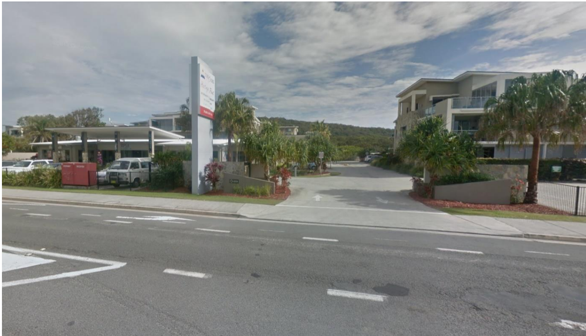
Figure 2-12 | Site view from Tweed Coast Road (south of site facing north)
