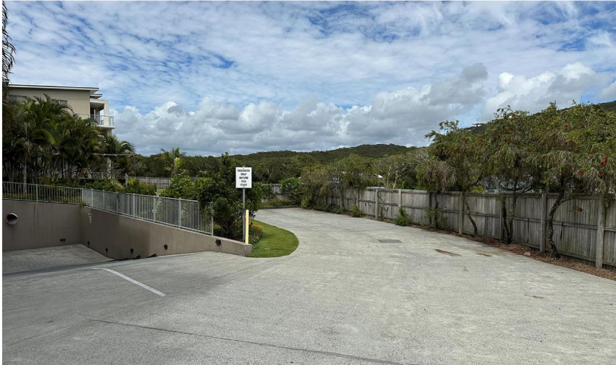
Figure 2-11 | Existing Accessway to Future Development Services (Source: TriCare)
