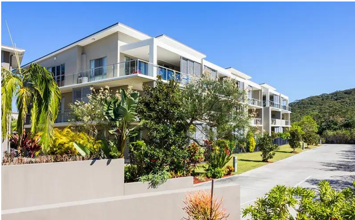
Figure 2-9 | Existing Seniors Housing Built Form (Source: TriCare)
