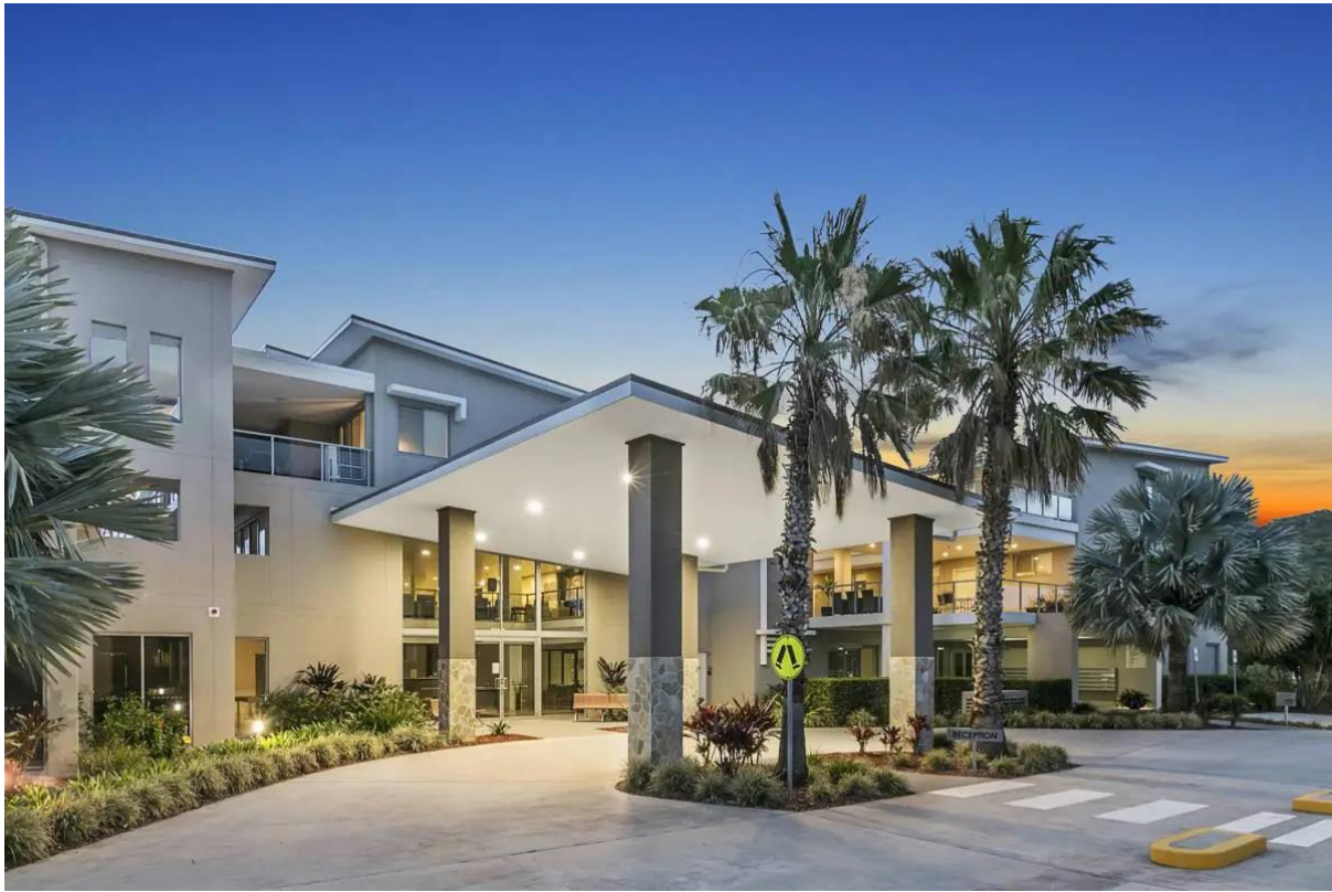
Figure 2-10 | Existing Building Entry (Source: TriCare)
