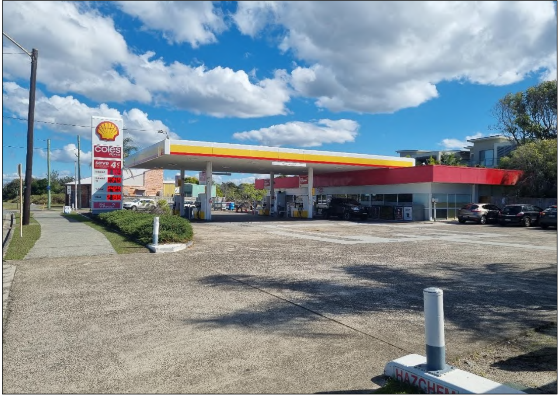
Photo 1: Image of the service station site located to the south east of the IA.
