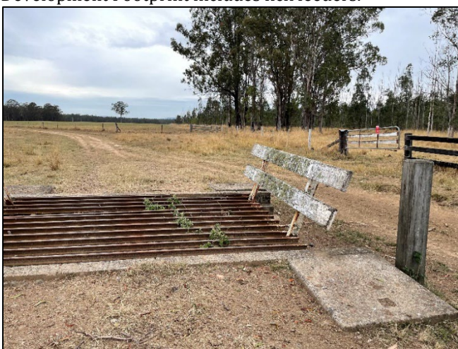
Plate 9: Agricultural infrastructure within the Development Footprint includes cattle grids.
