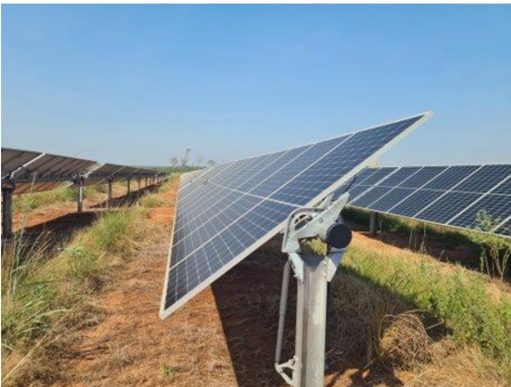
Photo 3.2 Example of typical single axis tracking system (Ark Energy, 2023)
