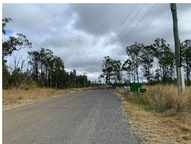
Photo 4.10 Road Upgrade Area, Main Camp Road
