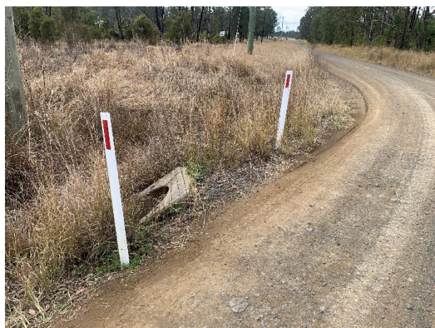
Photo 4.12 Example of concrete culvert on Main Camp Road and Avenue Road
