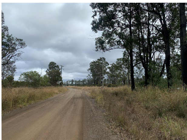
Photo 4.11 Avenue Road, near junction with Main Camp Road
