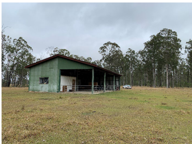
Photo 4.7 Shed located in the north of the Project Area
