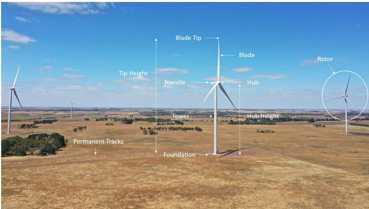
**Figure 3-2: Wind Turbine Generators installed at Stockyard Hill wind farm in Western Victoria**
