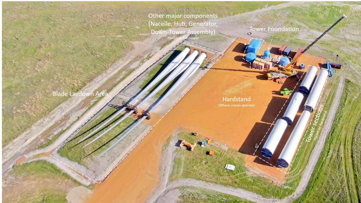
Figure 3-3: Hardstand with a blade laydown area (Esperance Wind Farm July 2021)
