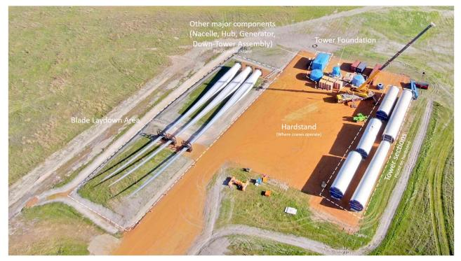
Figure 3-3: Hardstand with a blade laydown area (Esperance Wind Farm July 2021)
