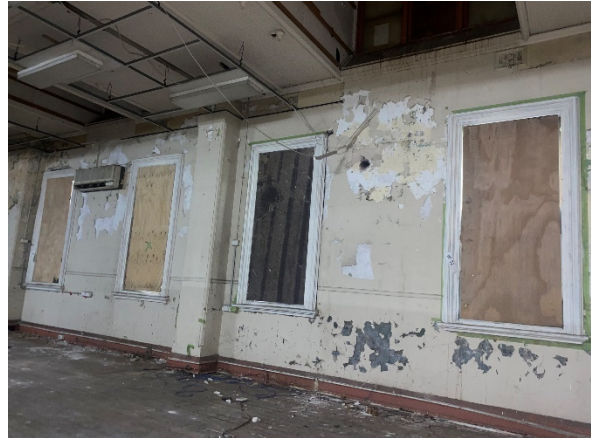
Figure 4.99: Paintwork peeling in Room F6
