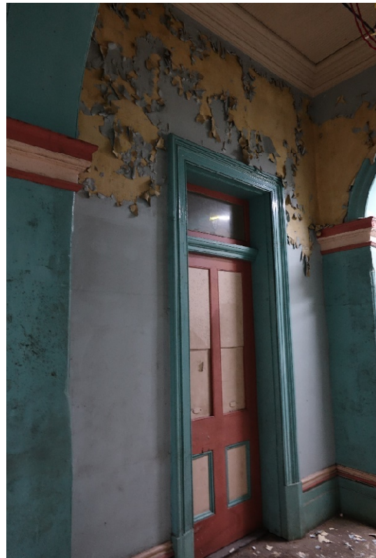
Figure 4.95: Paintwork peeling in Room G3C
