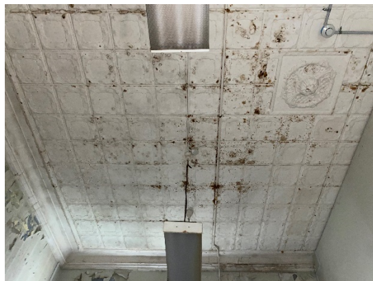
Figure 4.32: Pressed Metal Ceiling with ceiling rose visible (Room G21A.)
