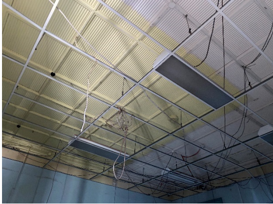
Figure 4.33: Corrugated Iron Ceilings with suspended T-Bar system (Room G5)
