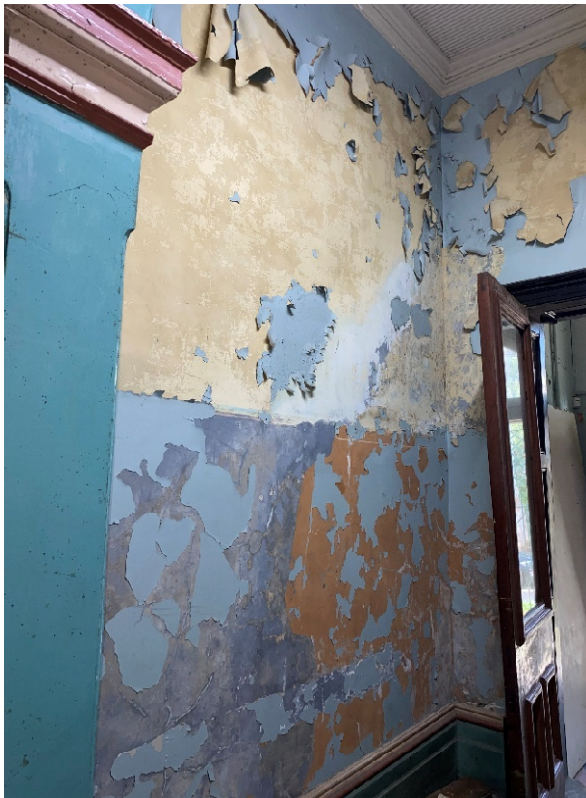
Figure 4.94: Paintwork peel and exposing previous paint colours in Room G3B
