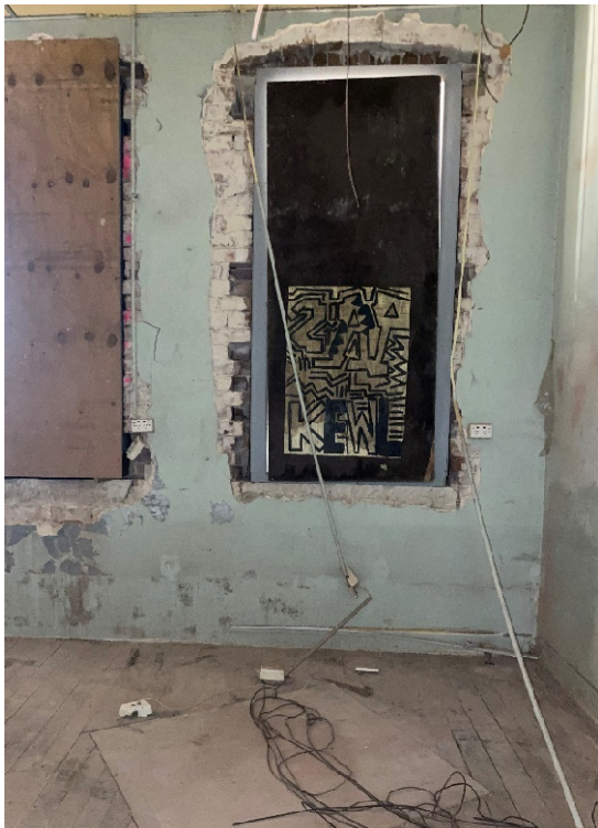
Figure 4.78: RoomG5 with no architraves surrounding window
