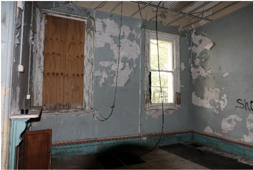
Figure 4.81: Architraves surrounding windows in Room G13
