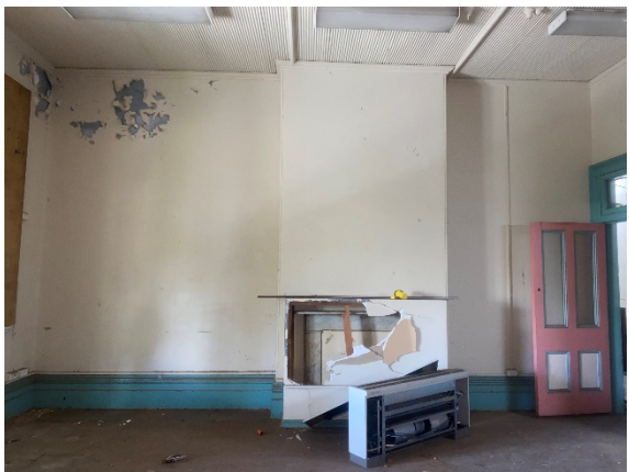
Figure 4.92: Fireplace partially exposed. Half boarded up with marble mantel and surrounds intact within 1887 phase of construction of CME Building (Room F1)
