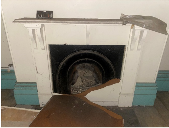
Figure 4.82: Timber mantle and surround of fireplace from the 1887 construction of CME Building (Room F2)
