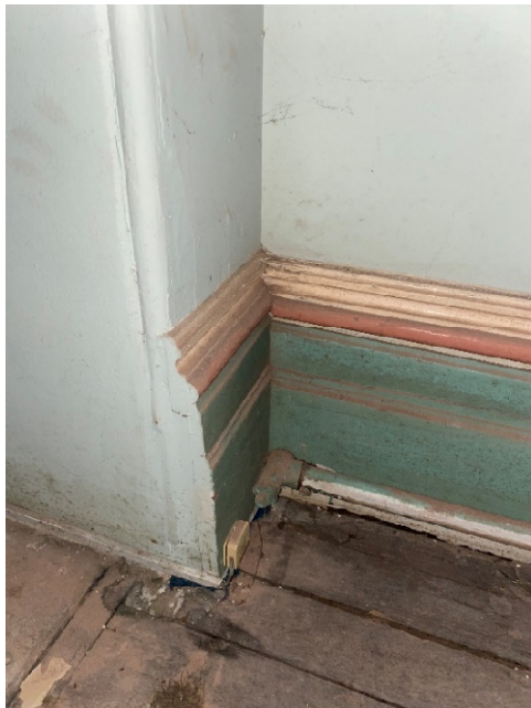
Figure 4.71: Skirting cut off around fireplace (Room G5)
