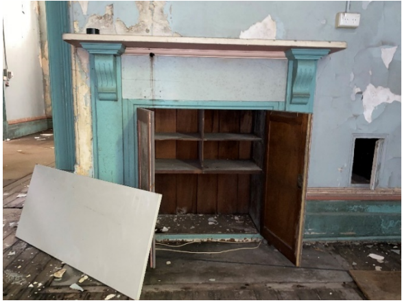
Figure 4.89: Fireplace with mantel and surrounds intact and firebox converted to a cupboard. Located within 1920s section of the CME Building (Room G13)
