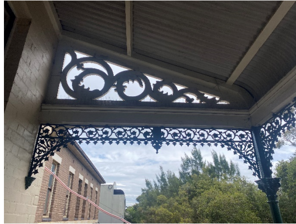
Figure 4.119: The exposed ironwork of the western end of the balcony (Room F16) as part of the 1887 construction of the CME Building with the Scientific Services Building visible in the background
