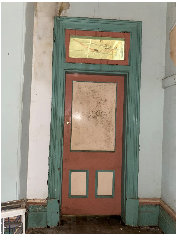
Figure 4.77: Architraves surrounding door and fanlight in Room G14,15,16
