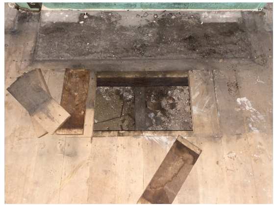
Figure 4.22: Square service floor cut (Room G4)
