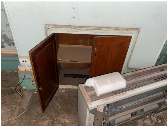
Figure 4.90: Fireplace with mantel and surrounds removed and firebox converted to a cupboard. Located within 1920s section of the CME Building (Room G16)
