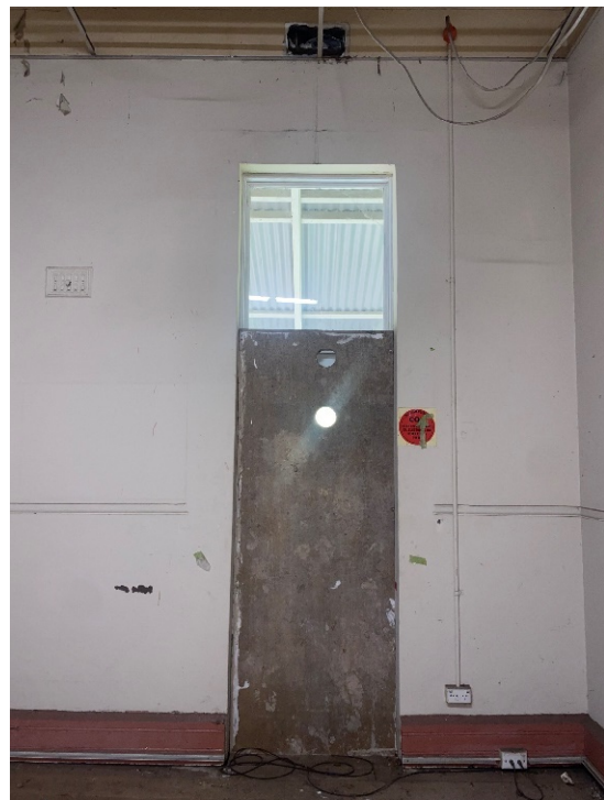
Figure 4.57: Room F6, doorway boarded up internally
