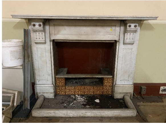
Figure 4.83: Fireplace with marble mantle and surround within CME Office (Room G10)
