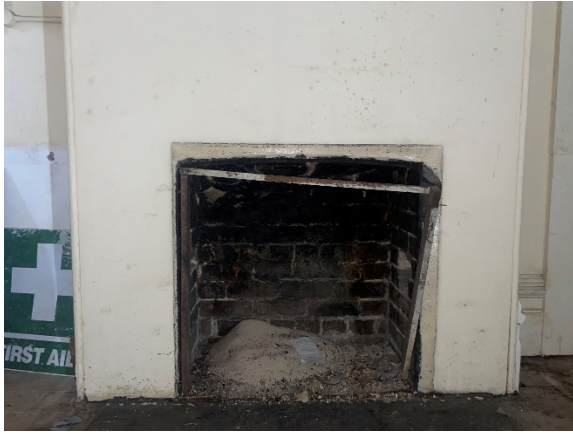
Figure 4.88 : Fireplace previously boarded up and mantel and surrounds removed located within original 1887 phase of construction of the CME Building (Room G1)
