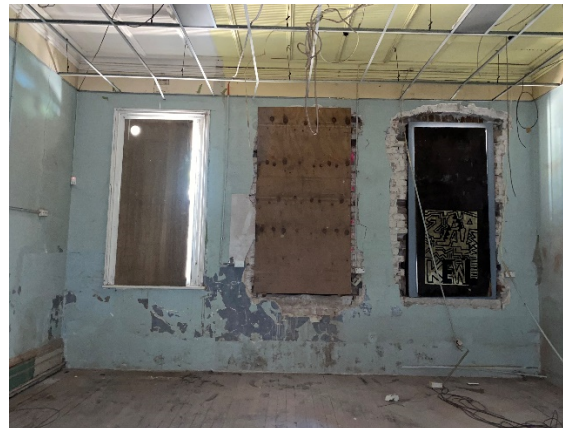
Figure 4.62: Northern wall of Room G5. Previously bricked up windows (two windows on the east) were unbricked during the 2016 Urban Growth work
