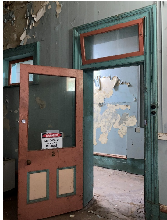
Figure 4.53: Room G12 doorway showing upper panel glazing and fanlight above
