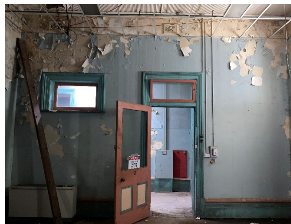
Figure 4.95: Paintwork peeling in Room G3C
