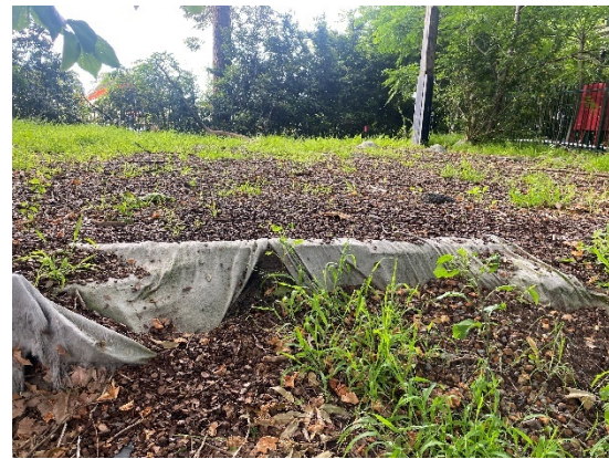
Figure 4.142: Area of eastern garden with geo-fabric, suggest previous inground works, within the eastern garden area
