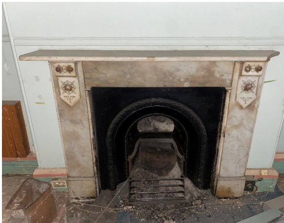
Figure 4.84: Fireplace with marble mantle and surround within 1900 addition section of CME Building (Room G6)
