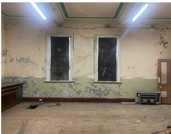
Figure 4.94: Paintwork peel and exposing previous paint colours in Room G3B
