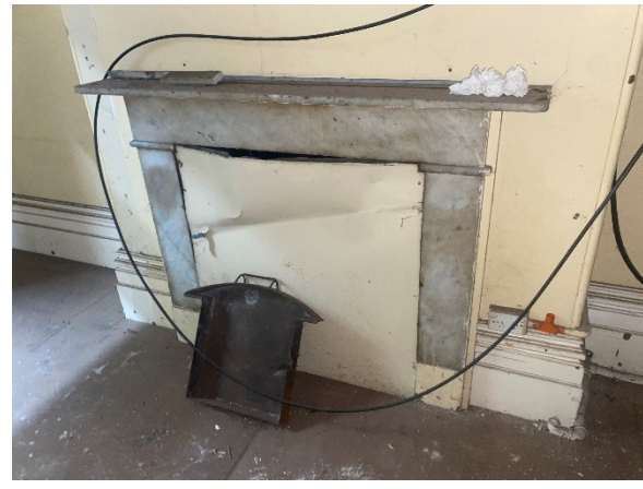
Figure 4.87 : Fireplace boarded up with marble surrounds from original 1887 phase of construction (Room F5A)
