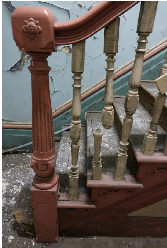
Figure 4.104: Ground floor remaining bannisters in poor condition with newel post in view.
