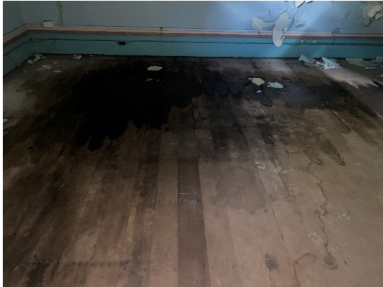
Figure 4.19: Water damage (Room F8)
