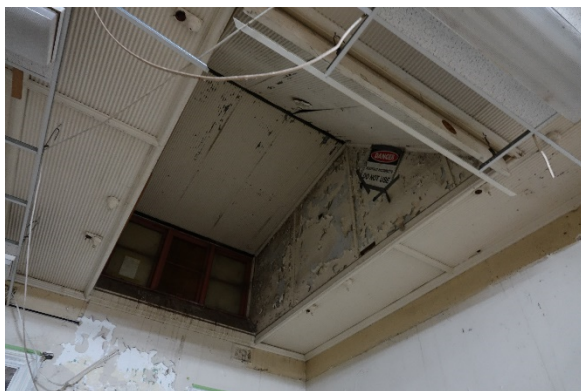
Figure 4.63: One of three skylights located within the 1920s addition area of Room F6 CME Building, boarded up,
