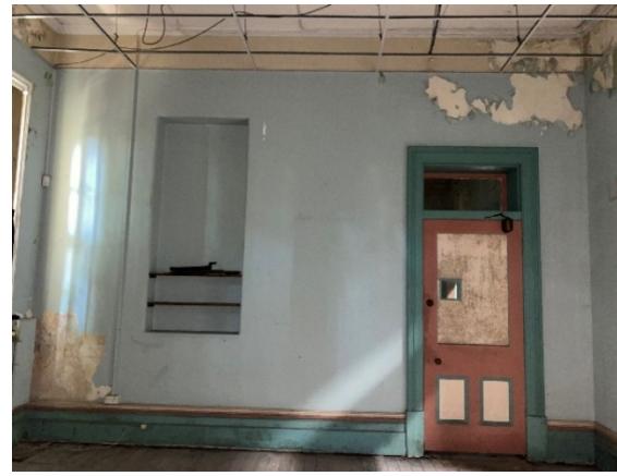
Figure 4.66: Western wall of Room G14 with bricked-in side of the original 1887 window visible
