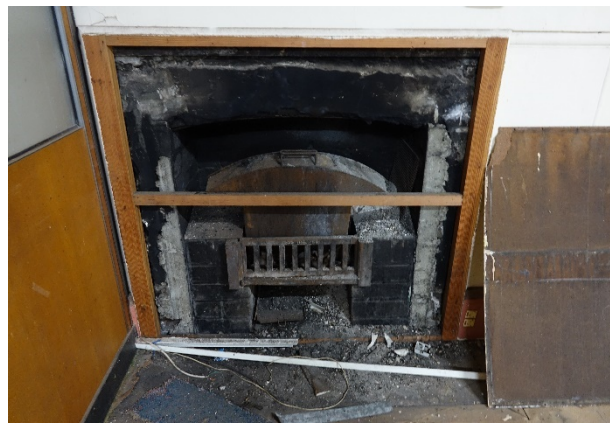
Figure 4.93: Fireplace with mantel and surrounds removed and firebox and grate still intact (Room F6)
