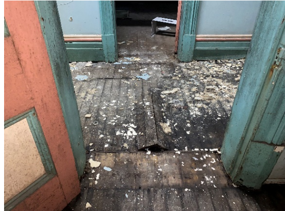
Figure 4.20: Raised floorboards due to water damage (Room G5)
