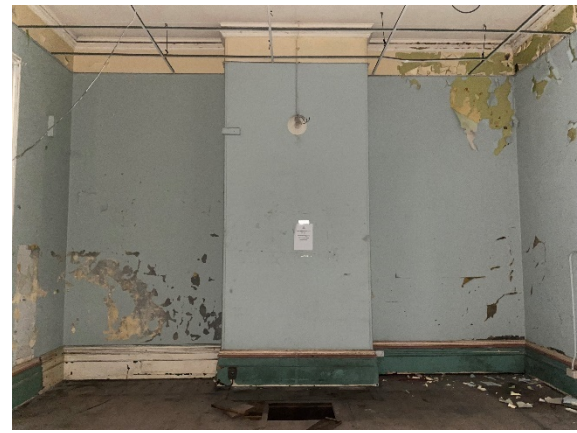
Figure 4.91: Fireplace bricked-in and marble/ surrounds removed within 1887 phase of the CME Building (Room G4)
