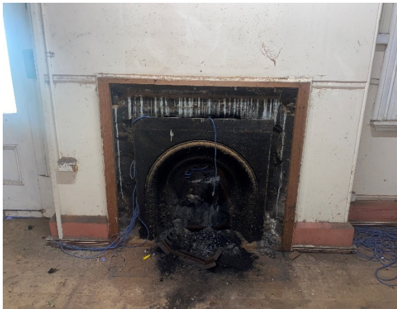
Figure 4.86: Damaged fireplace with mantle and surrounds removed (Room F6)
