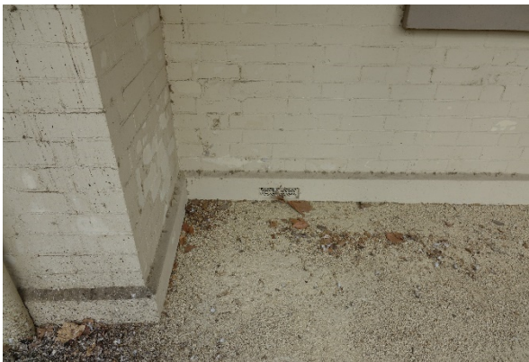
Figure 4.124: Brick Vent exposed
