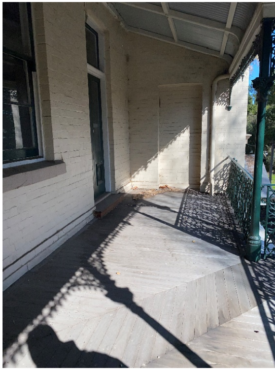
Figure 4.56: Room F17, bricked in doorway to Room F3B visible
