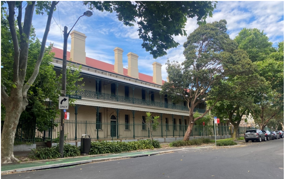
Figure 4.126: View of the northern façade of the CME Building from Wilson Street showing four remaining chimneys which were added during the 1900 addition works.
