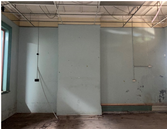
Figure 4.75: Majority of skirting in Room G5 has been previously removed.
