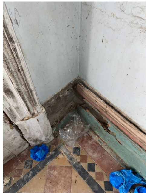
Figure 4.72: Termite Damage to skirting (Room G3A)
