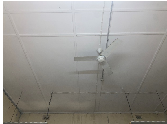
Figure 4.36: Masonite ceiling covering the timber tongue and groove ceiling (Room G1)
