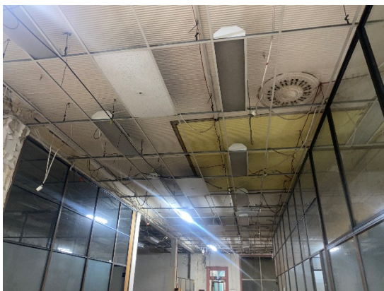
Figure 4.37: Corrugated Iron ceiling with ceiling rose visible and suspended T-Bar system (Room F6)
