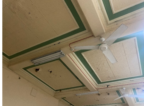
Figure 4.34: Pressed Metal Ceiling in CME Office (Room G10,)
