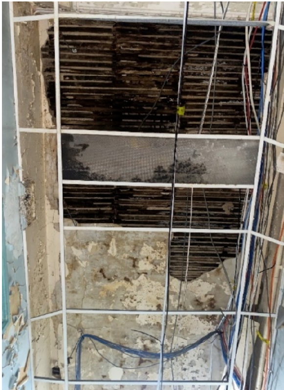
Figure 4.41: Damaged corrugated iron ceiling with suspended T-Bar system (Room G25)
