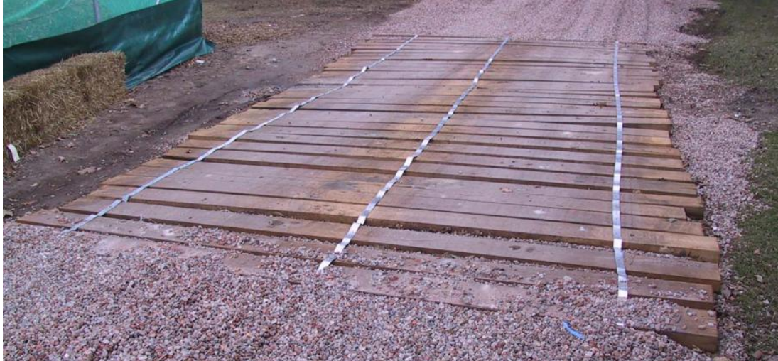
Figure 18 – Example of acceptable Tree Protection Area ground protection. (Photo: Arterra)
