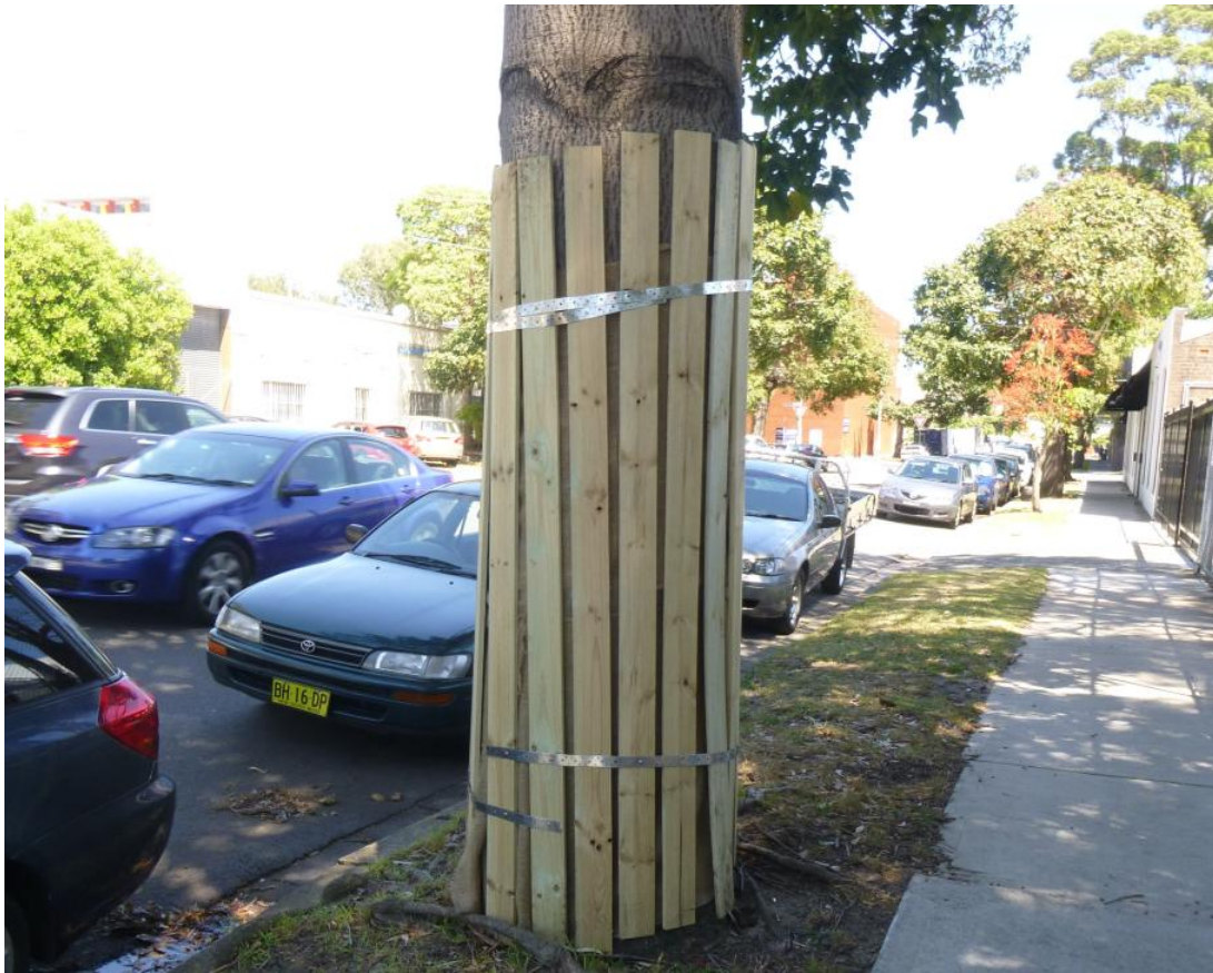
Figure 19 – Example of acceptable Trunk Protection batten installation. (Photo: Arterra)
