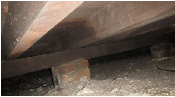
Figure 3.16: Detail of underfloor. (Source: Timber Inspection 2017)
