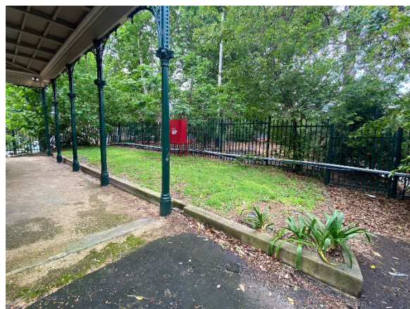
Figure 3.17: Northern view of security fence between the CME Building and gardens
