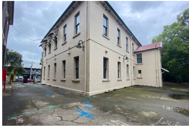
Figure 3.6: CME Exterior view north of the southern and western building façades
