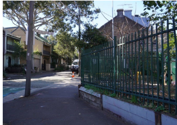
Figure 3.12: The north-eastern corner of the Paint Shop Sub-Precinct at the corner of Wilson and Eveleigh Streets, view north
