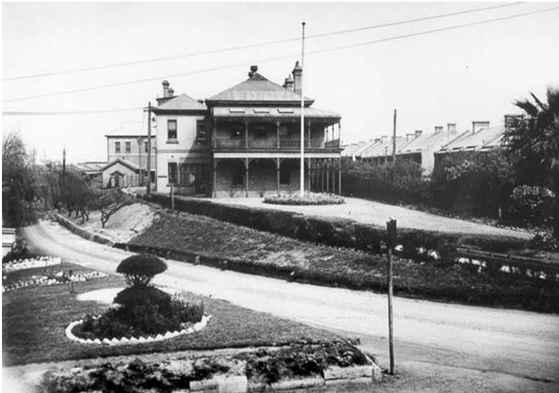
Figure 2.11: Eastern elevation – CME Building, entrance driveway and gardens c.1950 Source: Rappaport 1997
