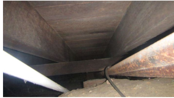
Figure 3.18: Detail of underfloor. (Source: Timber Inspection 2017)
