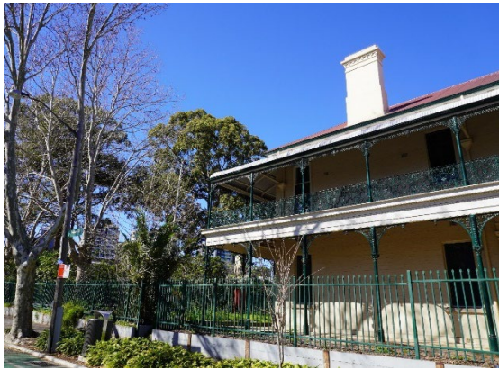
Figure 3.5: View southeast of the northern façade and verandah of the CME Building along Wilson Street and CME gardens
