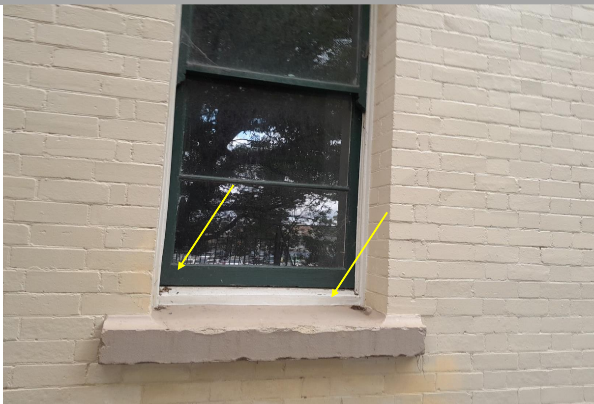
Photograph 10. Exterior, window frames – Lead containing paint systems to window frame and window frame surround as observed on [21.07.2022].
