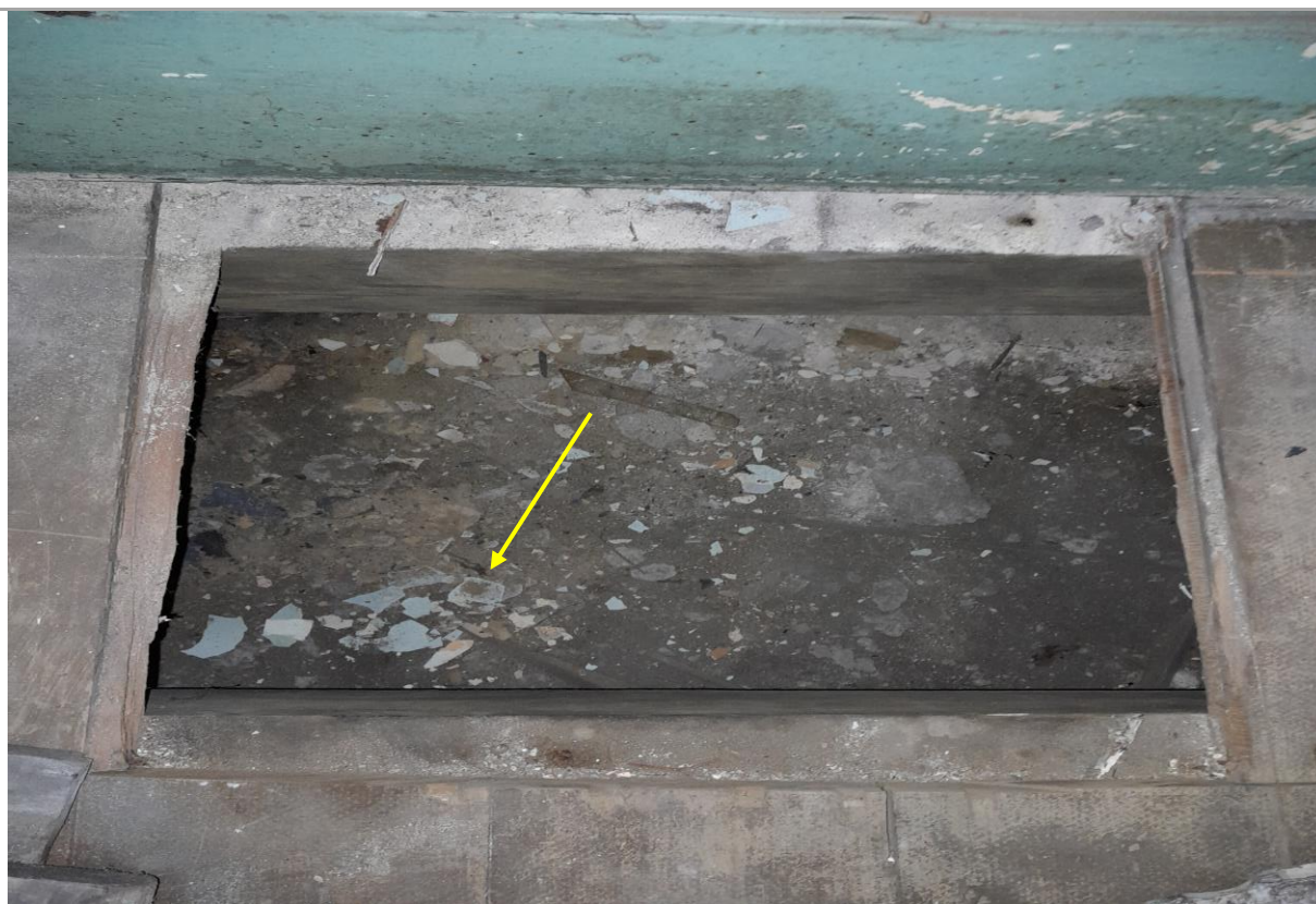
Photograph 1. Interior, subfloor – lead containing dust as observed on [04.07.2022].
