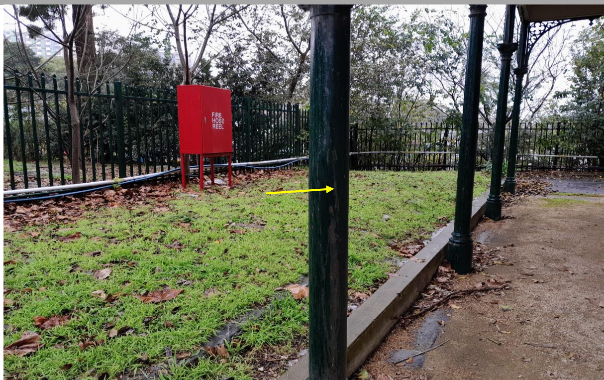
Photograph 12. Exterior, support poles – lead containing green paint system as observed on [21.07.2022].
