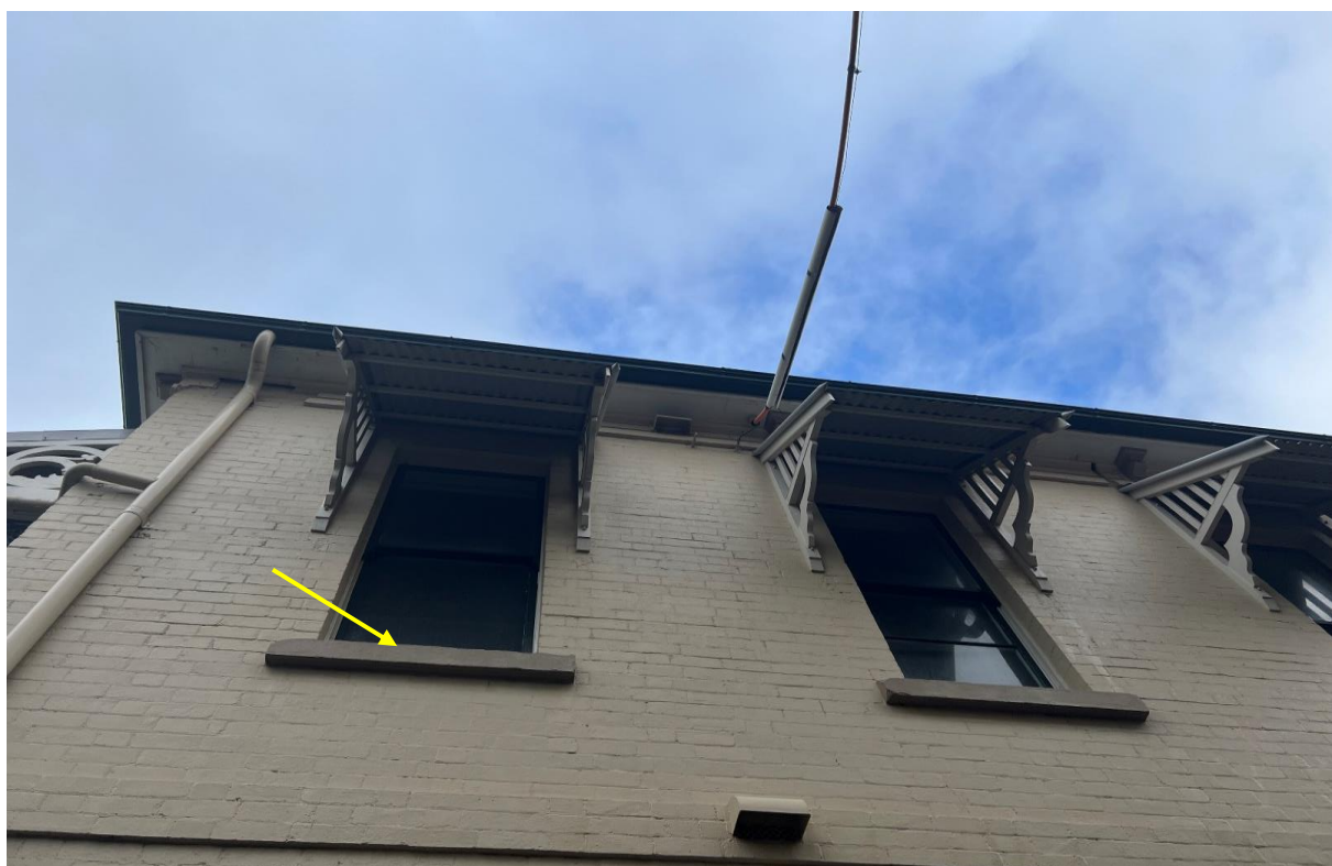
Photograph 13. Exterior, windowsills – lead containing paint as observed on [21.07.2022].
