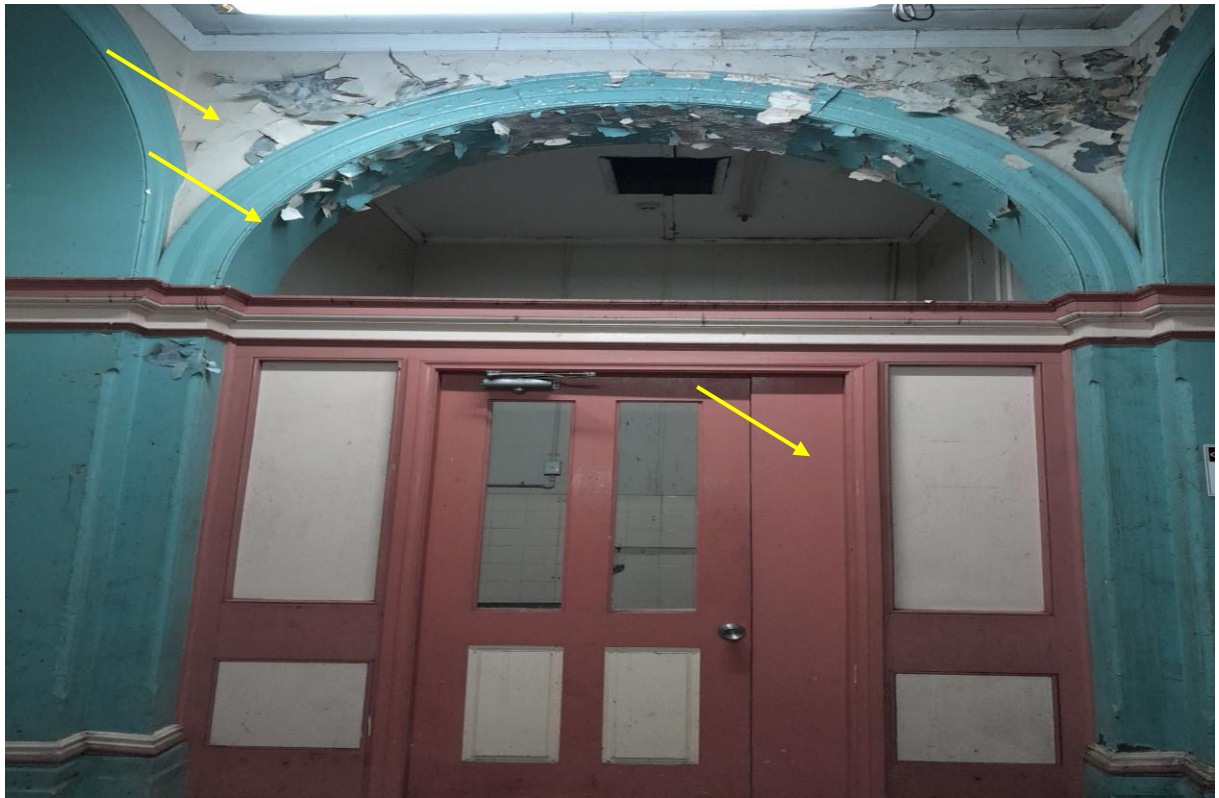
Photograph 15. Interior, level 1 hallway pink, turquoise and beige lead paint systems as observed on [04.07.2022].
