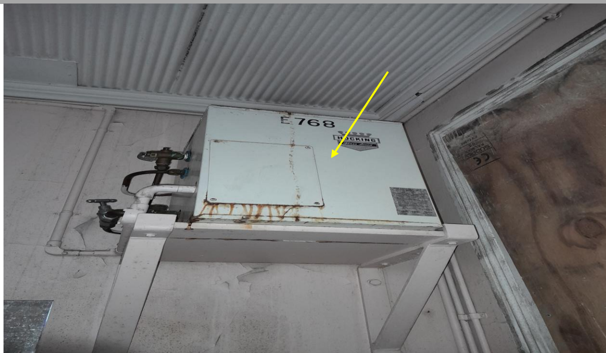
Photograph 6. Interior, level 1, ladies' toilet – Presumed SMF containing water heater as observed on [04.07.2022].
