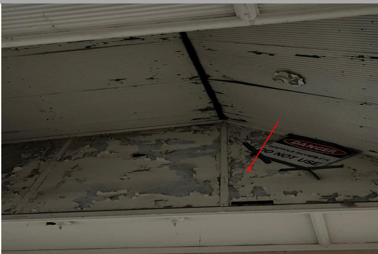
Photograph 4. Interior, level 1, room 21 – high level asbestos containing wall lining as observed on [04.07.2022].
