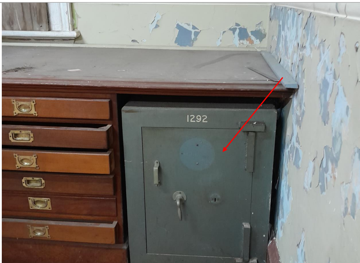
Photograph 7. Interior, ground floor, room 1 – Presumed asbestos containing internal insulation to safe as observed on [04.07.2022].
