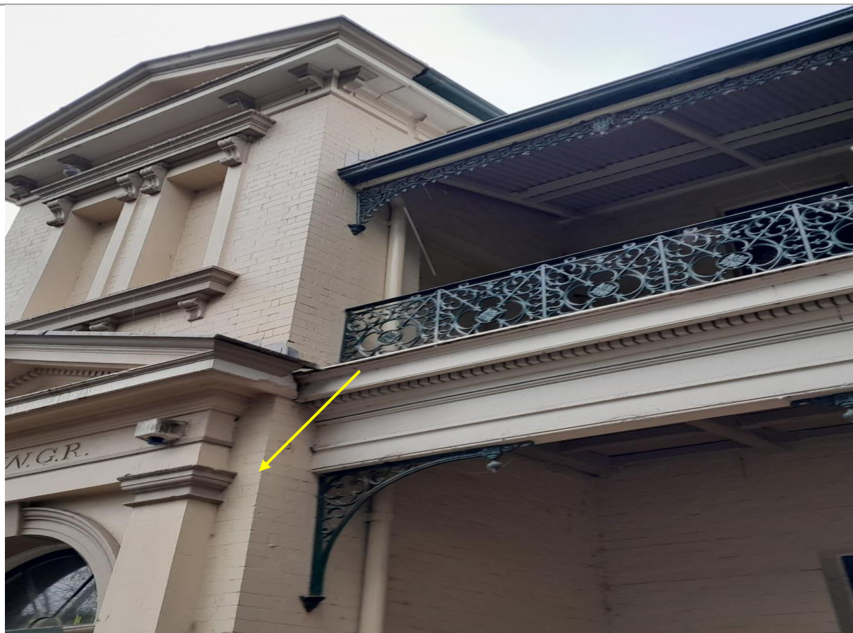
Photograph 11. Exterior, walls – Lead containing beige paint system as observed on [21.07.2022].
