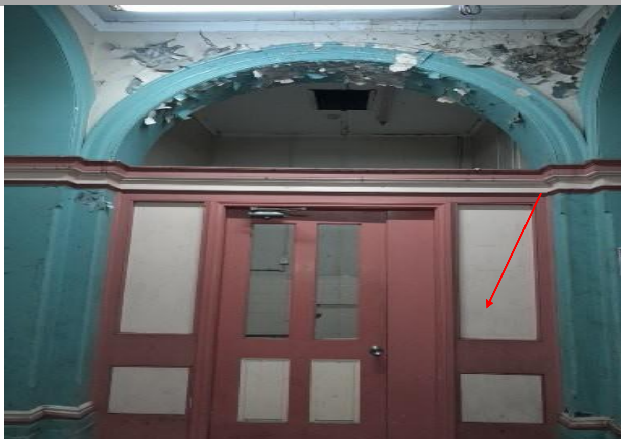
Photograph 2. Interior, level 1, north room kitchenette – asbestos containing wall lining as observed on [04.07.2022].
