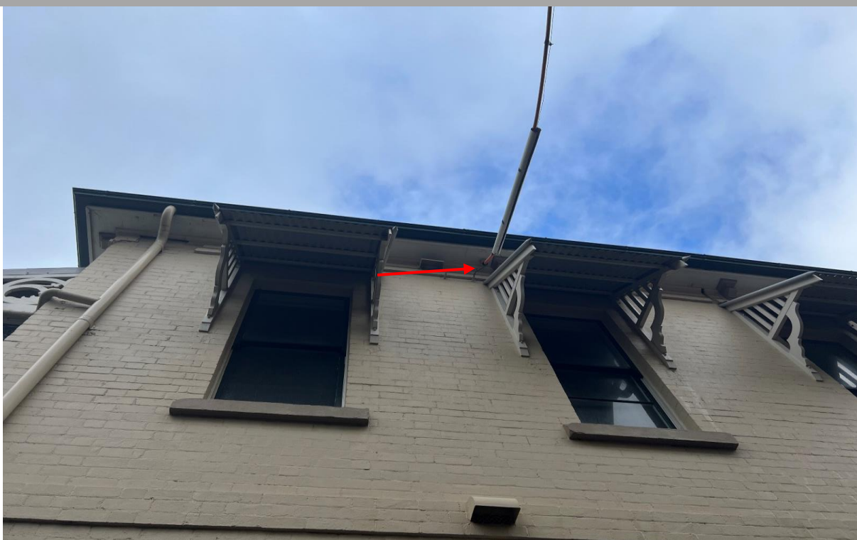
Photograph 8. Western exterior - presume asbestos containing high level flue as observed on [04.07.2022].
