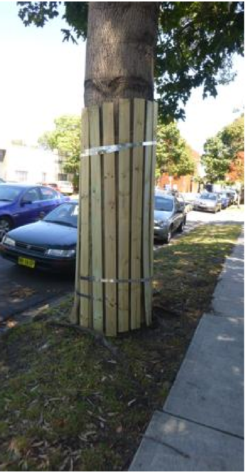
Example image of acceptable tree protection battens
