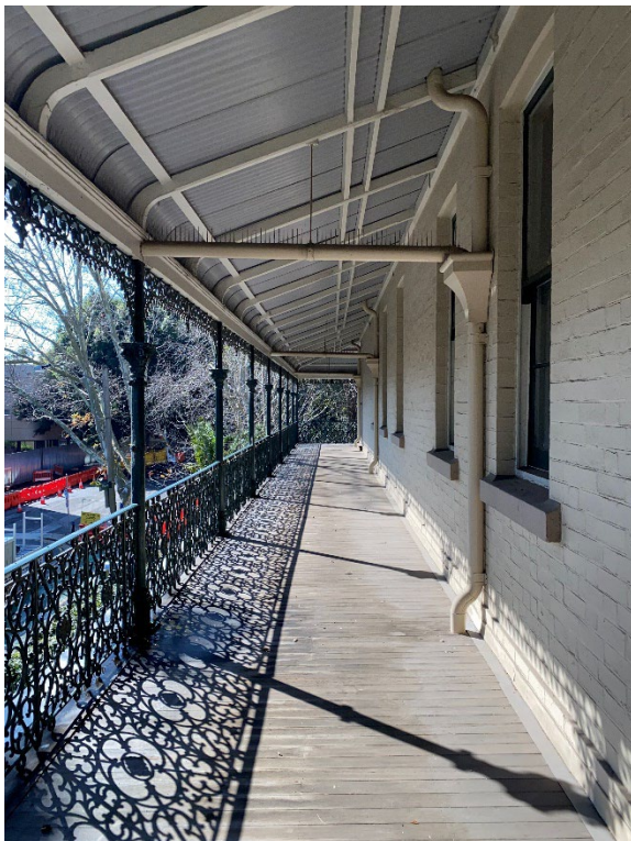
Figure 4.14: First Floor balcony showcasing the cast-iron columns and balustrade. Source: Curio, 2022.
