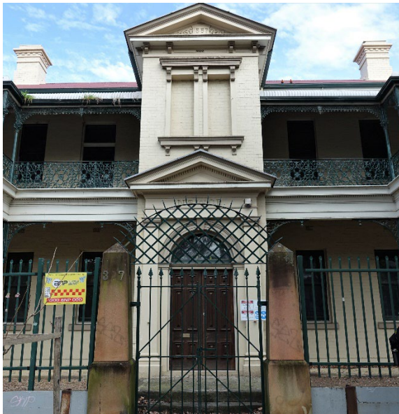
Figure 4.10: Front entry facing Wilson Street showcasing the neoclassical pediment, timber double doors and the northern fence (with likely original stone posts). Source: Curio, 2022.
