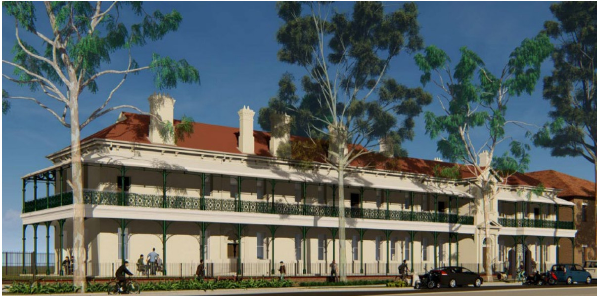
Figure 8.18: Illustrative image of the CME building along Wilson Street. The proposed glass balustrade will sit behind the cast-iron balustrade along the First Floor balconies. Source: CCG Architects, 2022.
