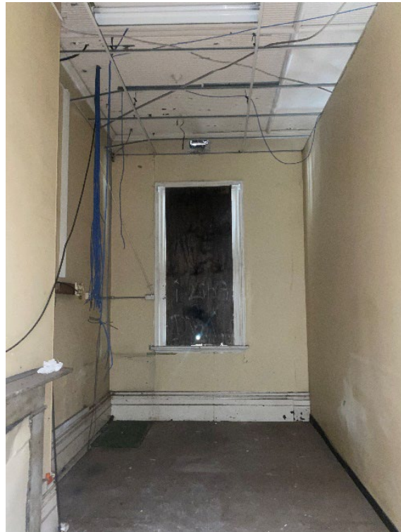
Figure 4.36: View of Room F5 currently subdivided by a plaster wall. This situation is repeated in other rooms (e.g., G21). Potential original fireplace can be seen in the bottom left corner of the image. Source: Curio, 2022.
