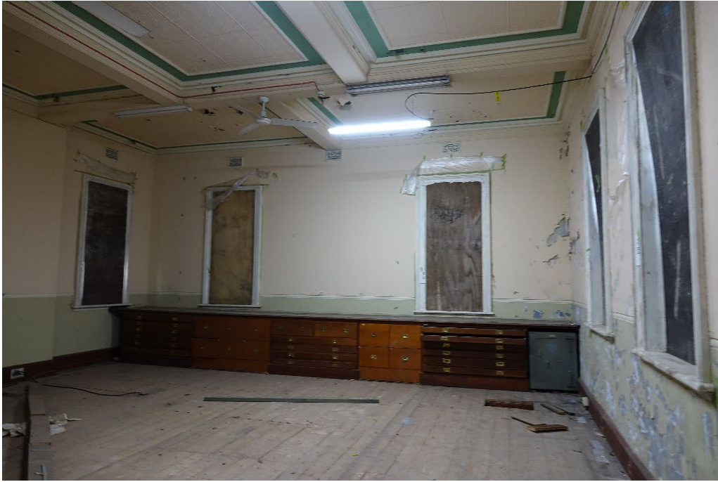
Figure 4.26: Former CME Office (G10). Built-in cabinet, safe, and detailed ceilings are unique features within this room and should be retained. Suspension files in the cabinet are made of inferior material and are likely later additions. Source: Curio, 2022.
