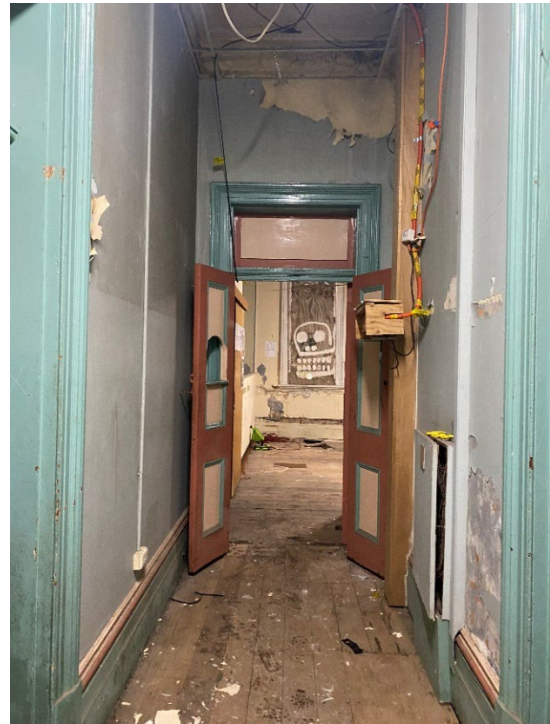
Figure 4.21: Corridor leading to the former Pay Office (G1). Double doors with pay window have been retained. Poor condition due to water damage can be seen on the ceilings, walls and floors. Source: Curio, 2022.
