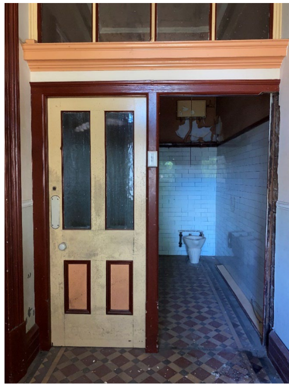
Figure 4.25: View of the former CME Toilet (G8). The tessellated tiles continue from the entry lobby (G9) and the two rooms are separated by a timber partition (western panel and frame currently missing). Original fixtures such as the toilet bowl and washbasin have been retained although damaged. Source: Curio, 2022.
