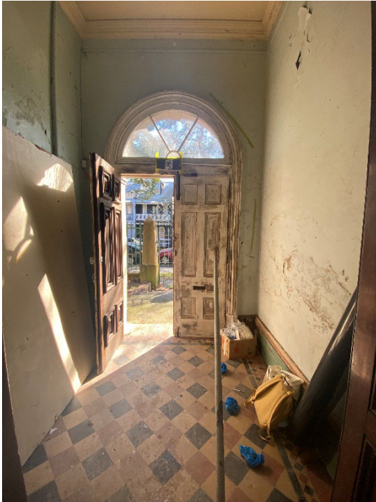
Figure 4.18: Main entry foyer (G3). Despite the poor condition of the room, original tessellated tiles, arched timber doors, and skirting details have been retained. Source: Curio, 2022.
