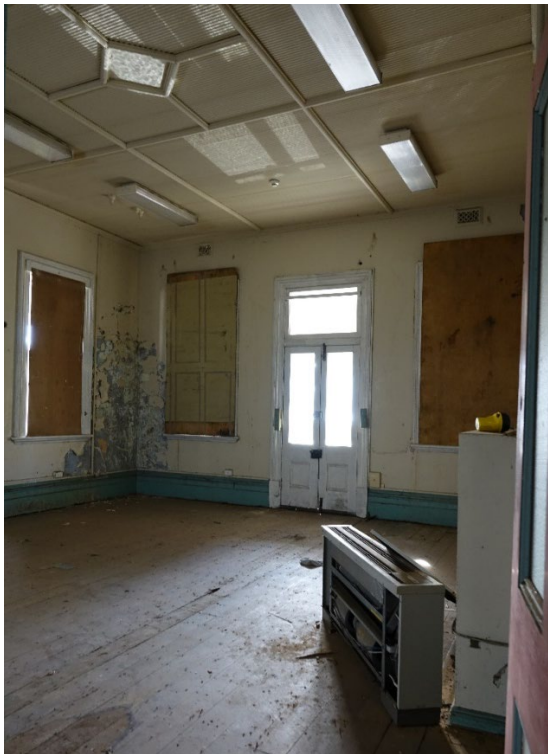
Figure 4.35: View of Room F1 showing double doors leading to the northwest balcony, timber floors, skirting and detailed ceiling. Source: Curio, 2022.
