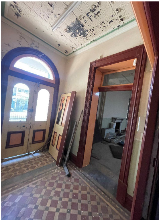
Figure 4.24: Secondary entry lobby (G9) leading to the former CME Office (G10). Original tessellated tiles, double doors, pressed metal ceiling, timber architraves, skirting and moulding details remain visible. Source: Curio, 2022.
