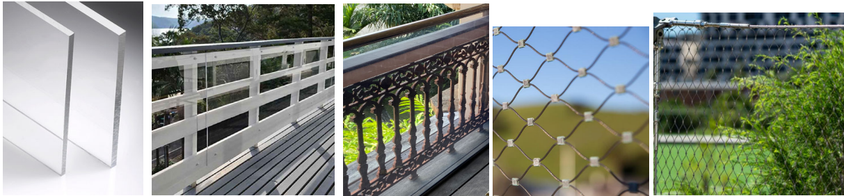
Figure 07. Perspex screening and tensile mesh barriers inferior in cleaning & maintenance and structural point of views and lack of integration with the original balustrade
