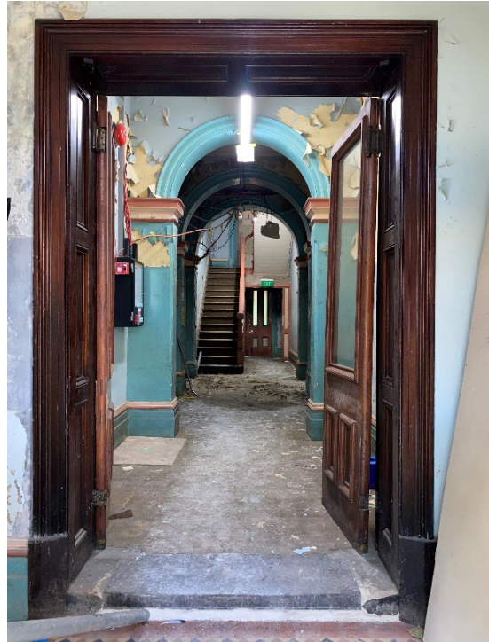
Figure 4.19: View from the main entry foyer to the circulation area (G3B/G3A). The timber double doors, skirting and moulding details remain visible. Source: Curio, 2022.
