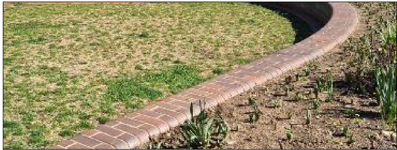
Brick Wall with Bullnose on Front and Back Leading Edge
