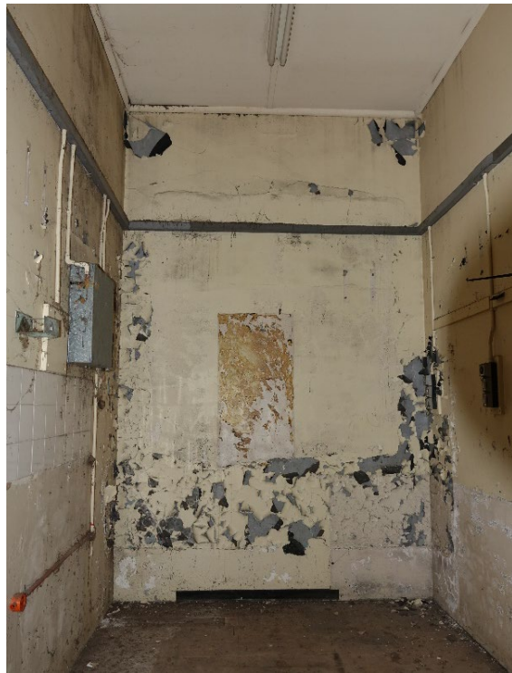
Figure 4.32: Photographic Dark Room (F3B). This room was later modified to accommodate the dark room and, therefore, the original windows on the northern wall have been covered. Source: Curio, 2022.
