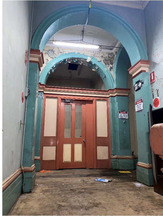
Figure 4.30: View from the staircase towards the circulation and enclosed room (F3A). The timber partition was a later addition to the site and is assessed as an intrusive element. Source: Curio, 2022.
