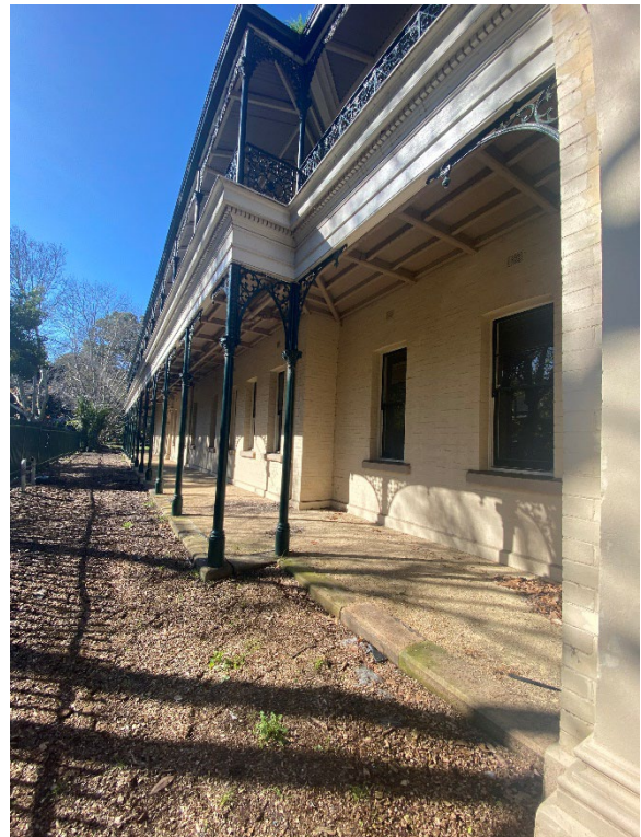
Figure 4.15: Ground Floor verandah showcasing the cast-iron columns and the decomposed granite flooring with sandstone edges. Source: Curio, 2022.
