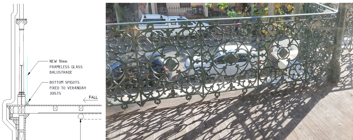
Figure 08. Detail of frameless glass screen behind the existing lattice ironworks balustrade.
