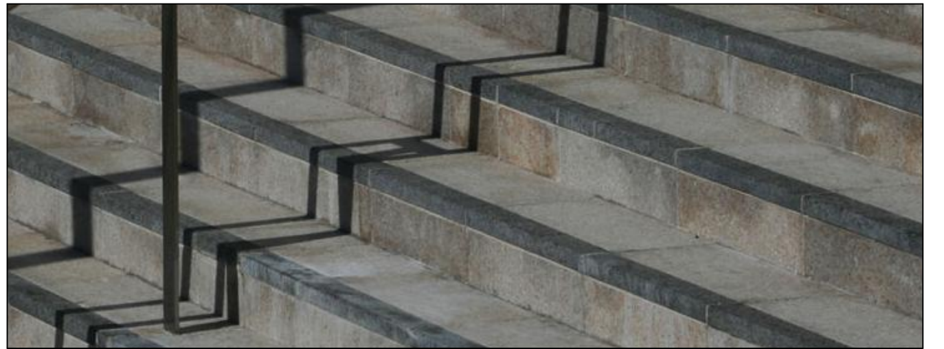
Contrasting Nosing Detail
