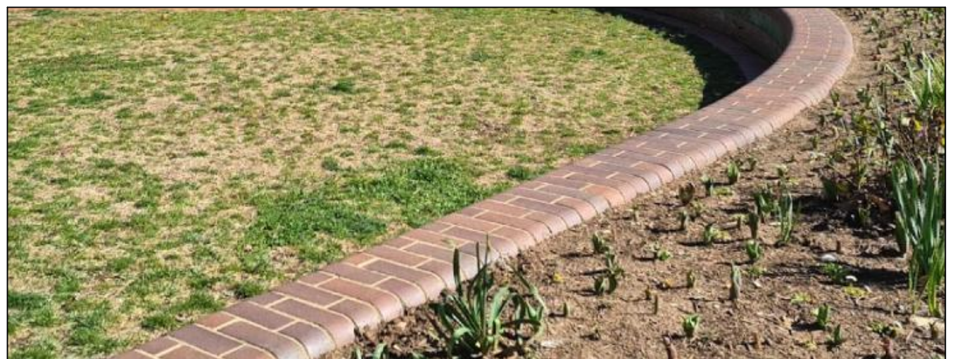
Brick Wall with Bullnose on Front and Back Leading Edge
