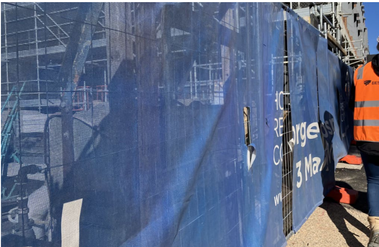
Shade cloth installed on ATF in place of hoarding.
