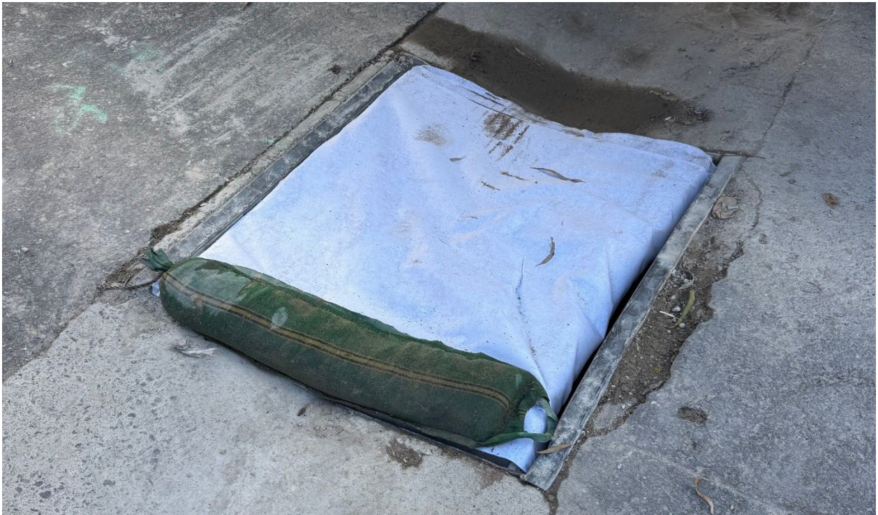
Close out of Site Observation OBS-01: Control measures reinstated at link bridge area.
