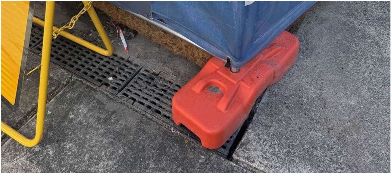
Close out of Site Observation OBS-01: Control measures reinstated at Kensington Street.
