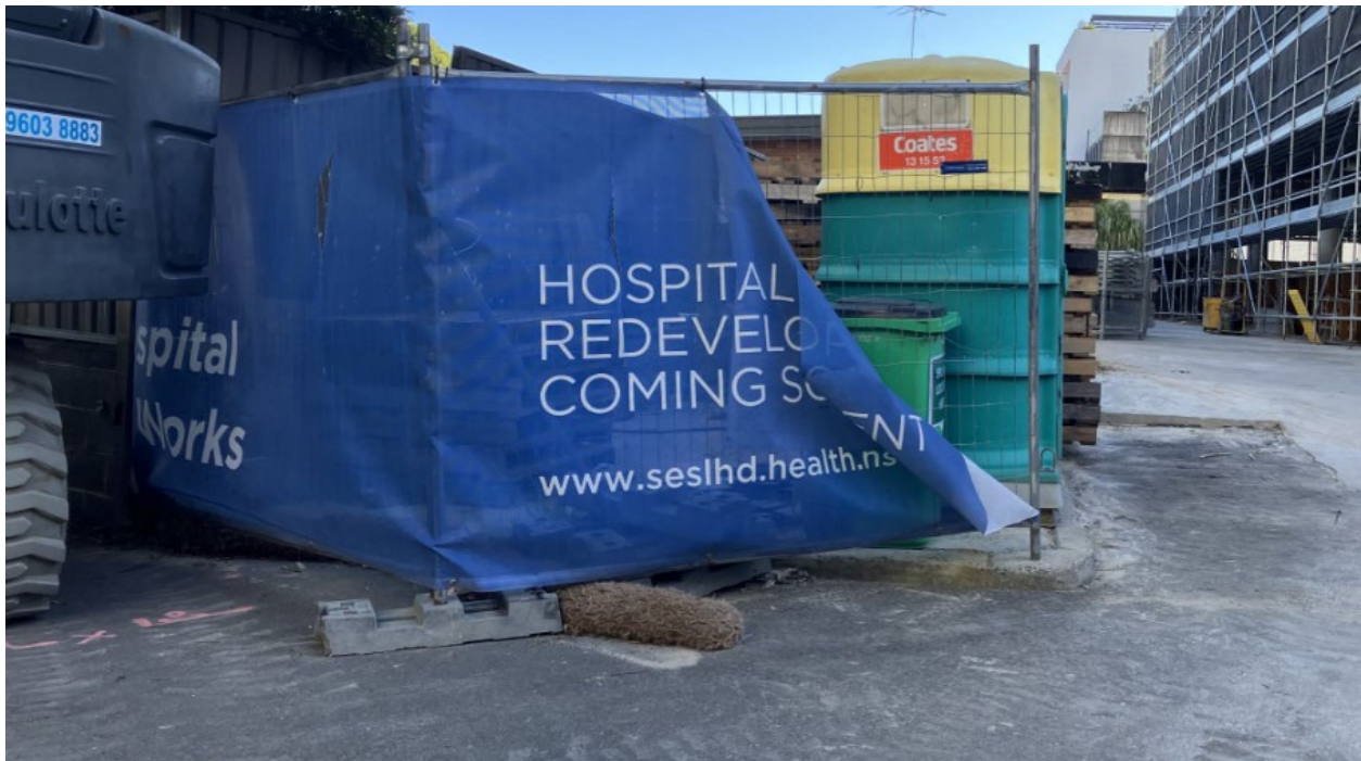
Coir logs in place at low point areas
