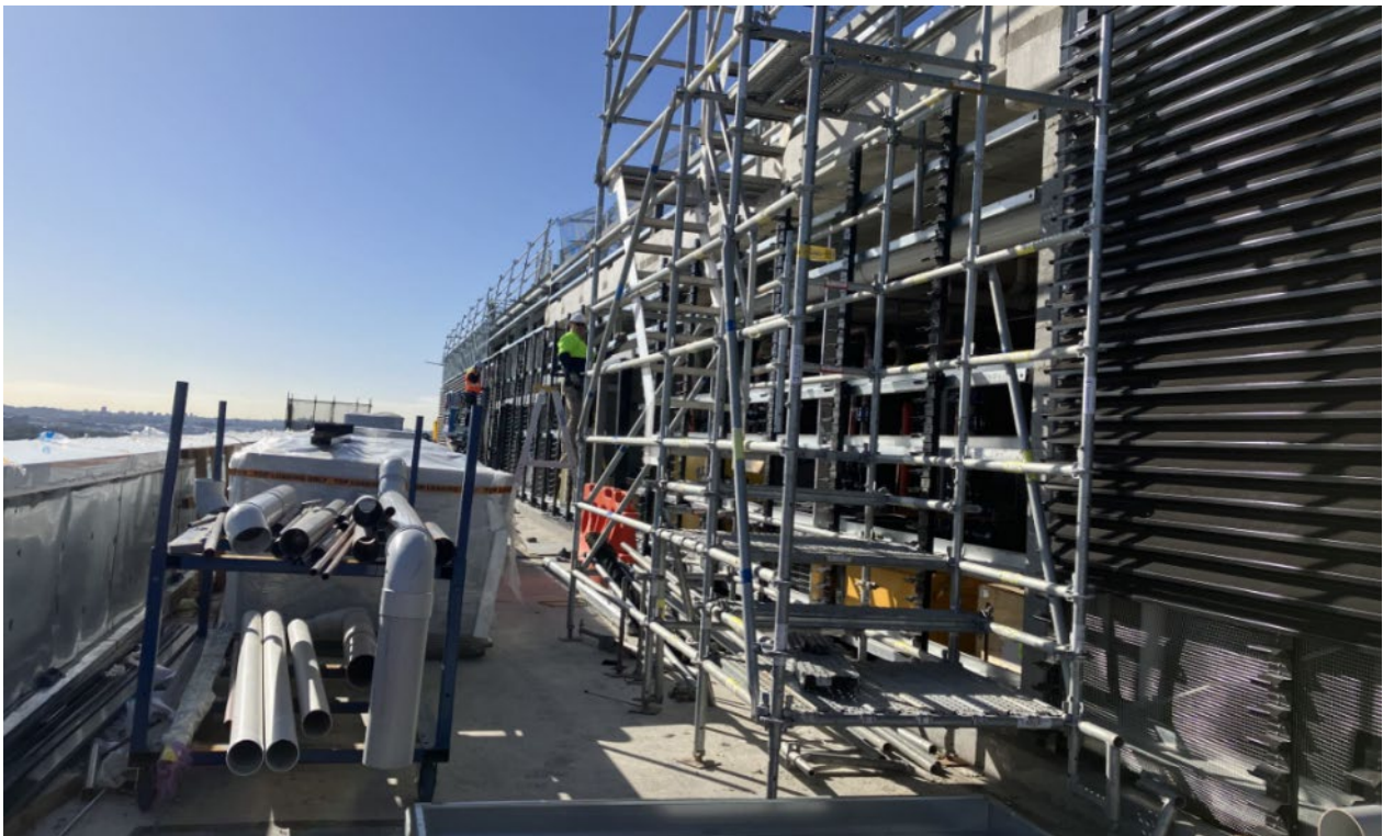
Rooftop works (level 8) involving façade installation.
