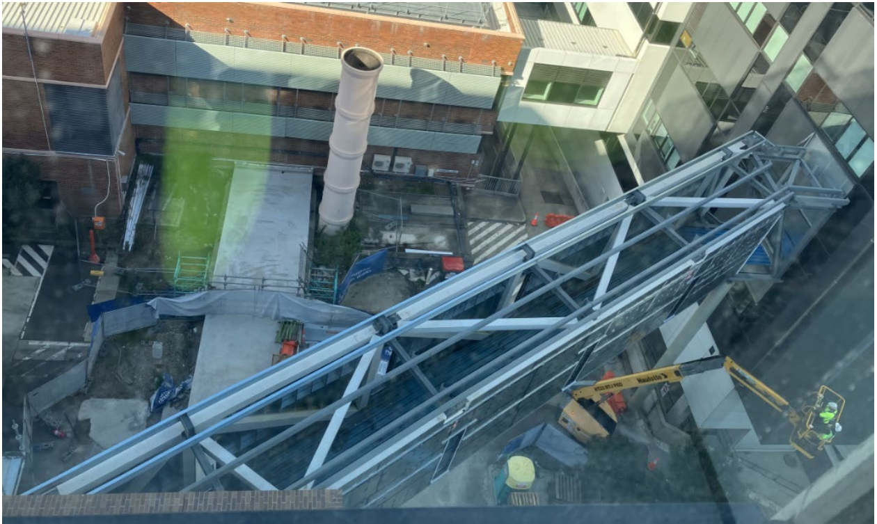
View looking down onto link bridge.
