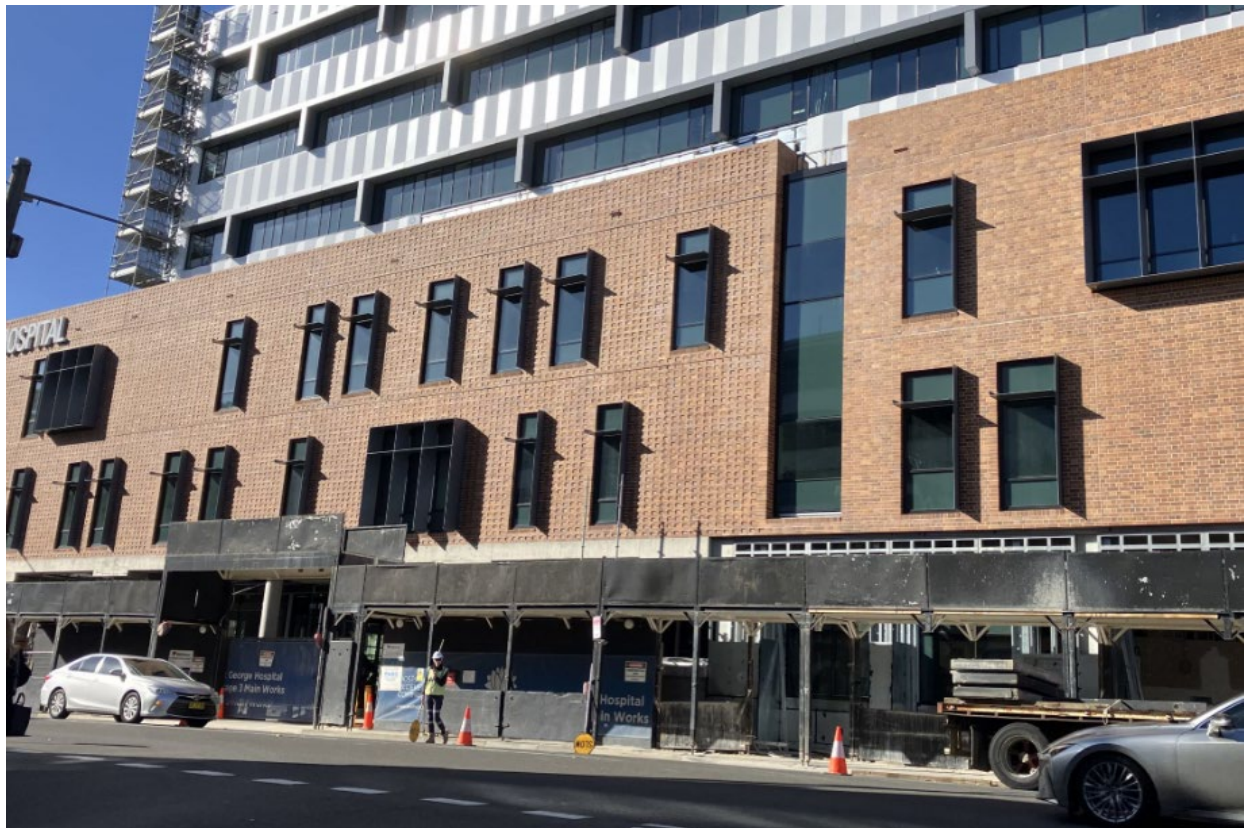
External of building at Kensington Street. Traffic controls in place.
