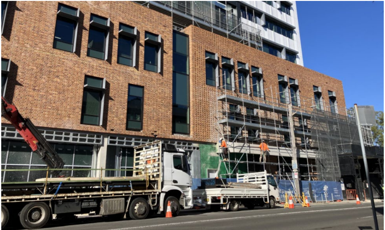
Vehicles parked in designated Works Zone at Kensington St.
