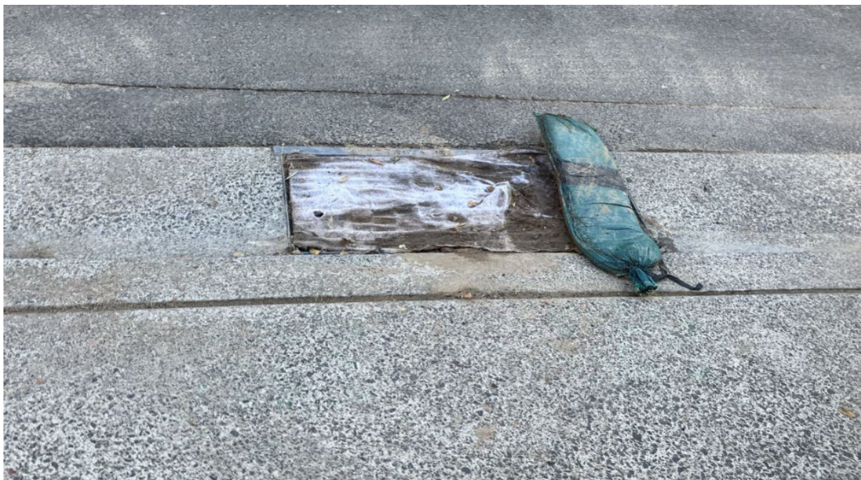
Pit draing protection on Kensington Street.
