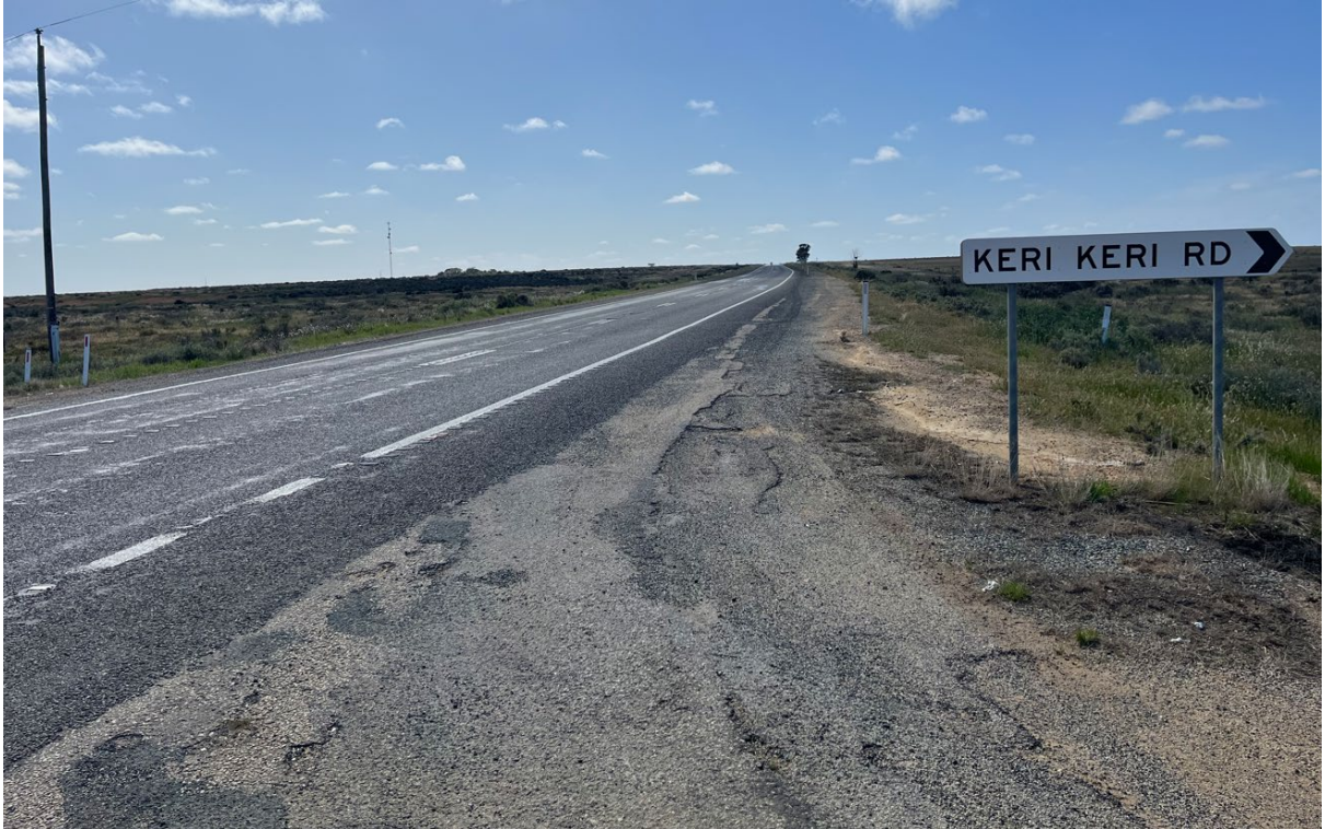
Figure 2.6: Sturt Highway at Keri Keri Road Intersection (looking east)
