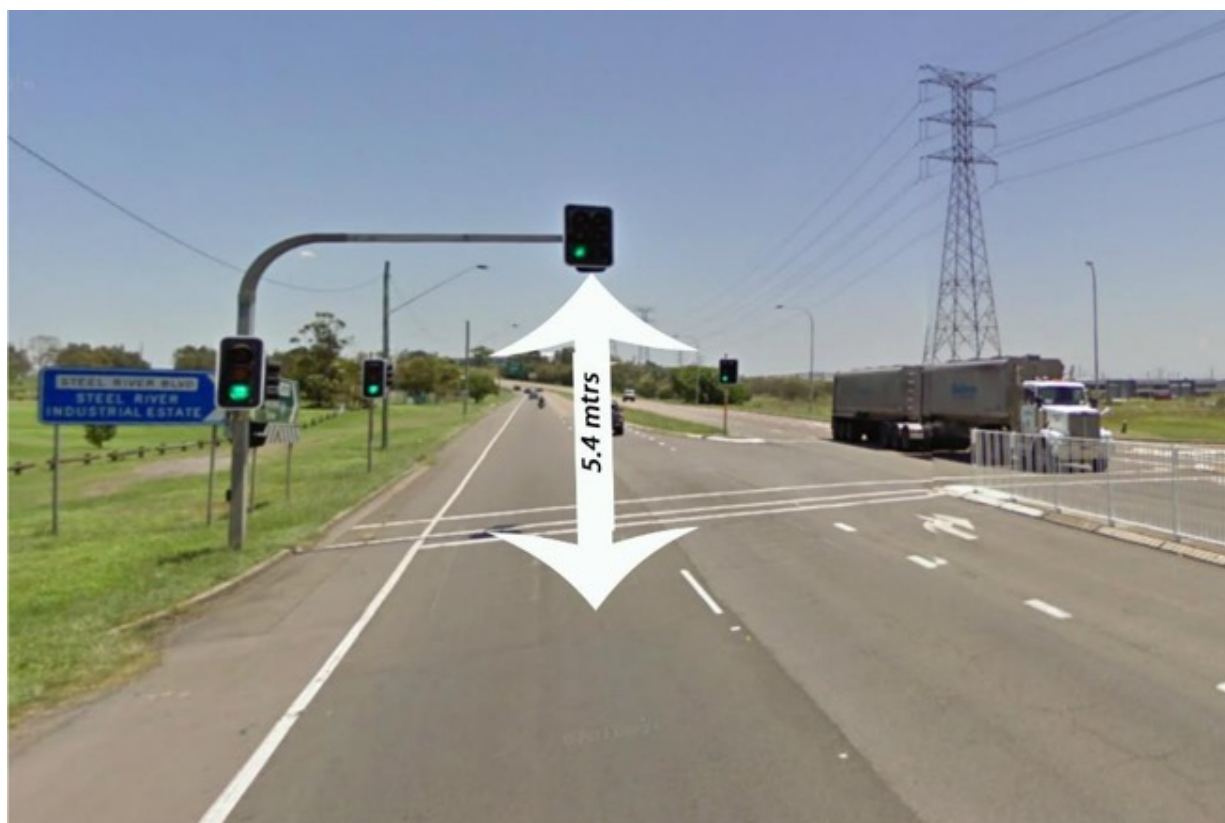
Figure 17 - Standard overhanging Traffic signals Mayfield to Hunter Expressway
