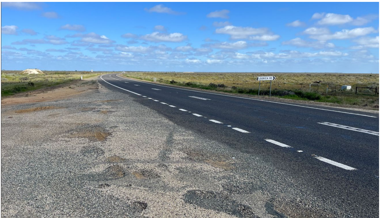
Figure 2.7: Sturt Highway at Keri Keri Road / Loorica Road Intersection (looking west)
