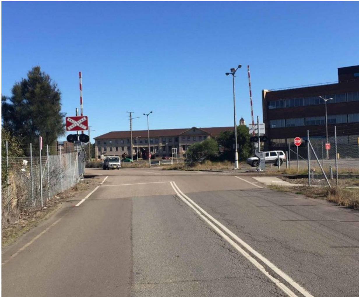
Figure 15 - Rail crossing over Selwyn Street
