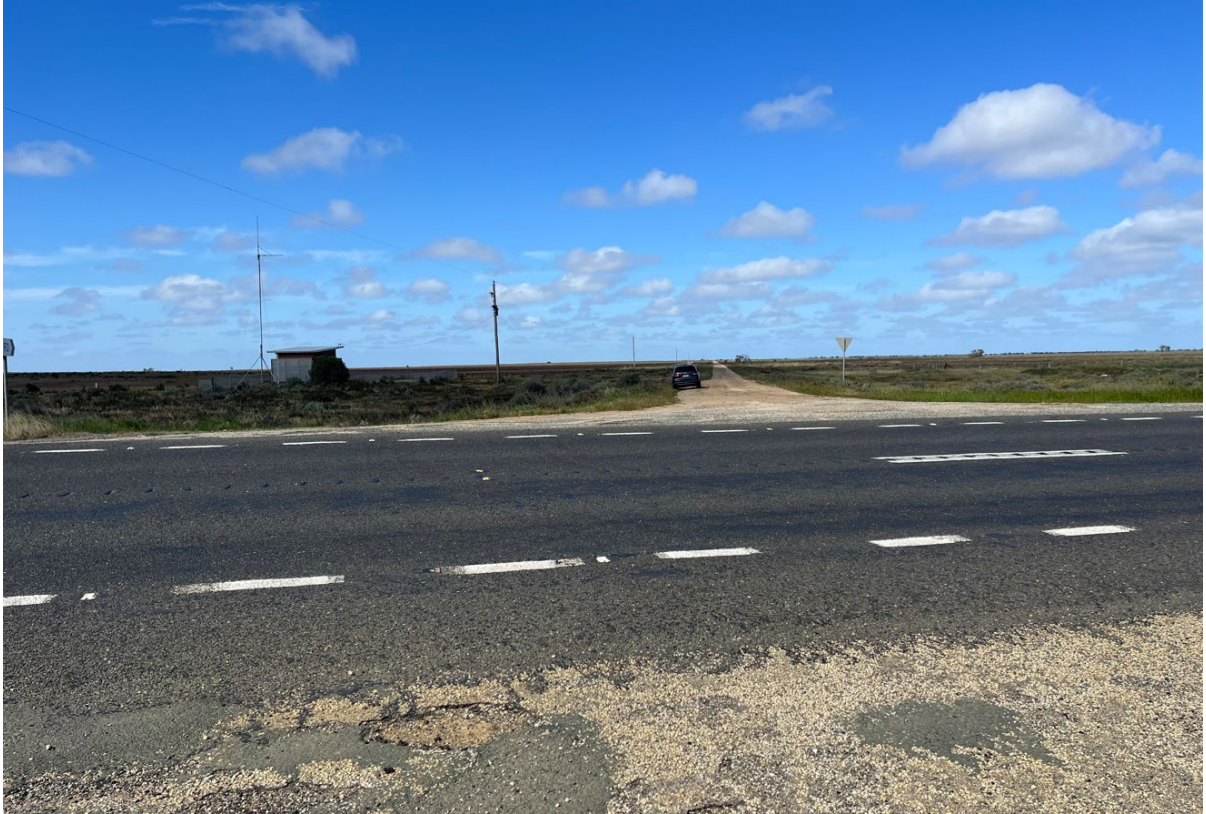
Figure 2.8: Sturt Highway at Keri Keri Road Intersection (looking south from Loorica Road to Keri Keri Road)
