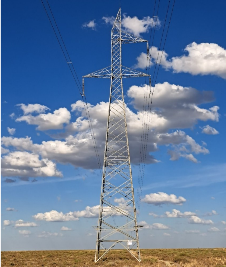
FIGURE 3-10 TYPICAL STEEL LATTICE TOWER STRUCTURE
