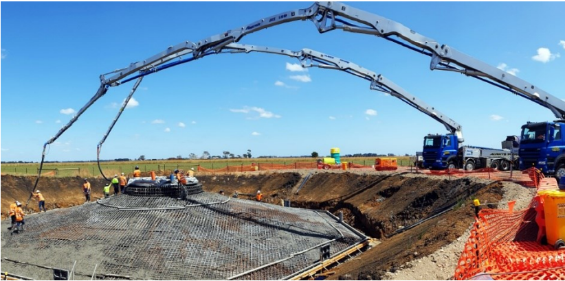
FIGURE 3-7 TYPICAL FOUNDATION BEING CONSTRUCTED
