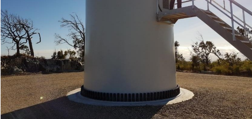
FIGURE 3-8 TYPICAL FOUNDATION POST-CONSTRUCTION
