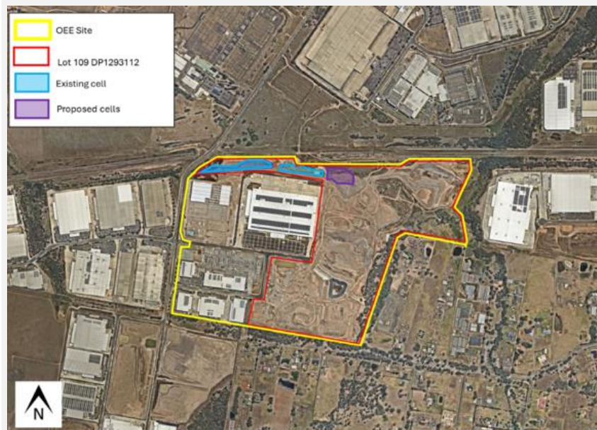
Figure 30: Aerial view of the broader site (outlined in yellow) and the three containment cells (Source: Nearmap)
