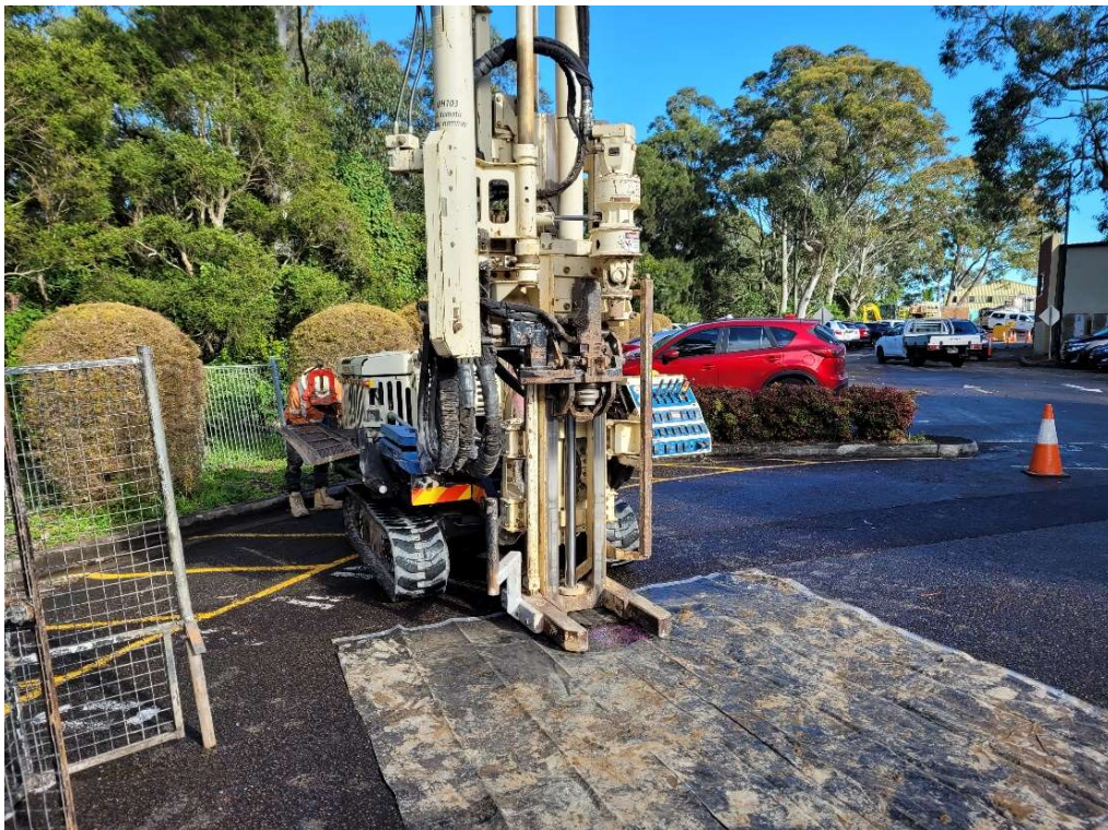
Photo 6: Rig used for drilling
