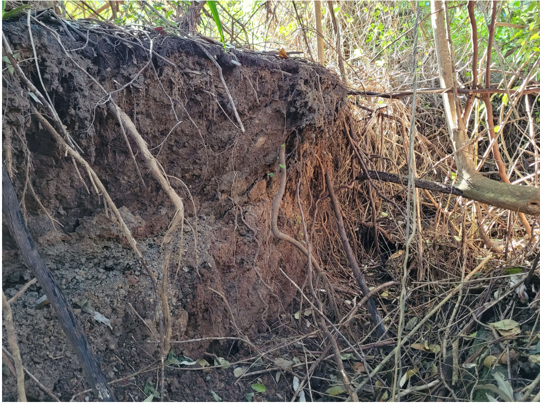
Photo 9: Exposed cut face at slope
